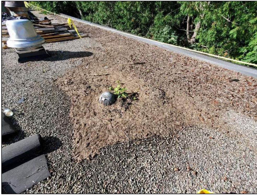
Debris around drains on lower, gravel and tar roof.
