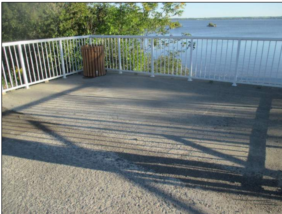
Severe scaling of north end deck top.
