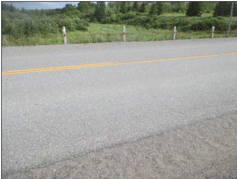
Transverse cracking in wearing surface.
