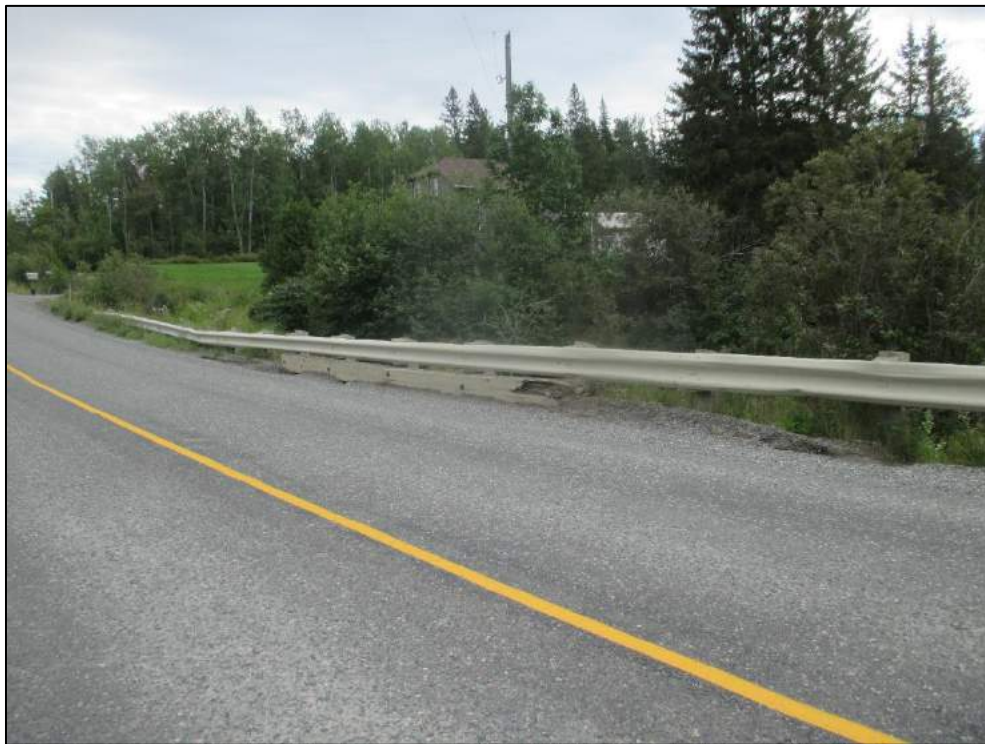
Collision damage and rotted curb at south.
