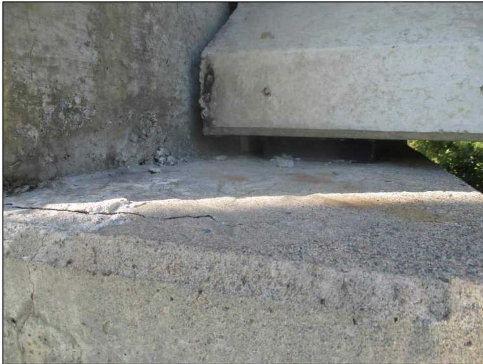
Crack, delamination at bearing seat and honeycombing of ballast wall.
