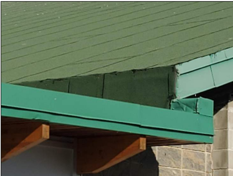
Damaged asphalt at south of building, flat roof.
