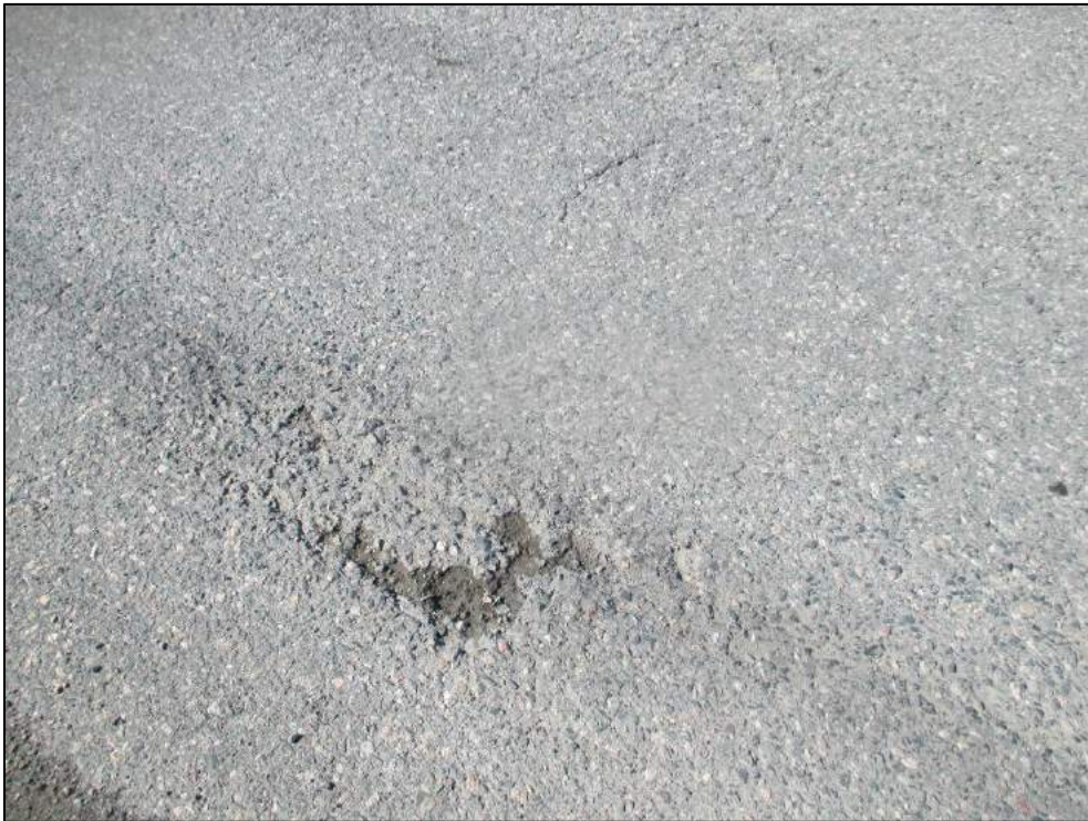
Bottom up defect.
