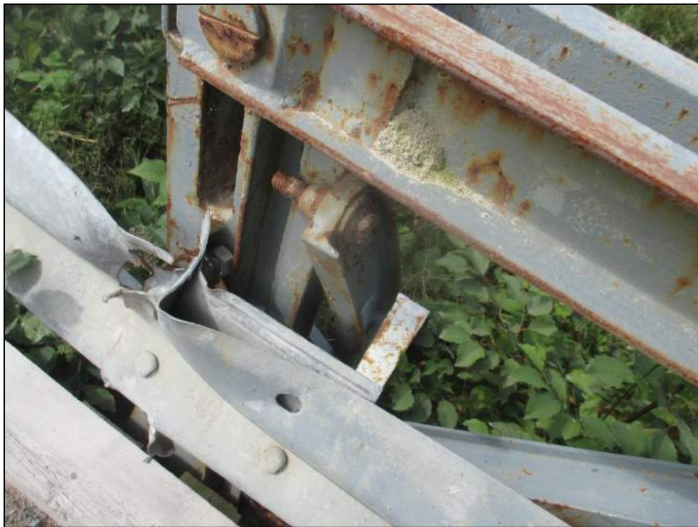
Impact damage on guidrail, damaged bracing at southwest.
