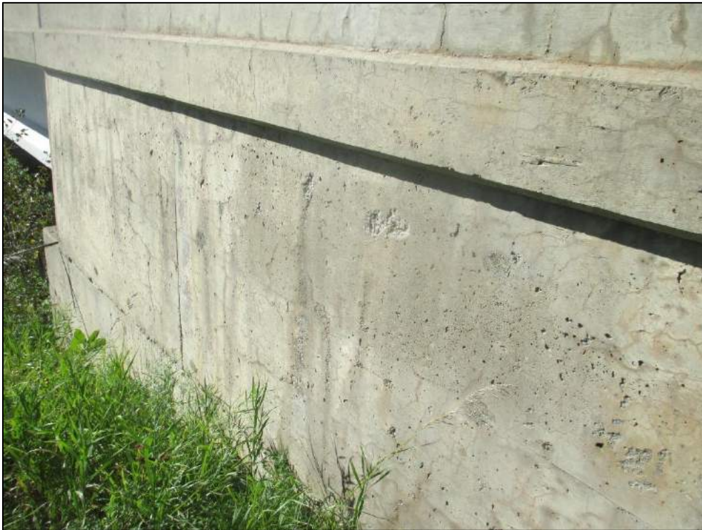
Map cracking, bugholes in southeast wingwall.
