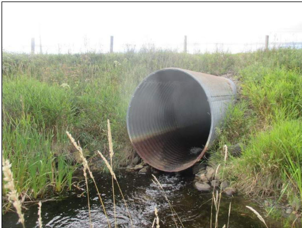
Severe undermining of north barrel end due to perforated bottom.
