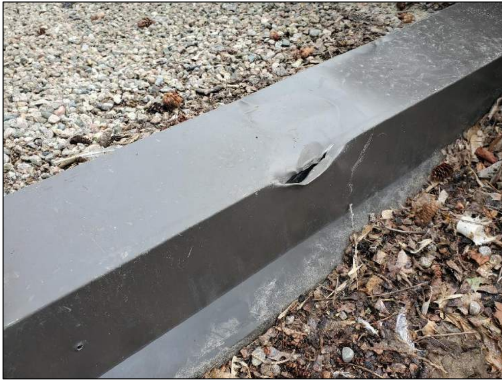
Damaged flashing at lower gravel roof.
