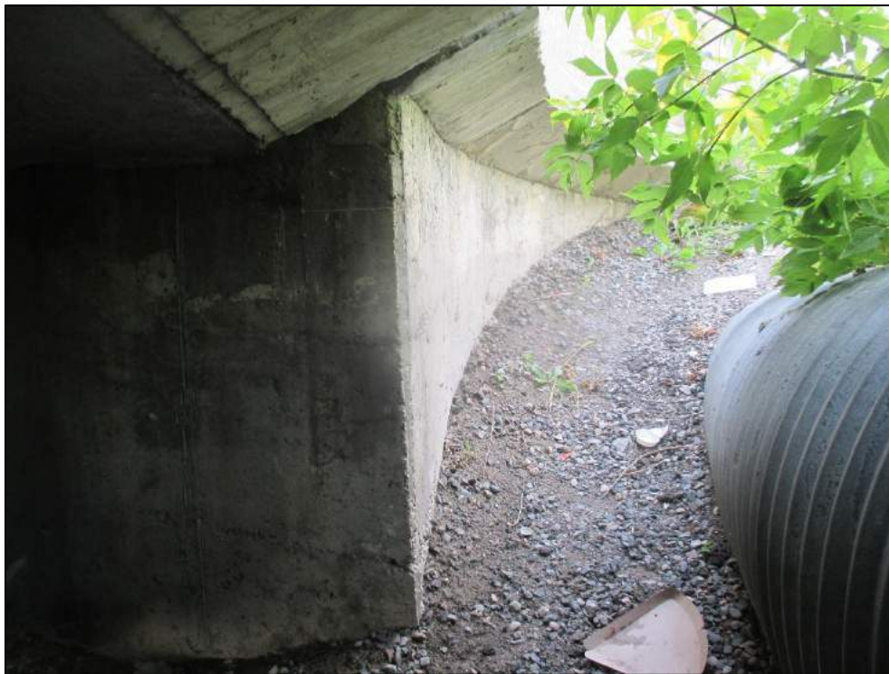
Honeycombing at southwest wingwall and ballast wall.
