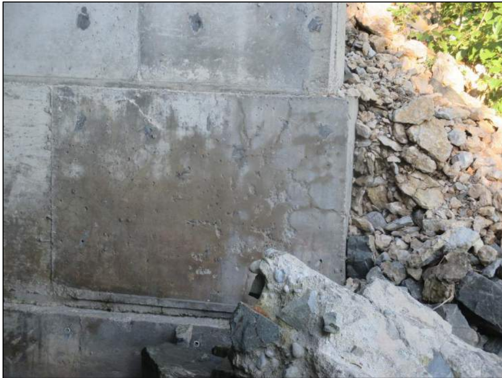
Scaling and map cracking at northwest wall.
