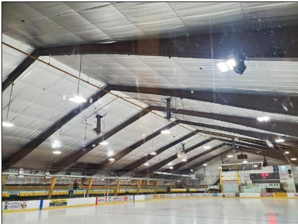
Glulam beams and insulation on interior of roof.
