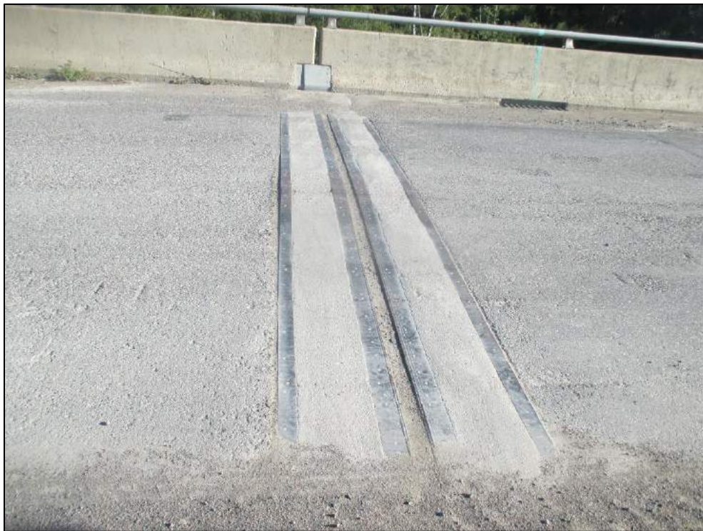
Sand in expansion joint, light scaling of concrete end dams.
