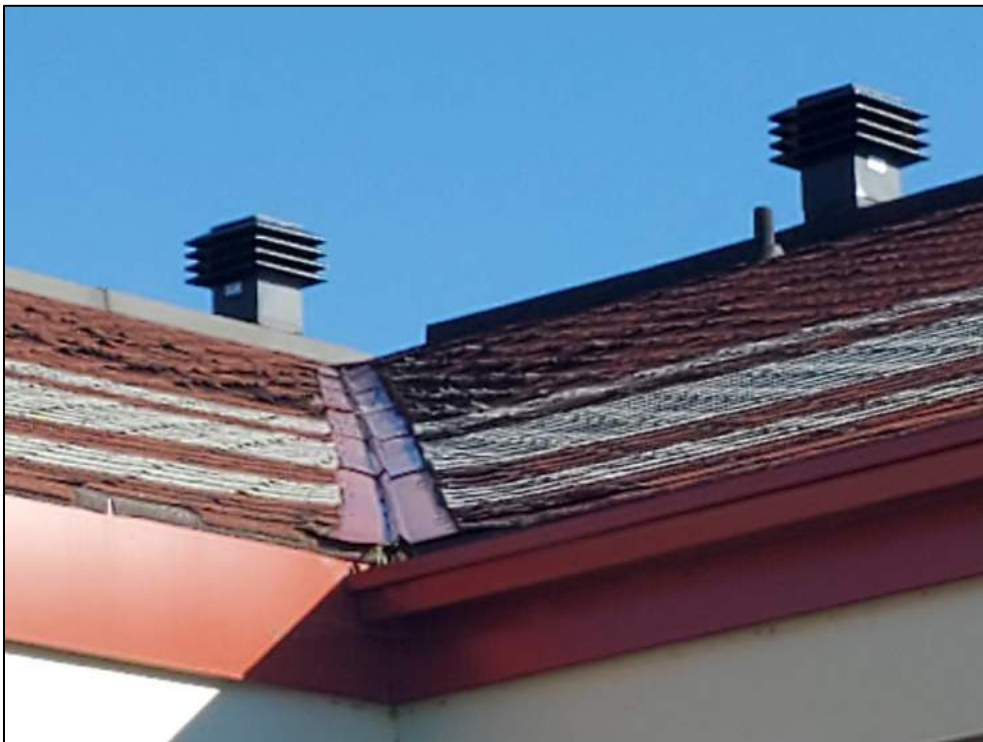
Extensive curling and damage to shingles.
