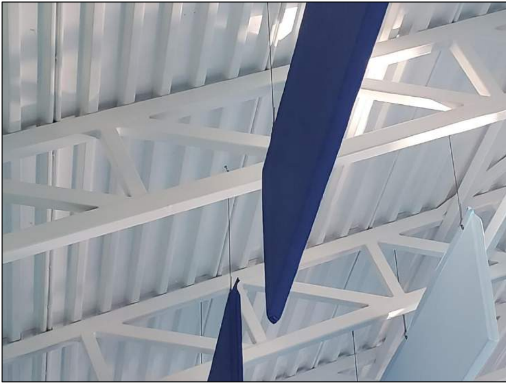
Painted decking and steel joists on roof of pool area (typ.).
