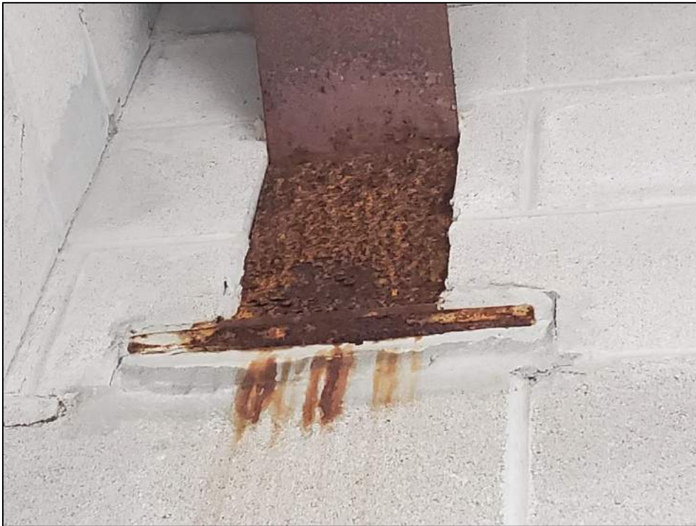
Moisture staining due to condensation and severe corrosion at girder ends in filter room.
