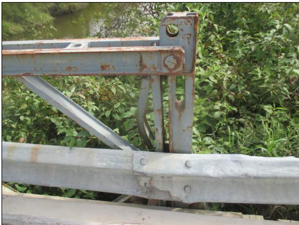
Damaged bracing at southeast.
