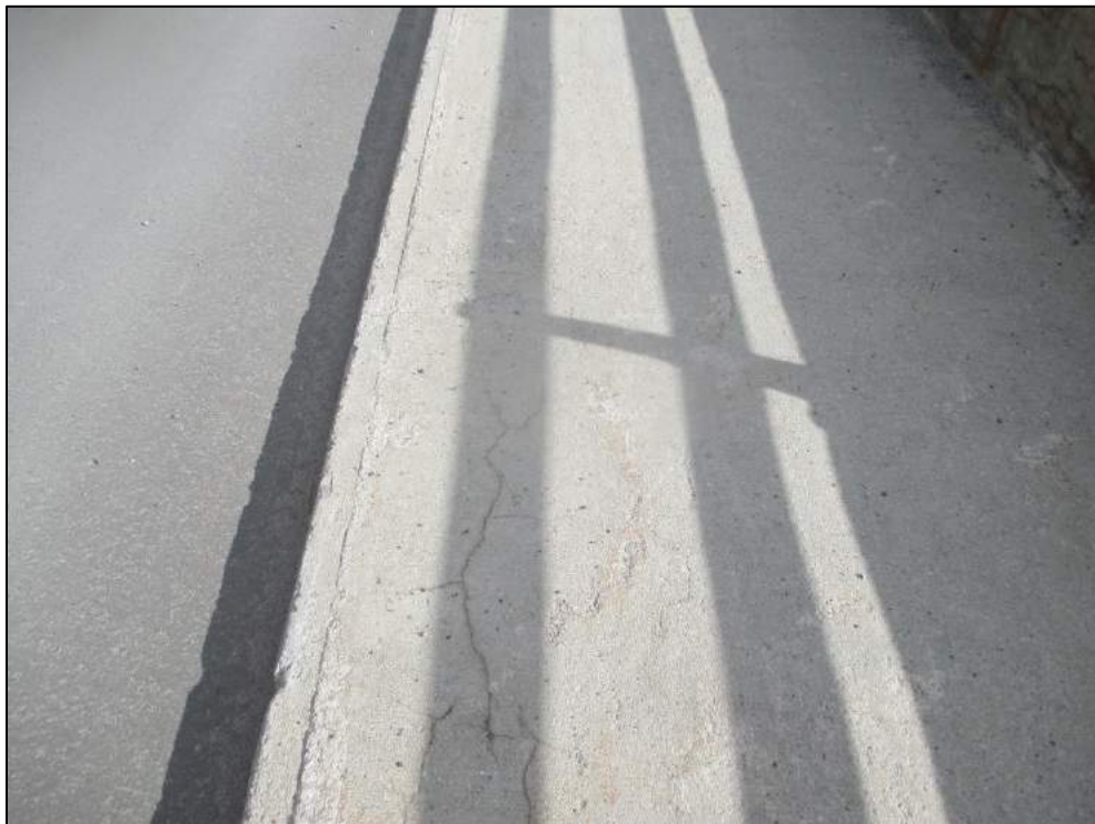
Cracking on sidewalk.
