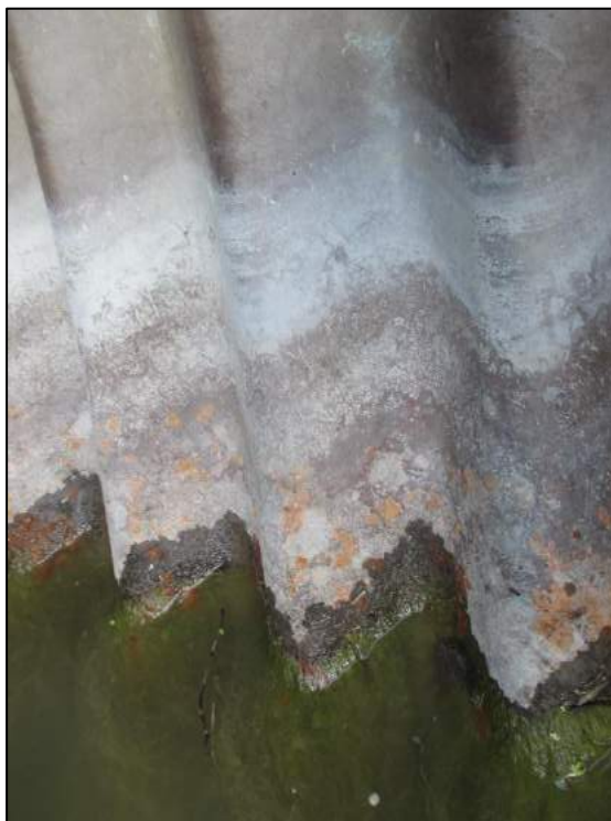
Light scaling at waterline
