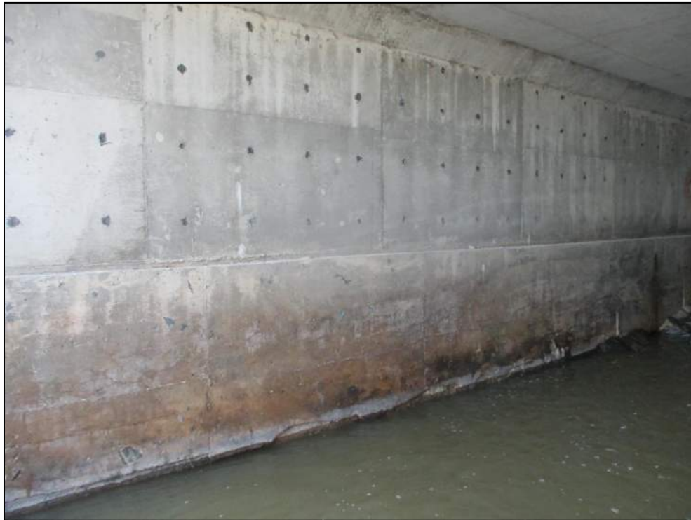
Severe scaling, undermining due to scouring action at northeast.
