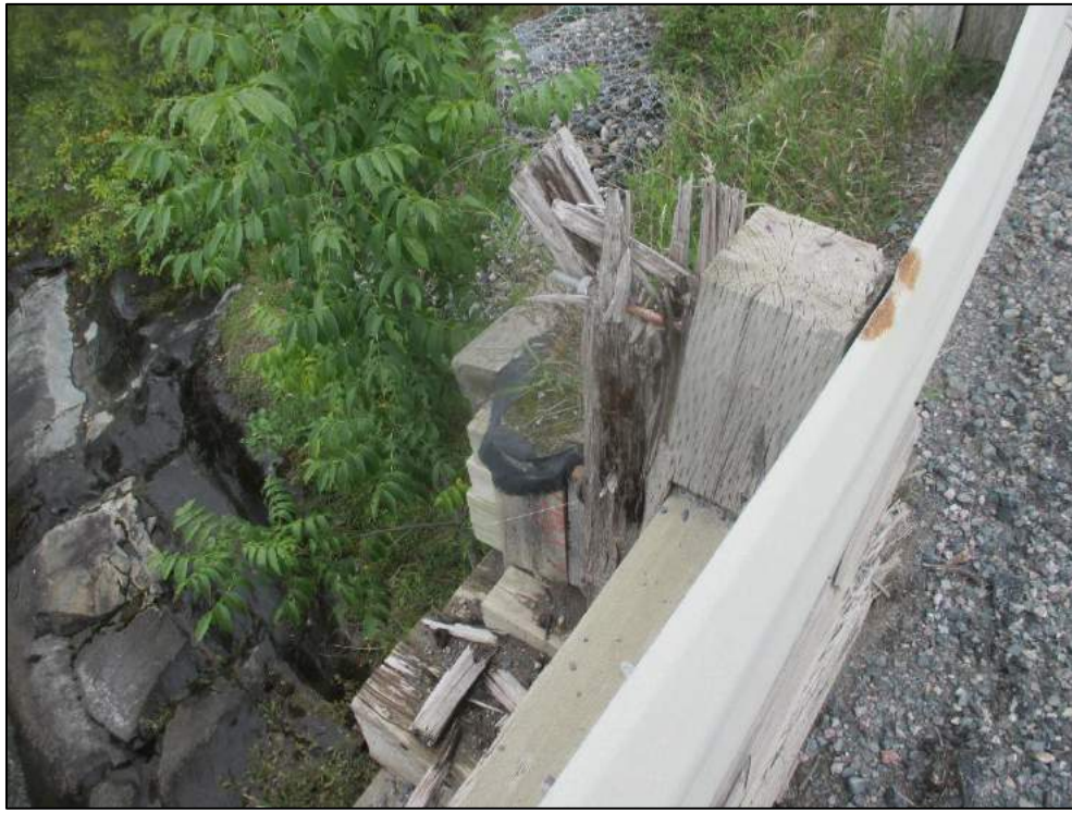
Rotted post with severe section loss at northeast.
