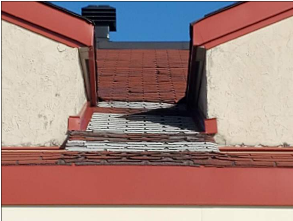
Deteriorated shingles at southeast.
