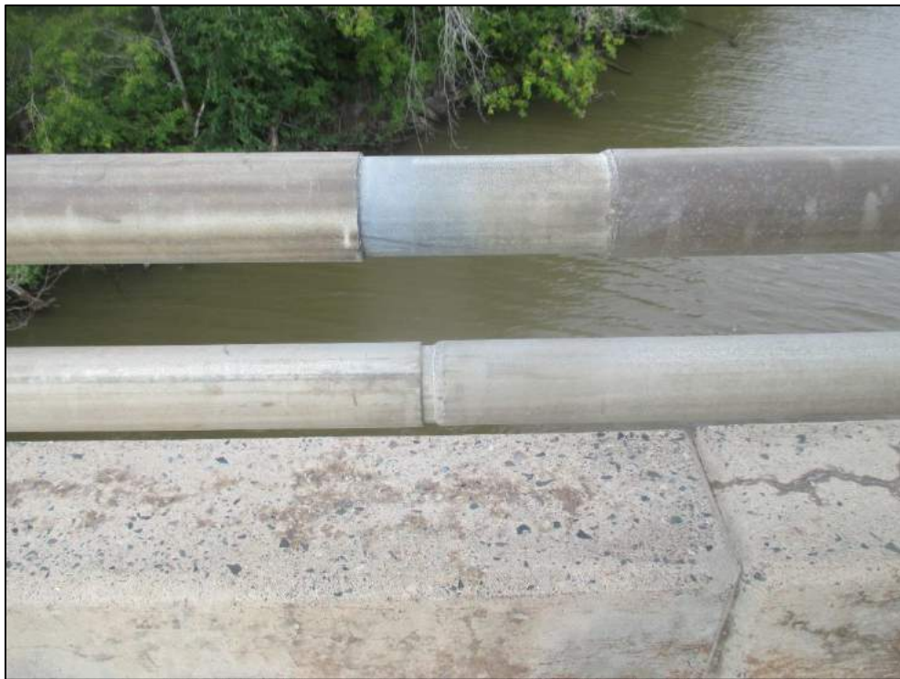
Excessive gap due to short handrail section at southwest.
