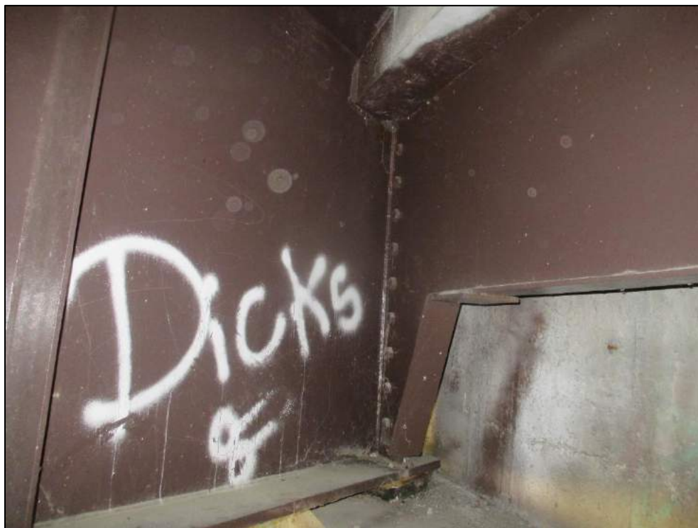
Girder end, corrosion at bearing seat.
