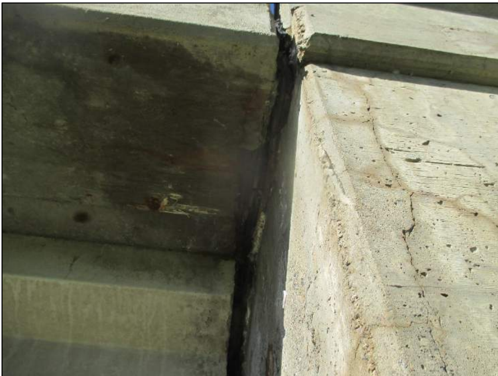
Crack in southeast wingwall, evidence of joint leakage at east abutment.
