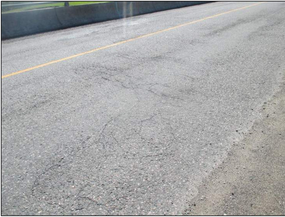
Map cracking on deck wearing surface.
