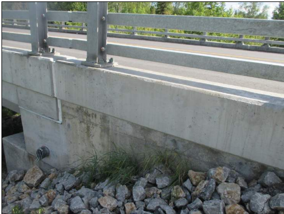
Northwest wingwall with narrow pattern cracking, bugholes.
