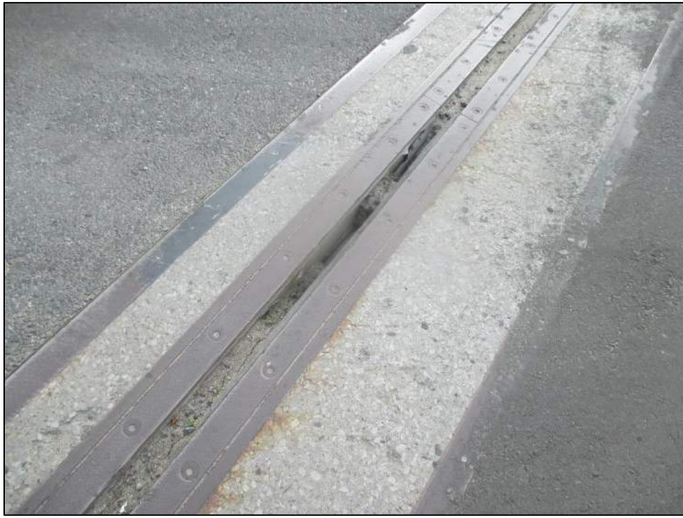
Torn seal and joint filled with sand at north.
