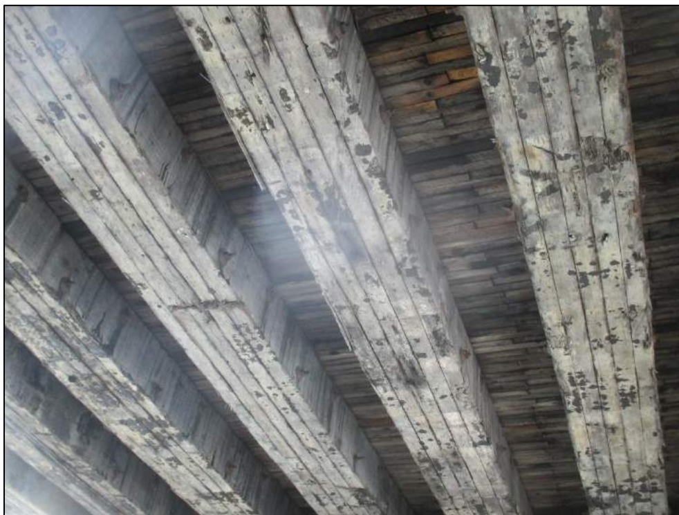
Severe checks, light rot of timber beams.
