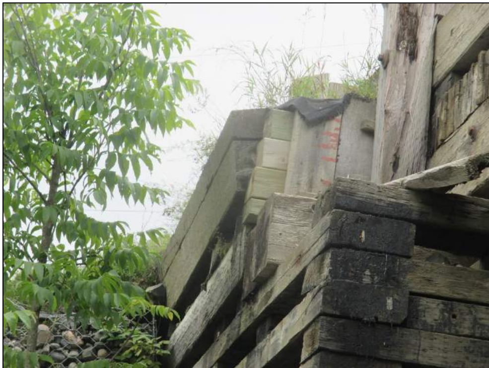
Rotated wingwall at northeast.
