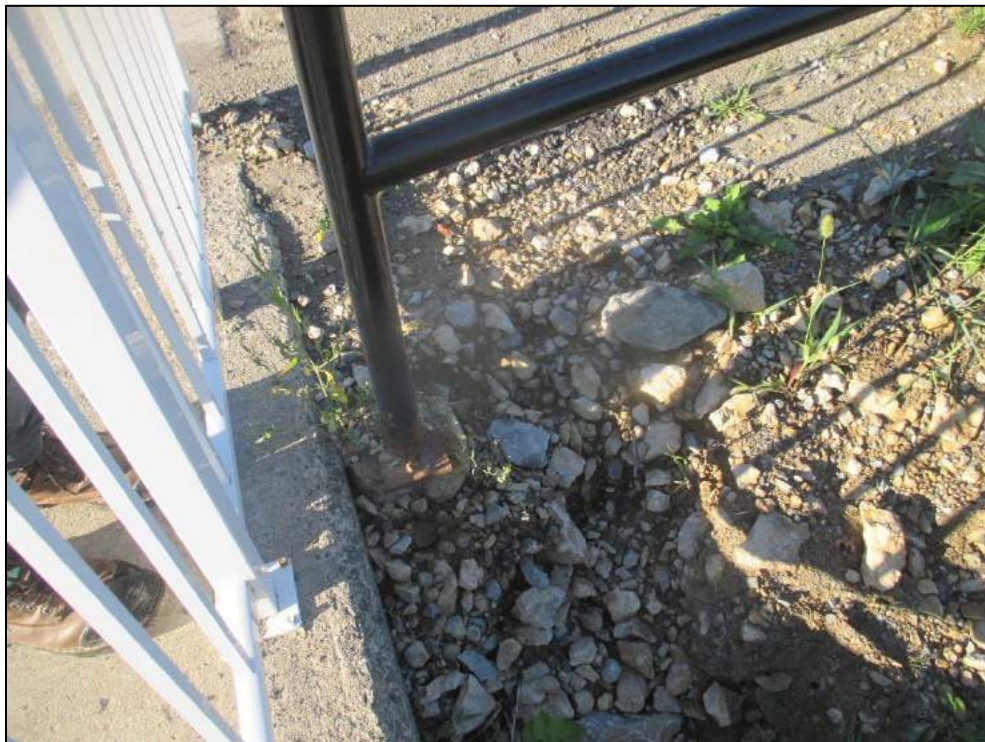
Rail post losing soil support at northwest, and deteriorate concrete.
