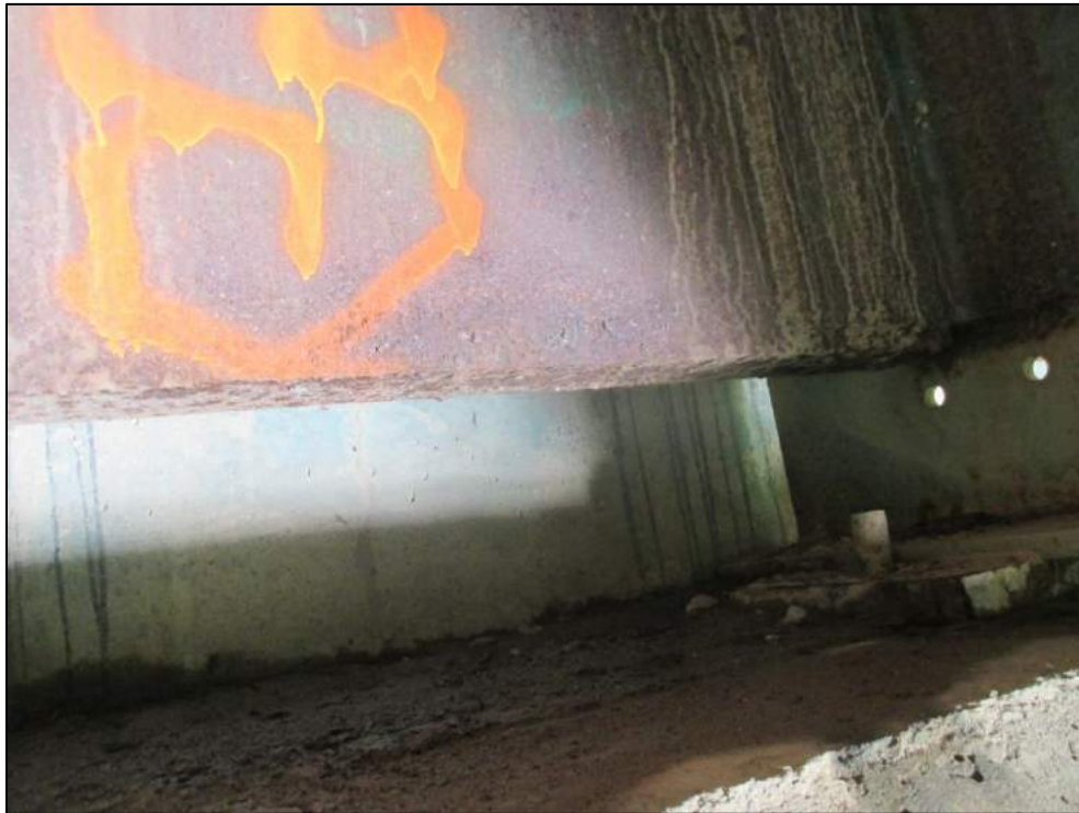
Medium corrosion of diaphragm.
