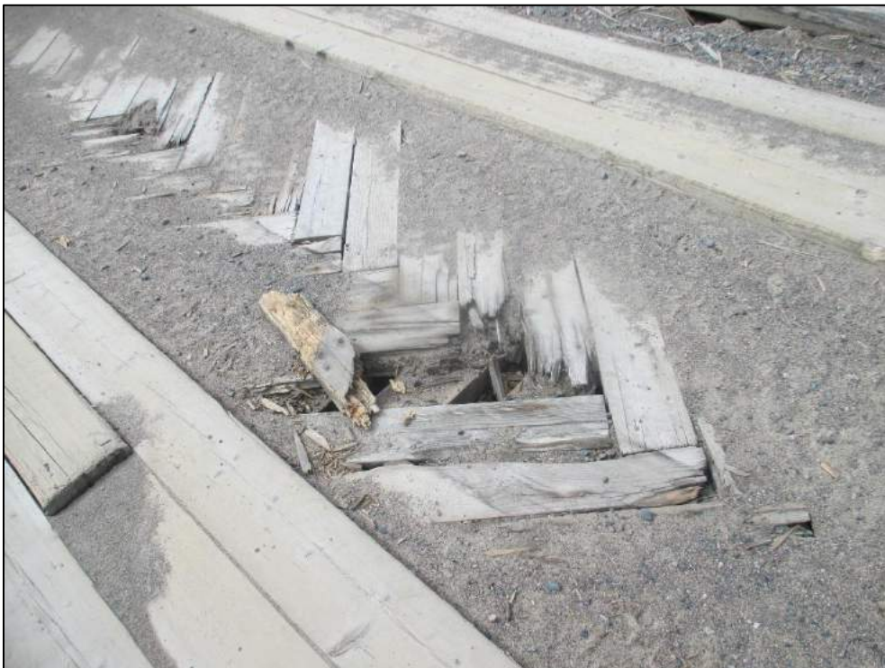
Severely damaged deck top.
