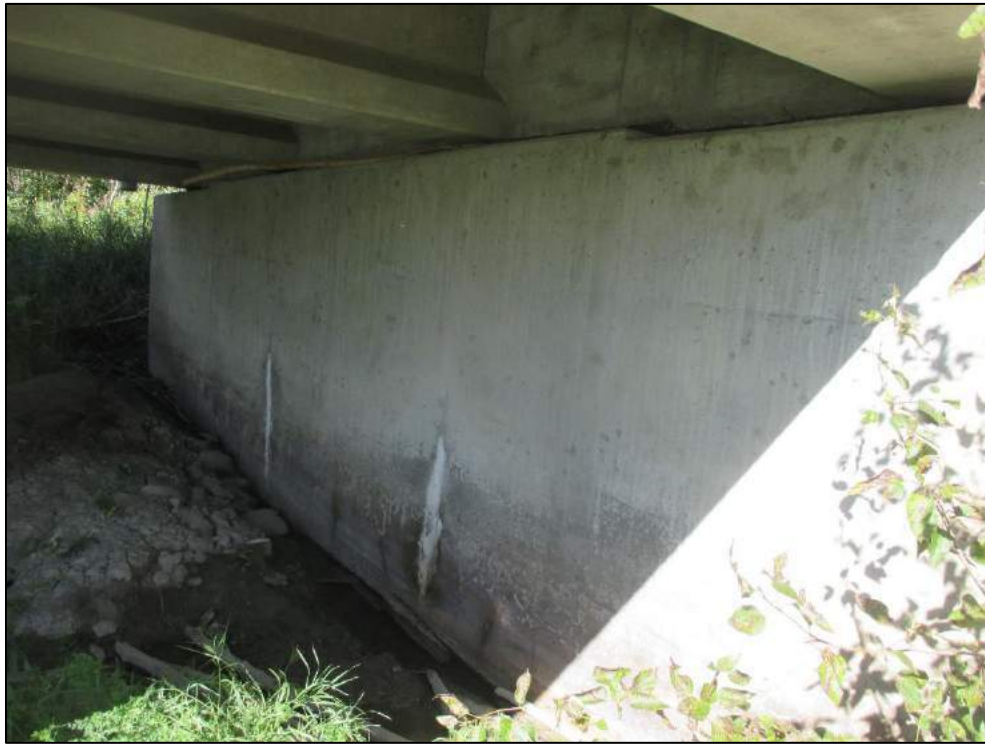
Cracks with efflorescence in east abutment wall.
