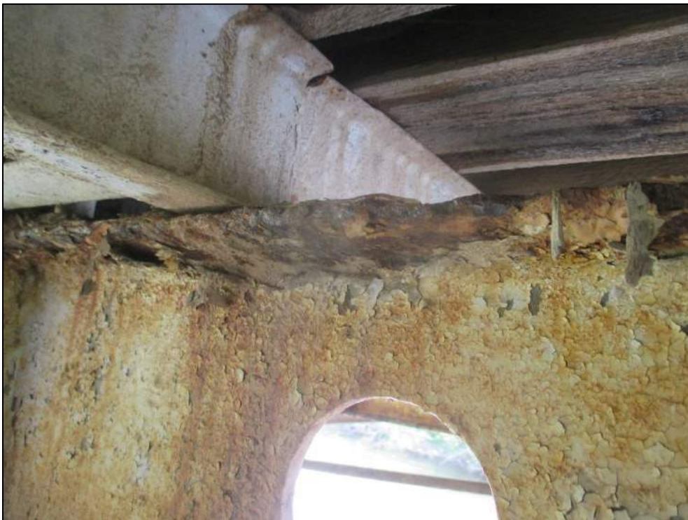
Severe corrosion and section loss of floor beams, failure of coating.
