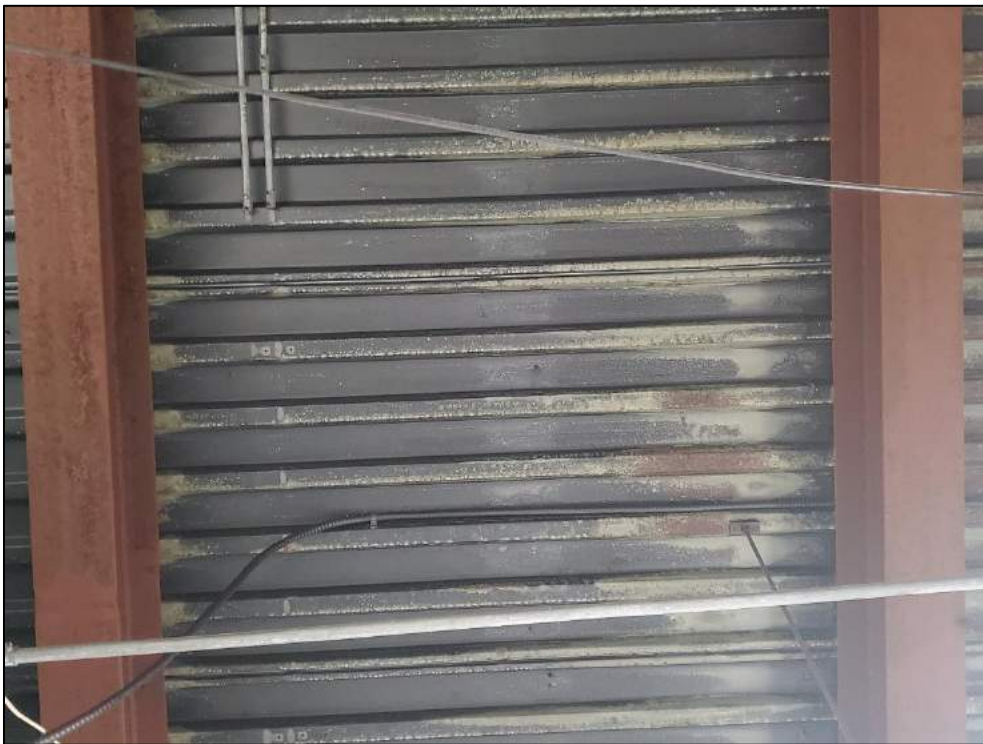
Damaged galvanized coating of steel decking in filter room.
