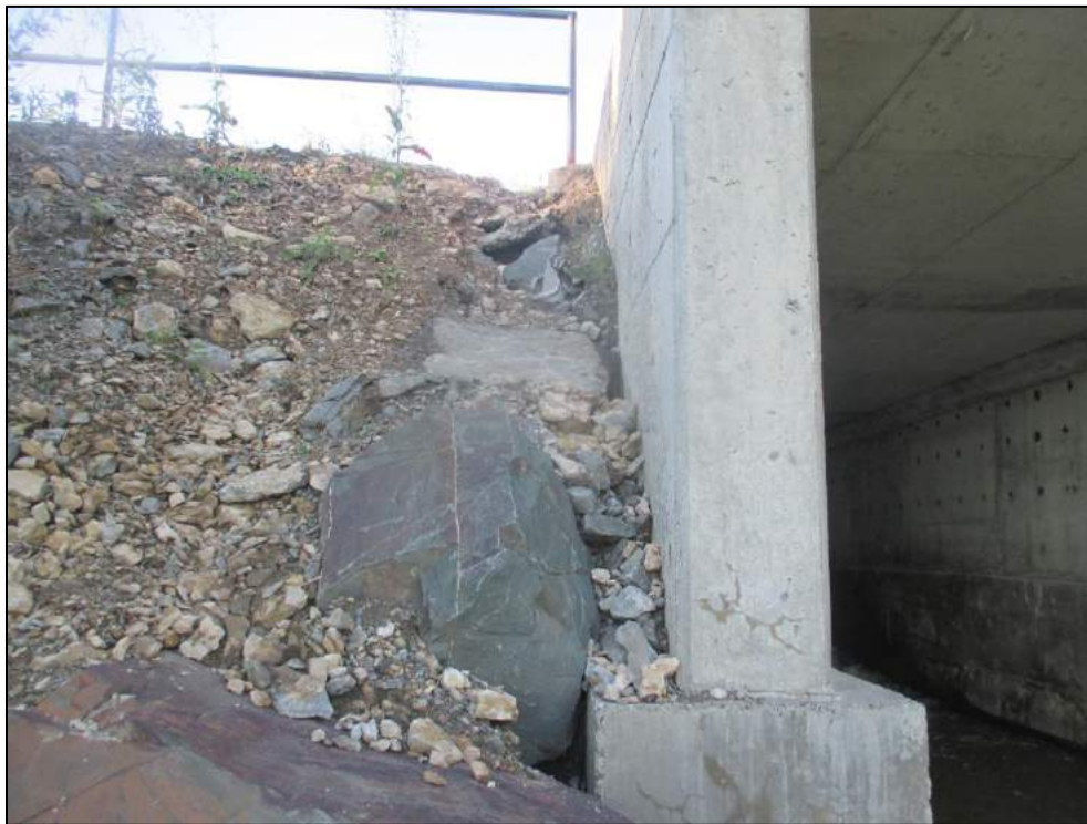
Washout at northeast, rail post losing soil support.
