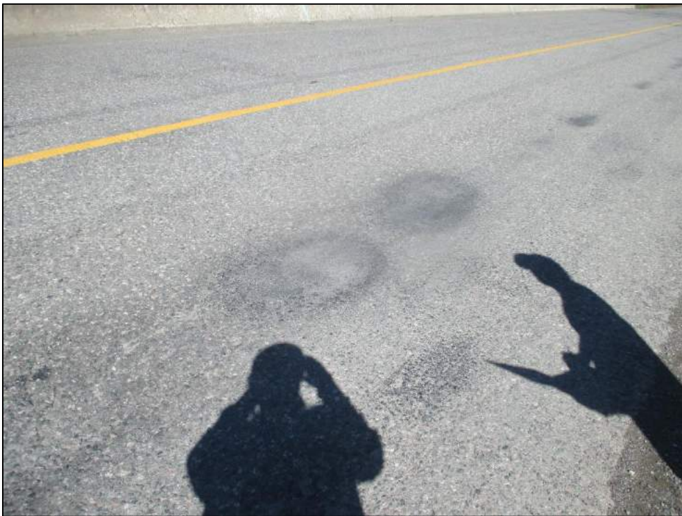
Patched potholes on wearing surface.
