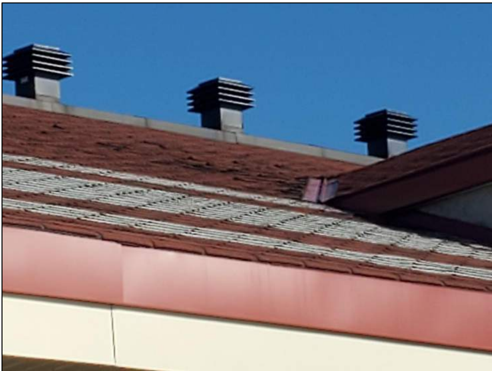
Deteriorated shingles at south
