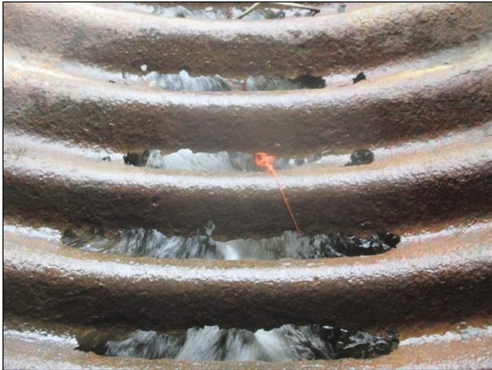
Full perforation of barrel bottom at north end.
