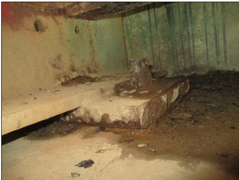
Medium corrosion of bearing.
