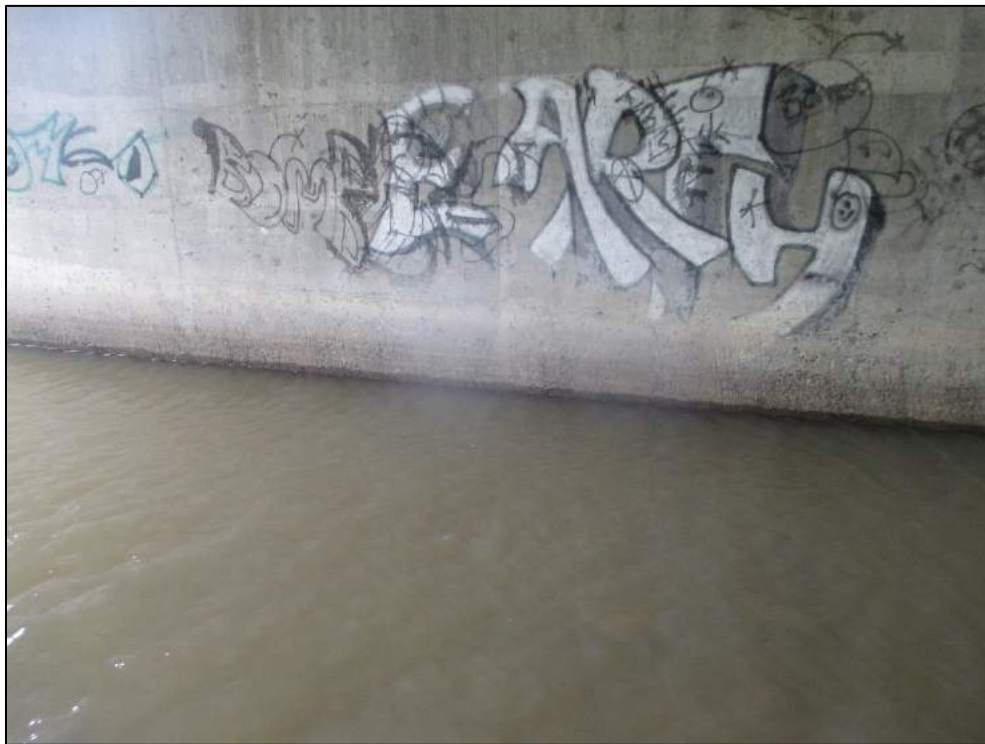
Scaling at waterline of north abutment.
