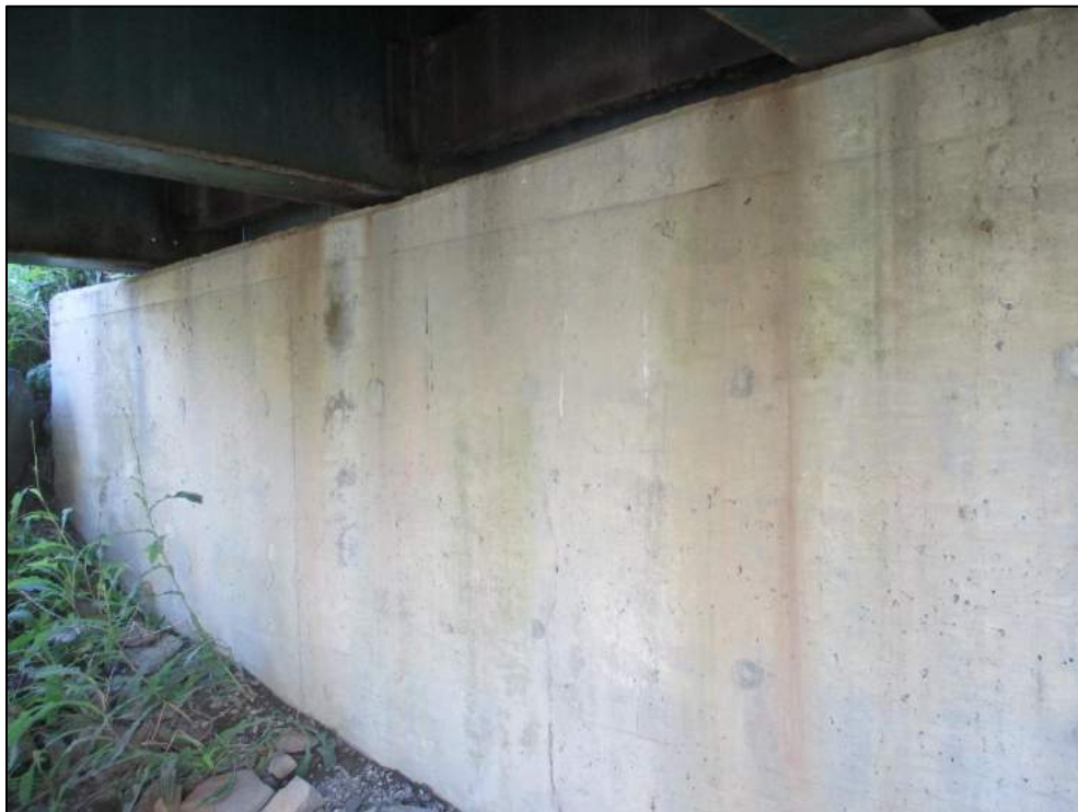
West abutment, multiple vertical cracks.
