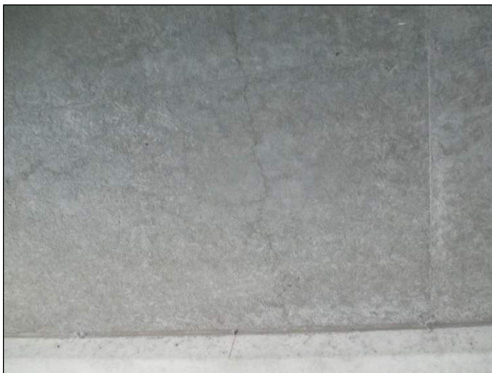
Medium transverse crack in soffit.
