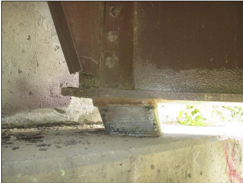
Excessive deformation of north bearings.
