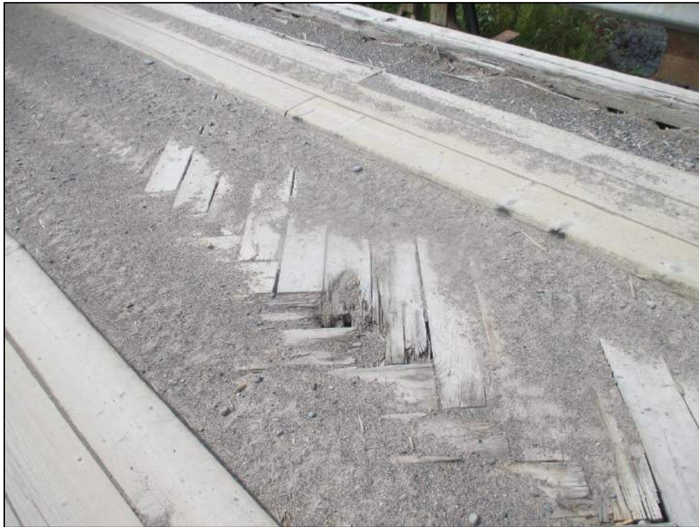
Severely damaged deck top.
