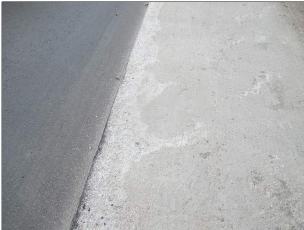
Scaling of sidewalk at northwest.
