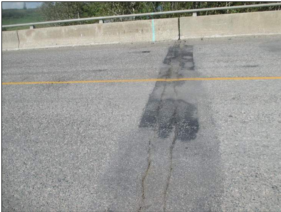
Failed, paved over joint at east.
