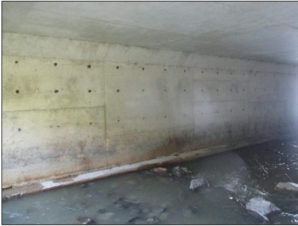
Cracking with moisture staining in southwest wall
