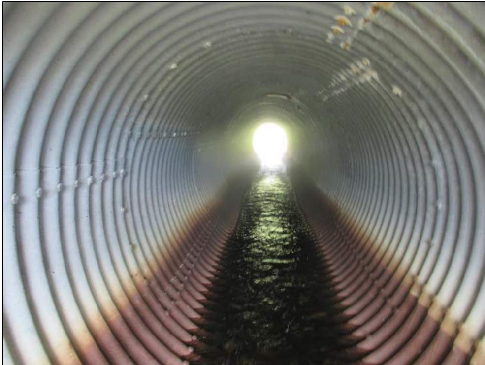
Barrel looking north, extensive corrosion along waterline.
