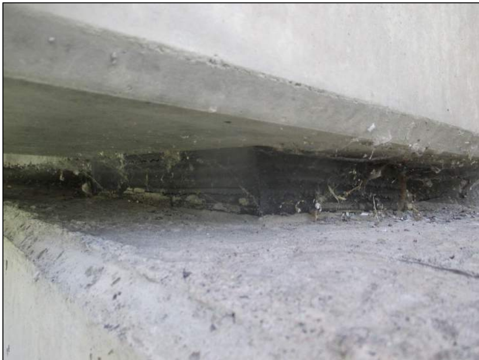
Wide crack in northwest bearing.
