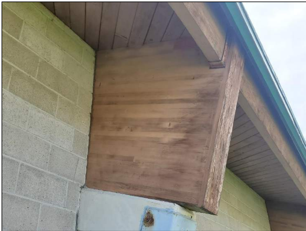
Dry rot on glulam beam ends.
