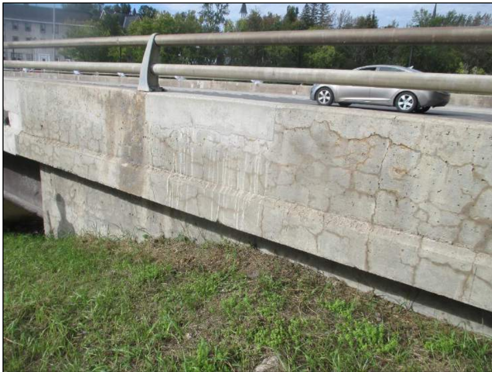
Extensive map cracking, possible AAR, at northeastern parapet wall and wingwall.
