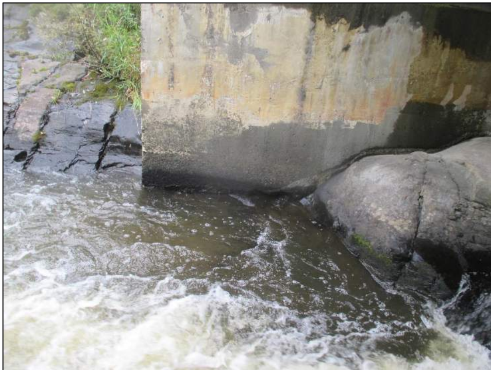
Undermining of abutment wall footing at northeast due to scour effect.
