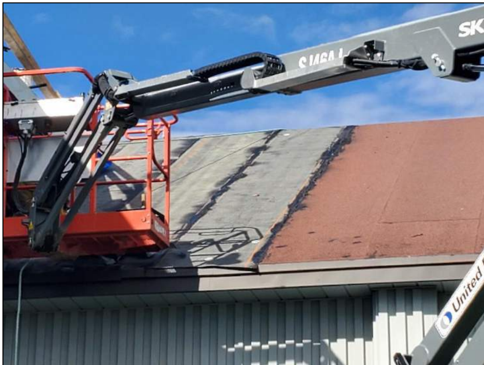
Roof in process of being replaced.
