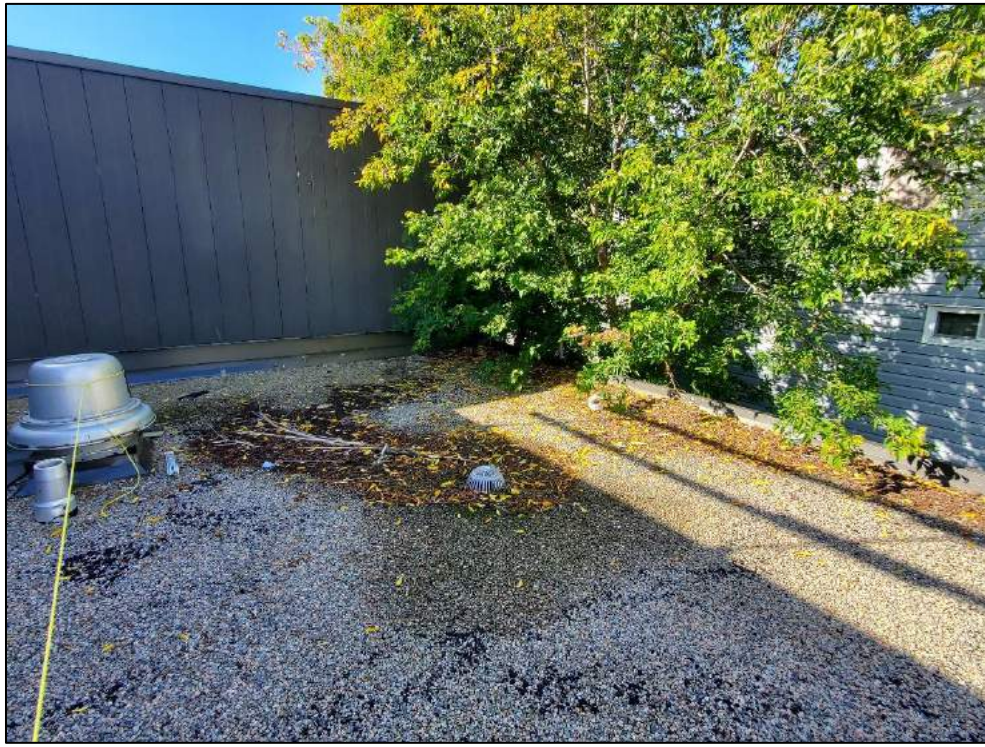
Tree overgrown onto roof, debris around drains.
