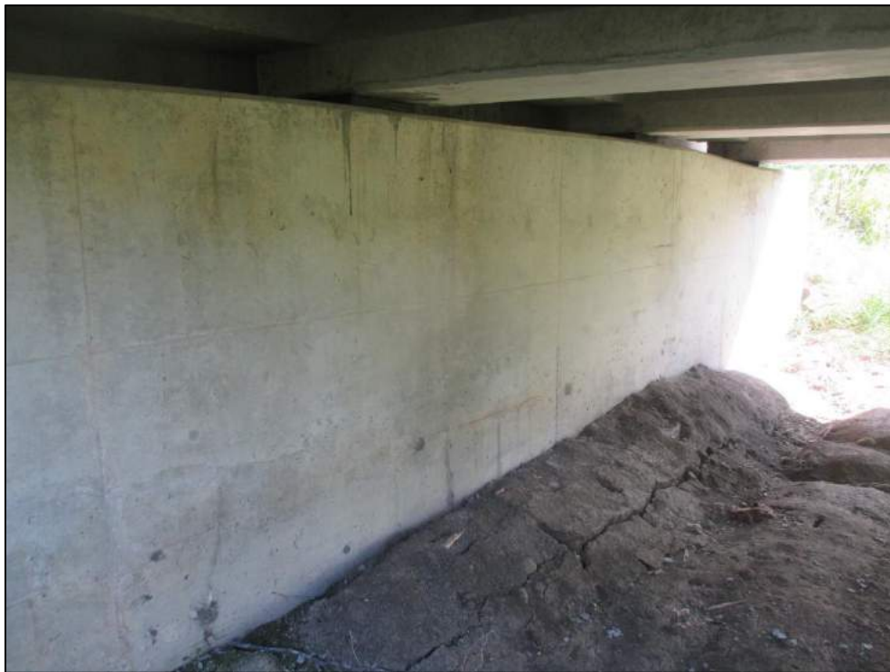
East abutment wall showing cracks.
