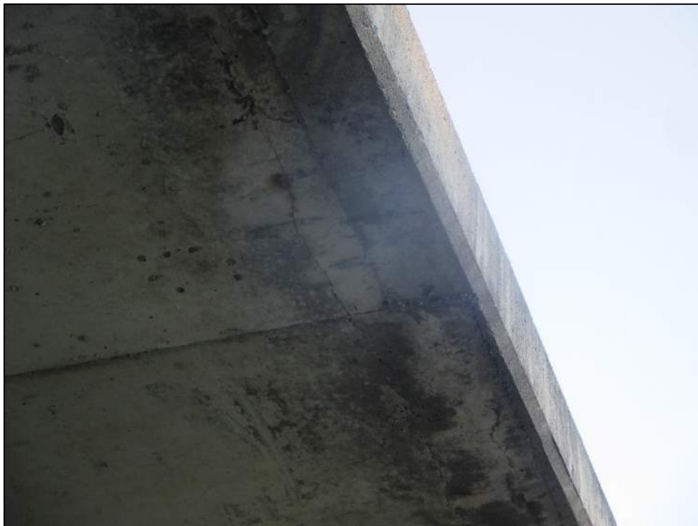
Crack, delamination, wet stains at north end soffit.
