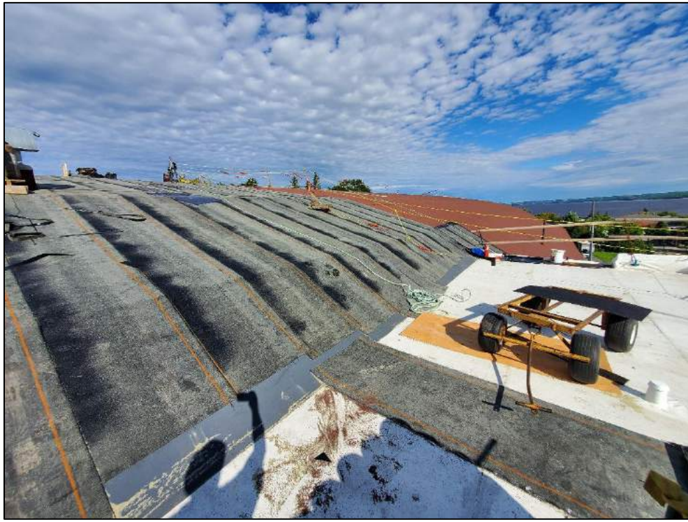
Center roof replacement and EDPM.
