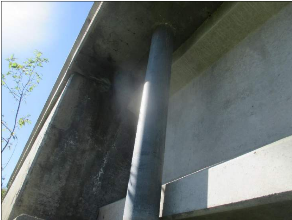
Wet stains and efflorescence on external soffit due to active leakage.
