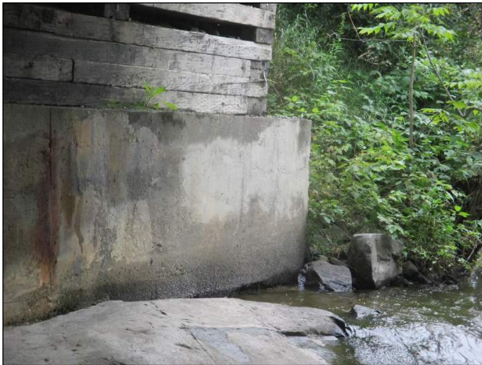
Undermining of abutment wall footing at southeast due to scour effect.
