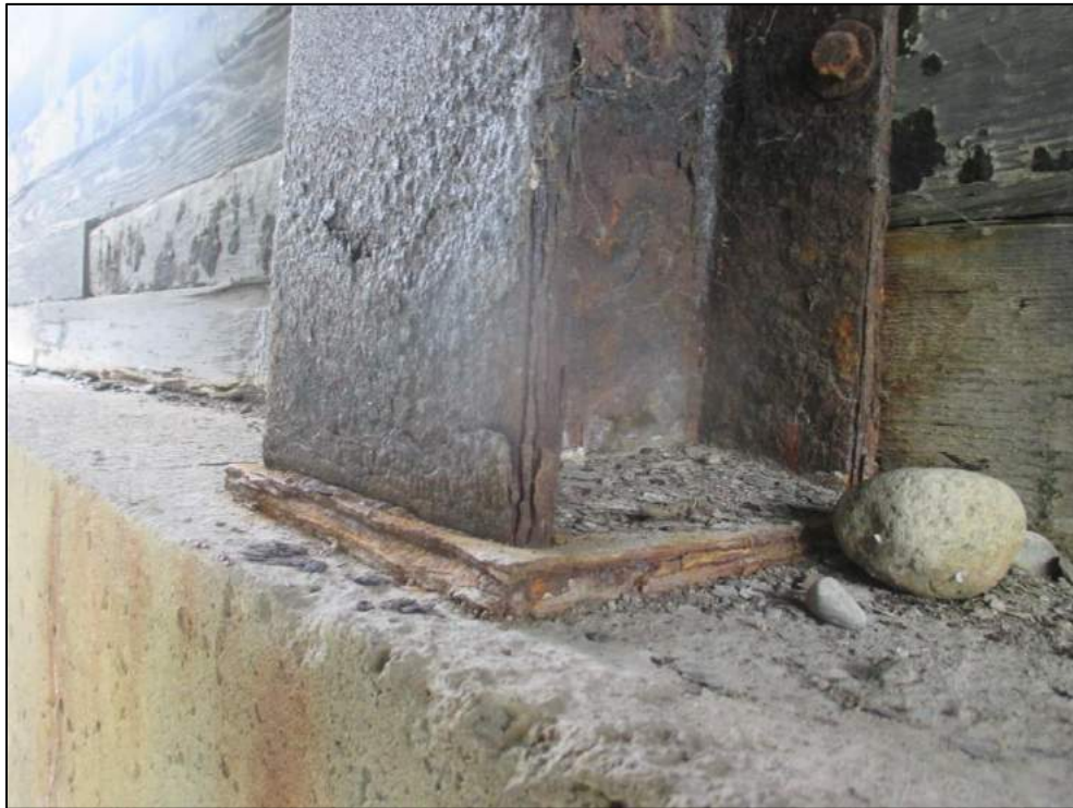
Severe corrosion with section loss of steel frame column base.
