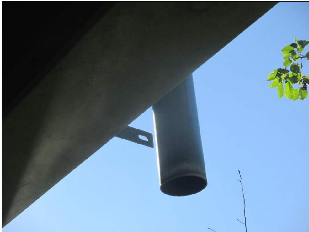
Drain pipe not connected to girders.
