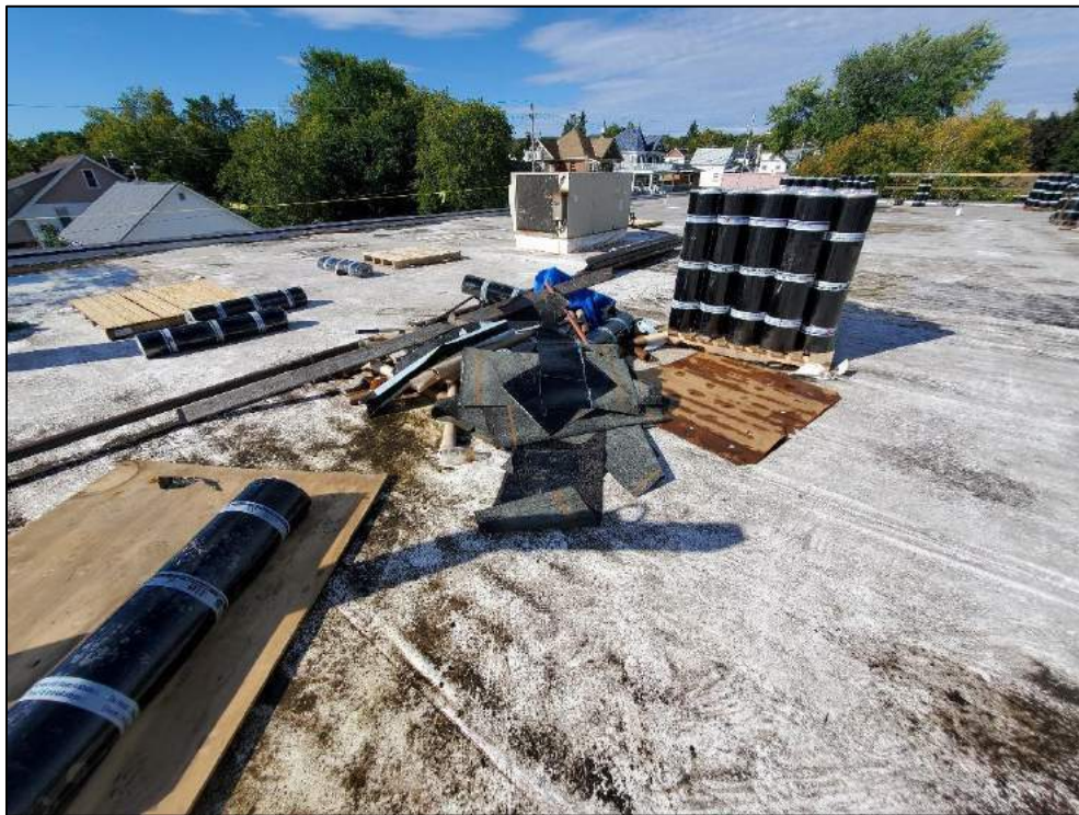
Construction debris on south upper roof with new EPDM coating.
