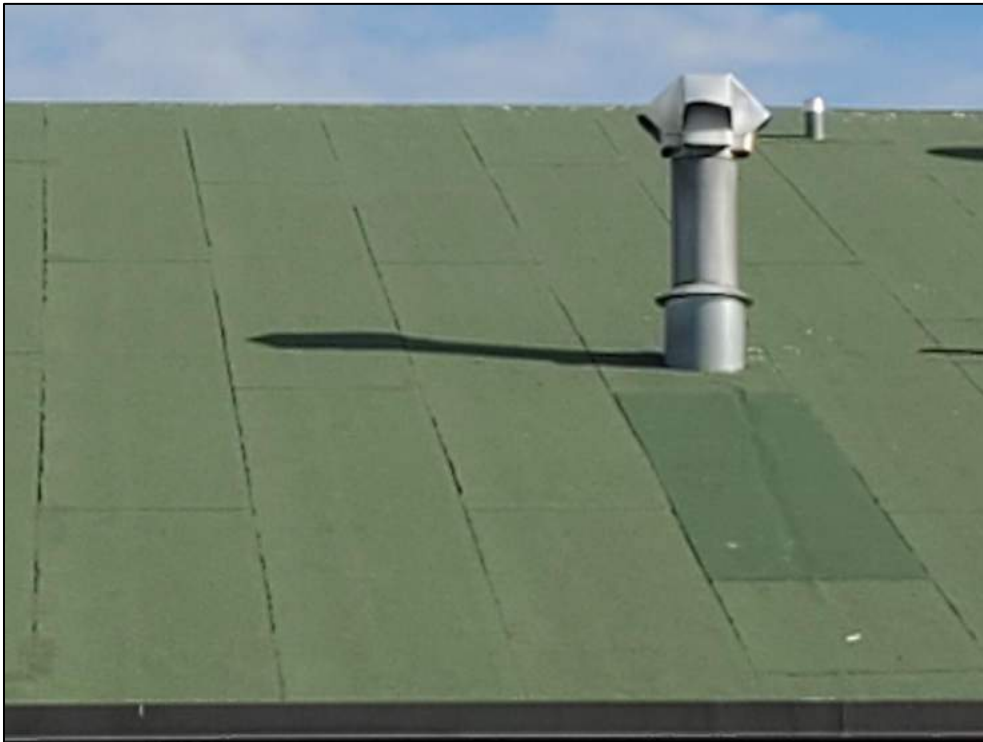
Existing patch of long strip asphalt on roof.
