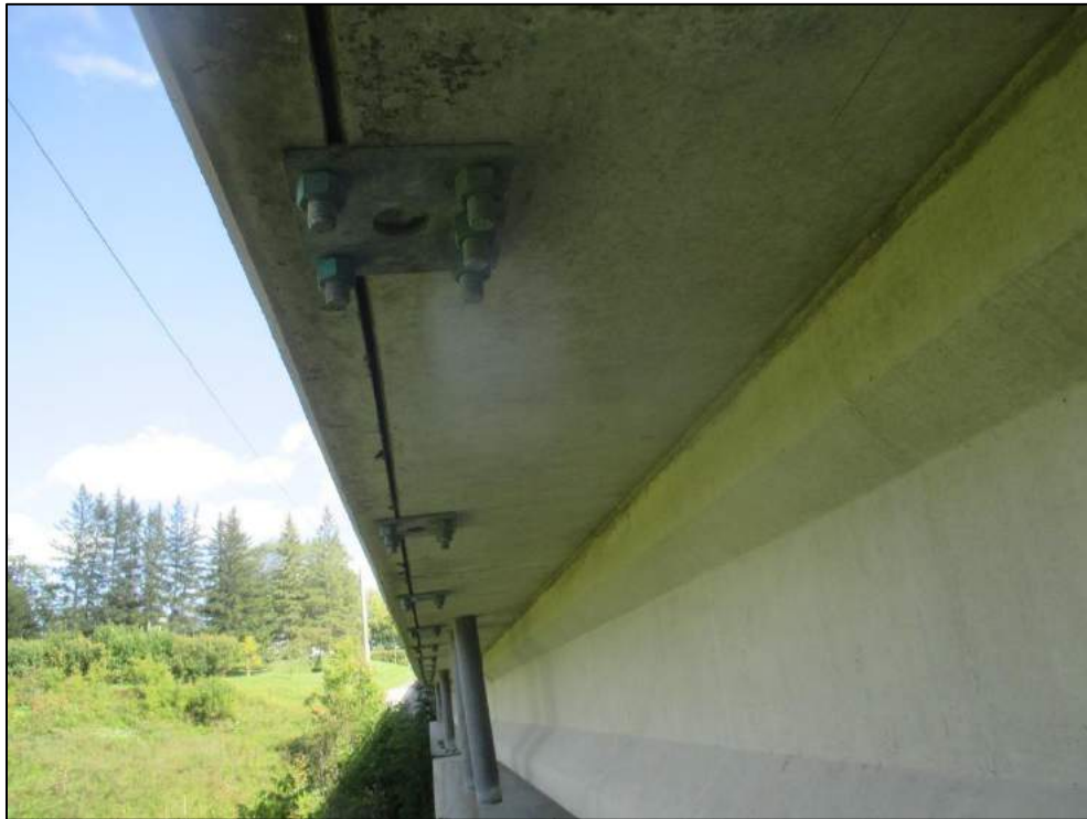
Exterior soffit and deck drains, hairline crack visible.
