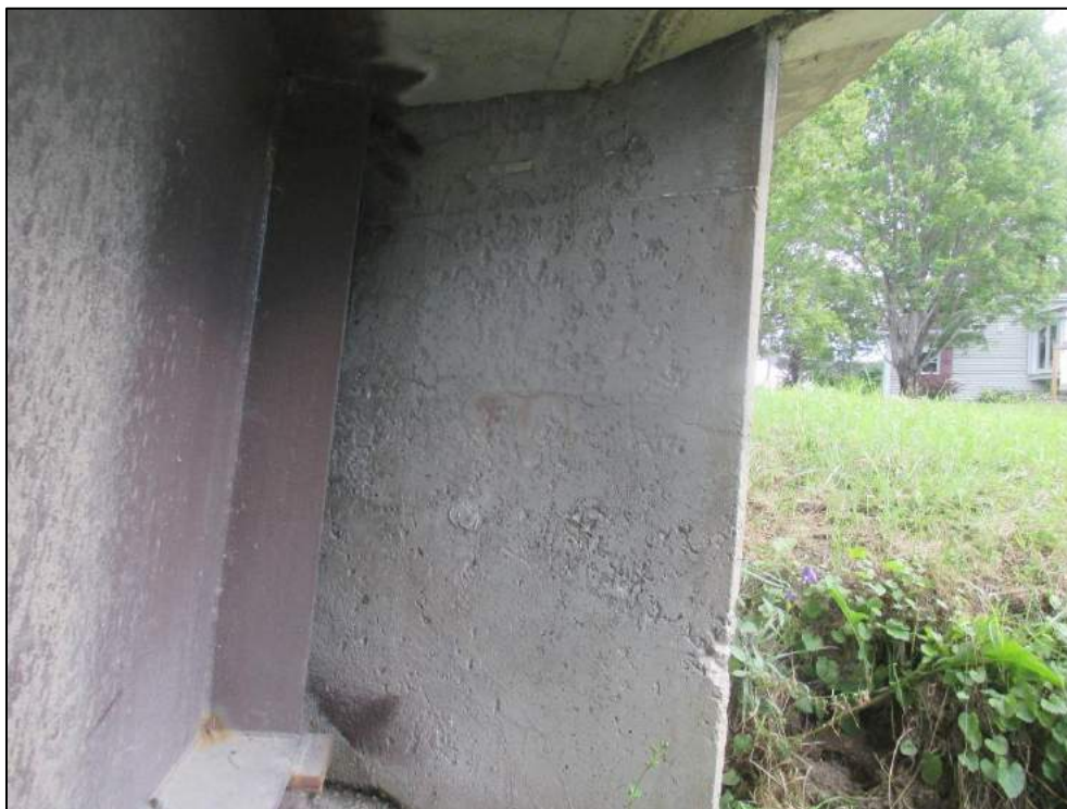
Cracking and honeycombing at northeast ballast wall.
