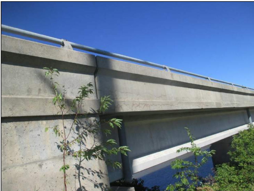
Map cracking on exterior of barrier wall.
