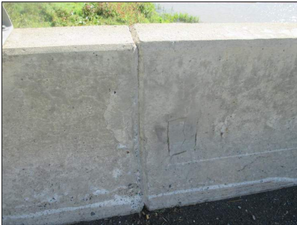
Delamination, cracking through previous patch at barrier wall
