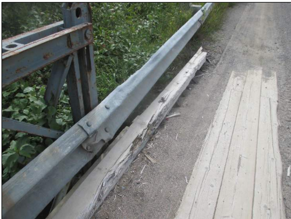
Severe splintering of curb at southeast.
