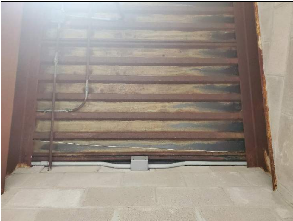
Extensive coating failure and corrosion of steel decking in filter room.
