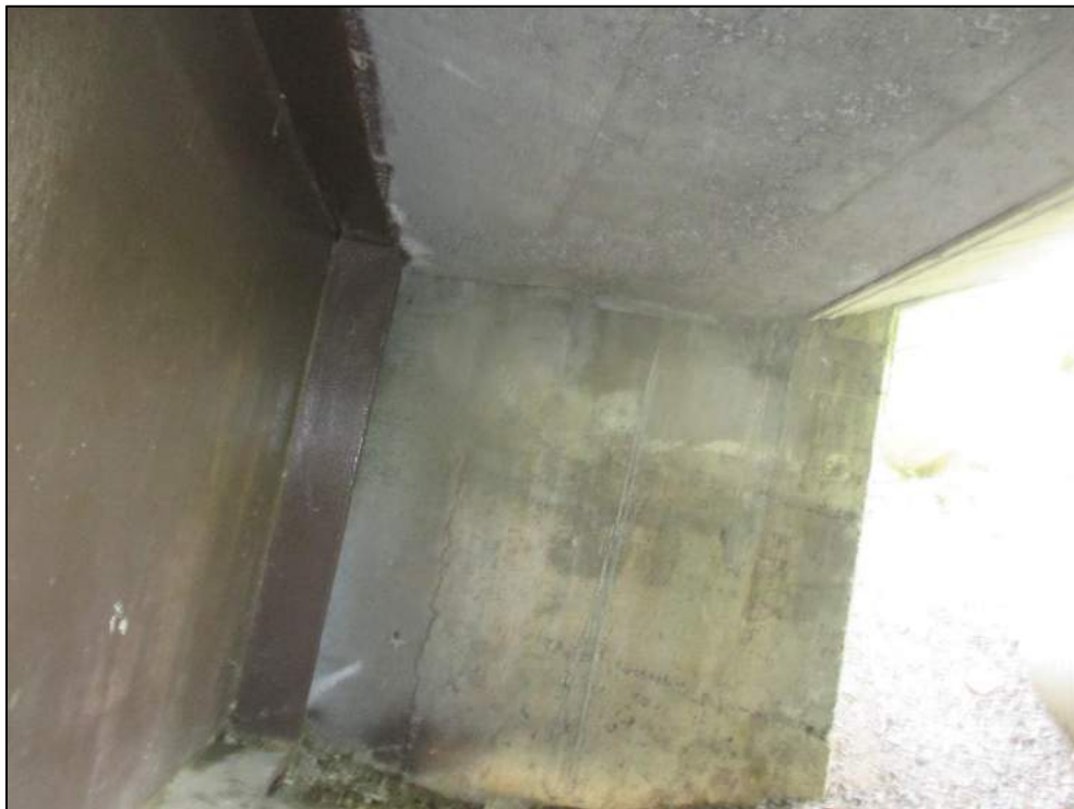
Crack in southwest ballast wall.
