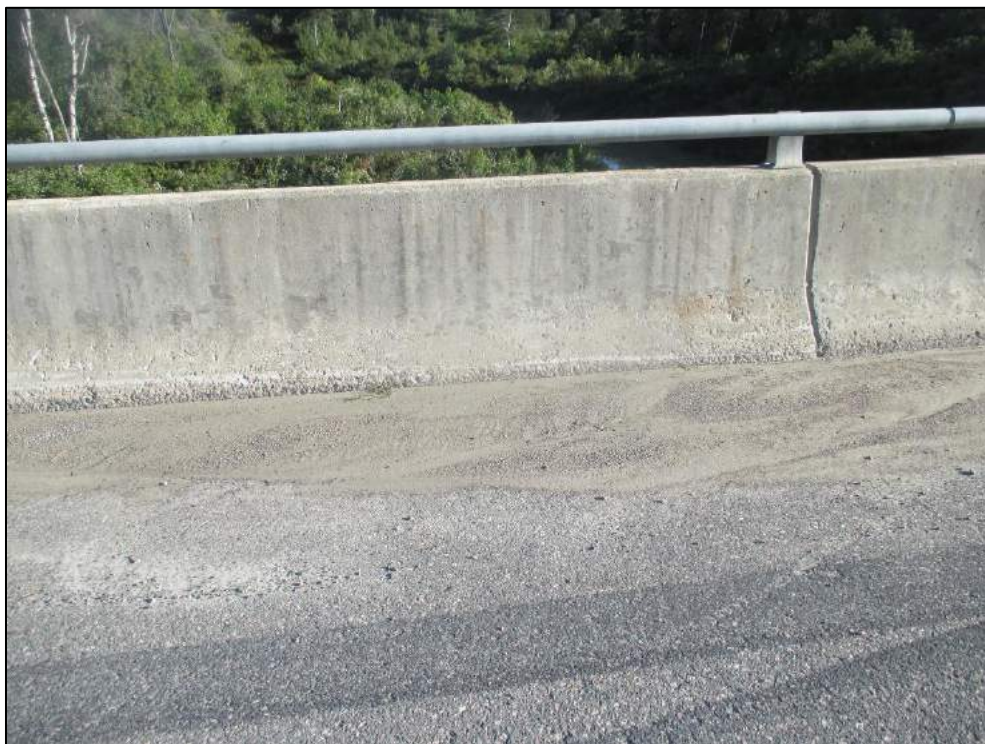
Medium to severe scaling at north wall.
