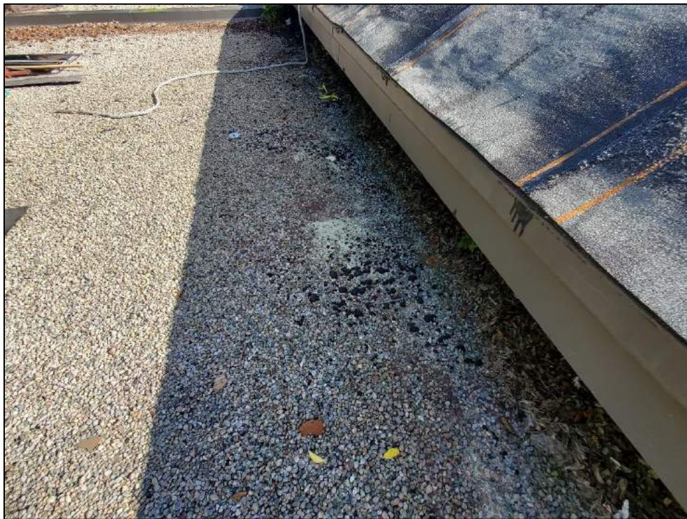
Displaced gravel and damaged tar coating due to runoff from upper roof.
