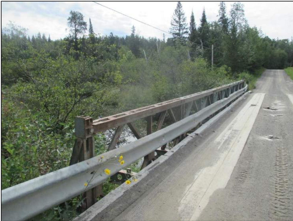
Collision damage at west rail, note no offset blocks present.
