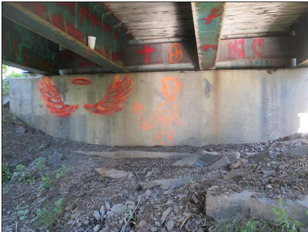
East abutment wall, narrow vertical crack visible at south.
