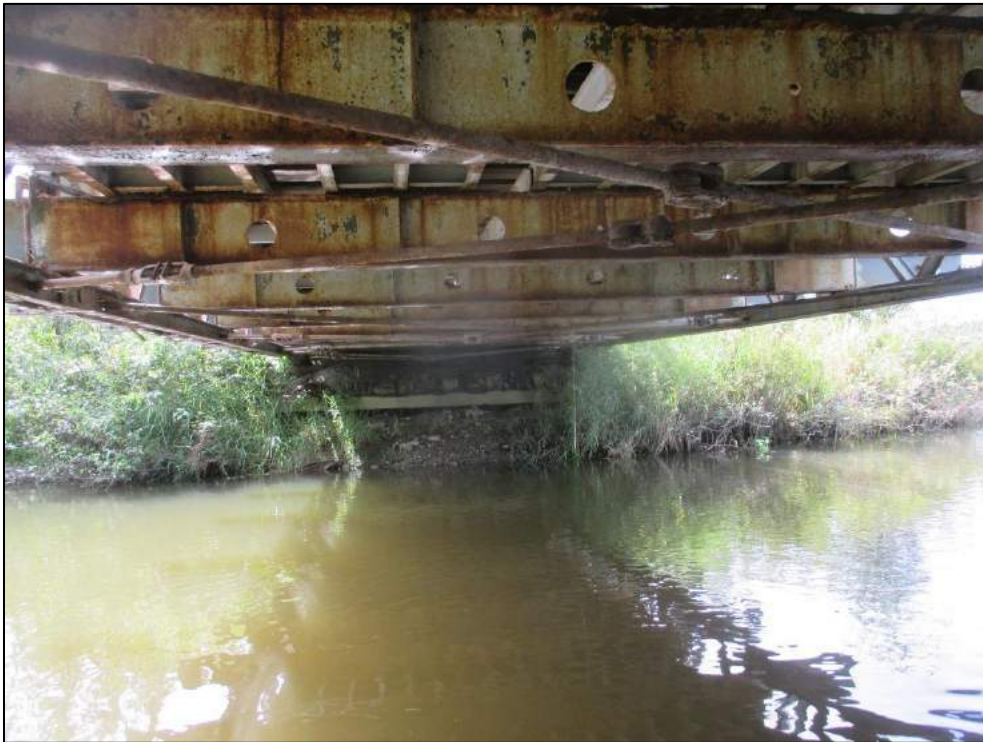
Underside looking south, severe corrosion of bracing and floor beams.
