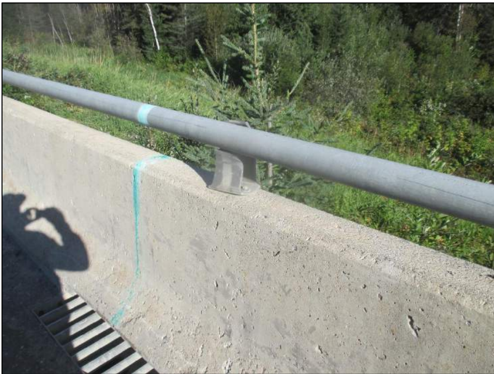
Damaged handrail bracket at northwest.
