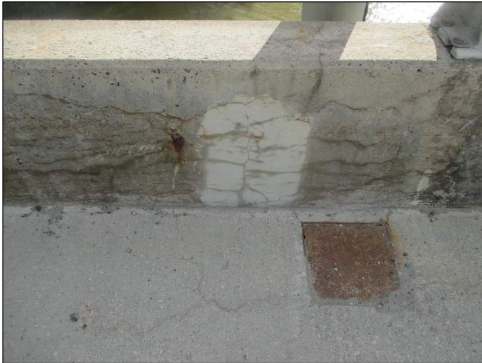
Patches, map cracking, delamination, and exposed corroded rebar on parapet wall.
