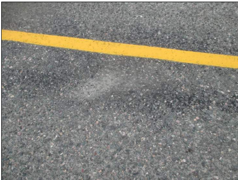
Pothole on deck wearing surface.
