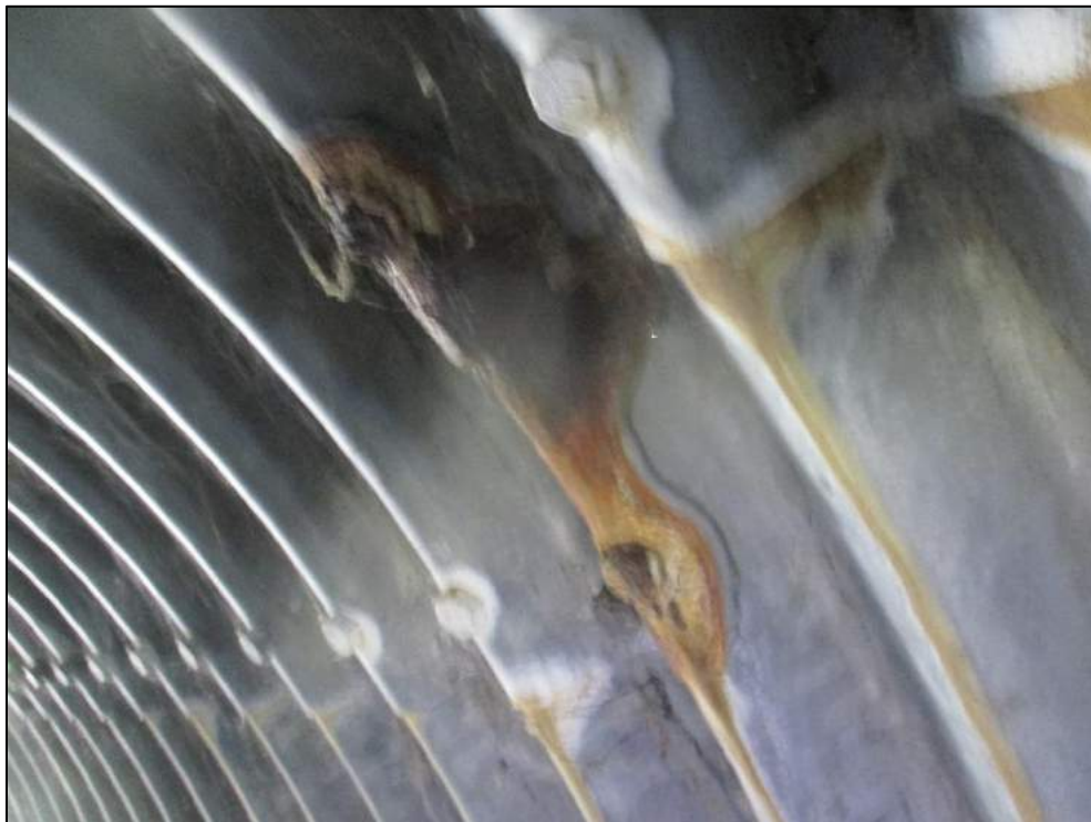
Severe corrosion and section loss at top of barrel.
