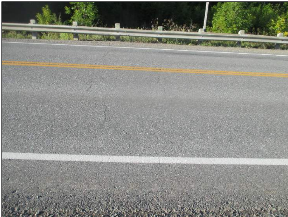
Cracking in wearing surface.
