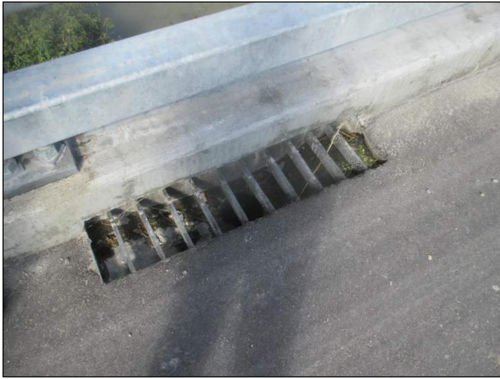
Deck drain, narrow cracks in curb.
