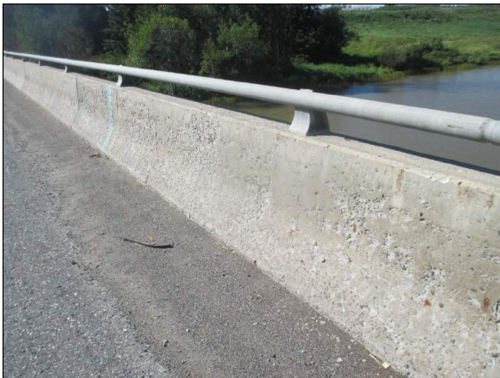
Very severe scaling along north barrier wall.
