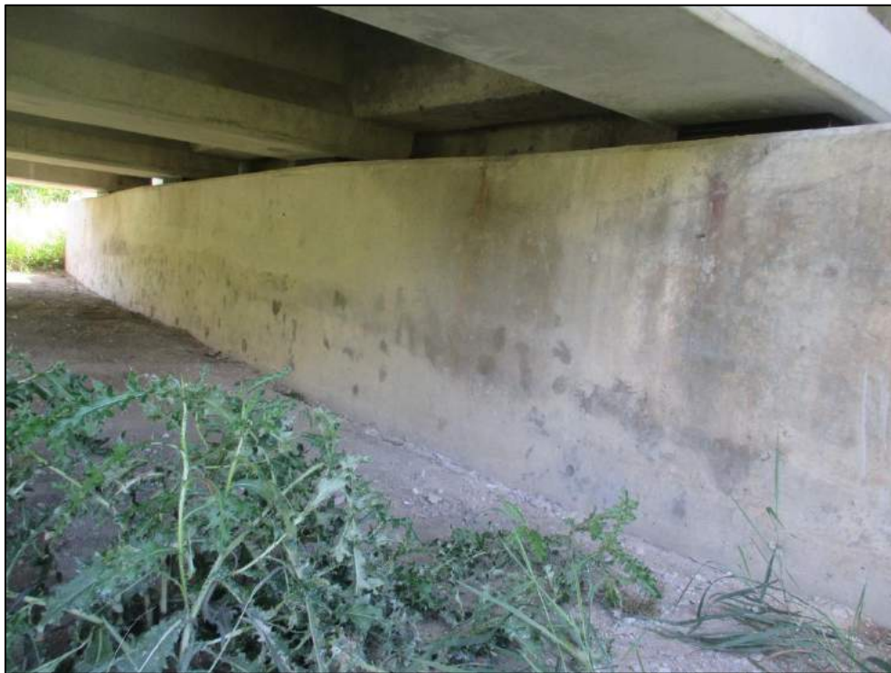
West abutment, pattern cracking with rust staining shown.
