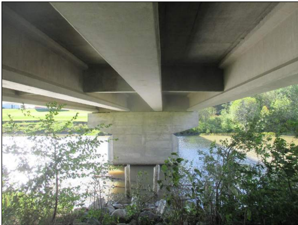
Soffit, girders, and east pier.
