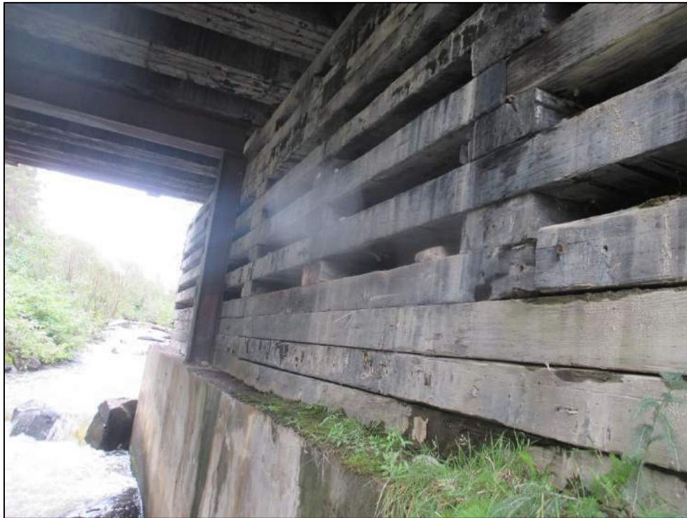
West abutment, light checks and medium weathering in timbers.
