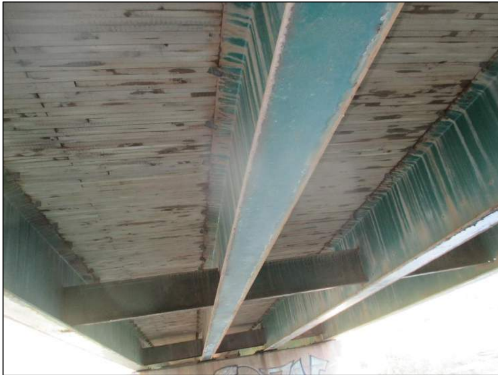
West span soffit, girders with wet stains and corrosion.
