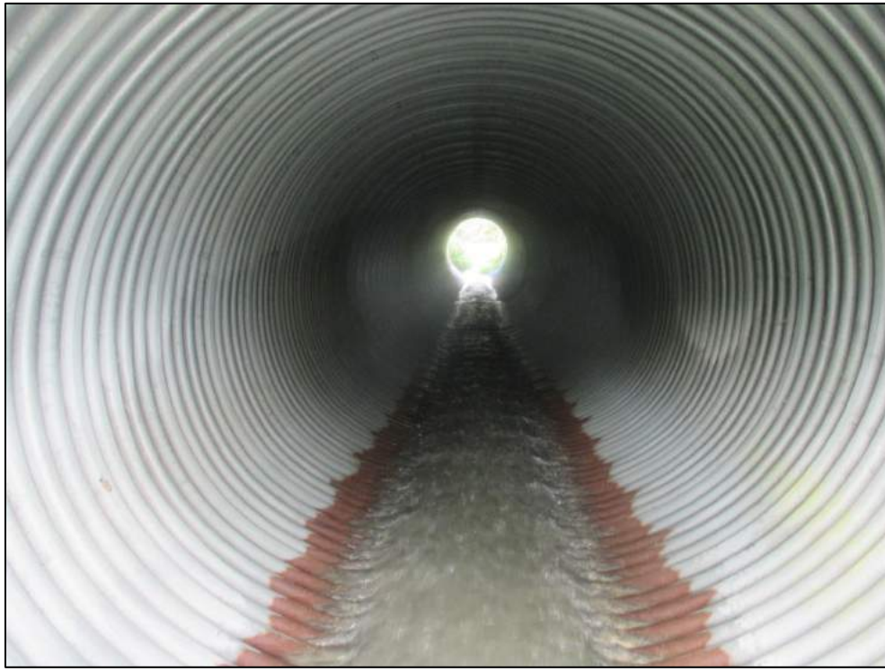
Barrel looking west, extensive light corrosion visible at culvert base.
