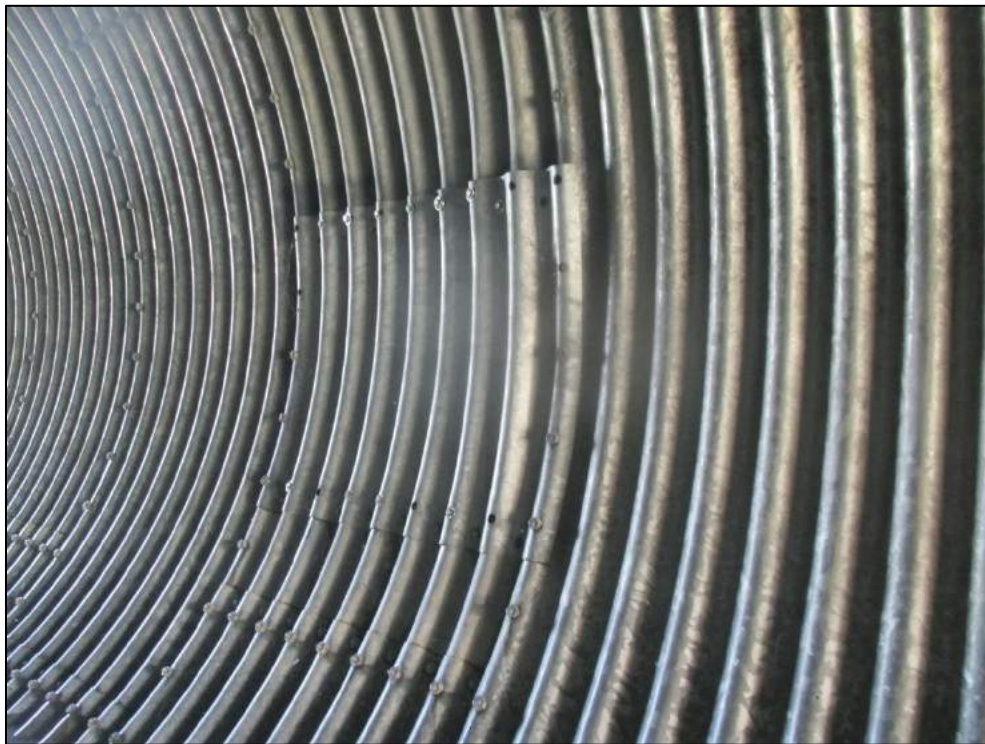
Barrel patch with missing bolts.
