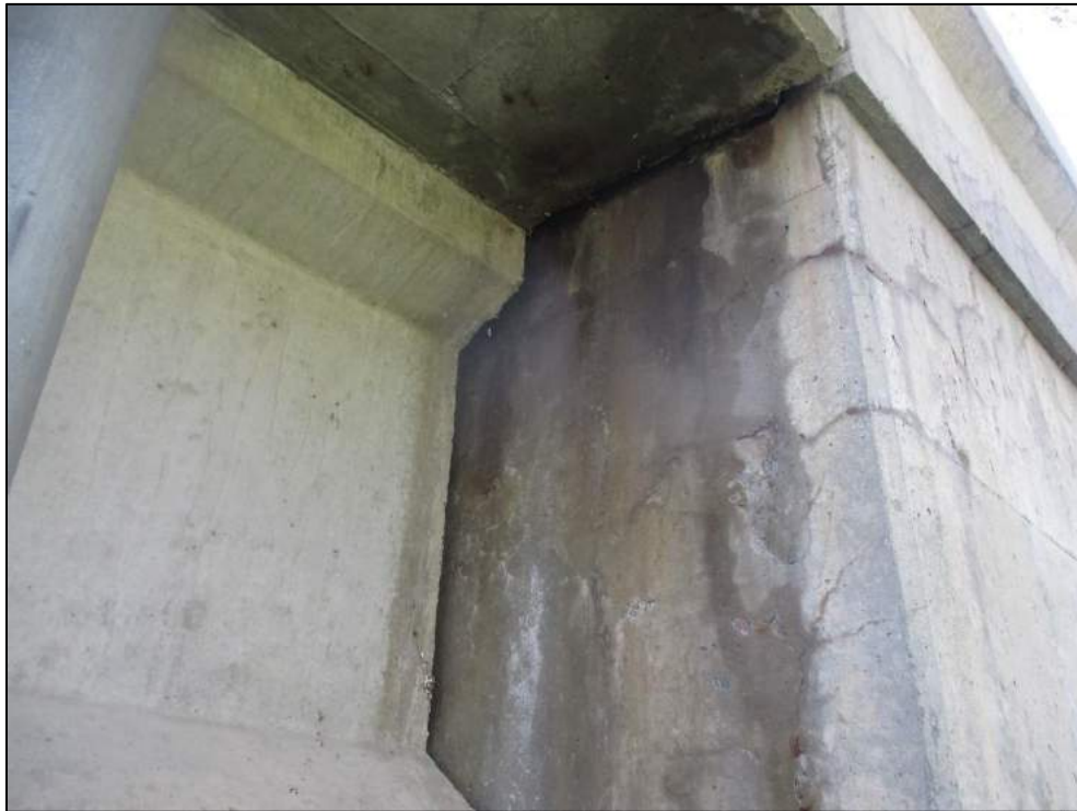
Wet stains on ballast wall due to joint leakage, spall and cracking in ballast wall.
