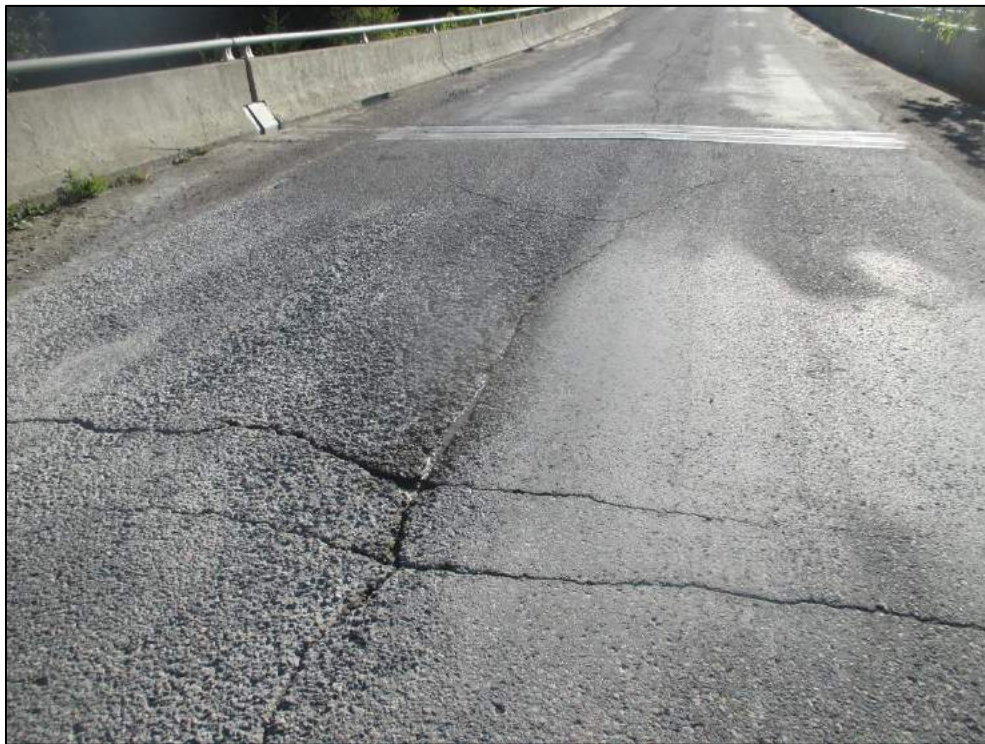
Wide cracks and dip at west approach with evidence of pooling water.
