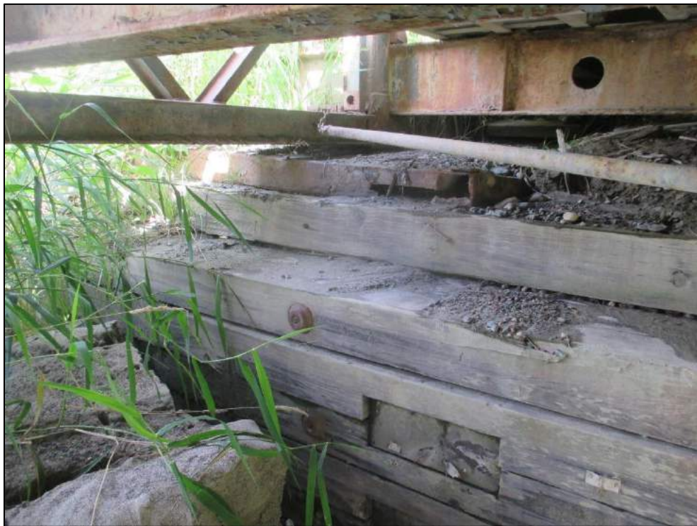
Severe corrosion and perforation of bearing plate.
