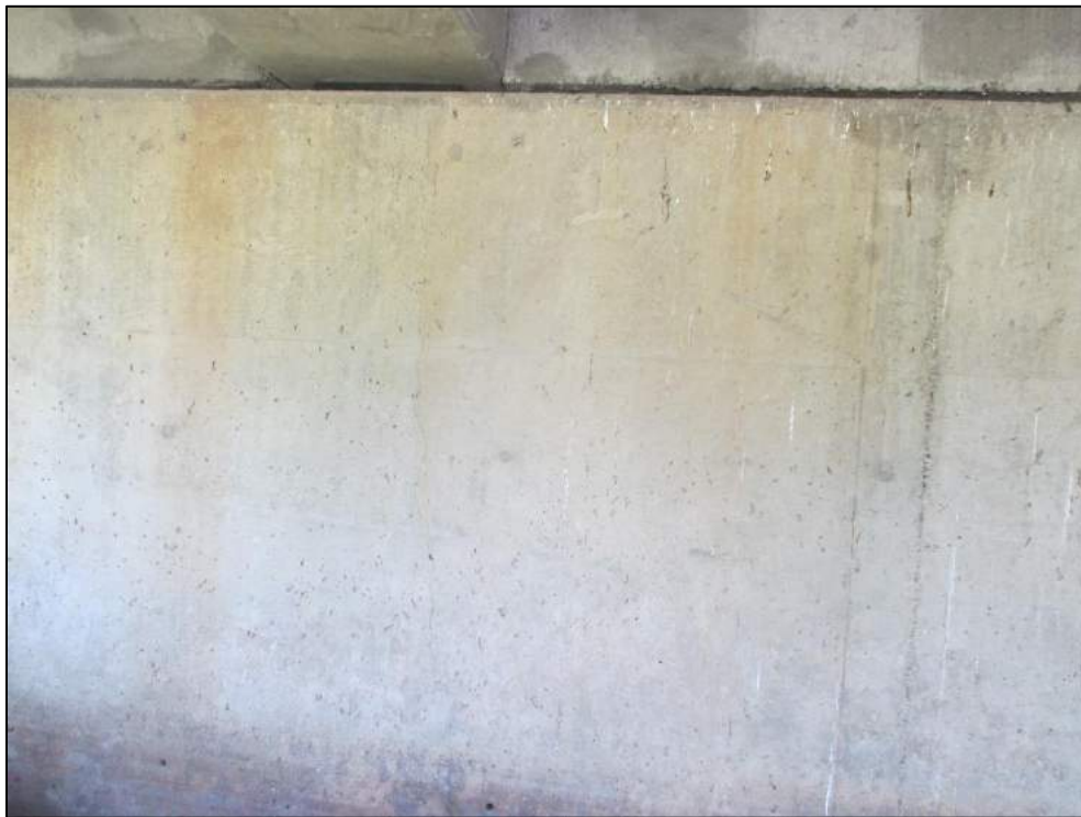
Full height crack on west abutment wall.
