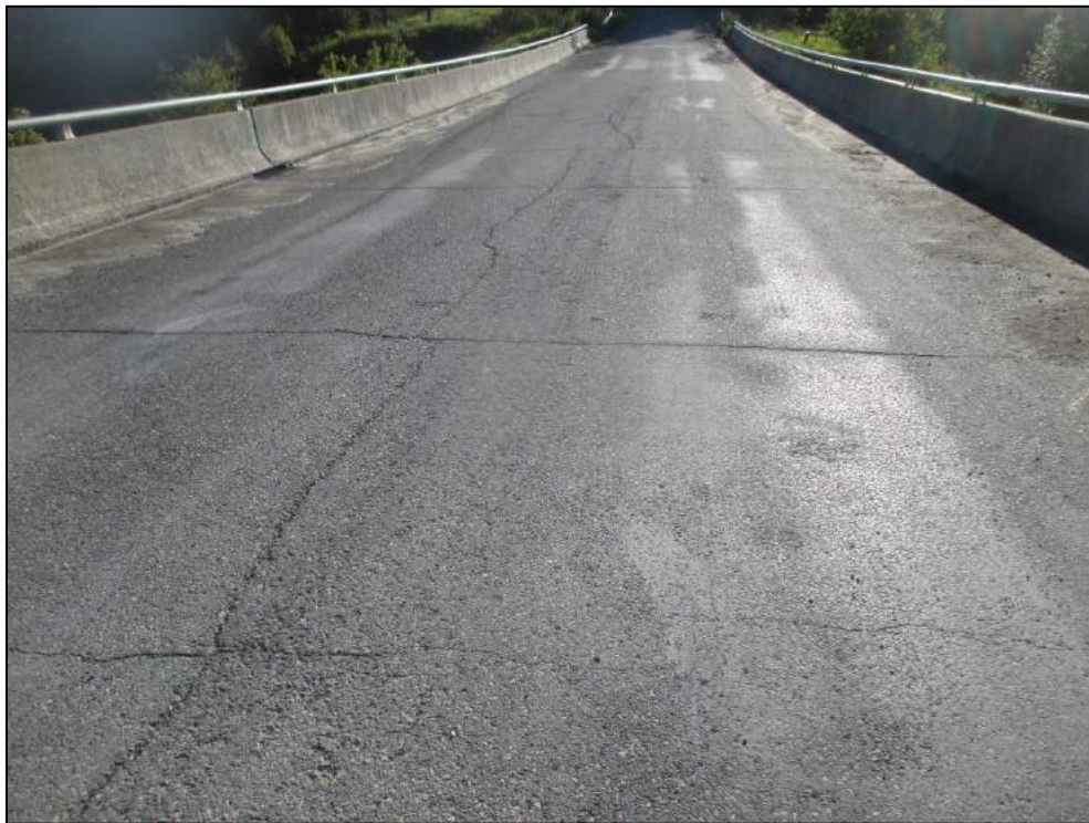
Wide longitudinal and transverse cracks on deck wearing surface (typ.)
