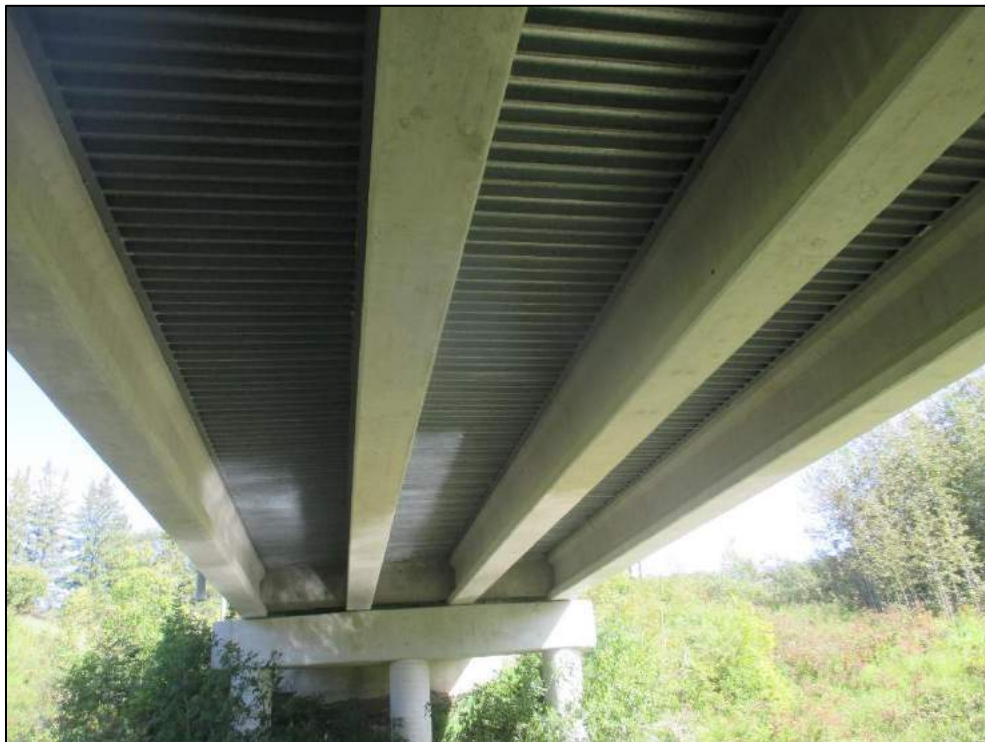
Steel decking at soffit and girders.
