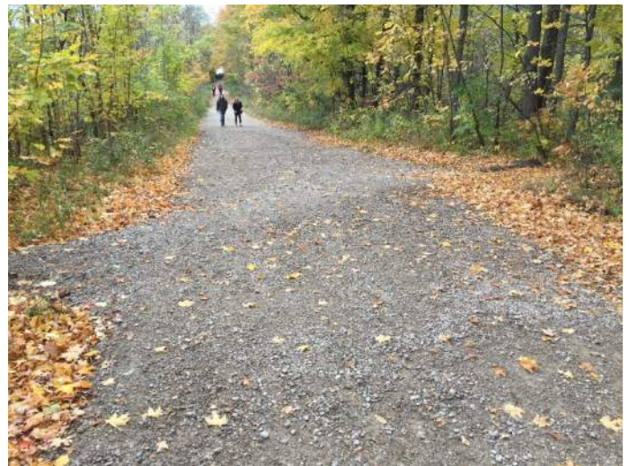
Figure 22 | Photo of rolling grade dip method to mitigate longitudinal slope rutting. Buried log used to create drain break hump (Mount Nemo, Burlington).
