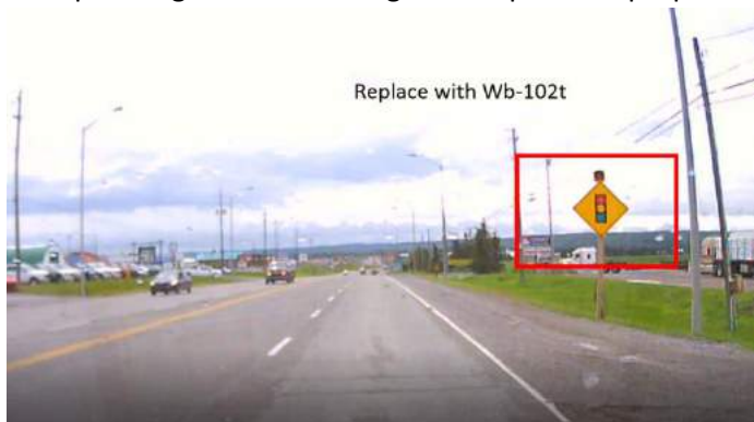
Figure 5 Coordinate flashing lights with traffic signals
