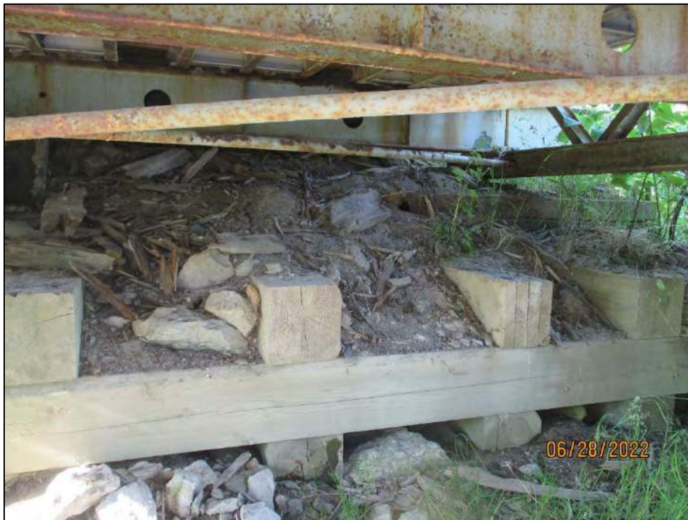
South Abutment (Rock-Filled Timber Crib)
