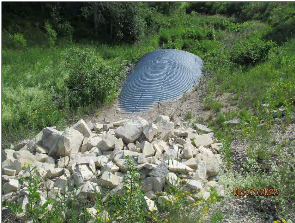
South (Outlet) Projecting End
