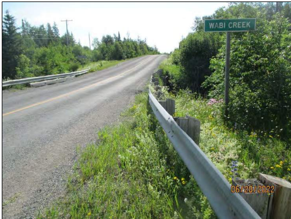
Collision damage and poor SBGR at S/W
