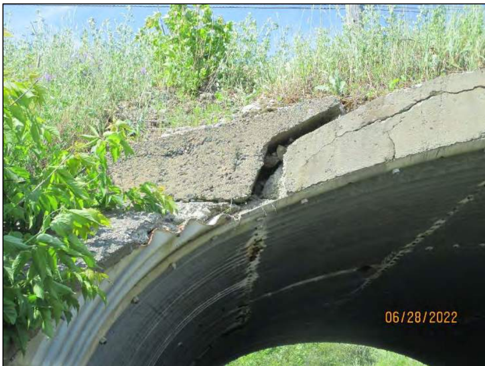
Concrete Damage (Typ.)
