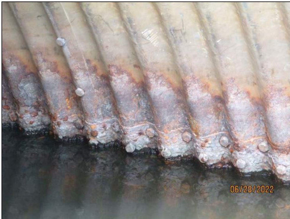
Culvert Barrel (corrosion at waterline) – Typ.
