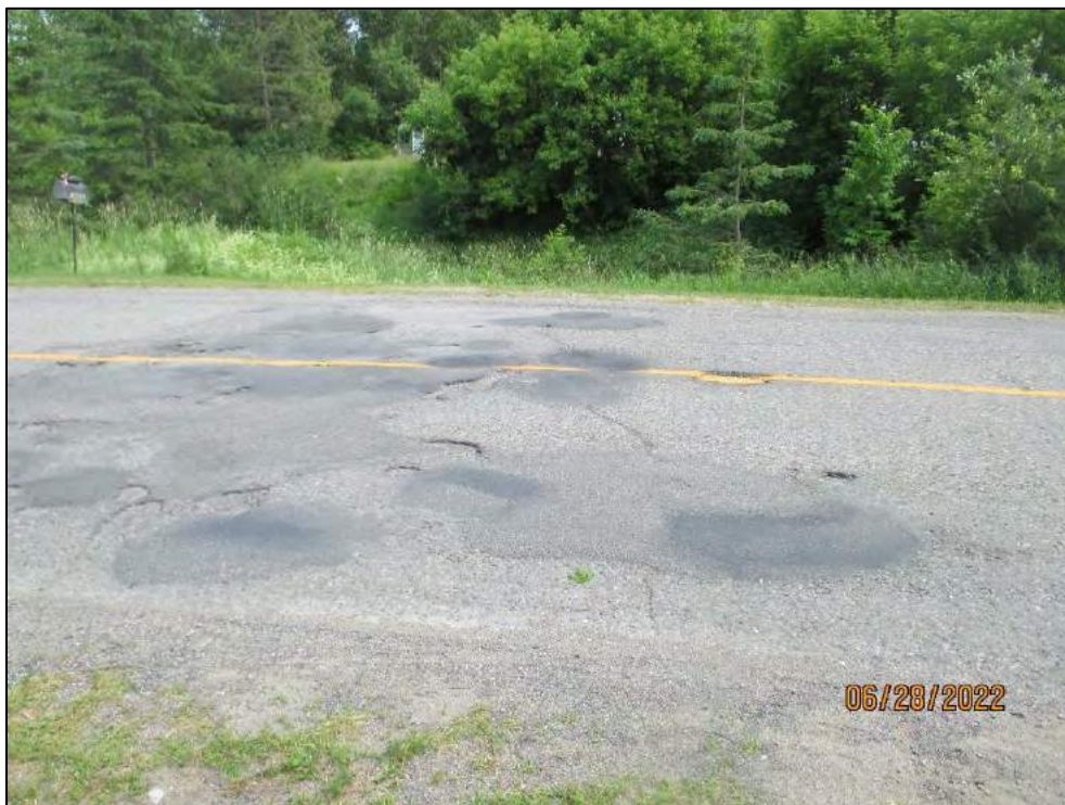
Approach Wearing Surface (Poor)
