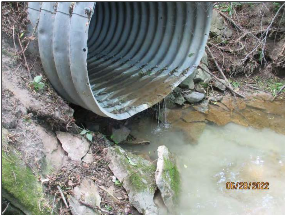
East Barrel (Scour at Outlet)
