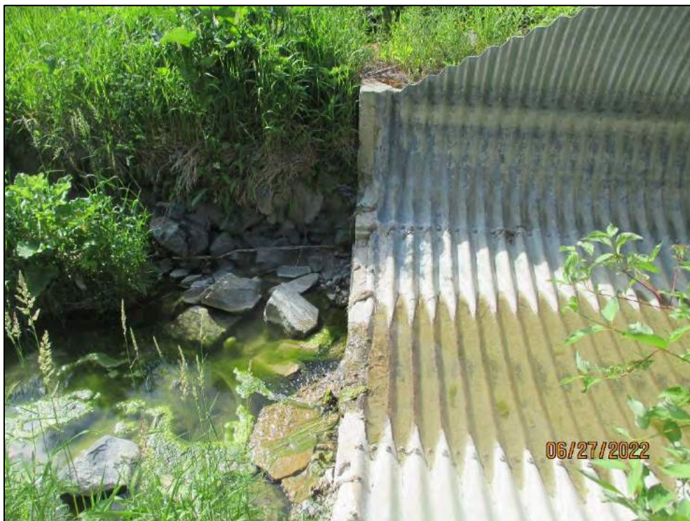
South Cut-Off Wall and Creek Scour at Outlet
