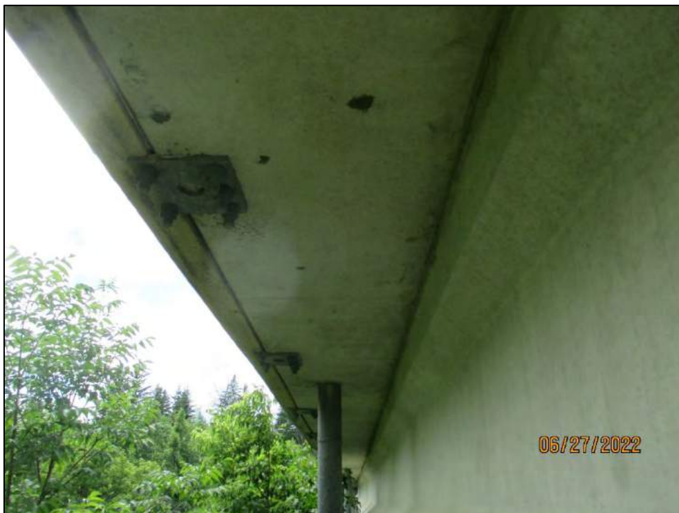
Deck Exterior Soffit – Note: Barrier Anchorages (Typ.)
