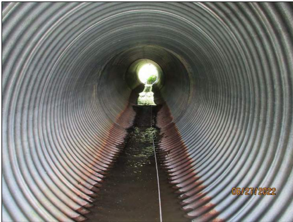
Culvert Barrel (looking North) – Note grade breaks
