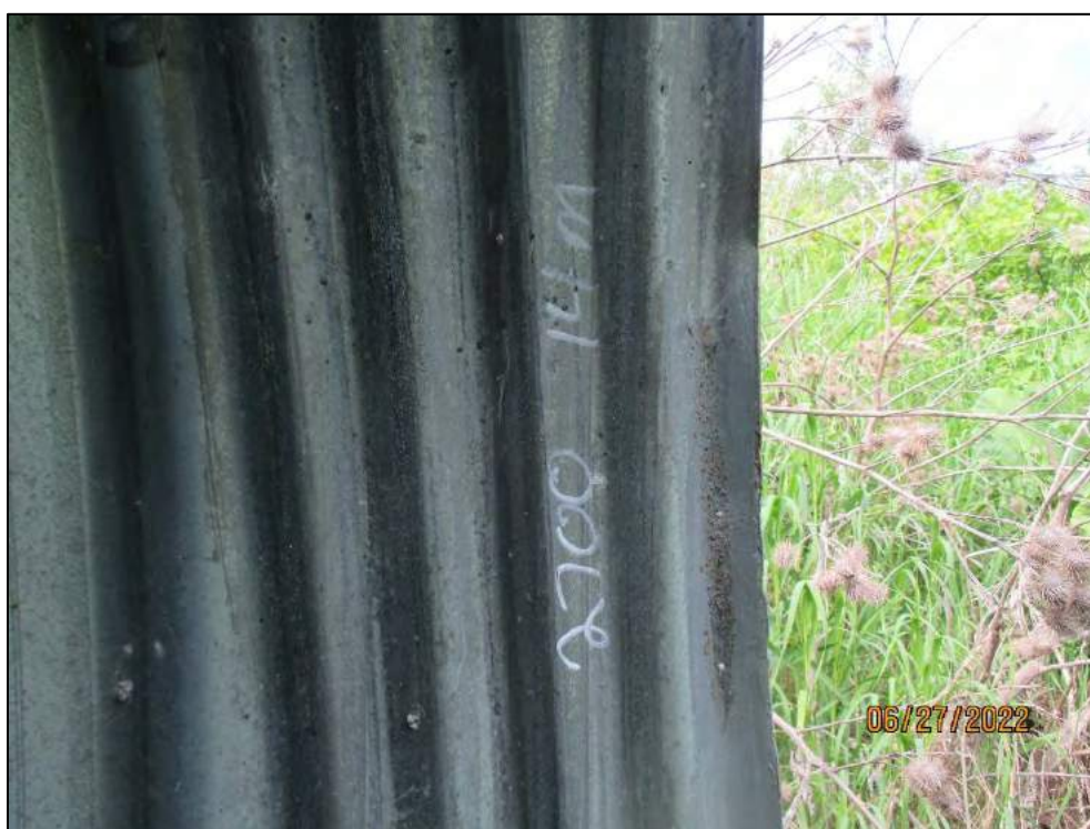
Culvert Barrel (2700mm Dia. – 2.8mm Thickness)
