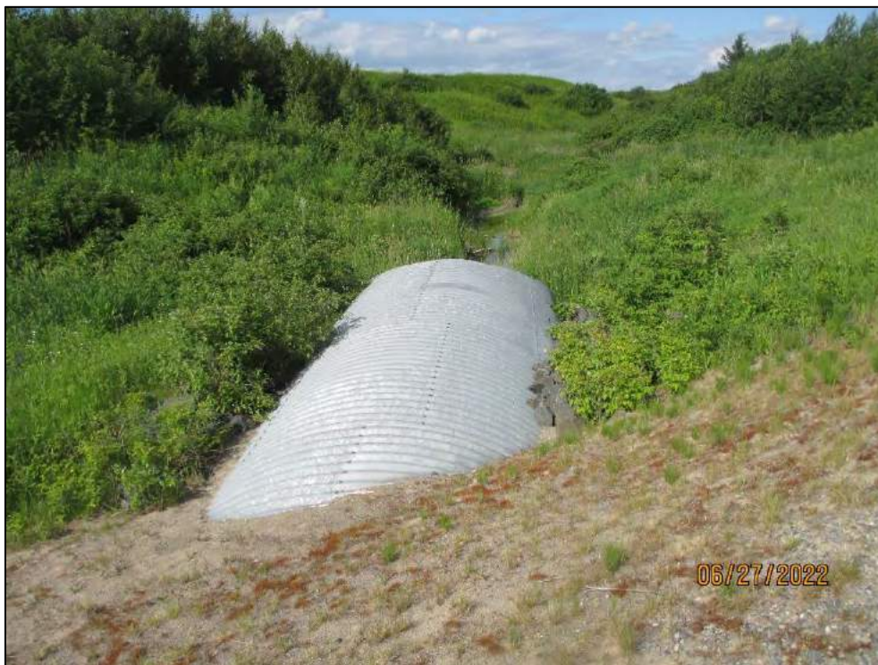
North (Inlet) Projecting End
