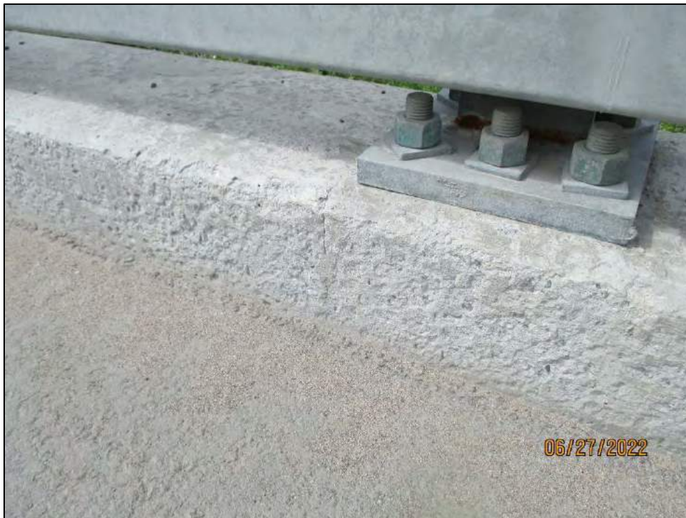
Concrete Scaling – North Curb (Typ.)
