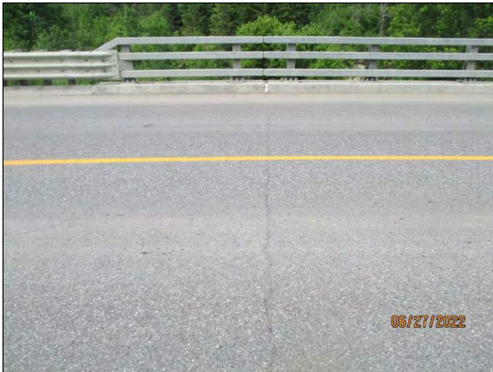
Deck End / Approach Slab (Cracking in Asphalt) – Typ.
