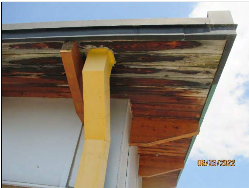
Dry Rot in Soffit Timbers (Typ. (South Roof Edge)
