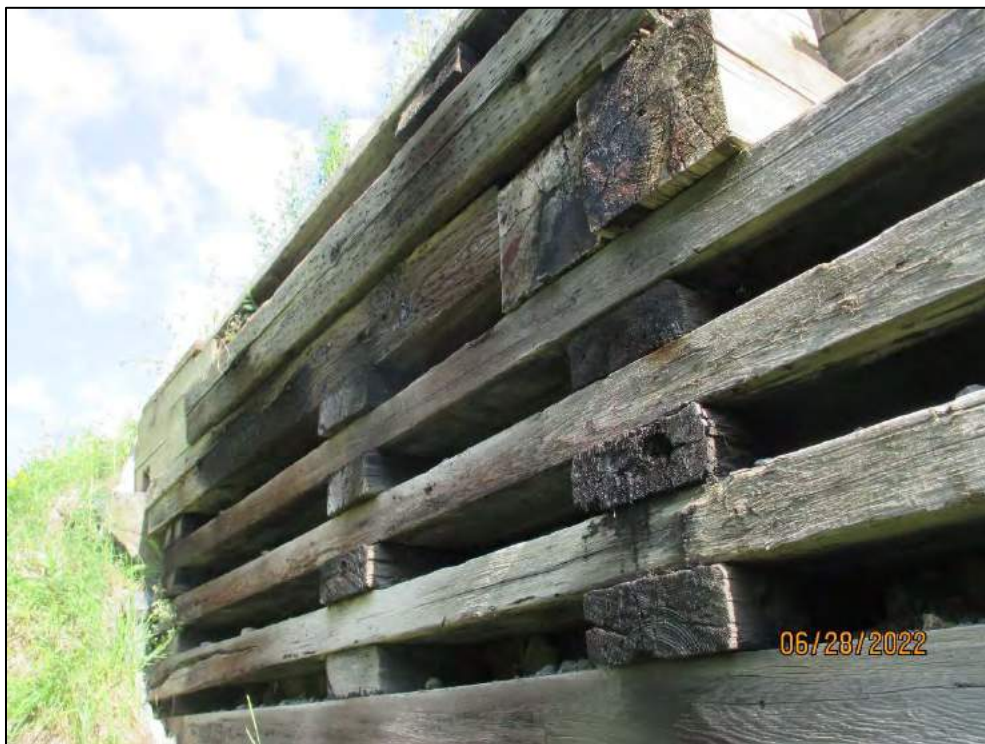
Bulging upper section of retaining wall
