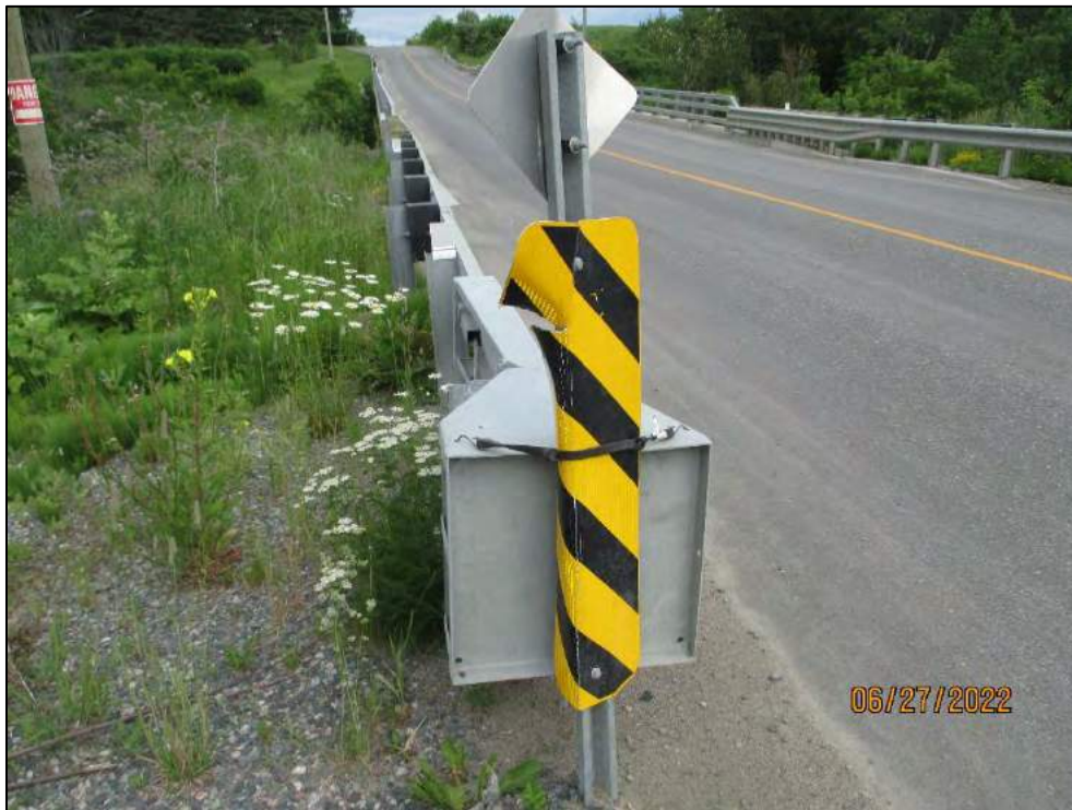
SBGR End Treatment (Torn Hazard Marker)
