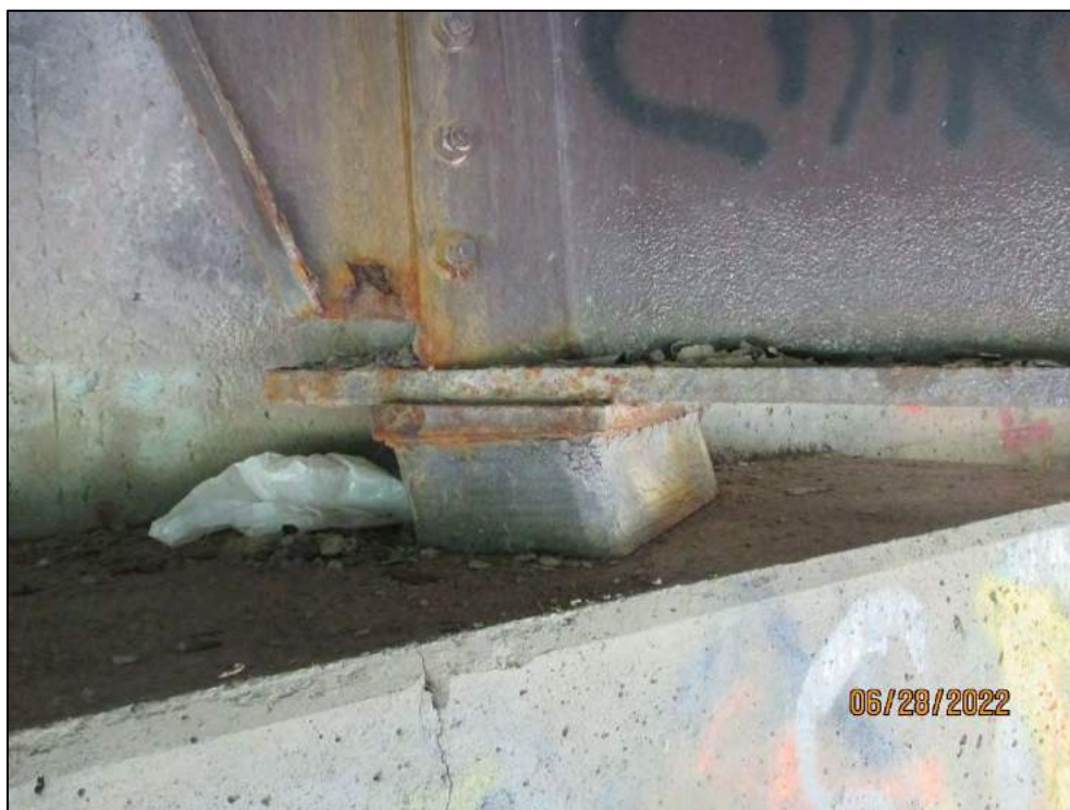
North Abutment Bearing (Typ.)
