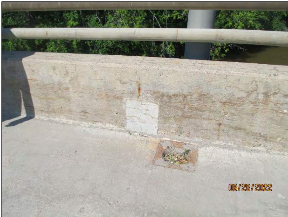
West Sidewalk / Parapet – Note: Deteriorated Junction Box Cover Plate
