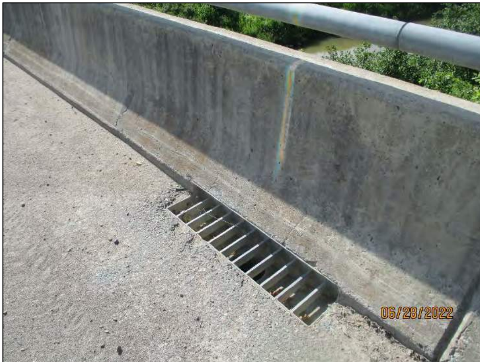
Deck Drain and Barrier (Typ.)
