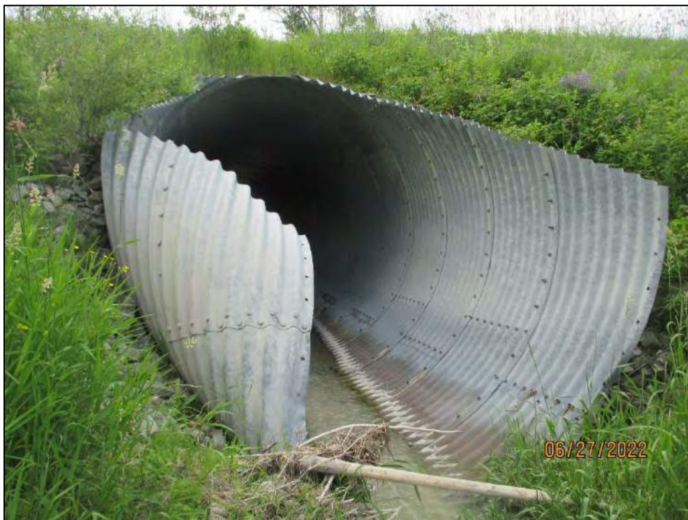
East (Inlet) Culvert Barrel Damage
