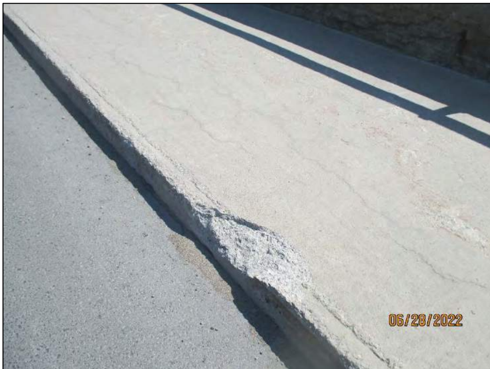
Scaling and Spall – East Sidewalk/Curb
