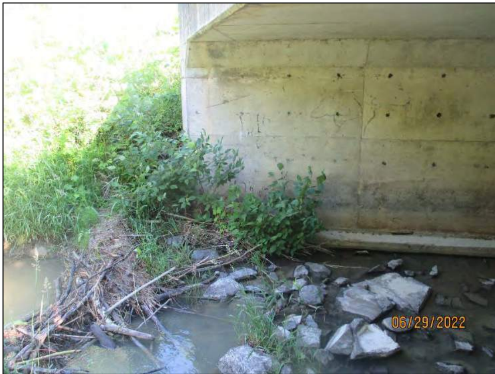
Debris / Blockage at Inlet
