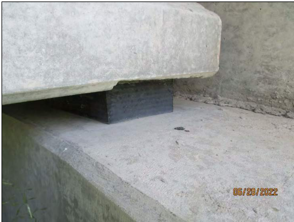
Girder End / Bearing (Typ.)
