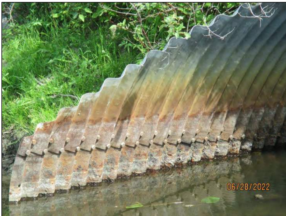
Culvert Barrel (corrosion and uplift at outlet) – Typ.
