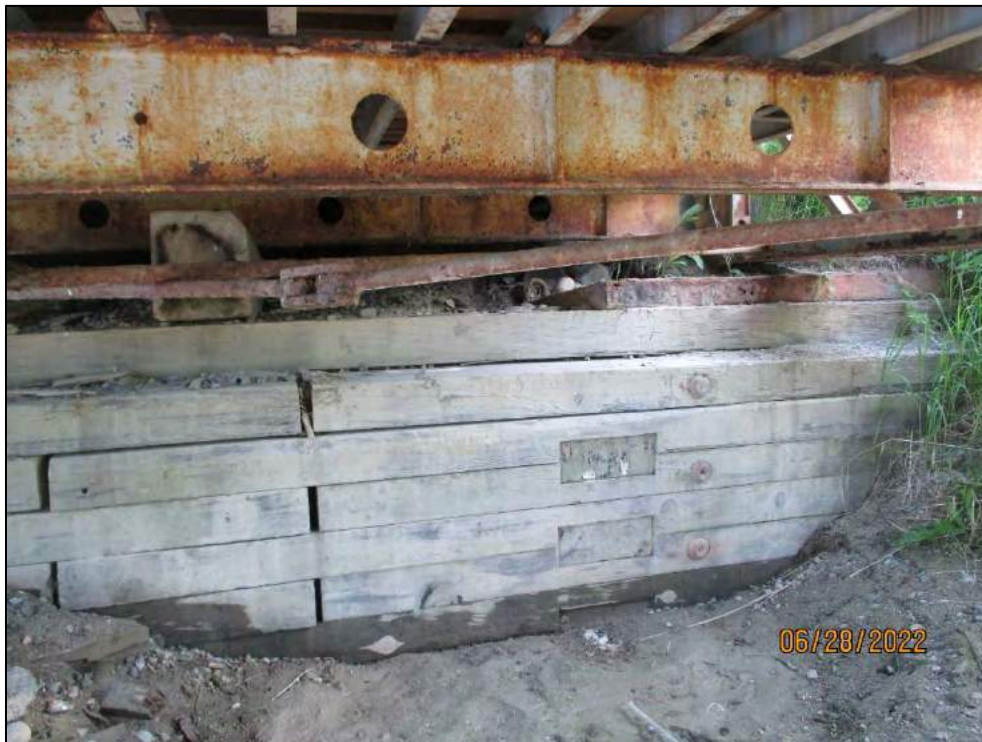
North Abutment (Timber Crib)
