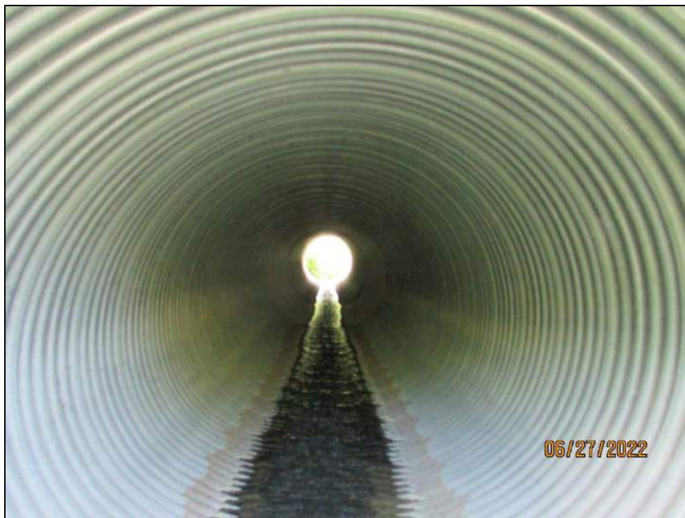
Culvert Barrel (Typ.)
