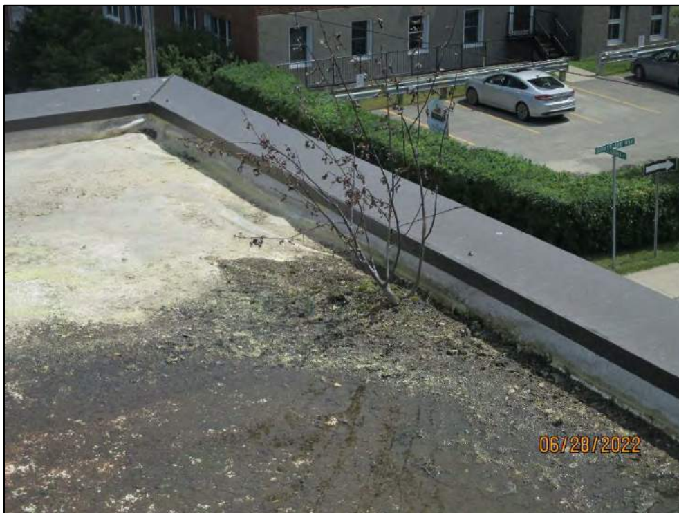
South (Upper) Flat Roof – tree to be removed
