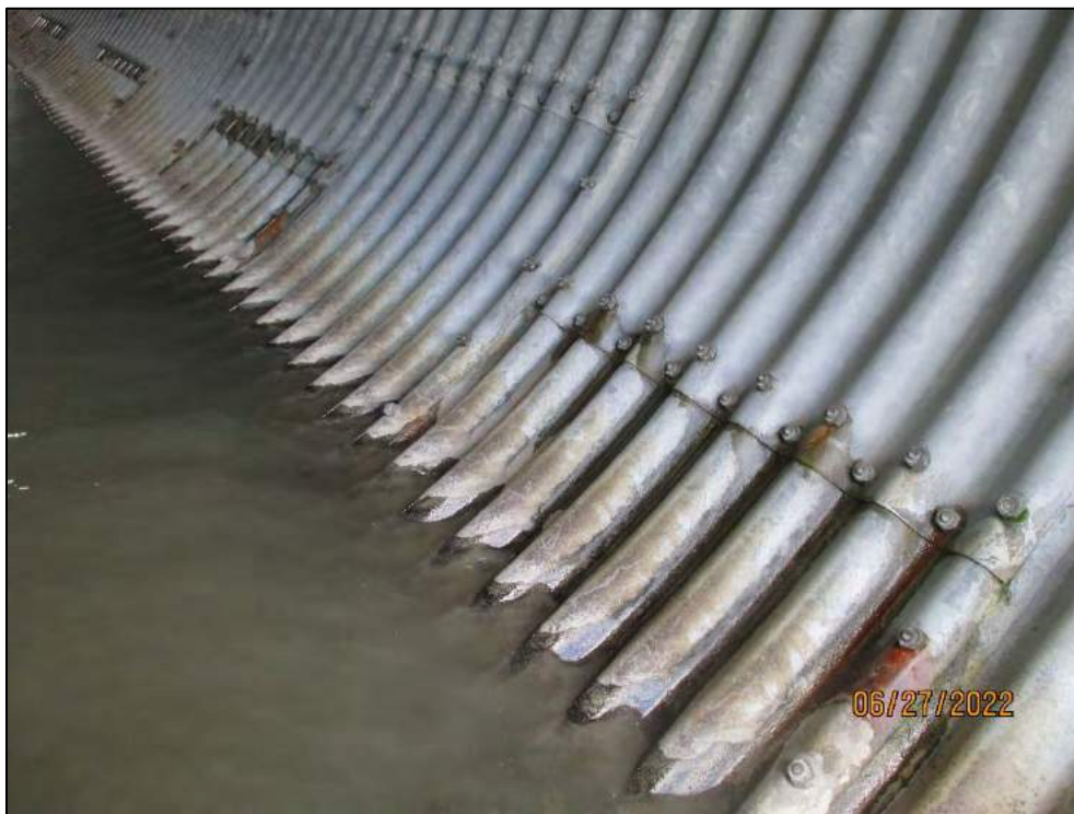
Culvert Barrel (minor corrosion at bolt seams)
