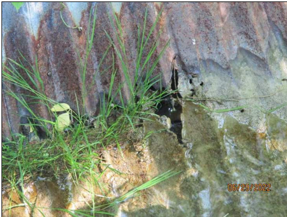
Culvert Barrel (Outlet) – Perforated Invert
