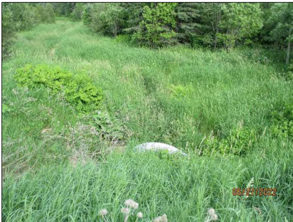
Culvert projecting end
