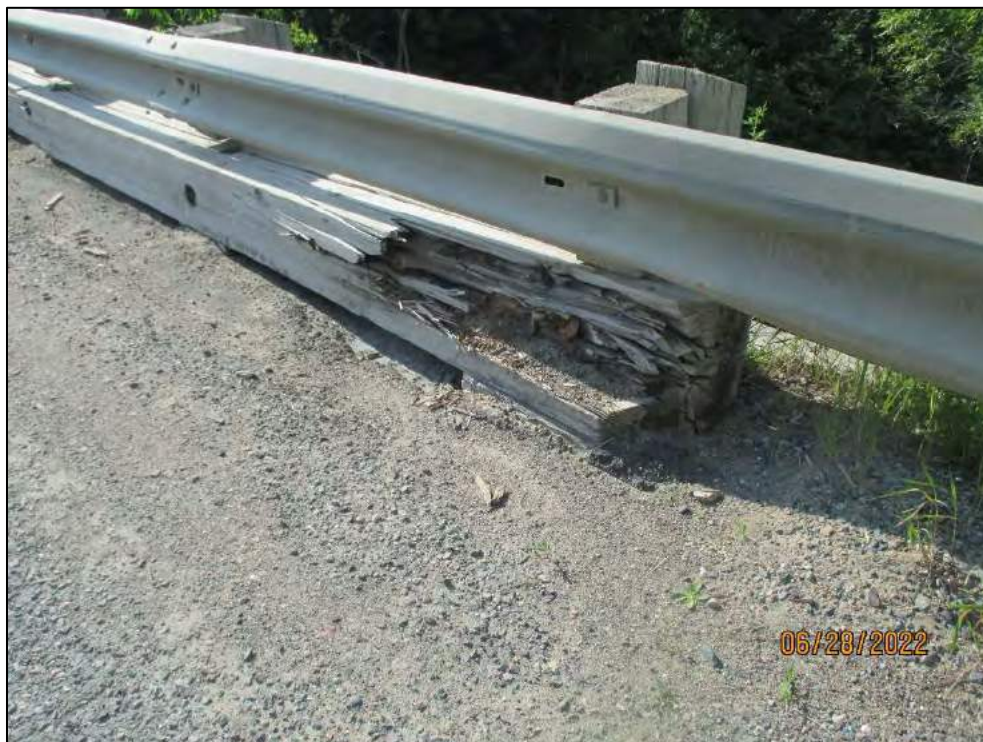
Curb damage at S/W
