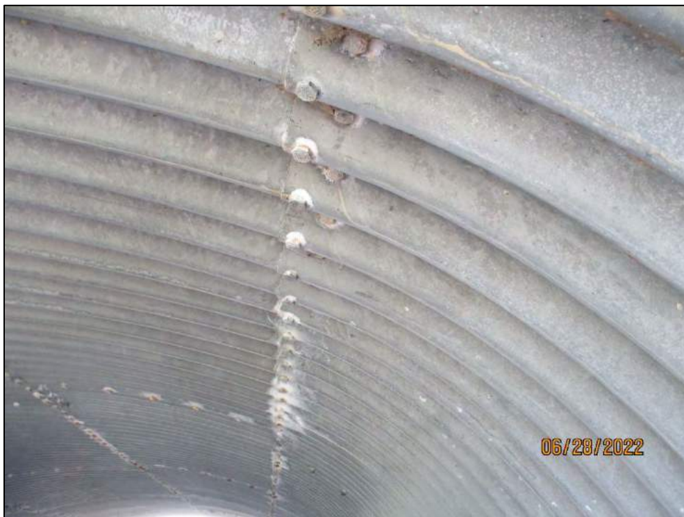
Barrel Obvert (Bolt Seam) – Typ.
