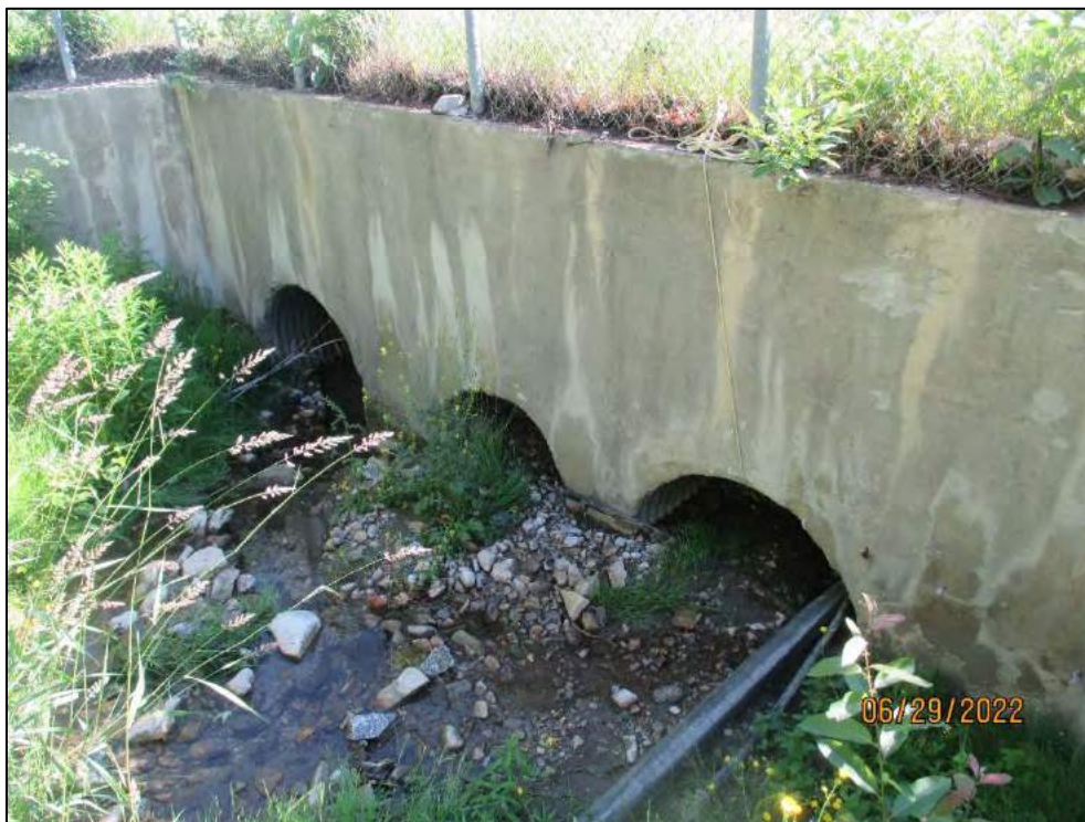
Culvert Headwall (Inlet)
