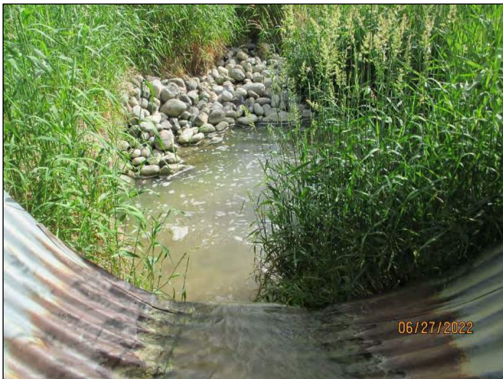
View South from Barrel (deep scour)
