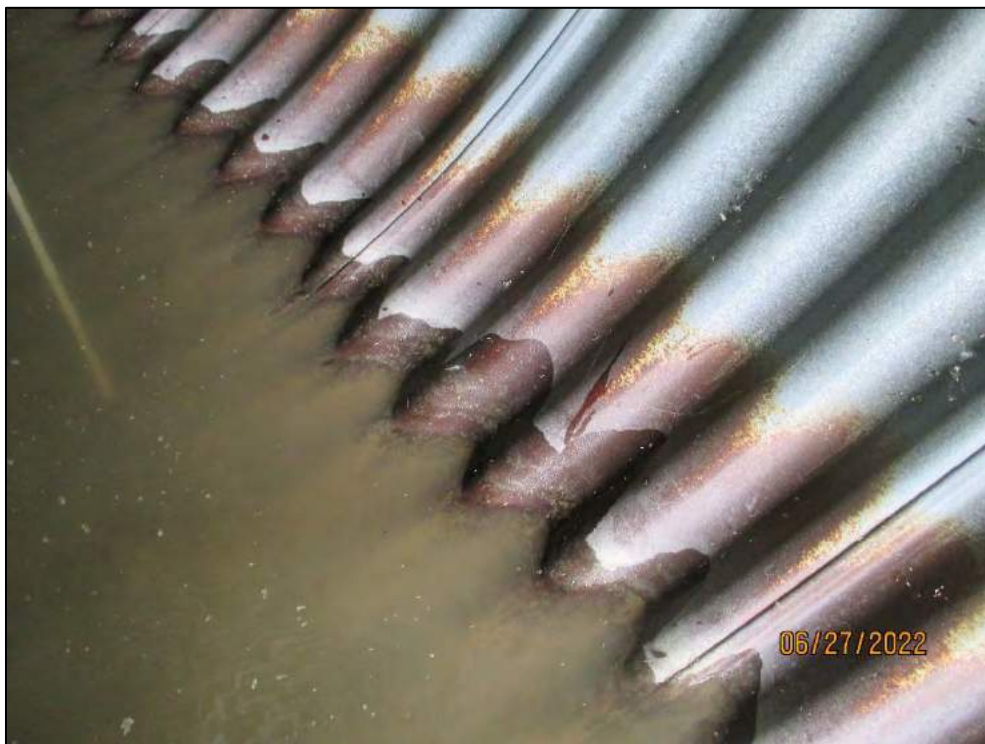
Minor Corrosion at Waterline
