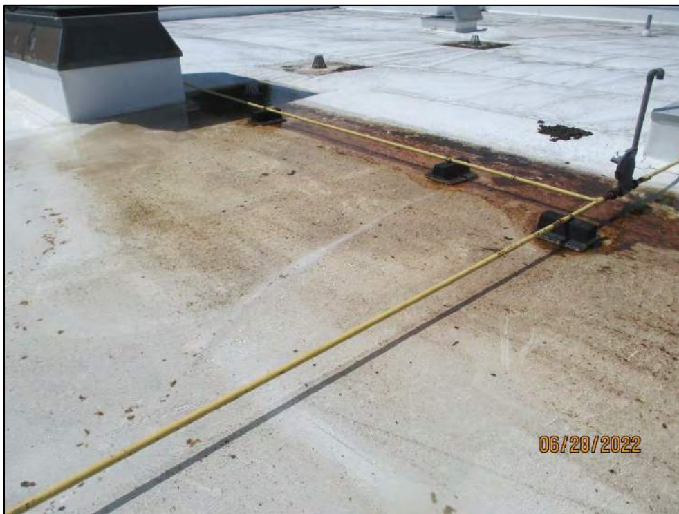
North Roof (water ponding at blocked drain)
