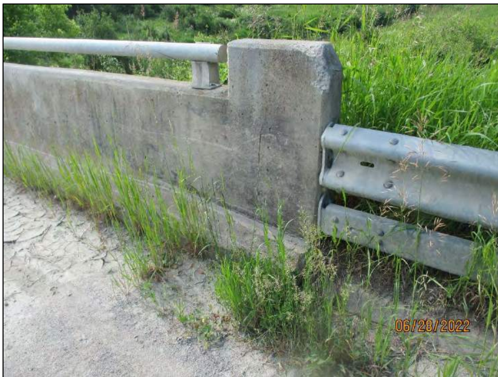
SBGR / Barrier Connection (Typ.)
