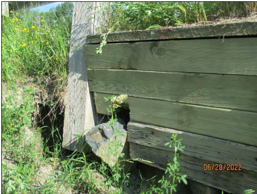
Displaced SBGR Port and rotating Retaining Wall section
