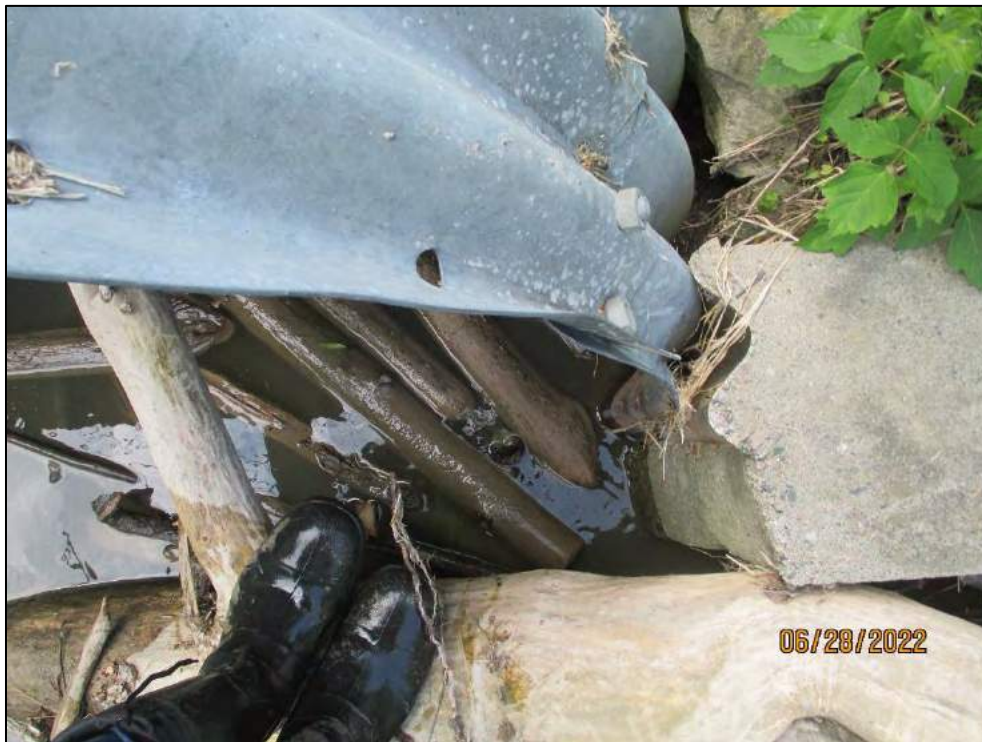
Culvert Damage (pulled from cut-off wall at inlet)
