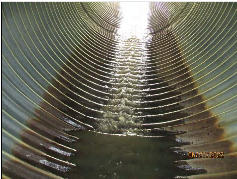
Culvert Barrel (looking South) – Note grade breaks
