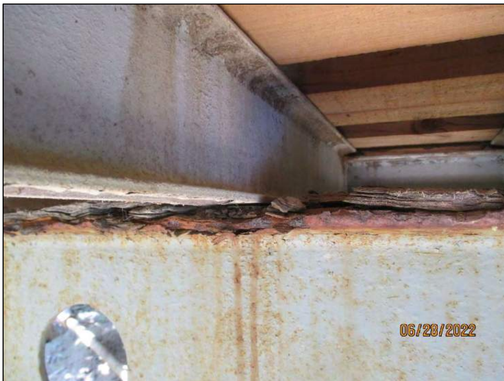
Transom / Floor Beam – Top Flange Corrosion (Typ.)
