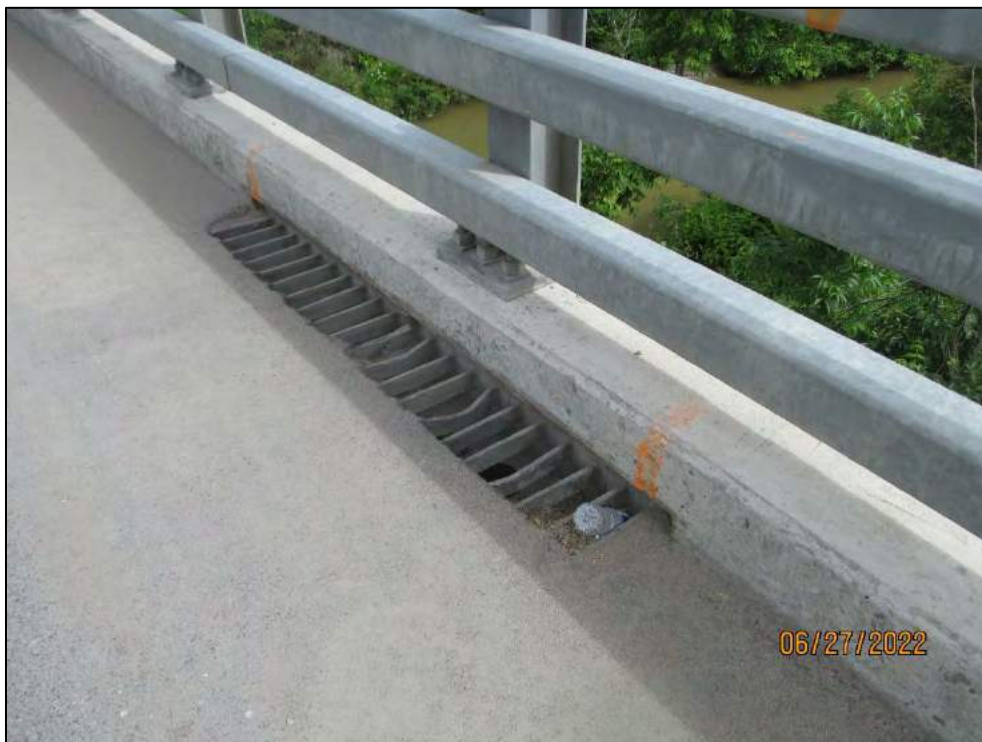
Deck Drain (Double Shown) – Curb – Barrier (Typ.)
