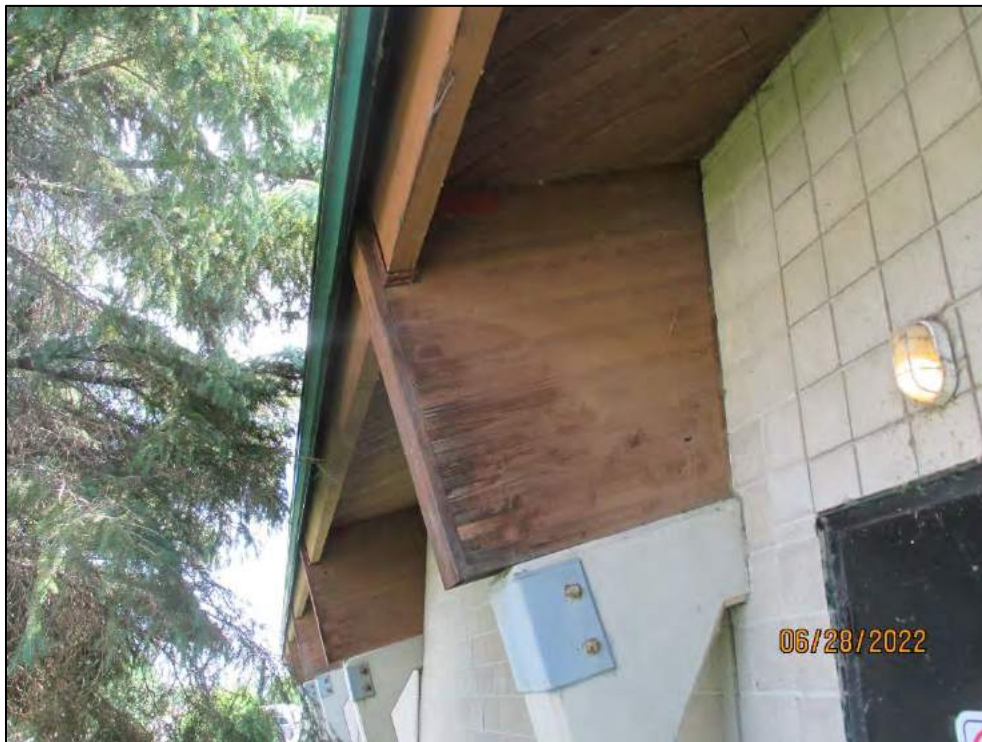
Projecting Glulam Roof Beams – Typ. (North Wall)
