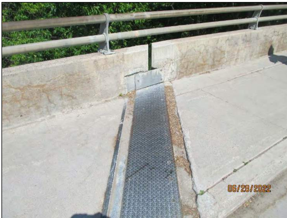
Expansion Joint (Cover Plate) – N/W (Missing Grout)
