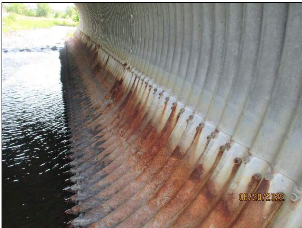
Barrel Corrosion (Typ.)
