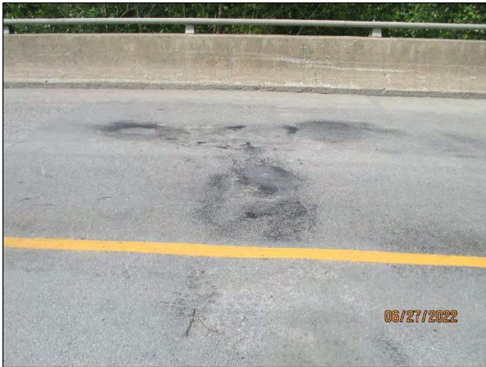
Deck Top- Wearing Surface Defects
