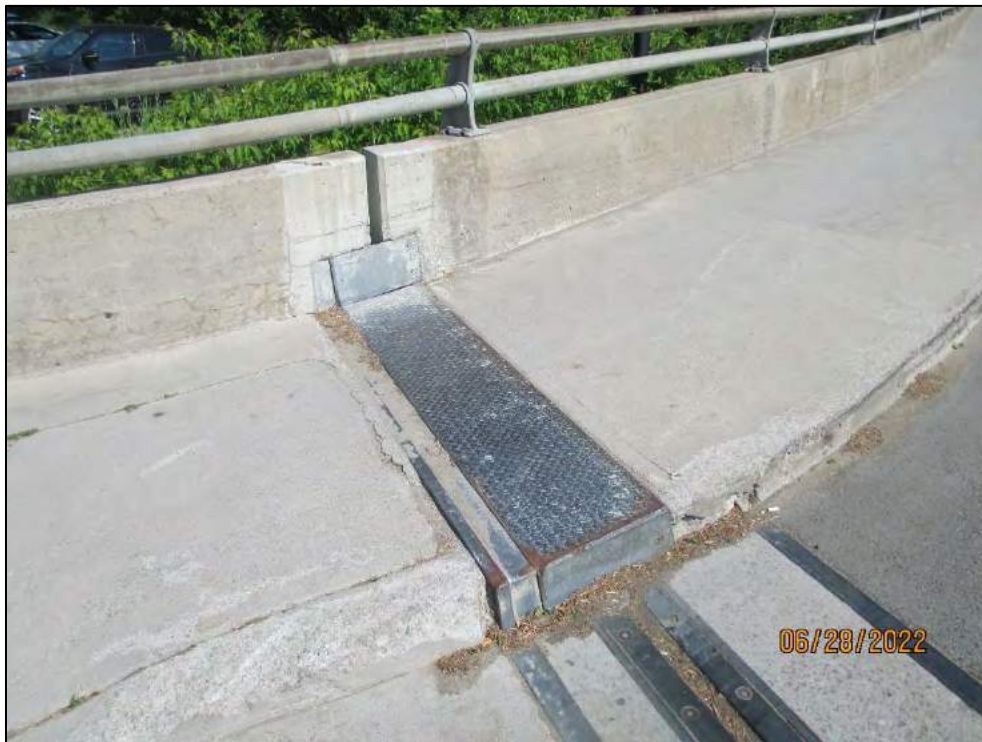
Expansion Joint (Cover Plate) – S/W
