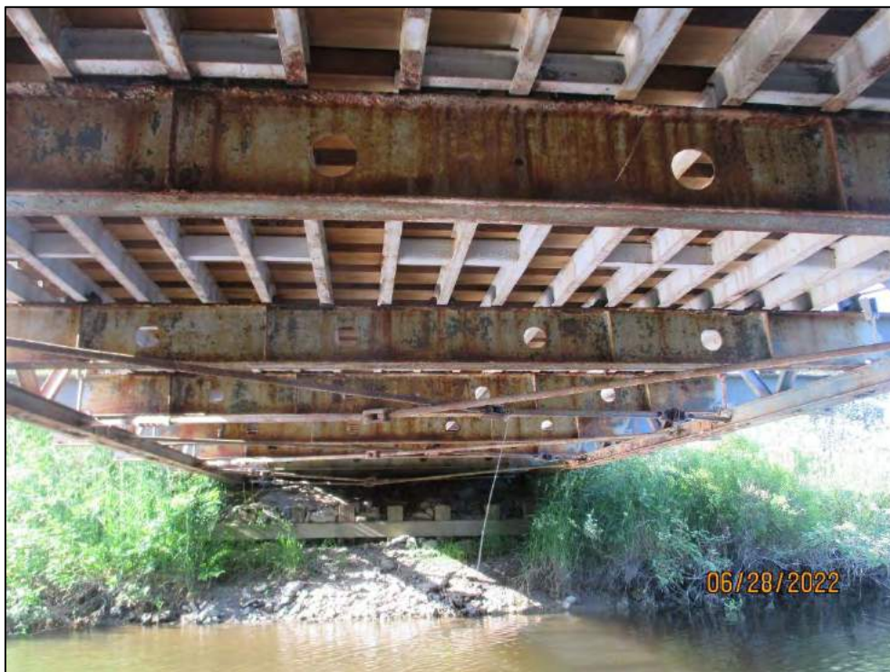
Underside of Bridge (Stringers & Bracing) – Typ.
