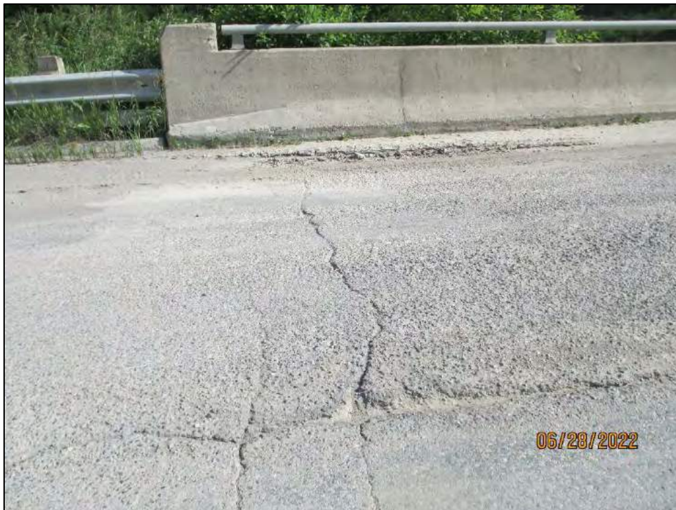
Approach Slab (West) – Potential Settlement
