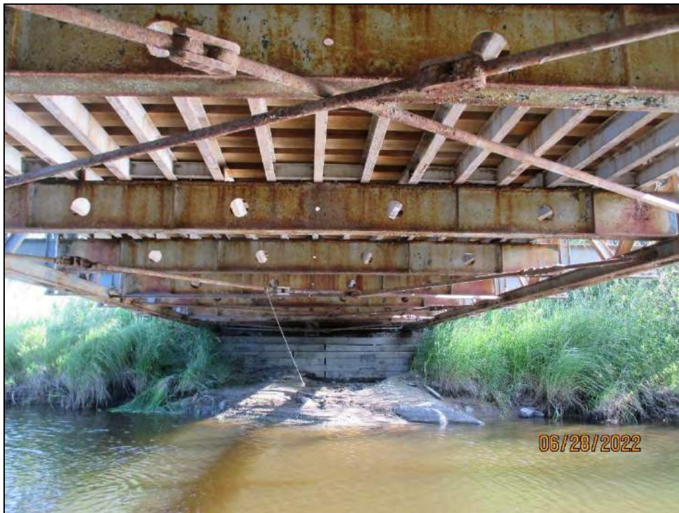
Underside looking north – Note: Coating Condition
