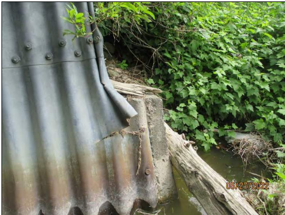
West (Inlet) Cut-Off Wall and Impact Damage to Culvert Barrel
