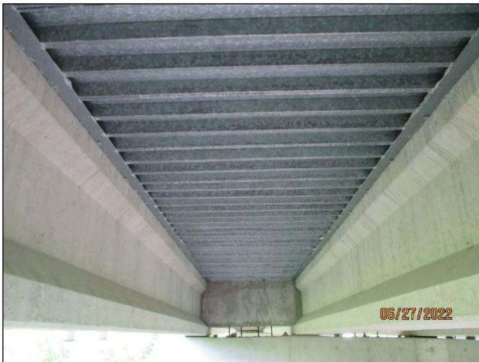
Deck Soffit (Interior) – Note: Stay-In-Place Form (Typ.)
