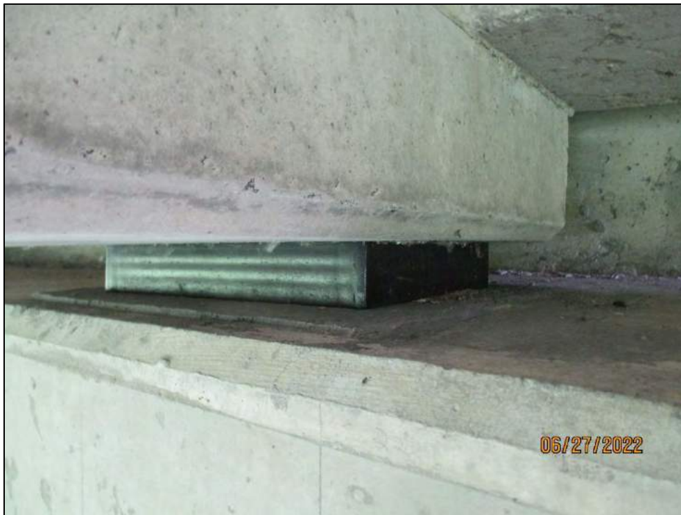
Abutment Bearing (Typ.)
