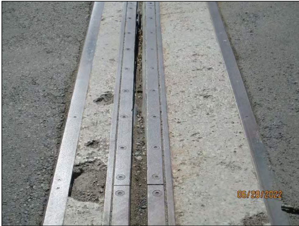
Expansion Joint (North) - Torn Seal and End Dam Deterioration
