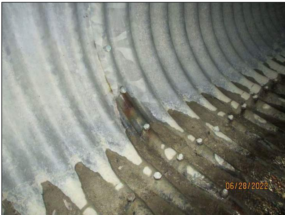
West Barrel (leakage at bolt seam)
