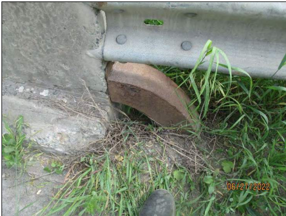
Utility Duct Sweep – South Wingwalls (Each End)
