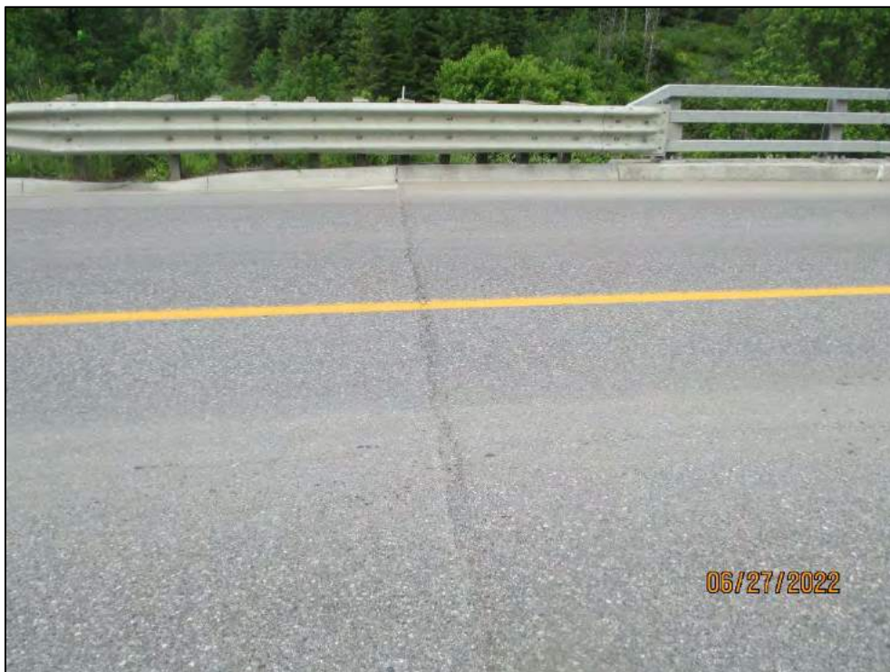
End of Approach Slab (Cracking in Asphalt) – Typ.
