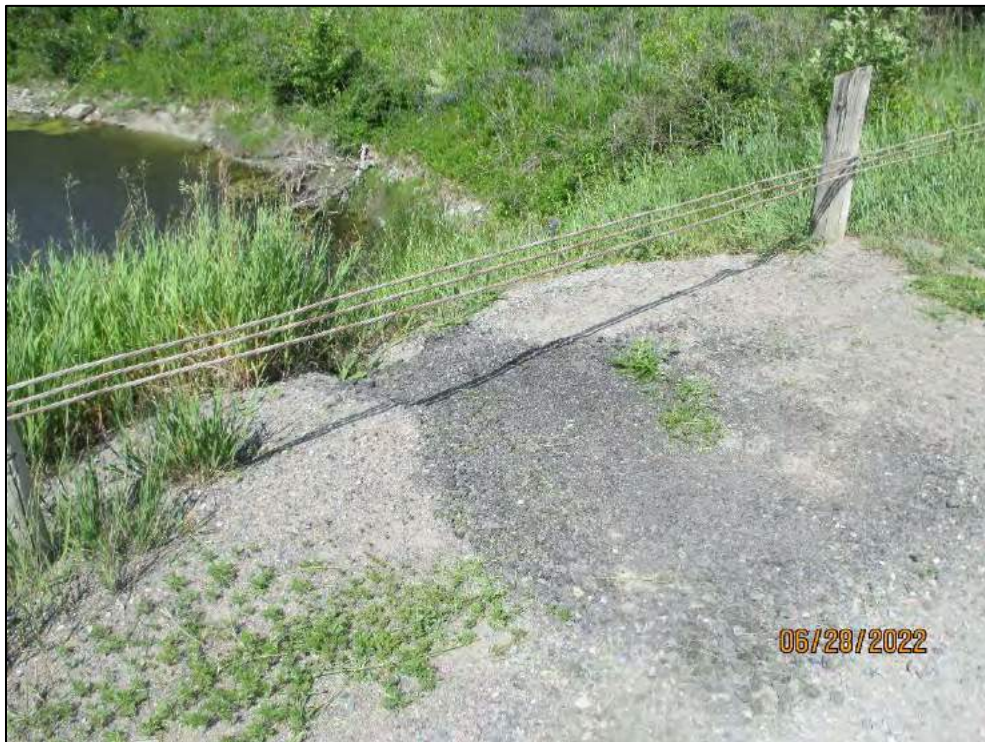
Shoulder Washout over Barrel (North)
