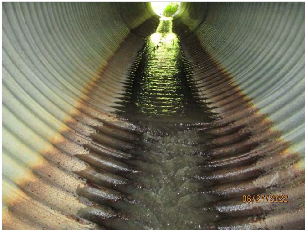
Culvert Barrel (looking North) – Note grade breaks
