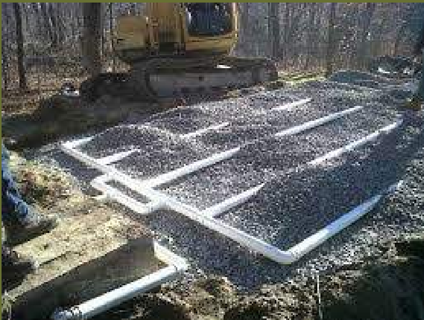
A typical class 4 septic system under construction
