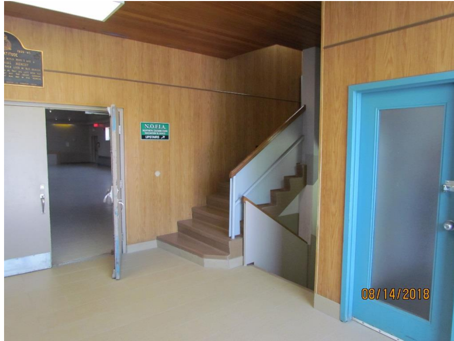
Photograph 11: Lobby view looking south west to stairwell. Note fire separation required between exit stair and lobby.
