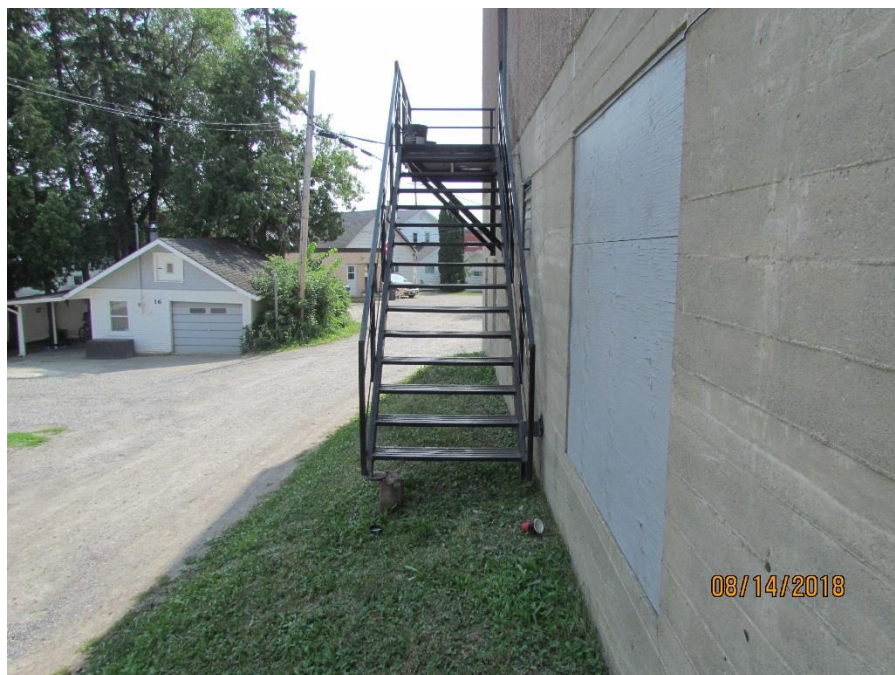
Photograph 6: East auditorium exit stair. Note left concrete foundation.
