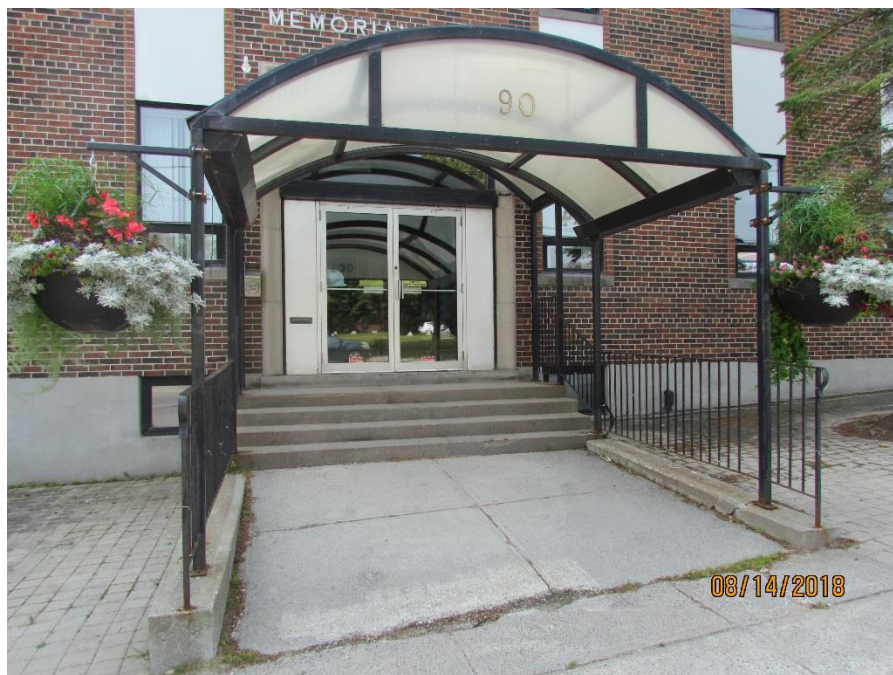
Photograph 4: Main building entrance/exit. Note level change to main floor is five (5) exterior steps and three (3) interior steps (refer to photograph 7).
