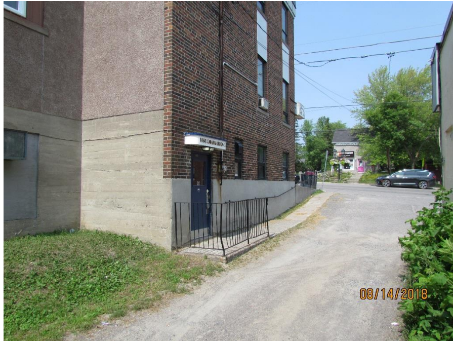
Photograph 5: Legion Hall entrance/exit (view from side alley). Note entrance is three (3) steps above the floor level of the hall. Note ramp concrete sidewalk (ramp) are not within the property limits.
