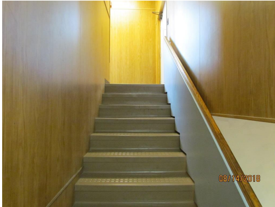
Photograph 13: Main stairwell view to second storey. Note fire separation required between exit stair and other parts of second storey.
