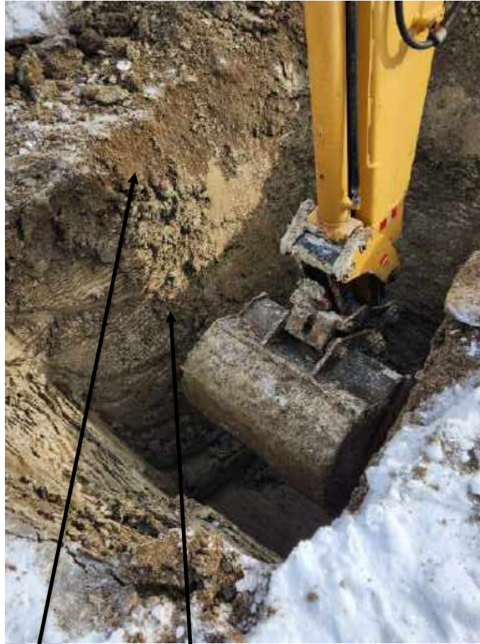
Photo #5- The Soil Strata of granular fill and the Brown Varved clay at 8ft to 10ft.
