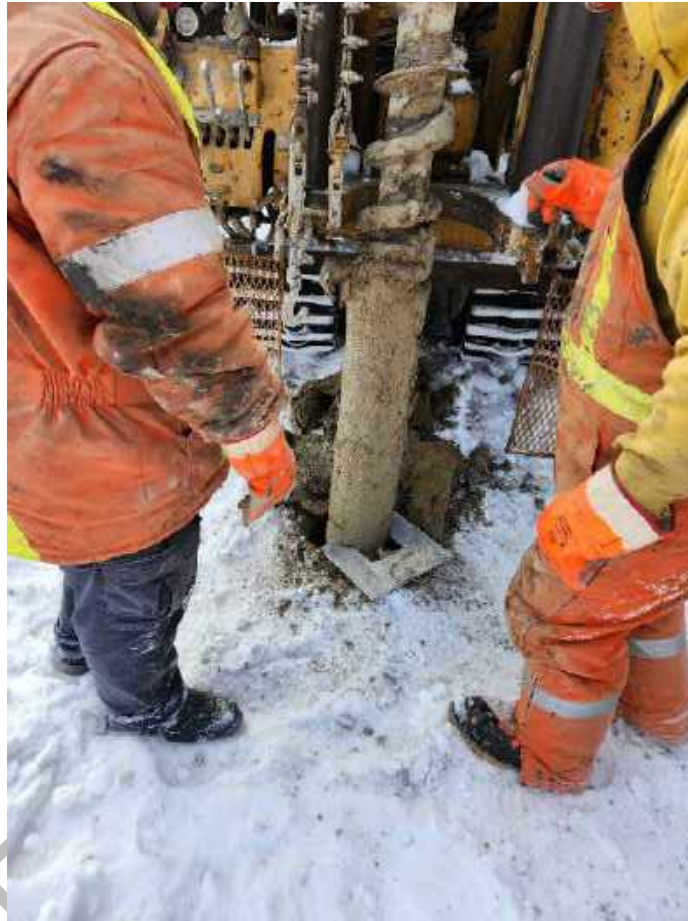
Photo 4- Soil Layers. Brown - Varved clay at 8 to 10 ft. depth showing the depth at Borehole #2
