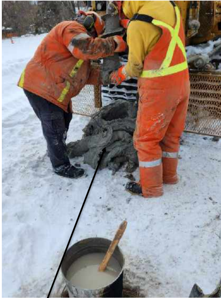
Photo #5- The blue clay being pushed up from the auger a 10ft to 12ft. depth. Borehole #2
