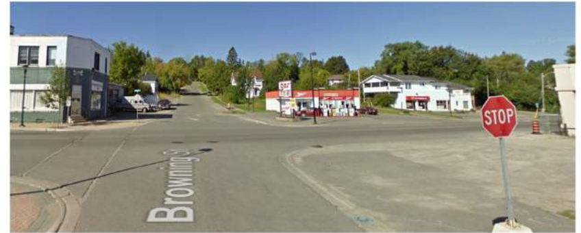
Example of a two-way stop-controlled intersection (Browning St and Lakeshore Rd) in Haileybury displaying a lack of clear pavement markings for stop bars, centerlines etc. and having no dedicated space for pedestrian crossings
