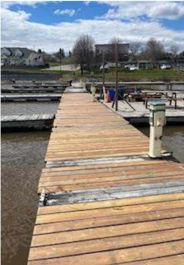
Figure 3 – Replaced decking along C-dock at the Haileybury Marina
