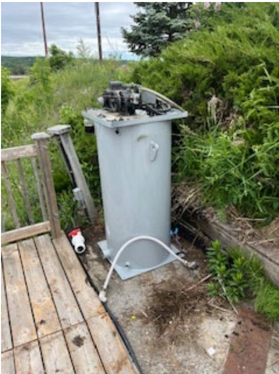
Figure 3 – TriTown Welding refurbished the vacuum pump at the New Liskeard Marina
