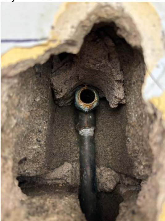
Figure 3 – A damaged pipe is seen in the wall of the Bun Eckensviller Community Hall. City staff repaired the line.
