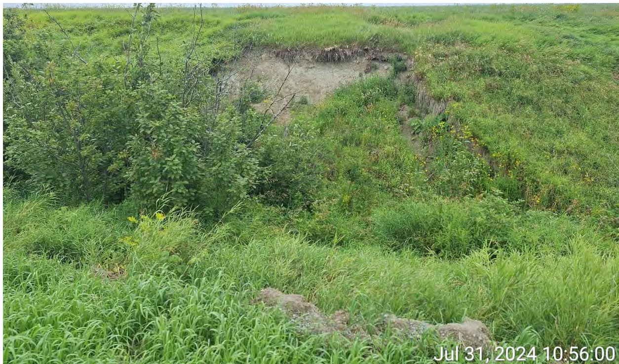
Figure 2 - Slope Failure Across from Outlet
