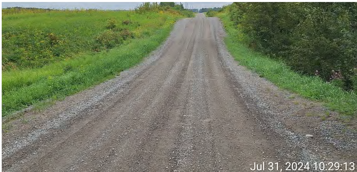
Figure 1 – Gravel Wearing Surface above Culvert
