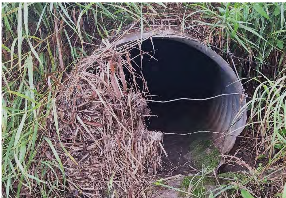
Figure 3 - Wire Fence Across Inlet holding debris
