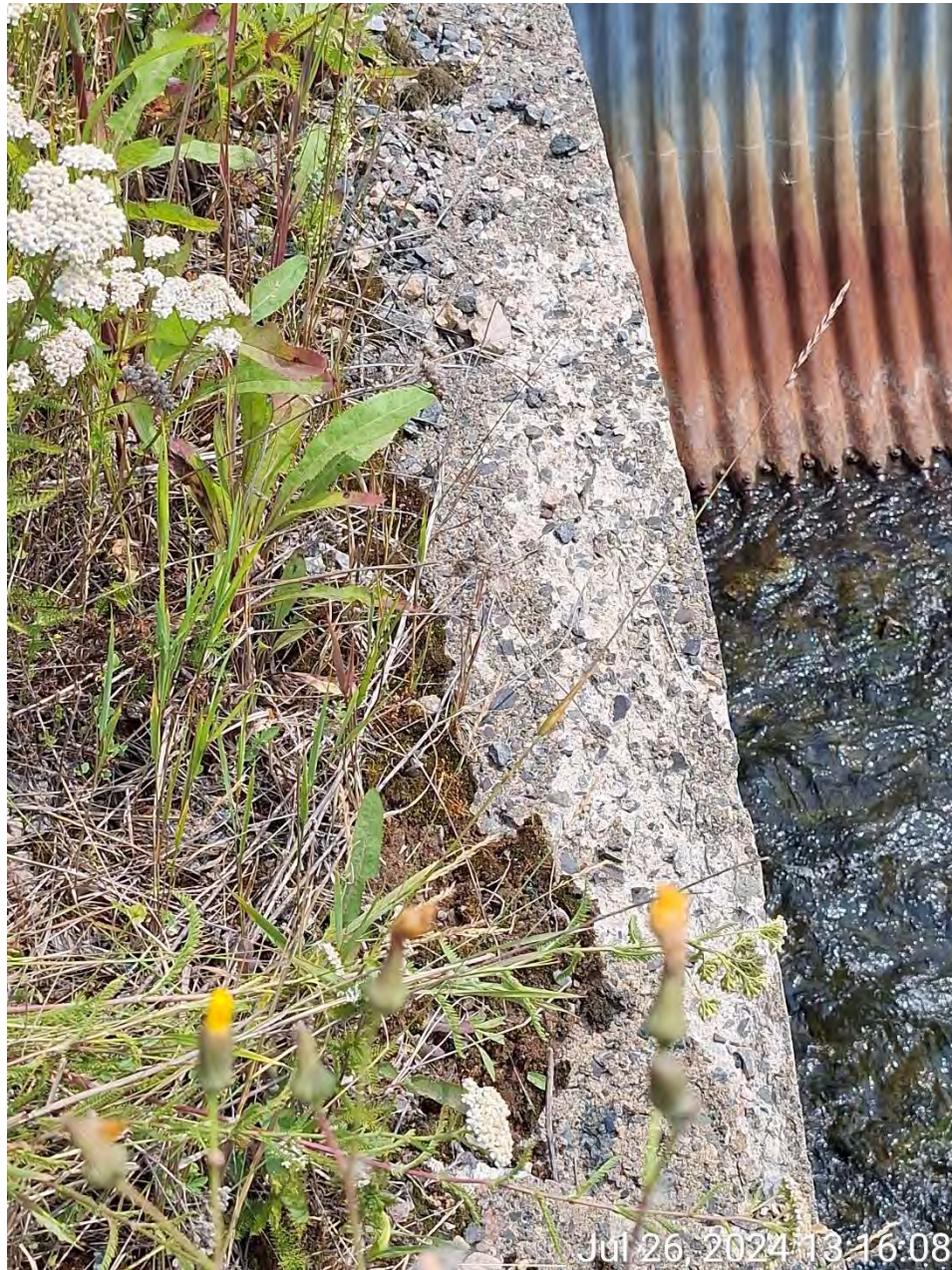
Figure 12: Disintegration of Concrete component.
