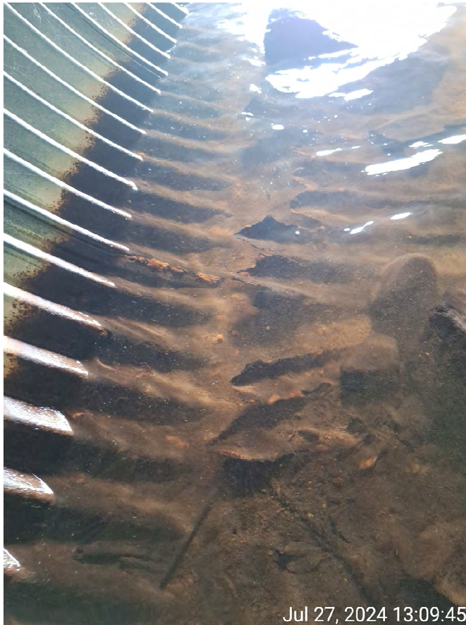
Figure 6: View of torn edge in bottom of culvert
