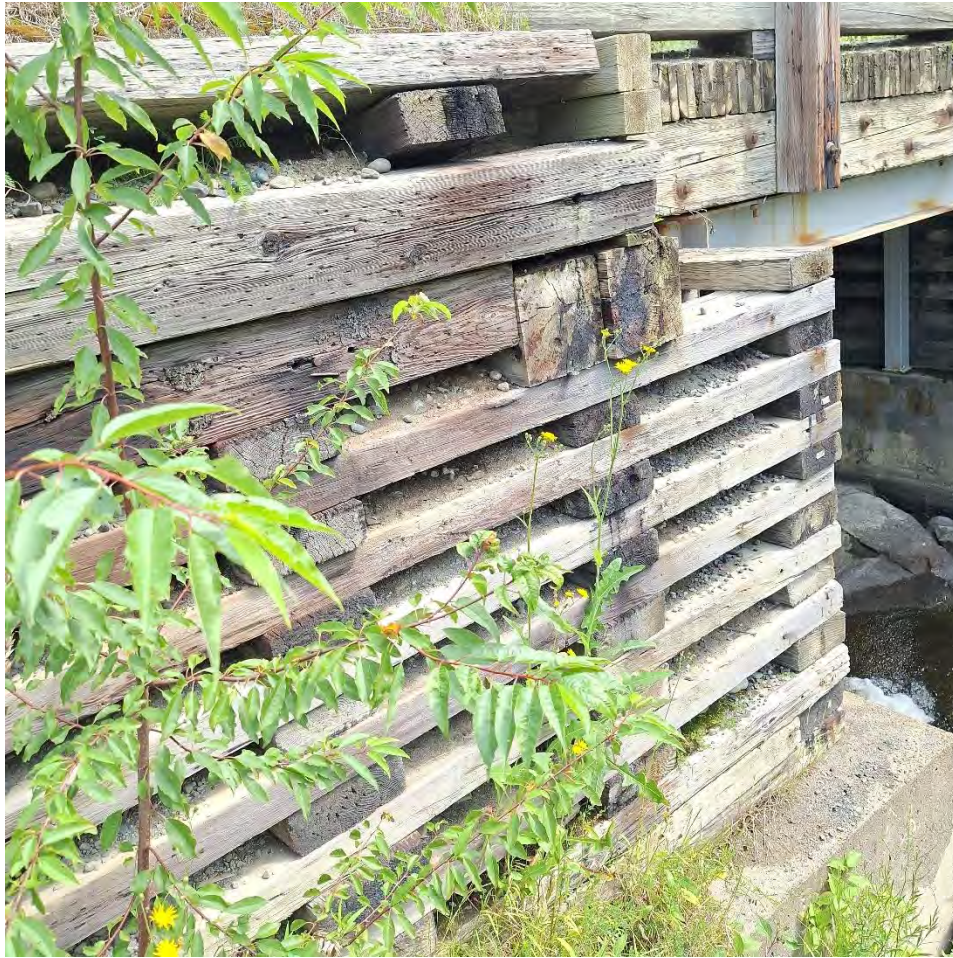
Figure 8 – Timber Crib
