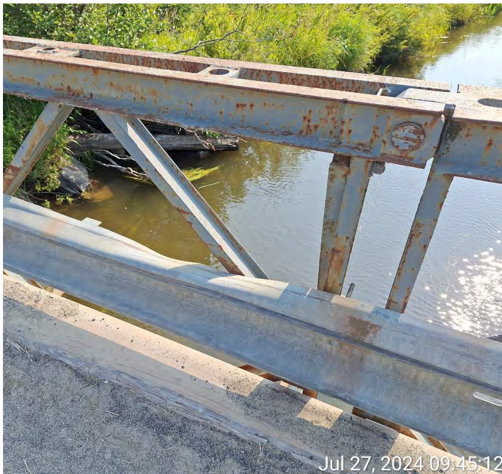
Figure 24: Connection (pin) showing surface corrosion.
