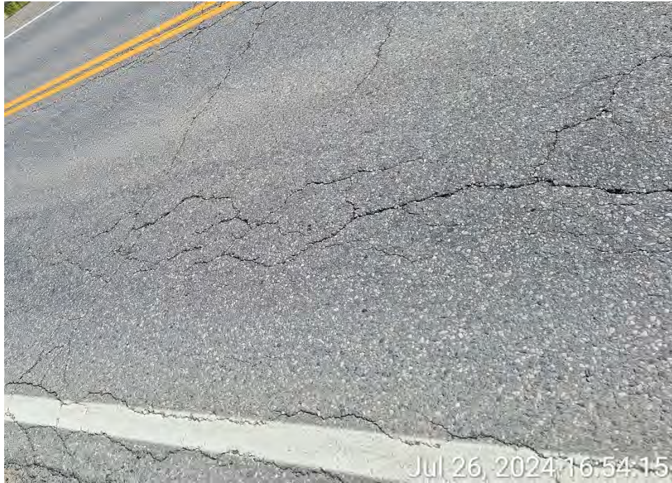
Figure 13 - Cracks in Wearing Surface
