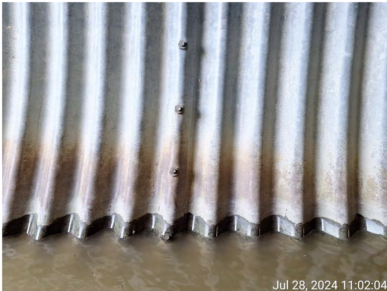
Figure 9: Light corrosion above waterline
