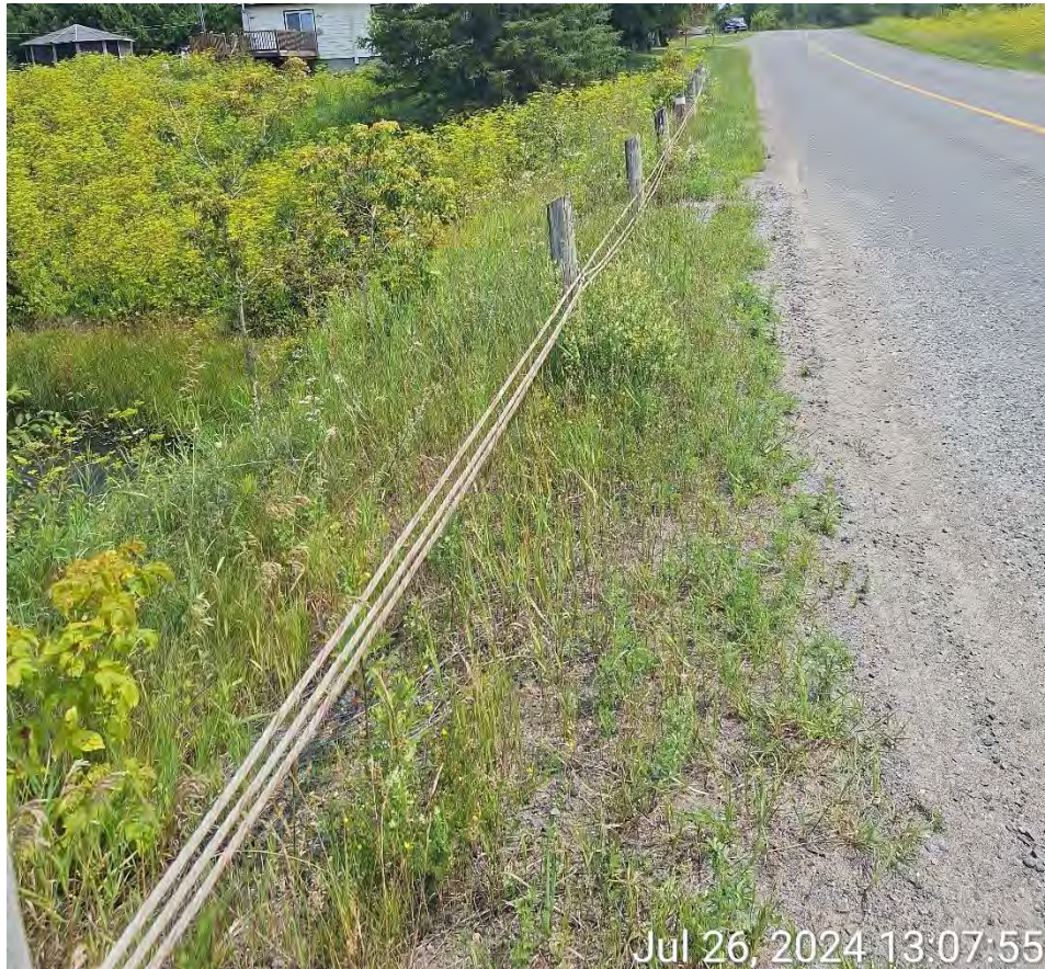
Figure 2 - 3 Cable Guide Rail – some sag in cable shown
