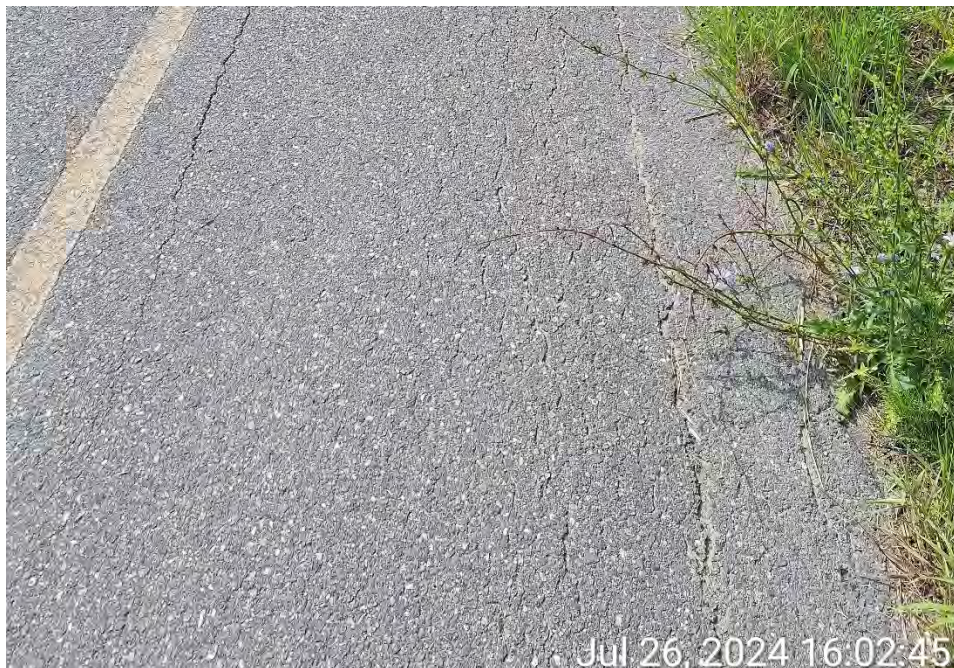
Figure 22 - Cracks in pedestrian path (sidewalk)
