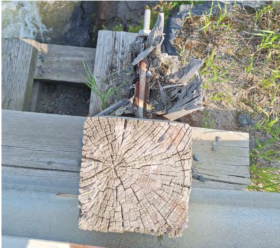
Figure 14 - Damaged Wooden Guide Rail Post
