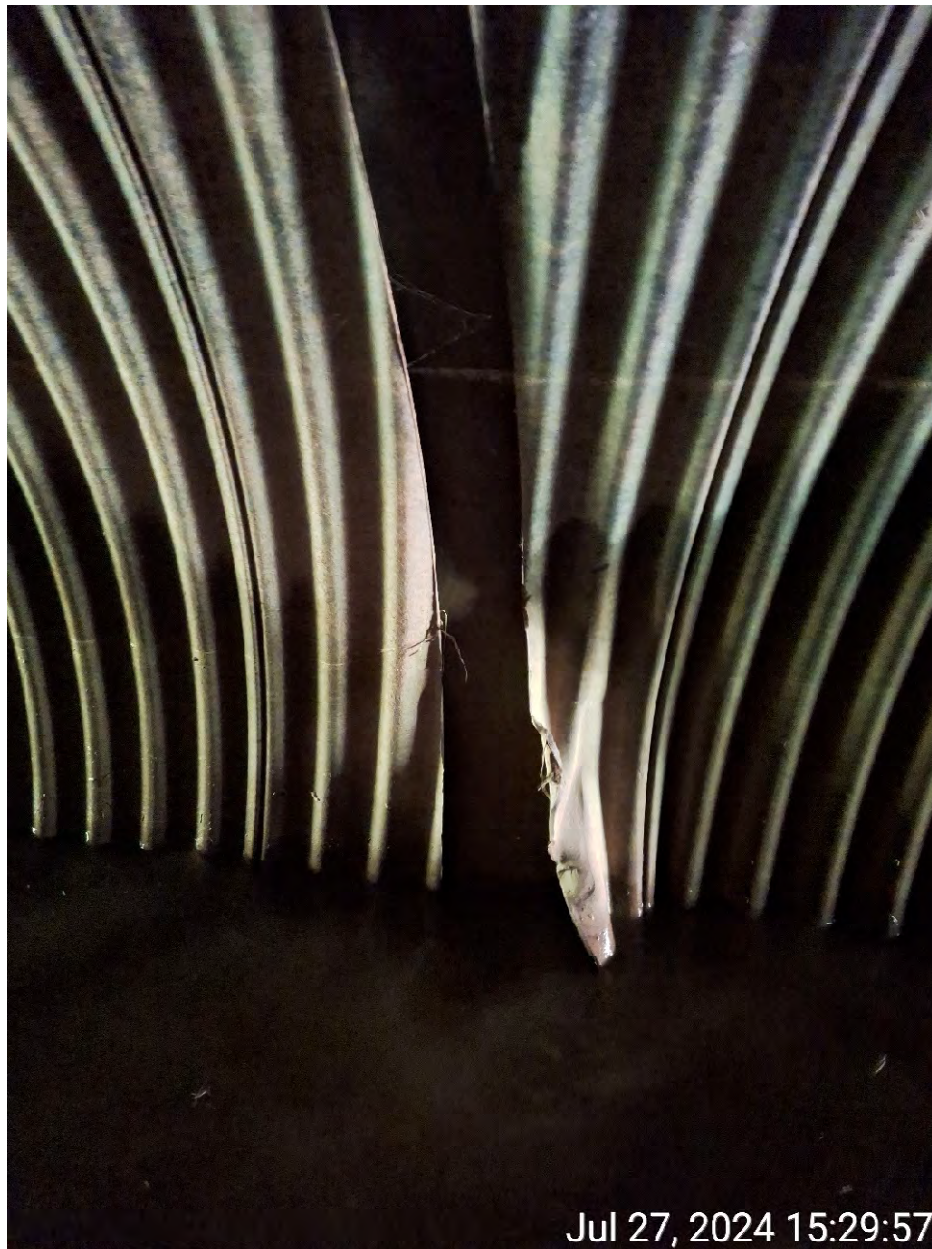
Figure 11: Deformation of a barrel end at a joint.
