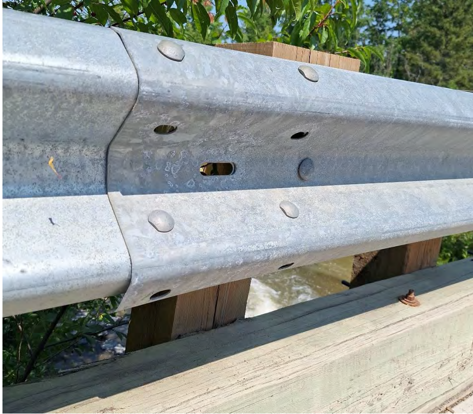
Figure 17 - Flared Rail also Missing Bolts
