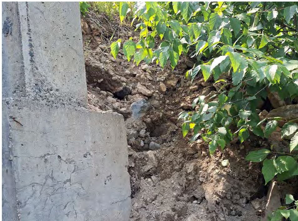
Figure 2 - Erosion on North Embankment
