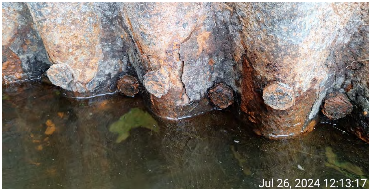
Figure 6 - Severe Corrosion of barrel and bolts at Waterline.
