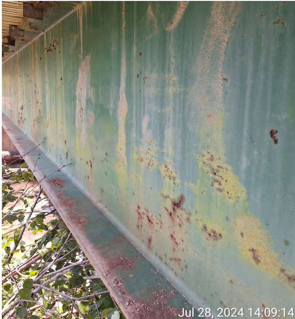
Figure 7 - Failed Coating and Corrosion on Steel Girders
