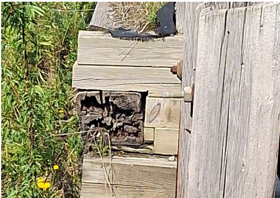
Figure 6 – Wood experiencing severe rot in wingwall
