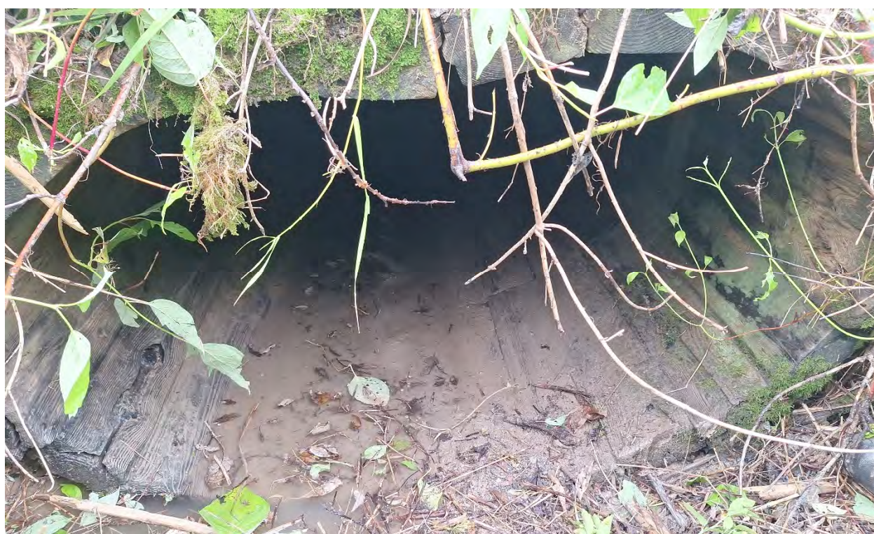
Figure 6 – Inlet, with some debris cleared away
