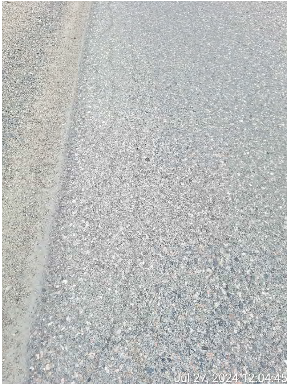
Figure 10: Edge cracking in asphalt pavement
