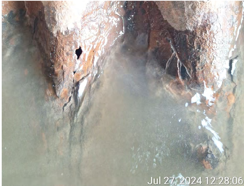
Figure 2 – hole through the bottom of the barrel which was a result of severe corrosion.
