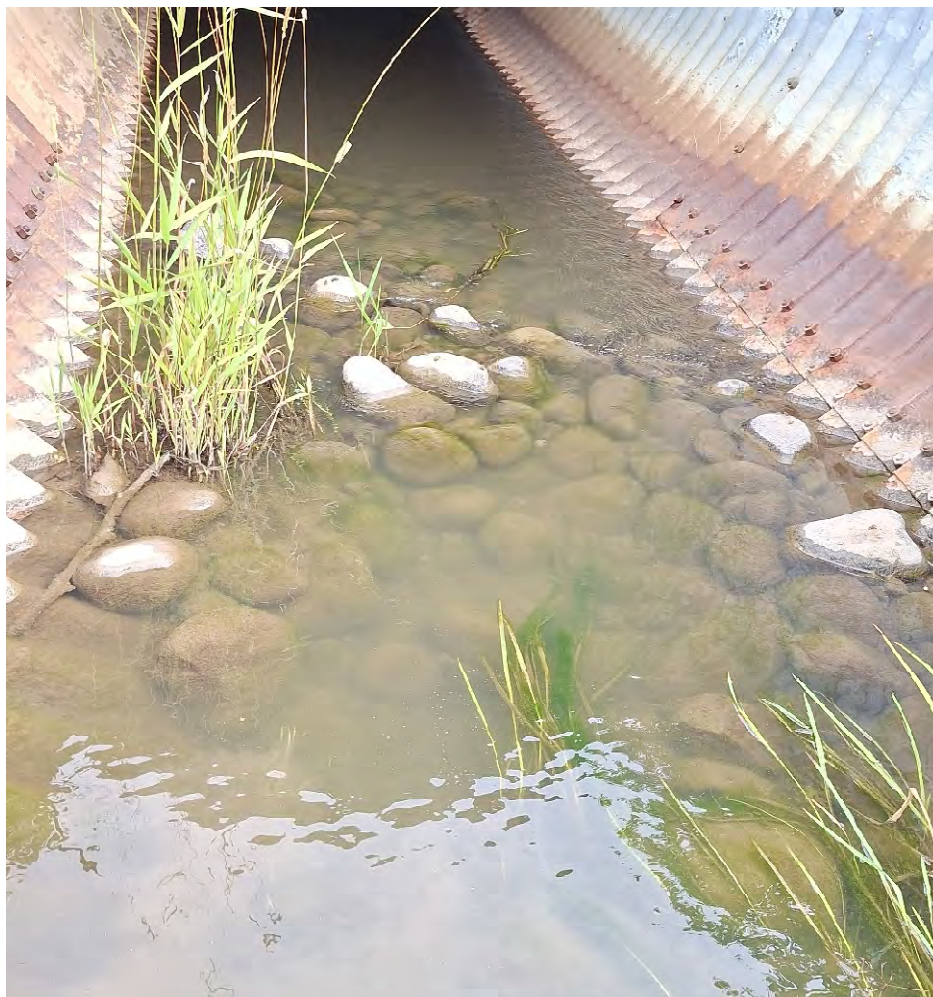
Figure 1 - Debris at Inlet
