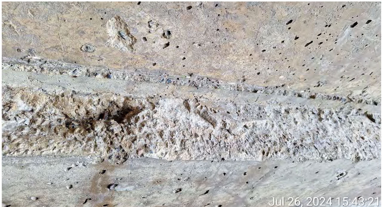
Figure 10 - Disintegration of Top of Footing
