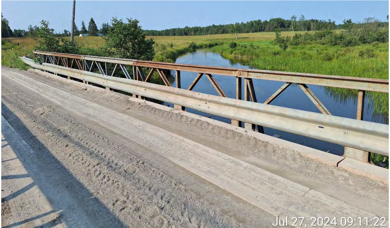
Figure 3: Modular bridge panels (Trusses) and guiderail, West side.
