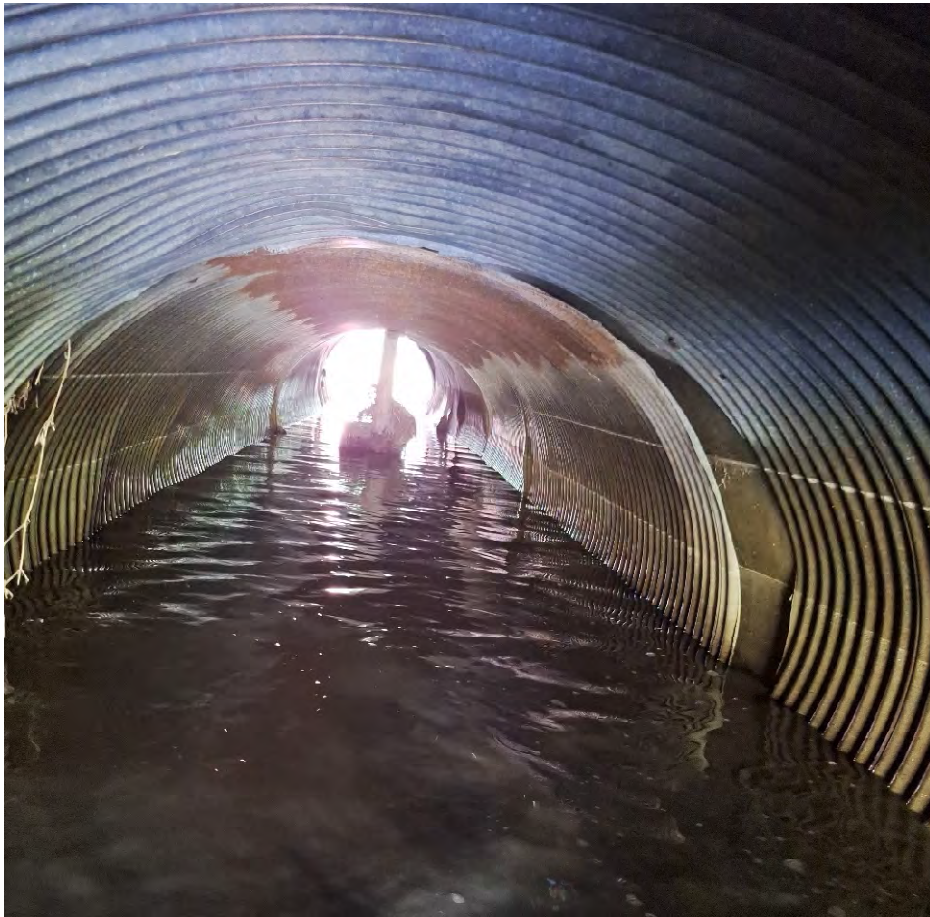
Figure 8: Corrosion overhead
