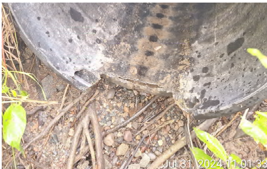
Figure 3 - Damage to invert at the Outlet
