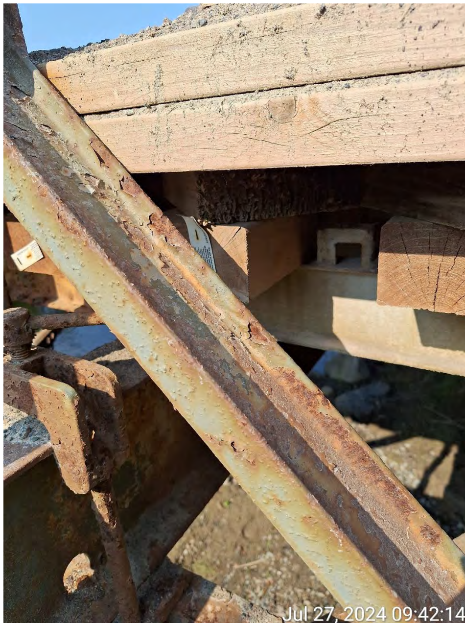
Figure 21: Corrosion and coating failure of raker.
