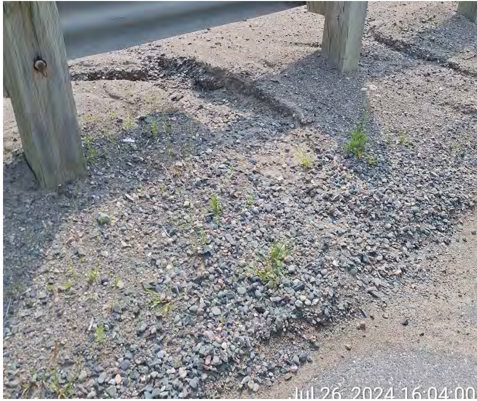
Figure 17 - Erosion Under Guiderail
