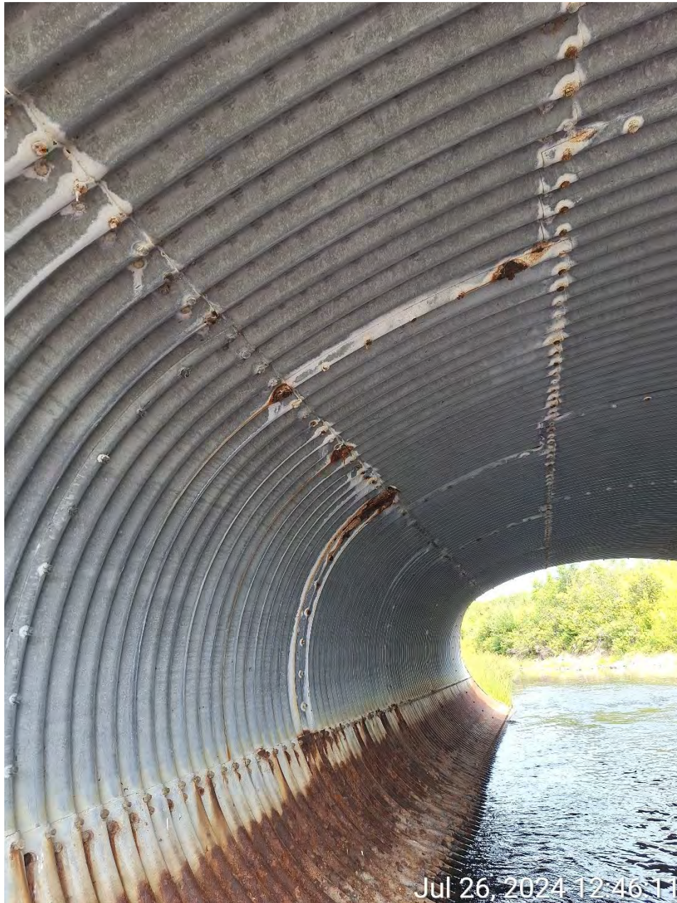
Figure 9: Efflorescence at bolts and culvert joints overhead.
