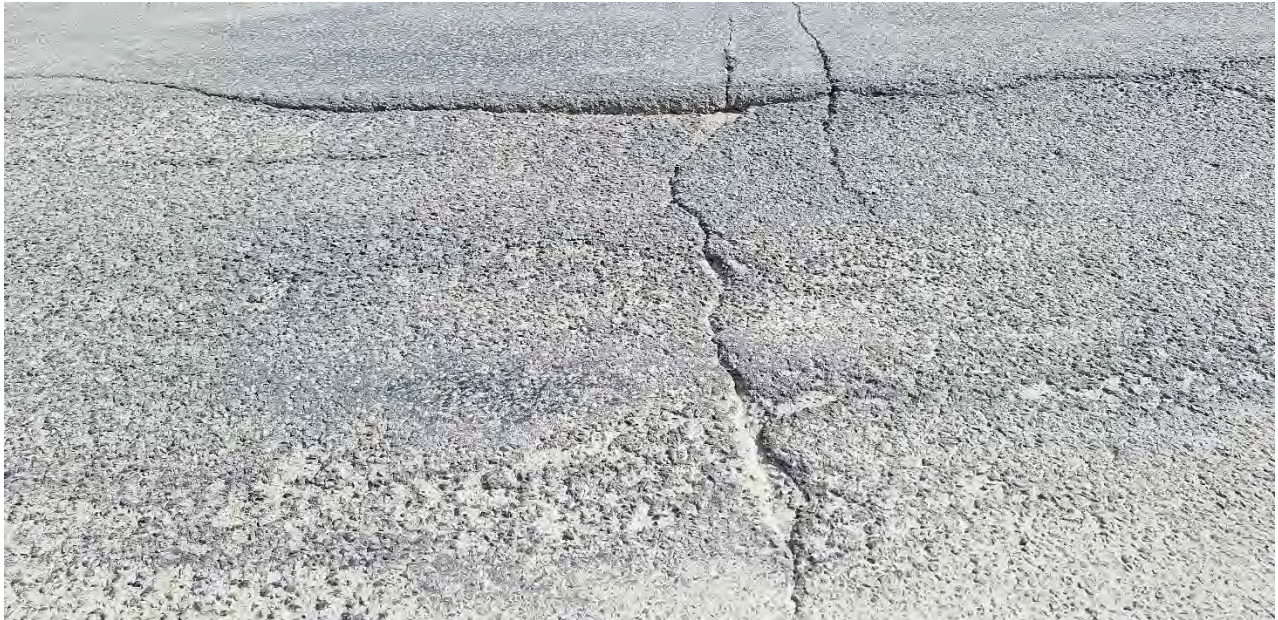
Figure 16 - Cracks in Wearing Surface
