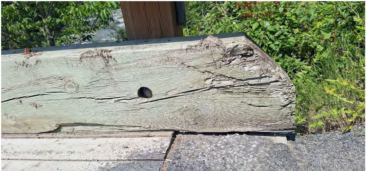
Figure 14 - Damaged Timber Curb
