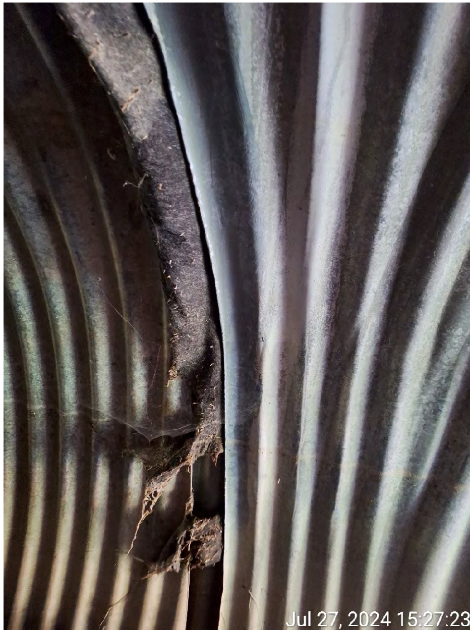
Figure 9: Joint gap with geotextile intruding into the barrel
