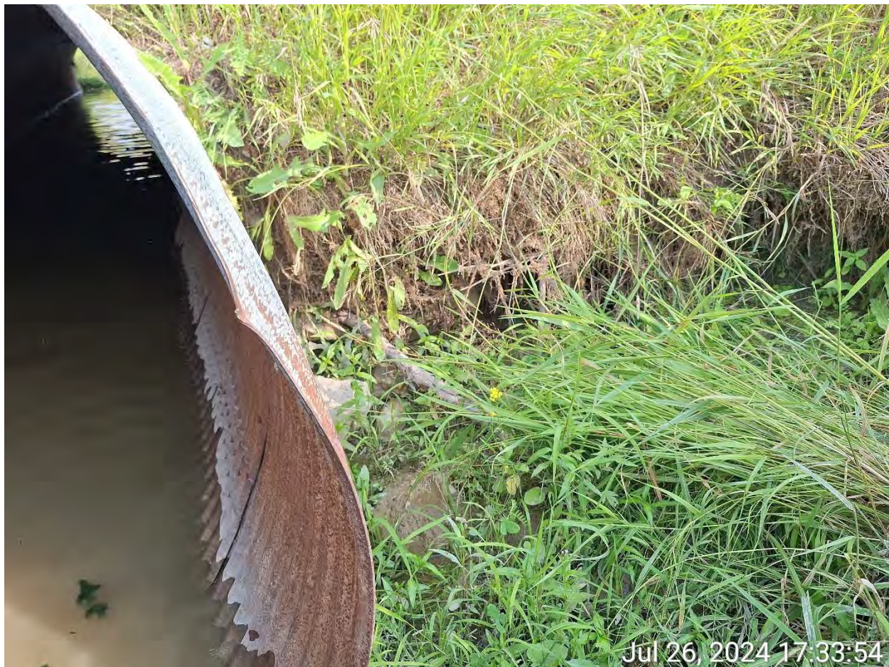
Figure 7: Bank Erosion.
