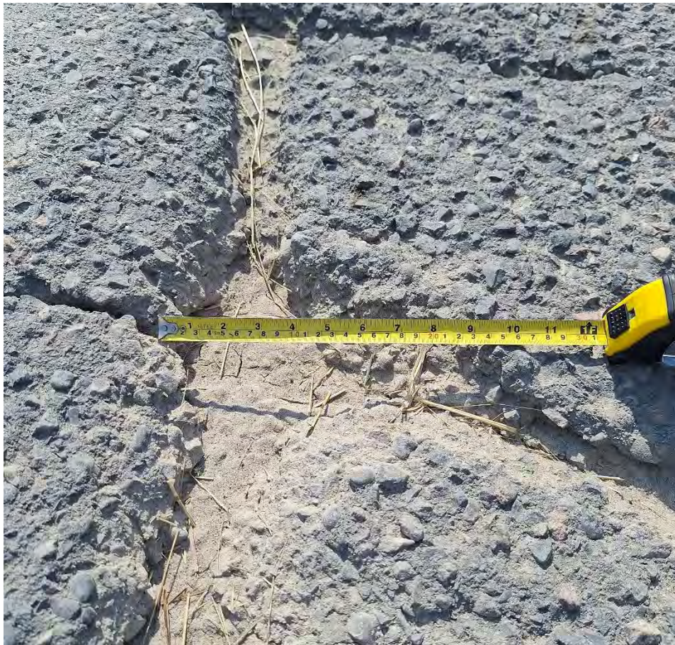
Figure 17 – Very wide Crack on Wearing Surface
