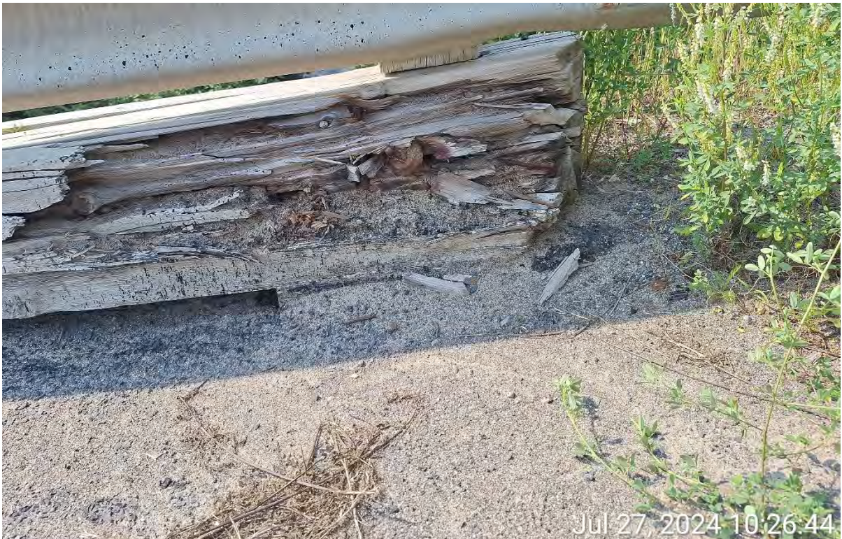
Figure 13 - Damaged Timber Curb
