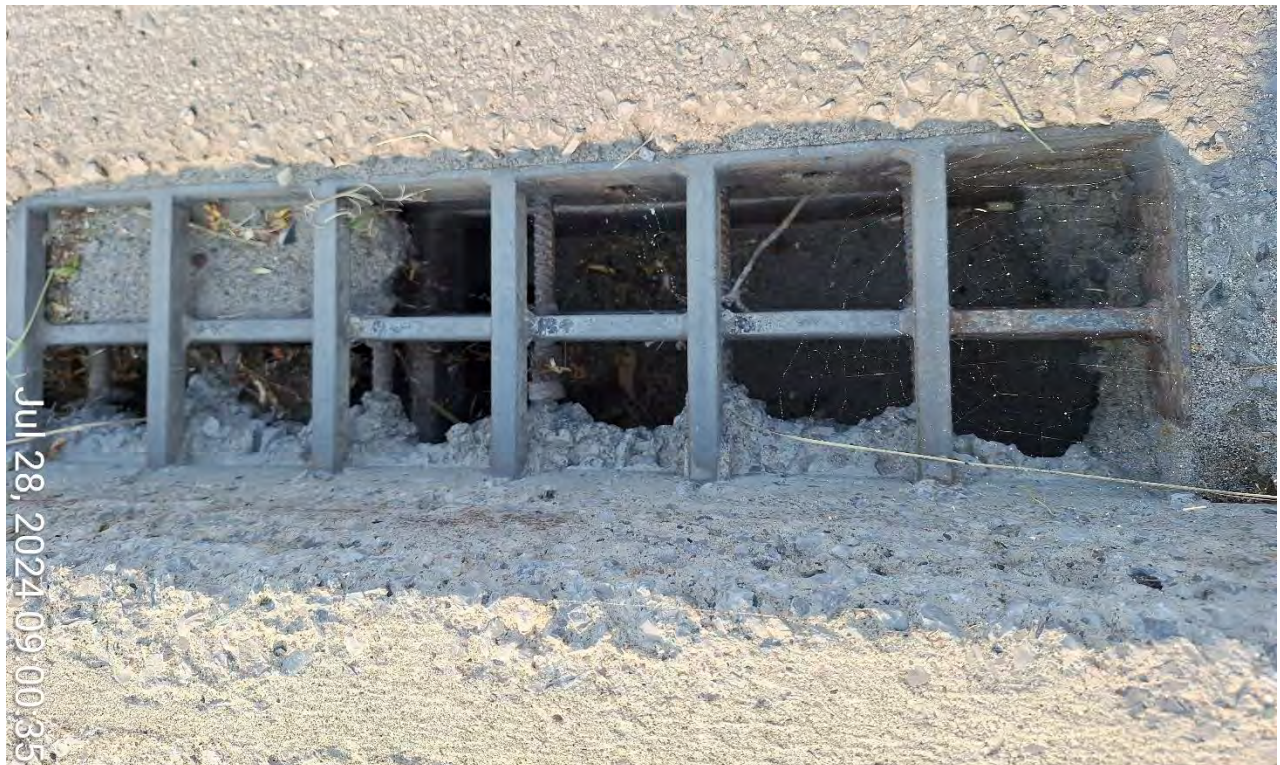
Figure 14 - Slight Debris Build Up in Deck Drain
