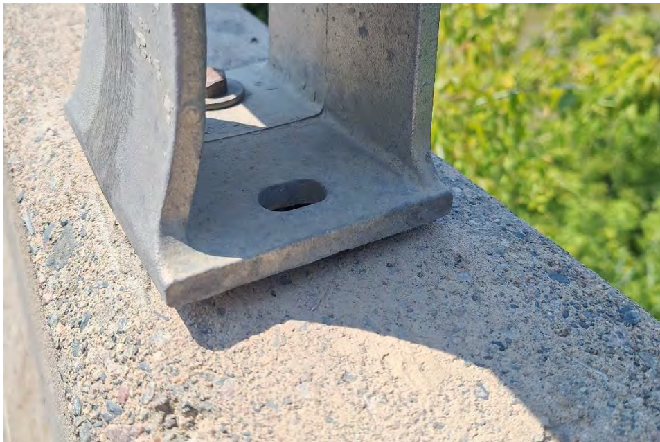
Figure 15 - Missing Bolt on railing mount.
