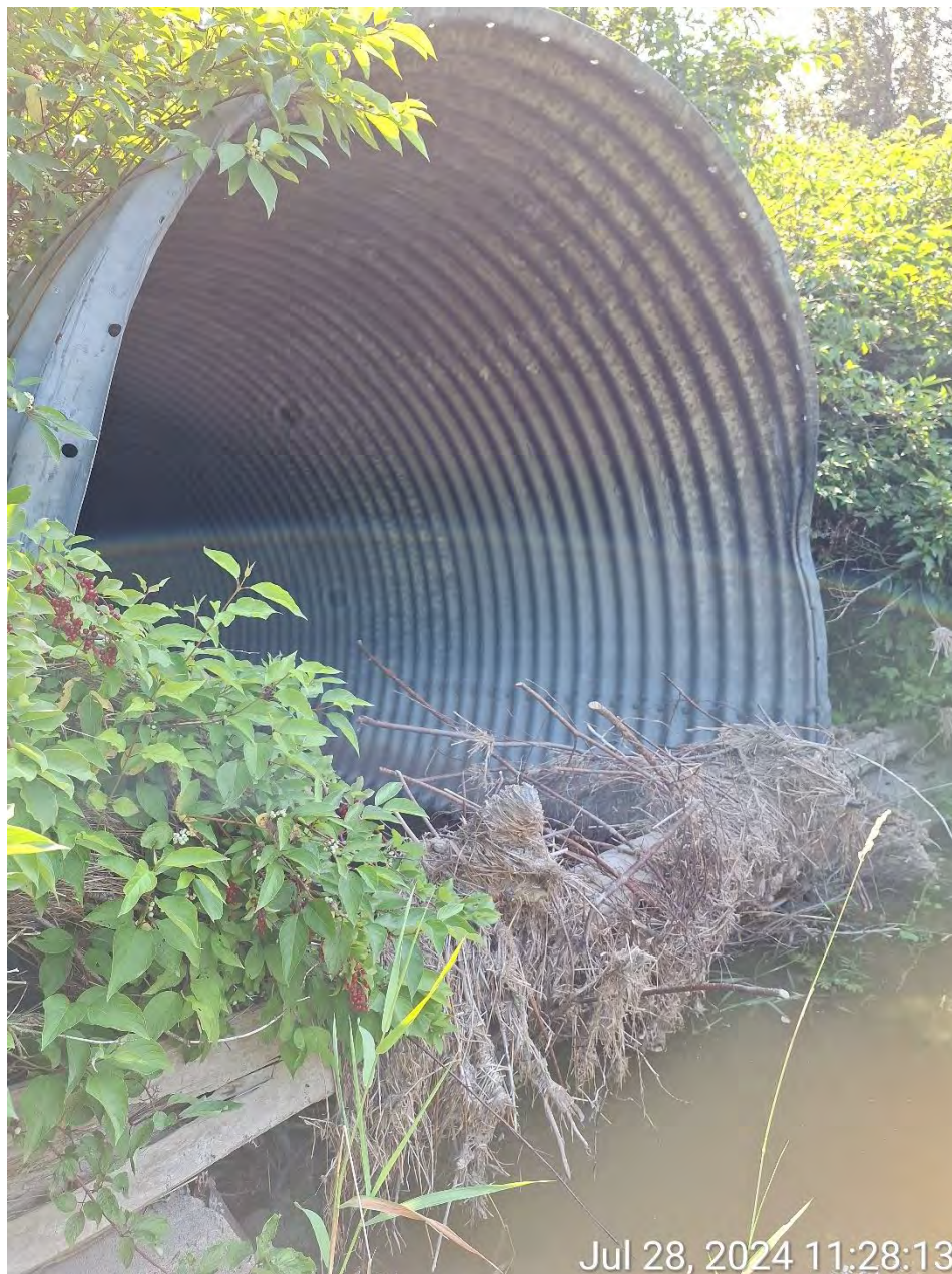
Figure 5: View from upstream of inlet debris
