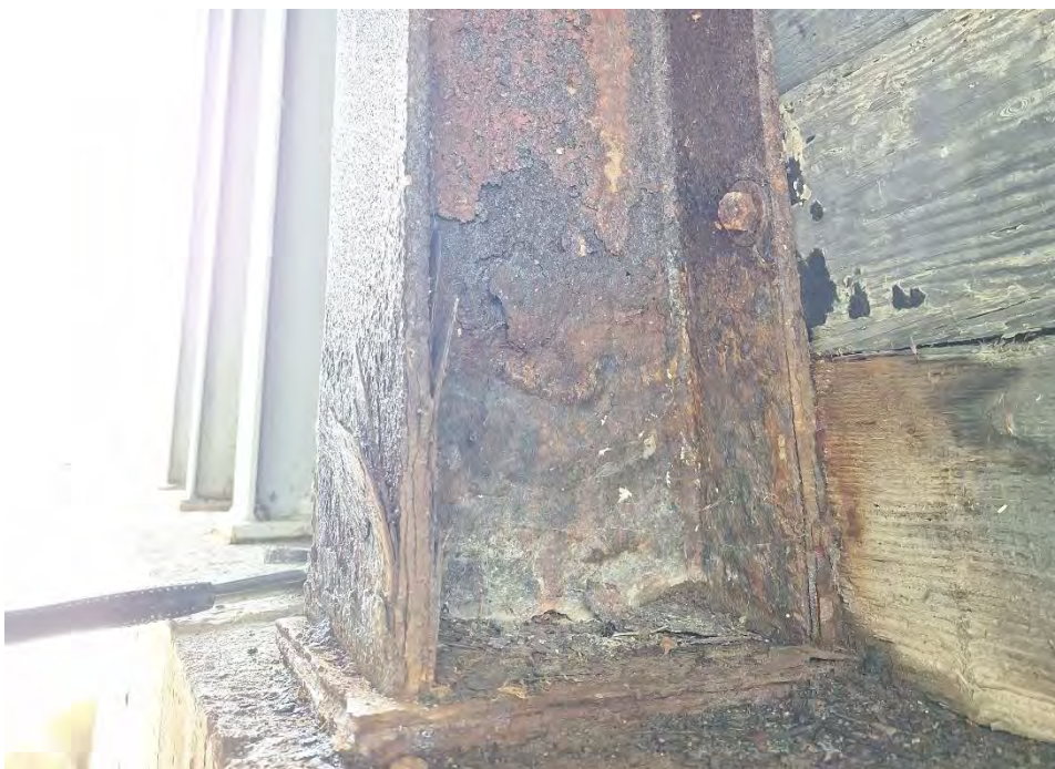
Figure 10 – Severe Corrosion with flakes and section loss at Bottom of 5 th Column from South
