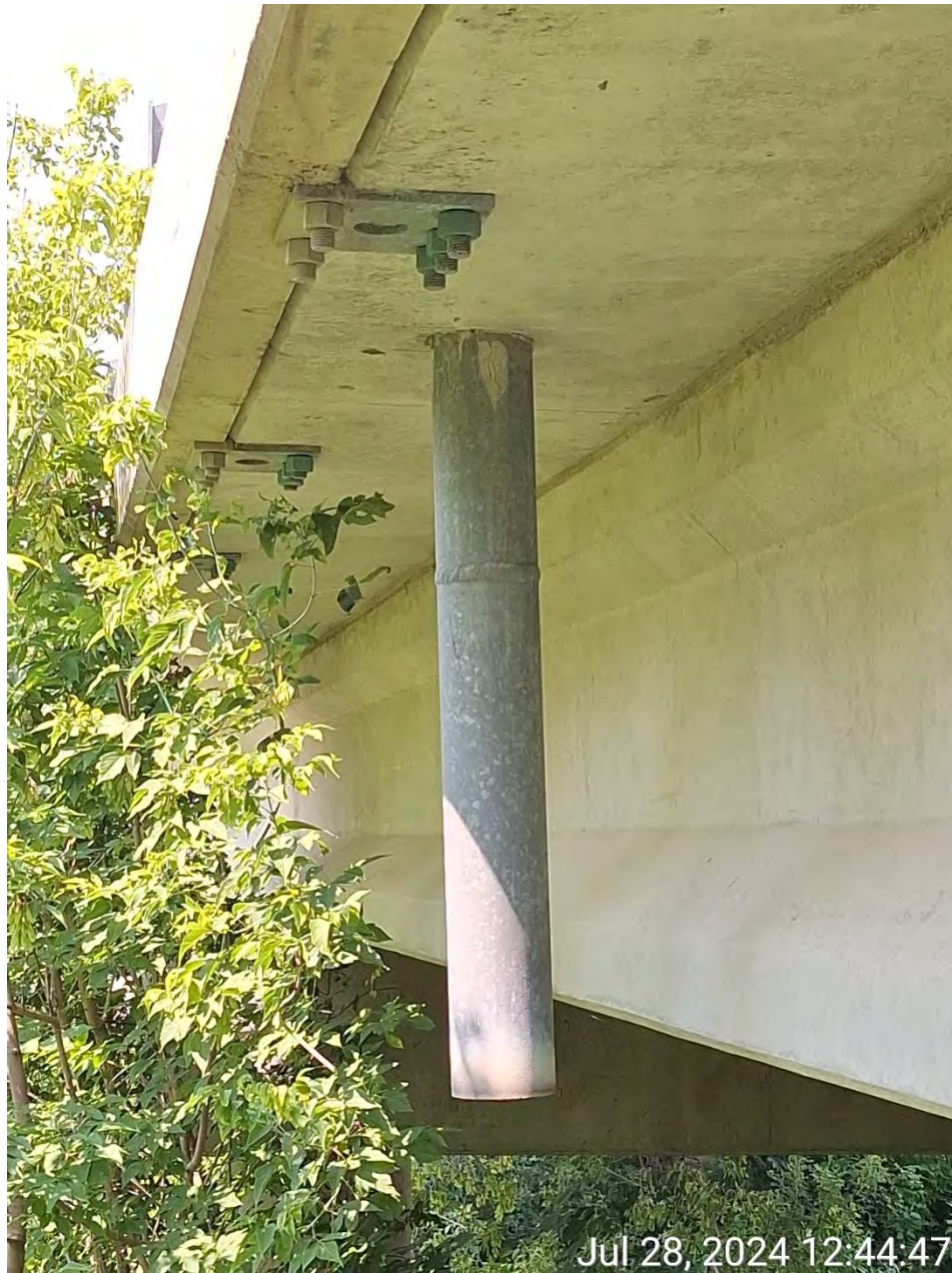
Figure 14: Deck Drain
