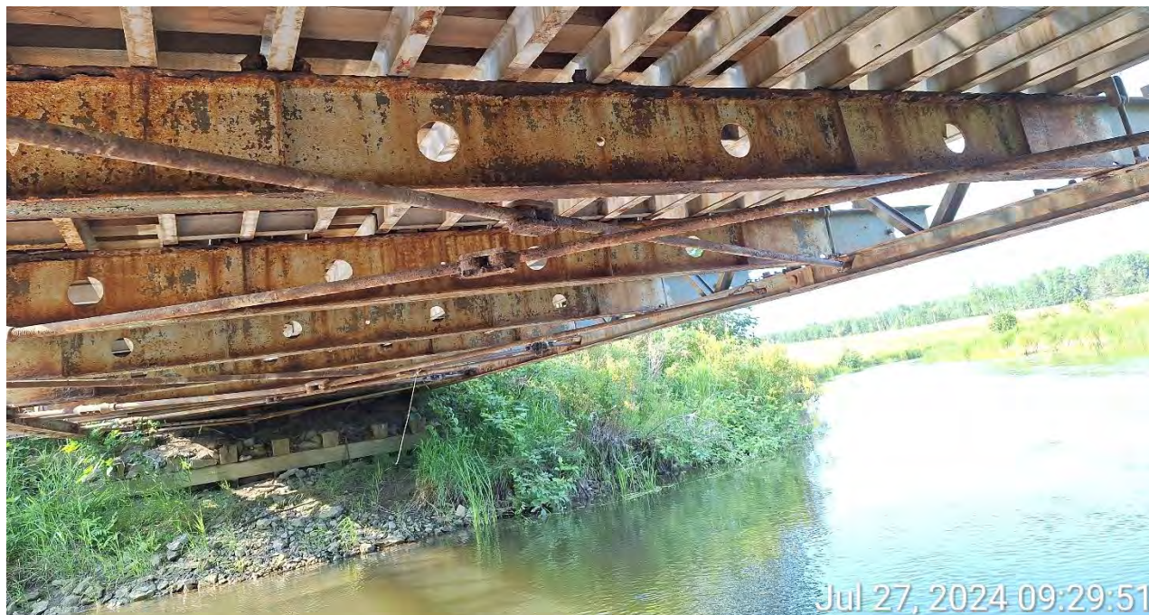
Figure 19 – Bracing with severe corrosion.
