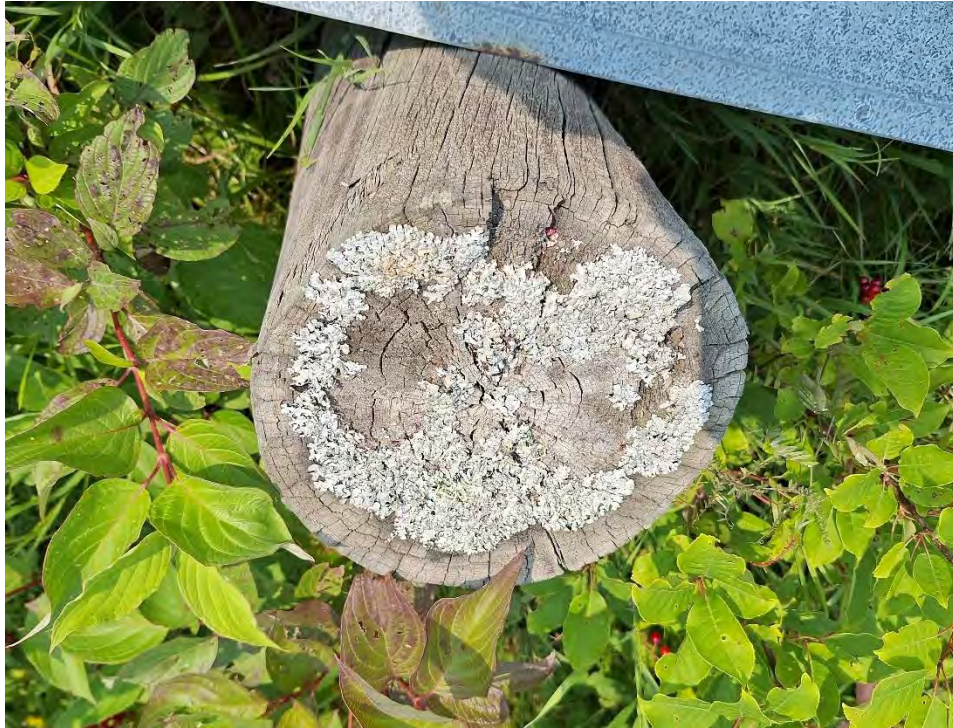
Figure 3 - Weathering and Growth on Post
