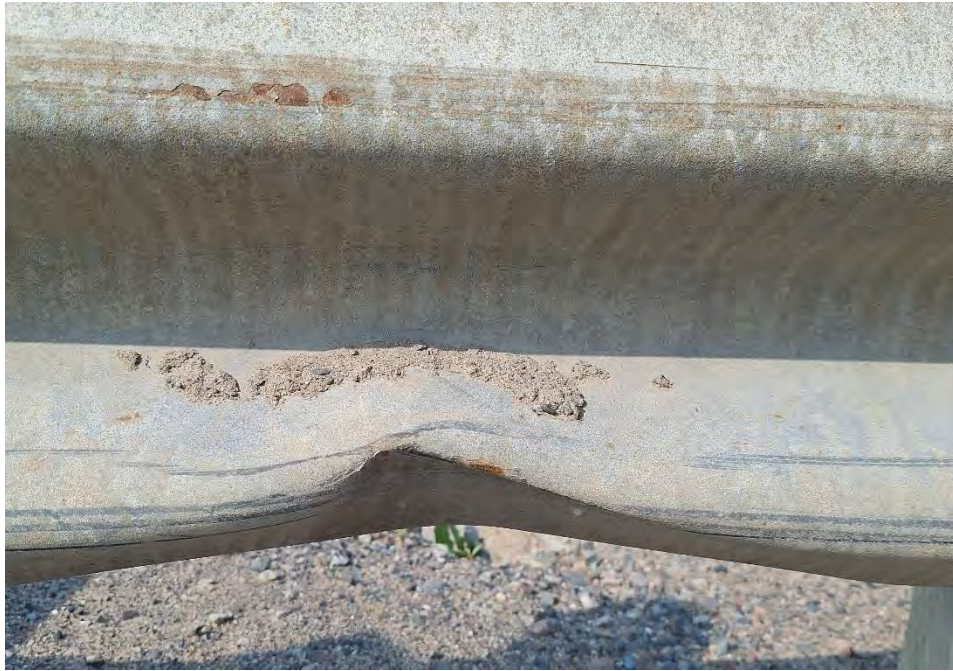
Figure 19 - Damaged Rail, bent with light corrosion.
