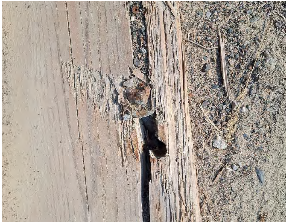
Figure 6 - Split Curb and distorted bolt.
