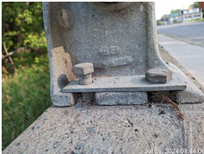
Figure 15: Railing mount with loose bolt.
