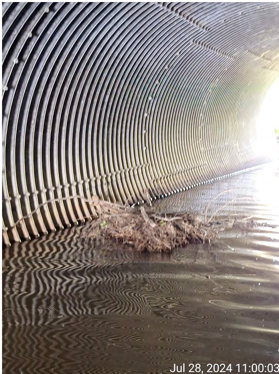
Figure 8: Debris in culvert barrel
