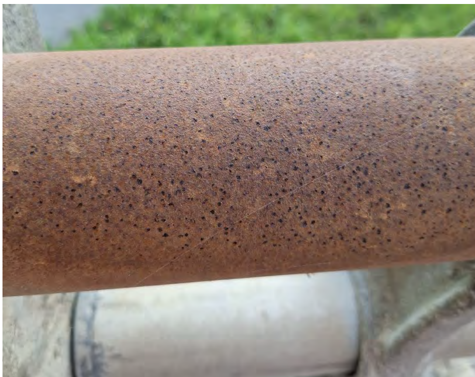
Figure 8 - Corrosion on railing with some pitting.
