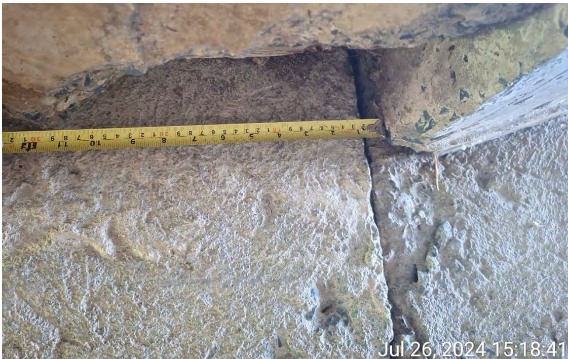
Figure 8 - Severe Spall on Barrel Wall Near Joint
