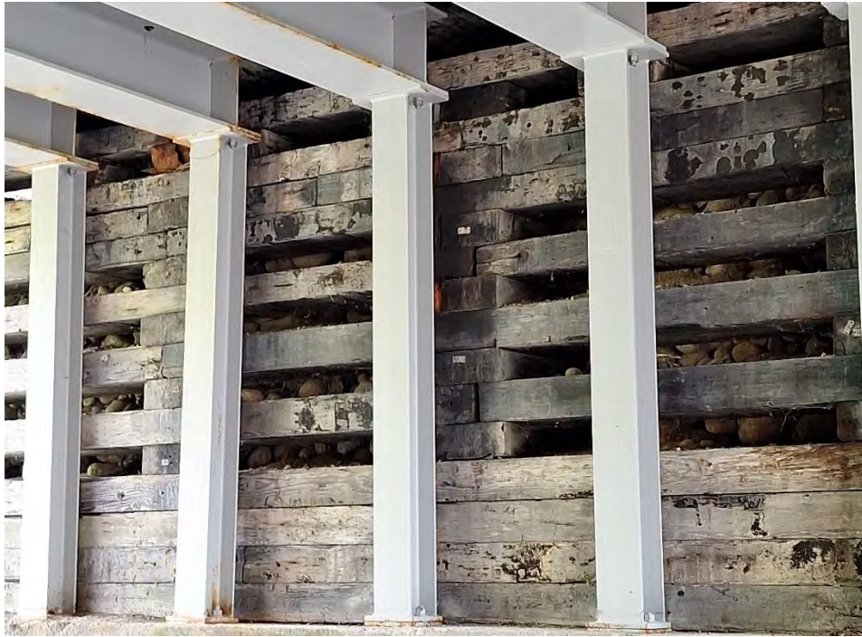
Figure 11 - Coated Steel Columns and Girders
