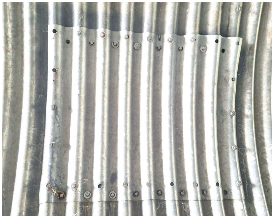
Figure 6 - Repair Patch with Missing Bolts
