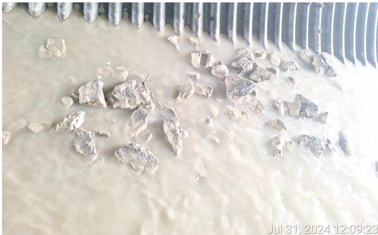
Figure 7 - Debris in Culvert Barrel
