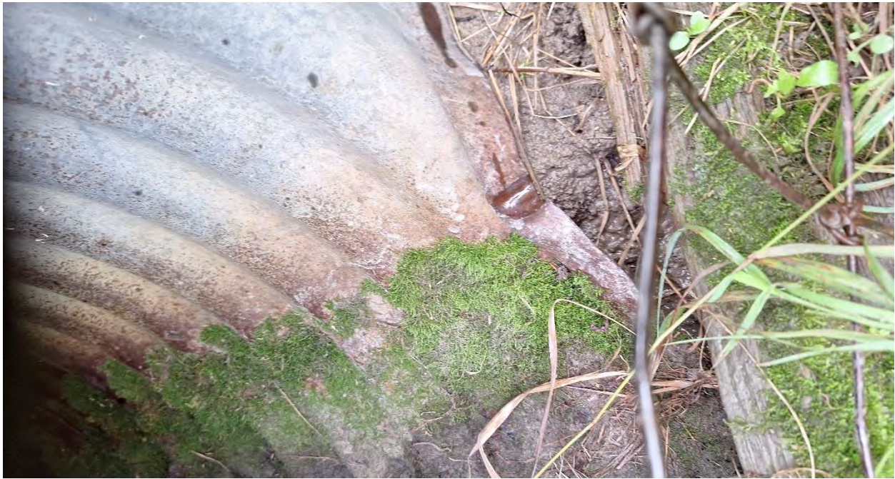
Figure 4 - Damaged West End, growth in barrel
