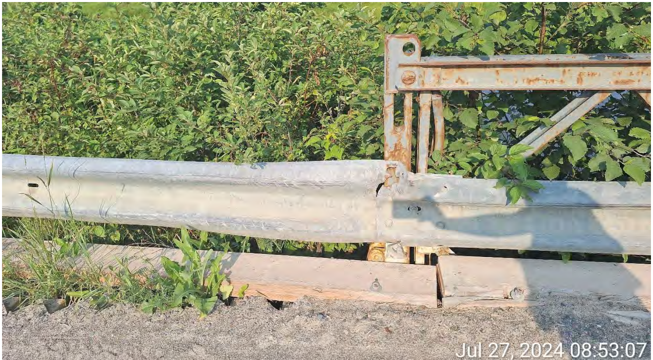
Figure 8 - Damaged Guide Rail
