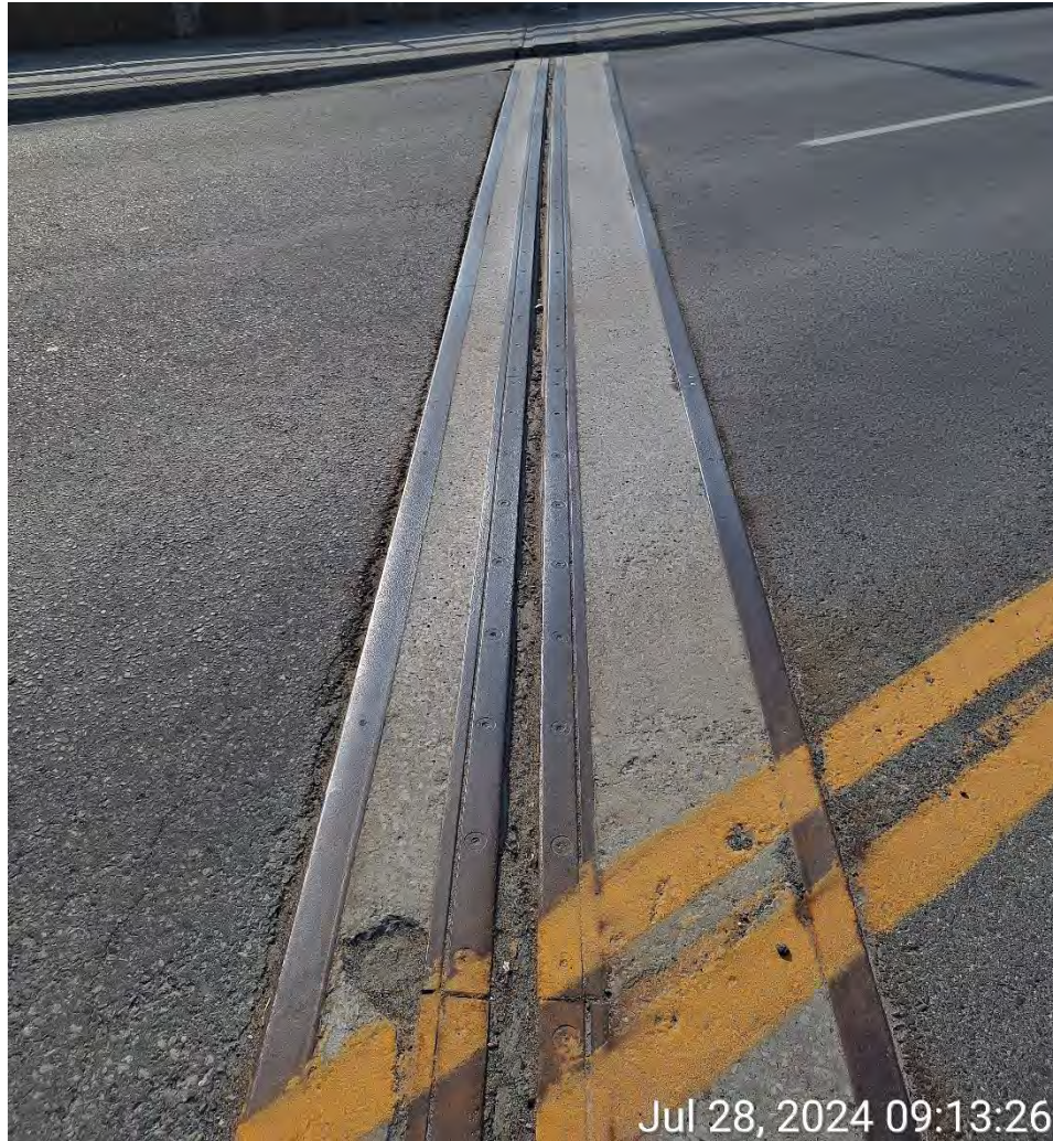
Figure 11 - Expansion Joint
