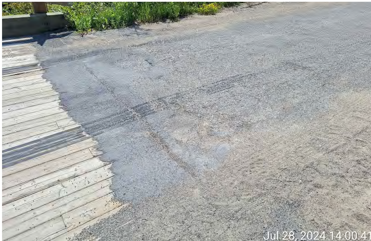
Figure 19 – Depressions in approach Wearing Surface
