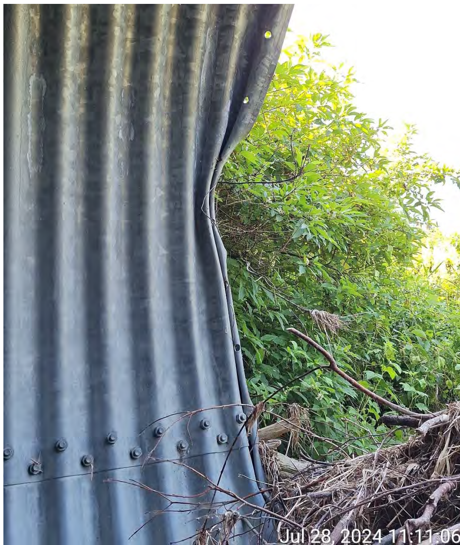
Figure 10 - Damage at Inlet
