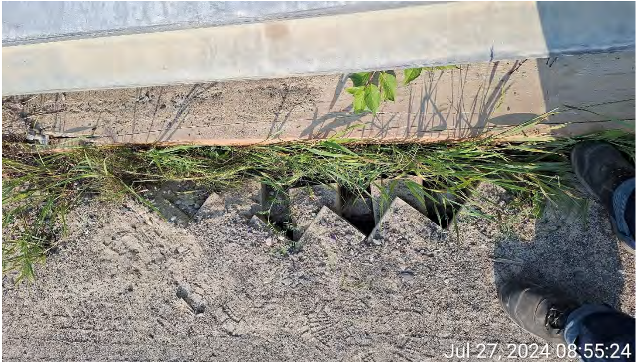
Figure 5 - Loose Curb separated from deck
