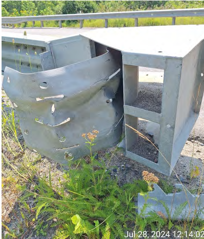
Figure 4: Damaged SBEAT at NW quadrant.
