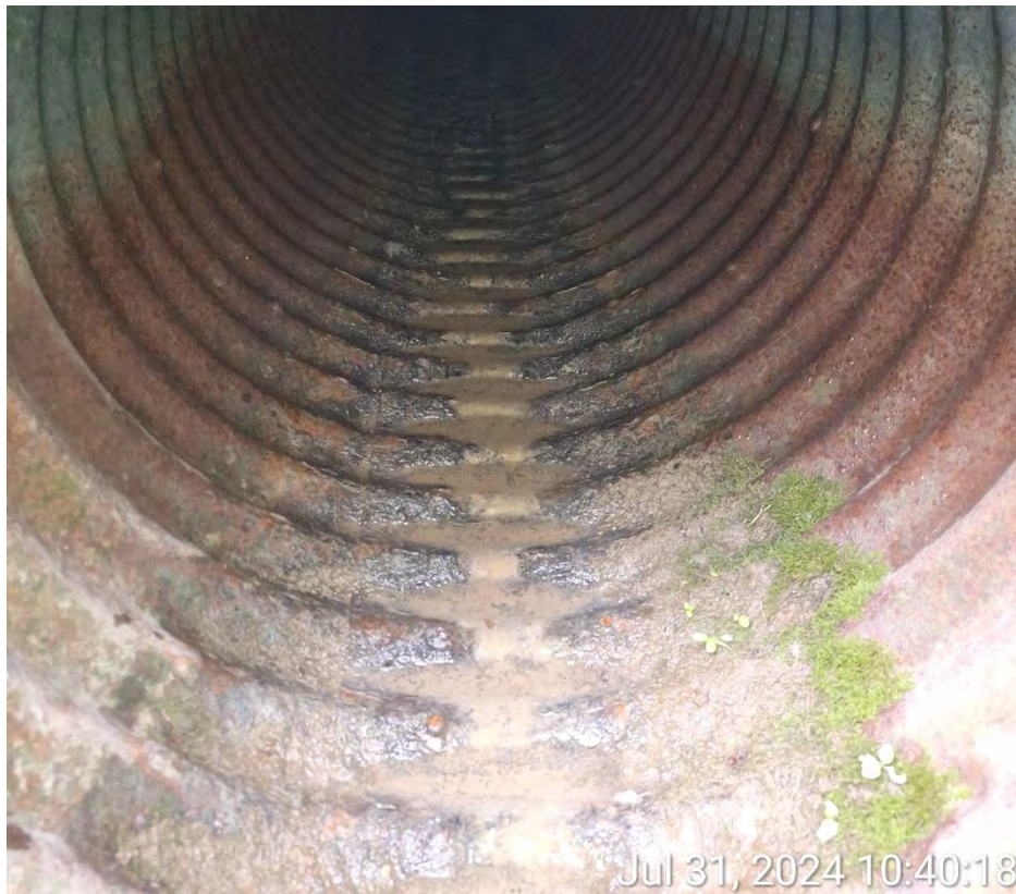
Figure 5 - Corrosion of varying severity throughout Barrel
