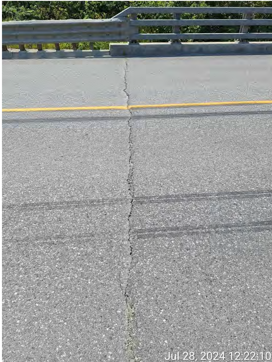
Figure 7: Severe Crack in Wearing Surface
