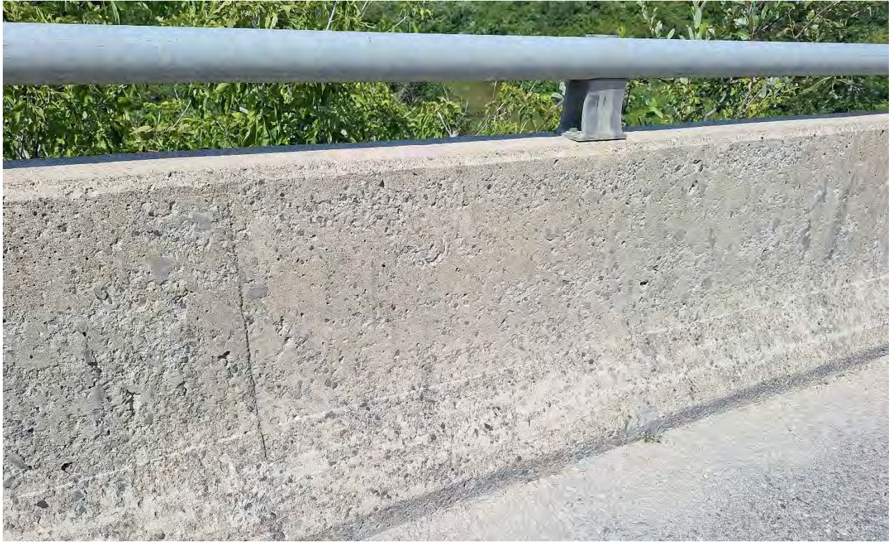
Figure 12 - Scaling on Barrier Wall
