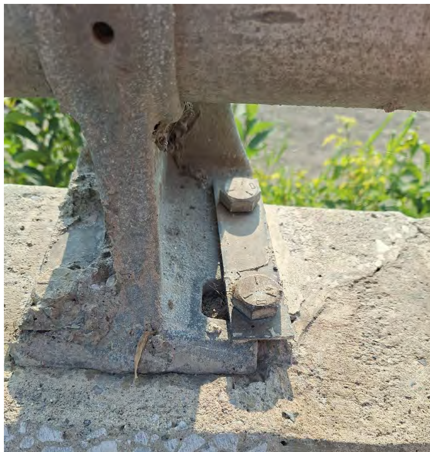
Figure 16: Loose railing mount.
