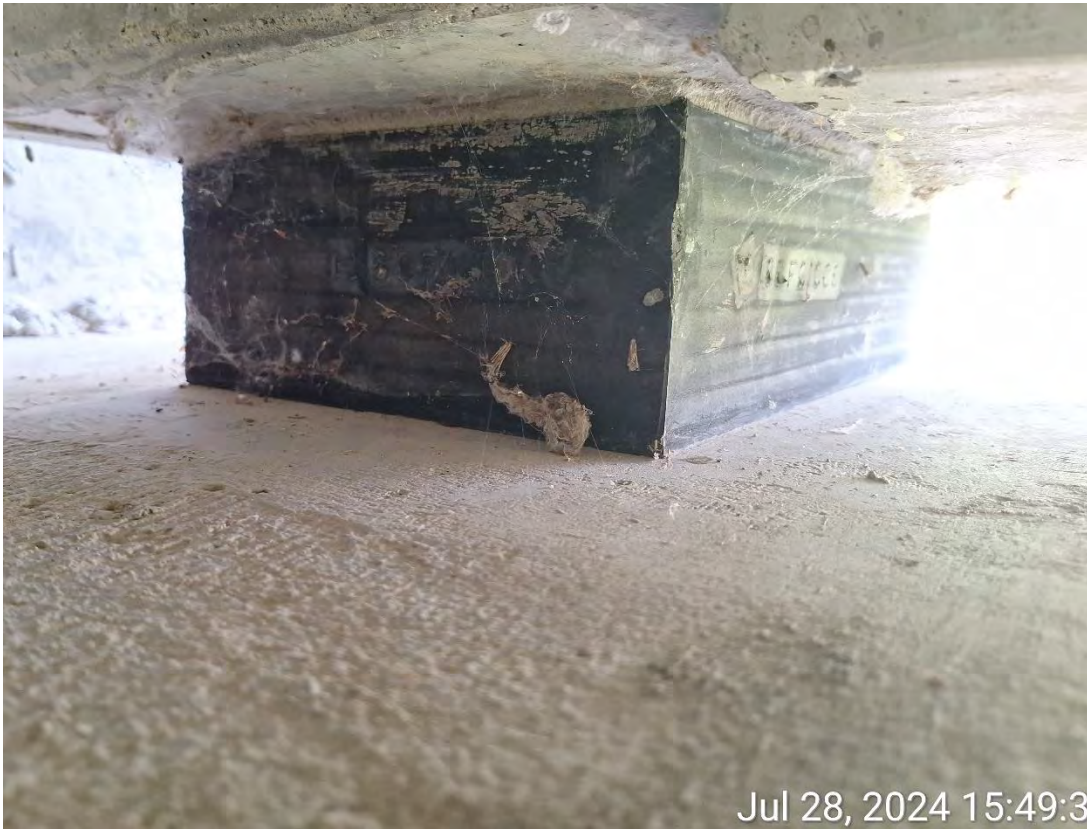
Figure 9 - Abutment Bearings
