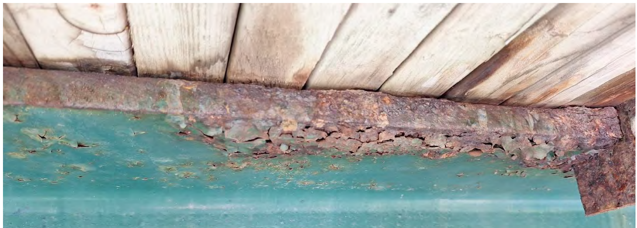
Figure 8 - Corrosion at Top Flange of Girder
