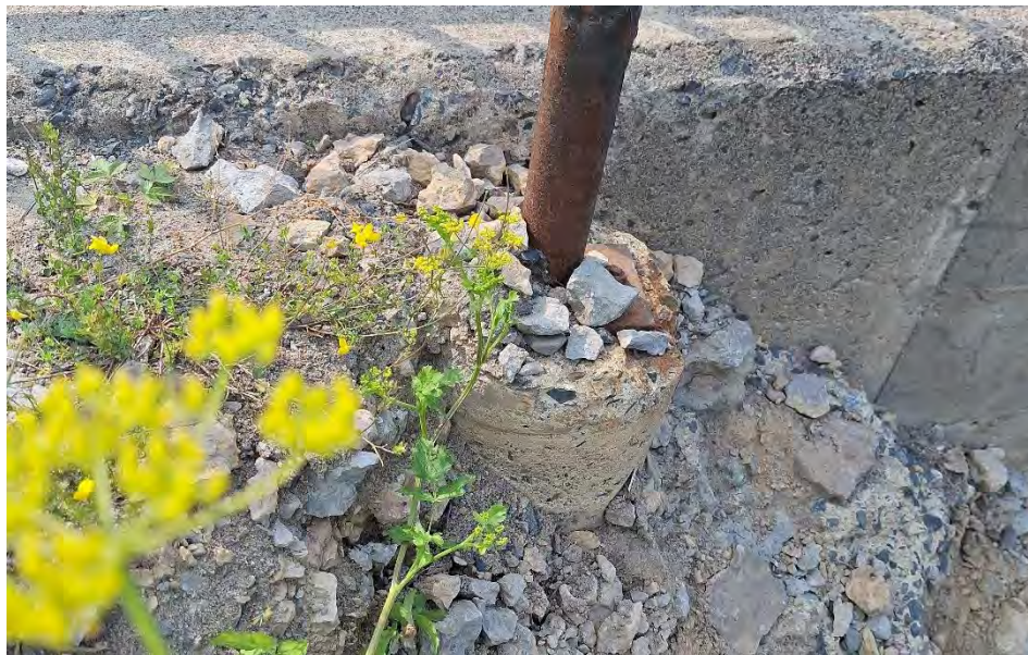
Figure 16 - Exposed Footing of pedestrian railing adjacent to erosion.
