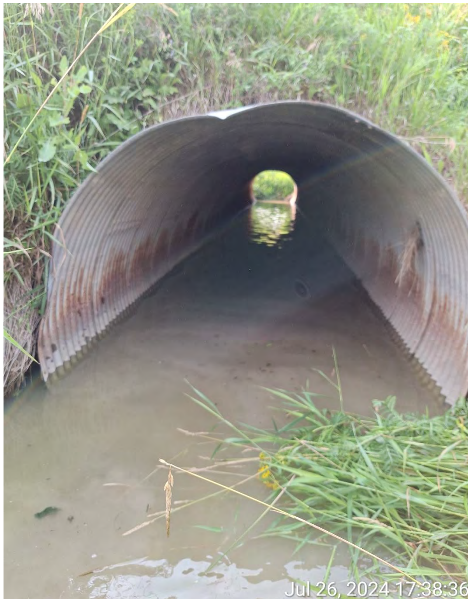
Figure 4: View along barrel, corrosion on both sides near spring line is present
