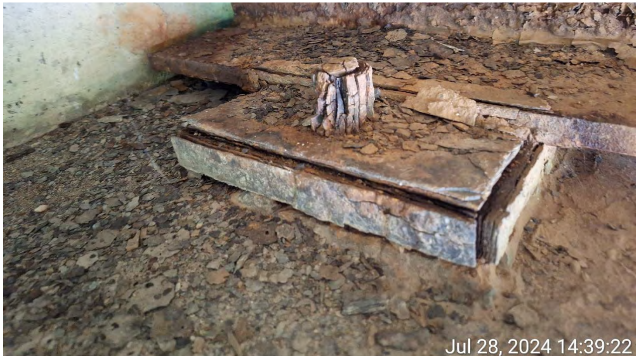
Figure 4 - Severely Corroded Abutment Bearing plate and pin. Large flakes evident.
