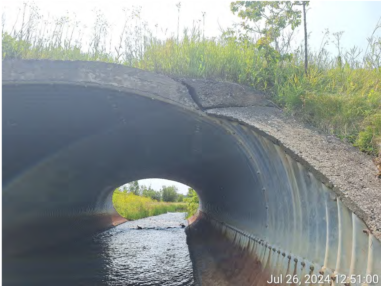
Figure 7: Previous Suspect Concrete repair with a gap between other concrete parts
