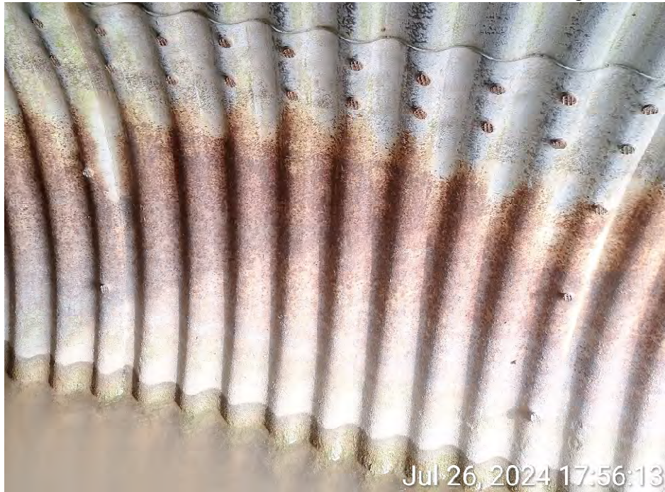
Figure 4 - Corrosion on lower Half of Barrel
