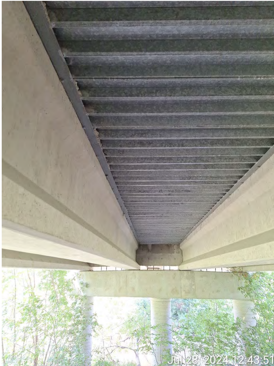
Figure 10: Corrugated Steel decking, rebar extending from pier cap upwards. .
