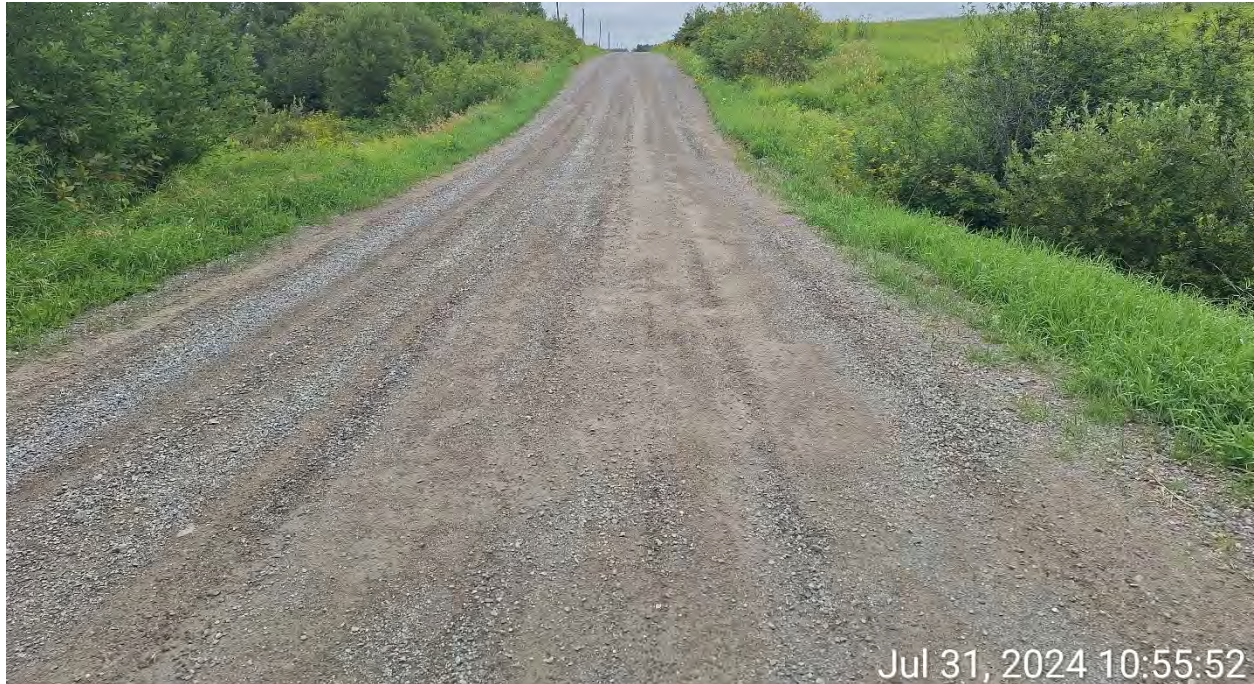
Figure 1 – Gravel Wearing Surface
