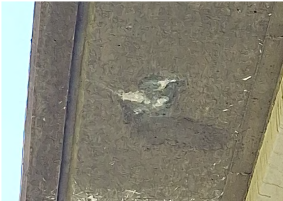
Figure 10 - Efflorescence on Exterior Soffit
