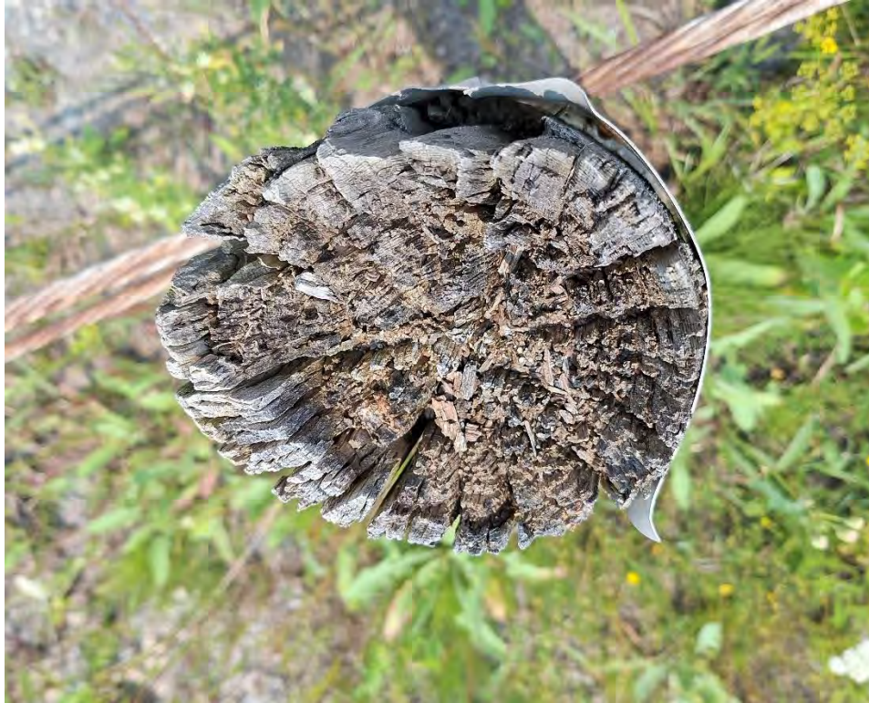
Figure 3 - Deteriorating Wooden Post
