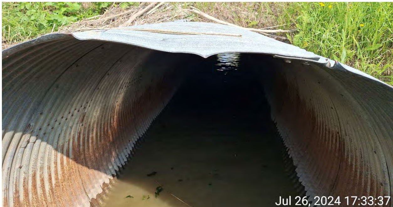
Figure 1 - Damaged Barrel
