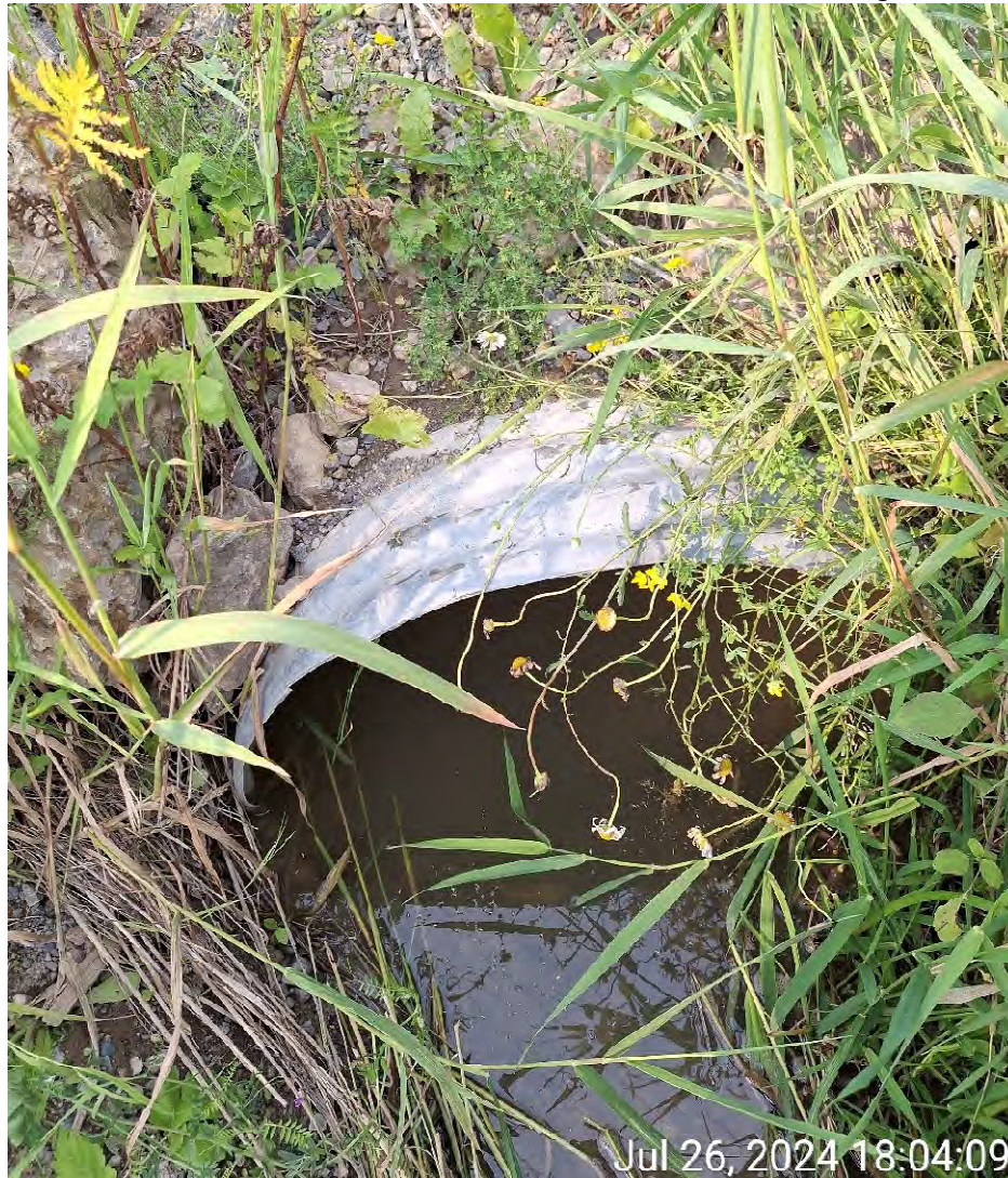
Figure 7: 900mm culvert adjacent to inspected culvert. East end not found.
