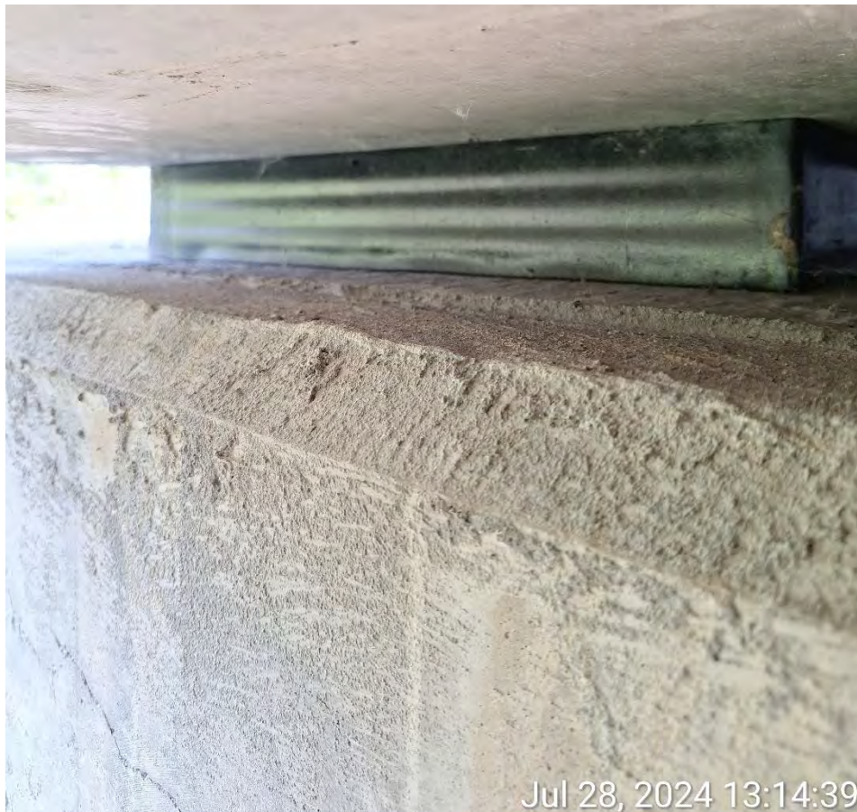
Figure 13: Bearing pad with some bulging.
