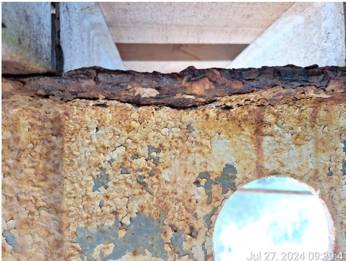
Figure 16: Transom top flange showing corrosion.
