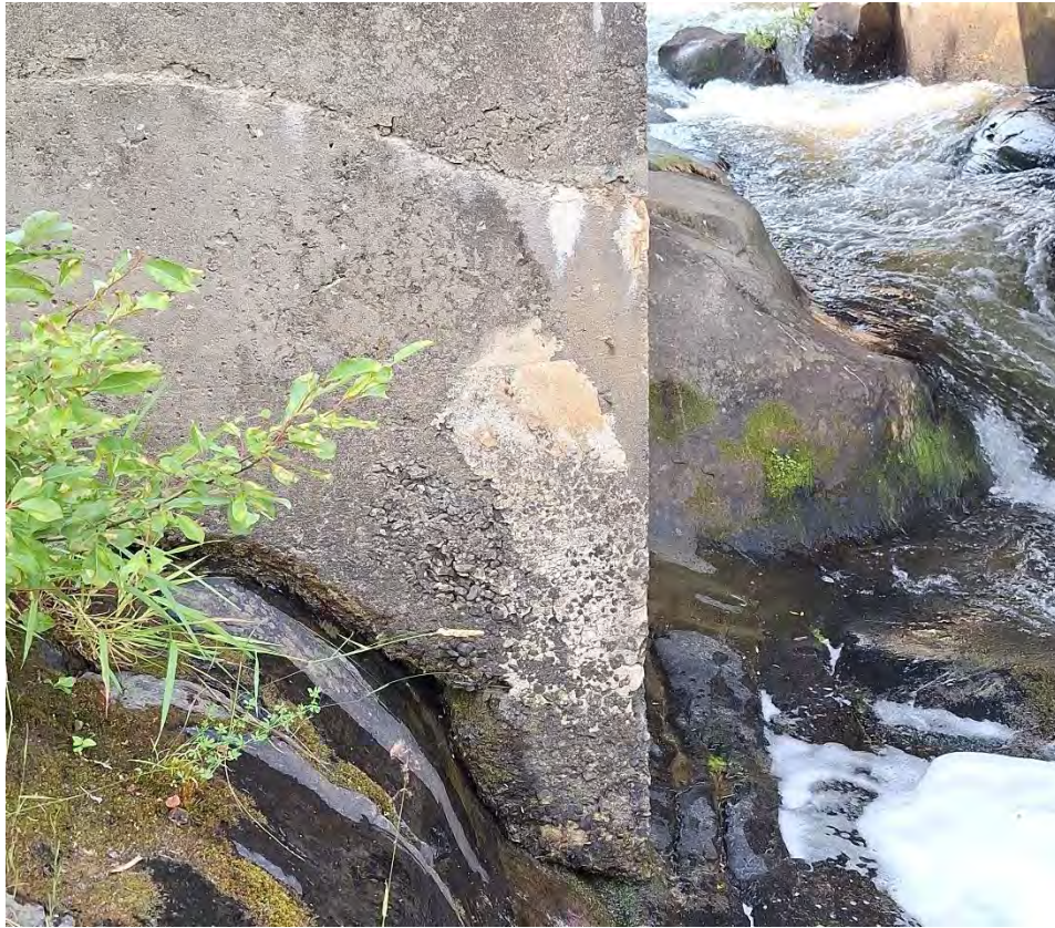
Figure 5 - East Abutment Wall Undercutting
