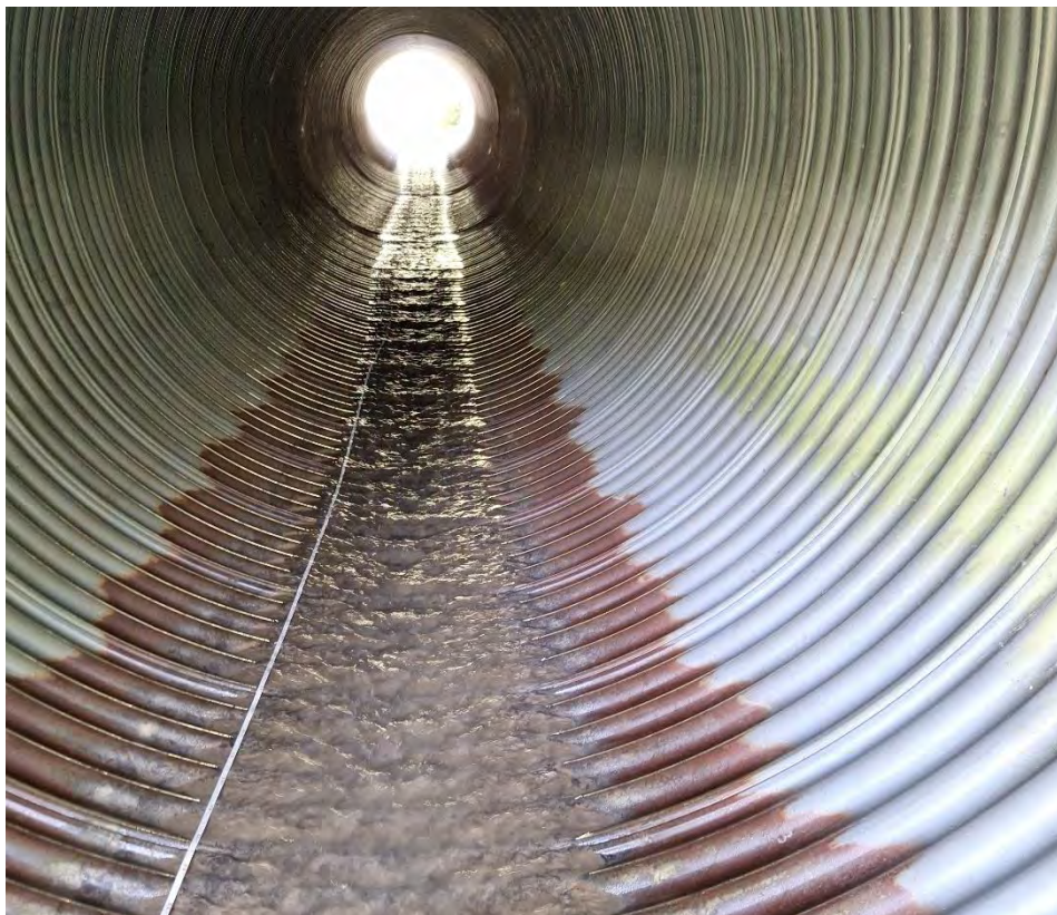
Figure 6 - Corrosion at Bottom of Barrel
