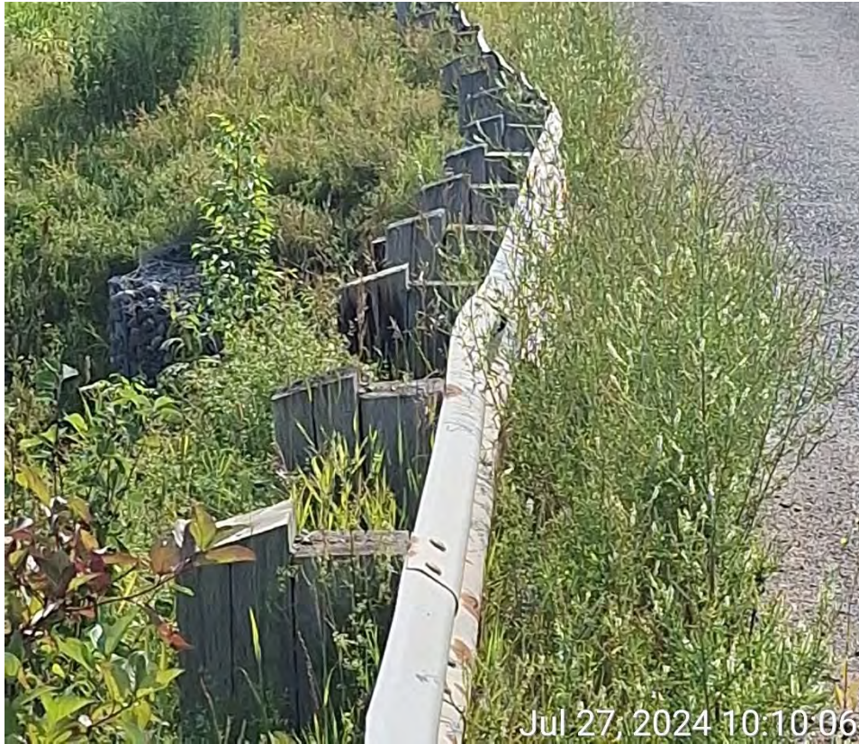
Figure 16 - Guide Rail showing impact damage
