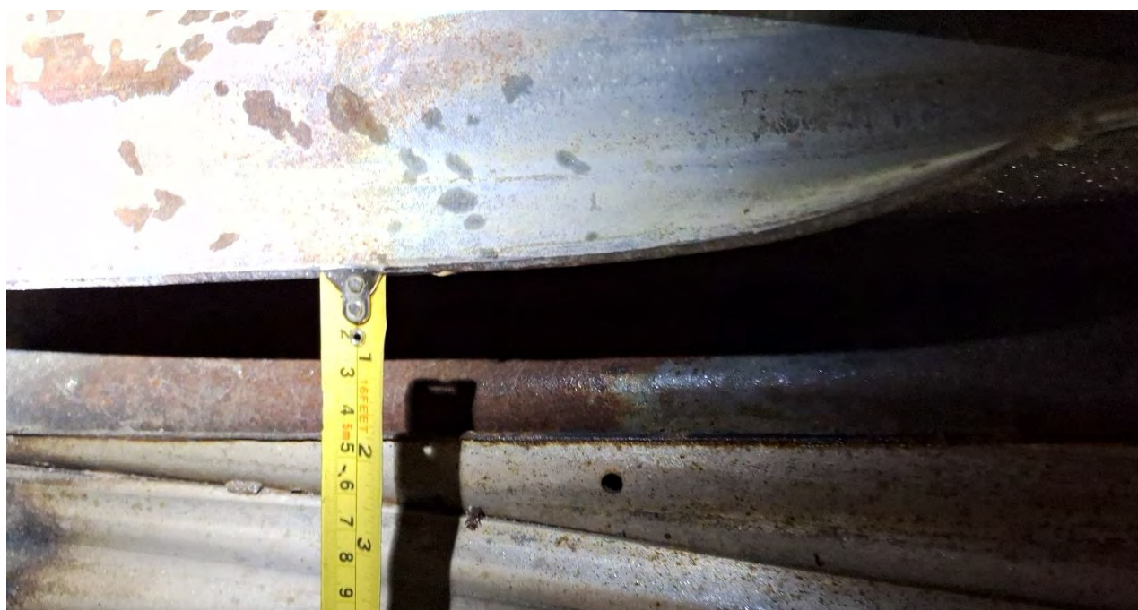
Figure 7 – Gap between culvert barrel pieces at Bottom of Barrel
