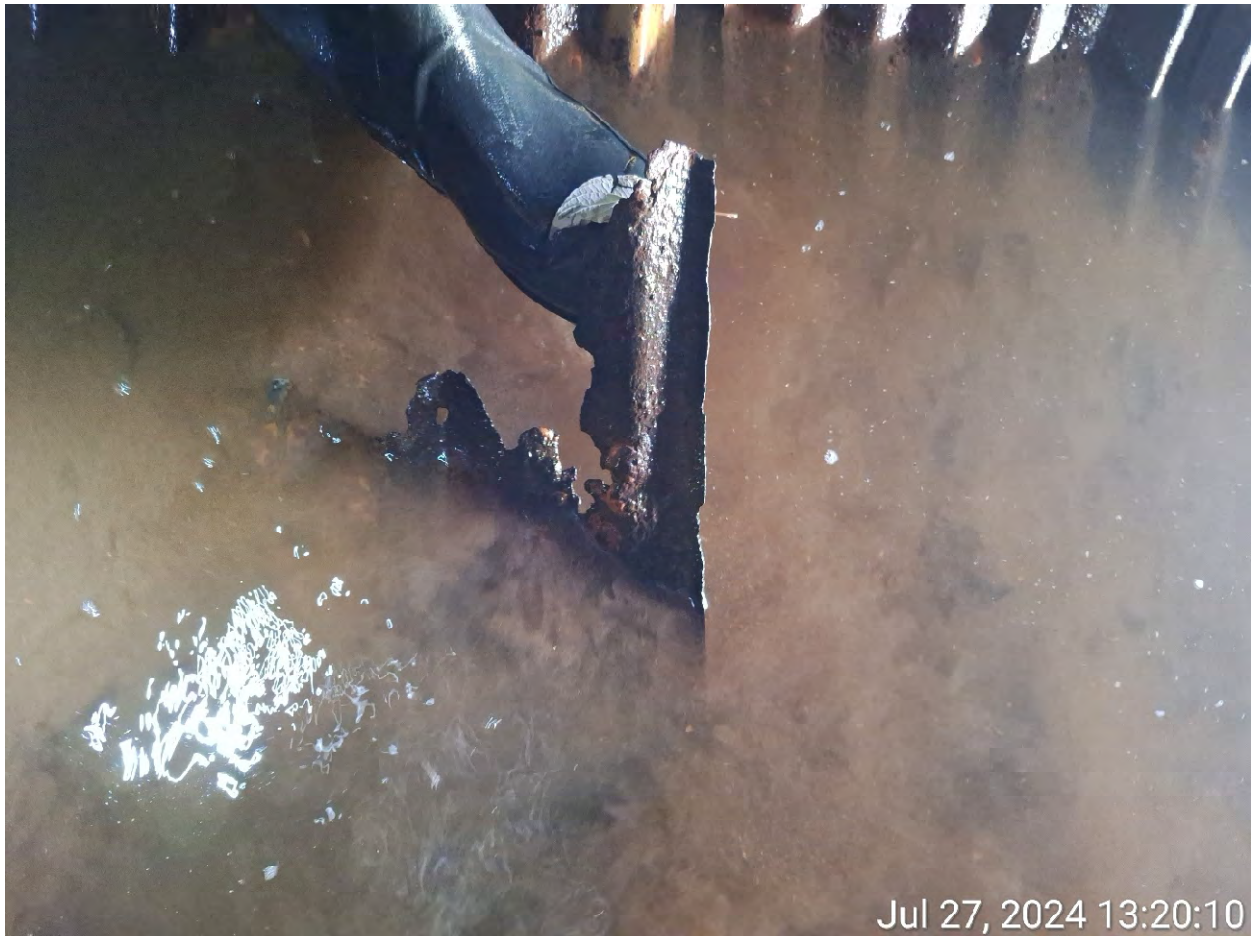
Figure 7: Torn piece of culvert barrel extending beyond water surface
