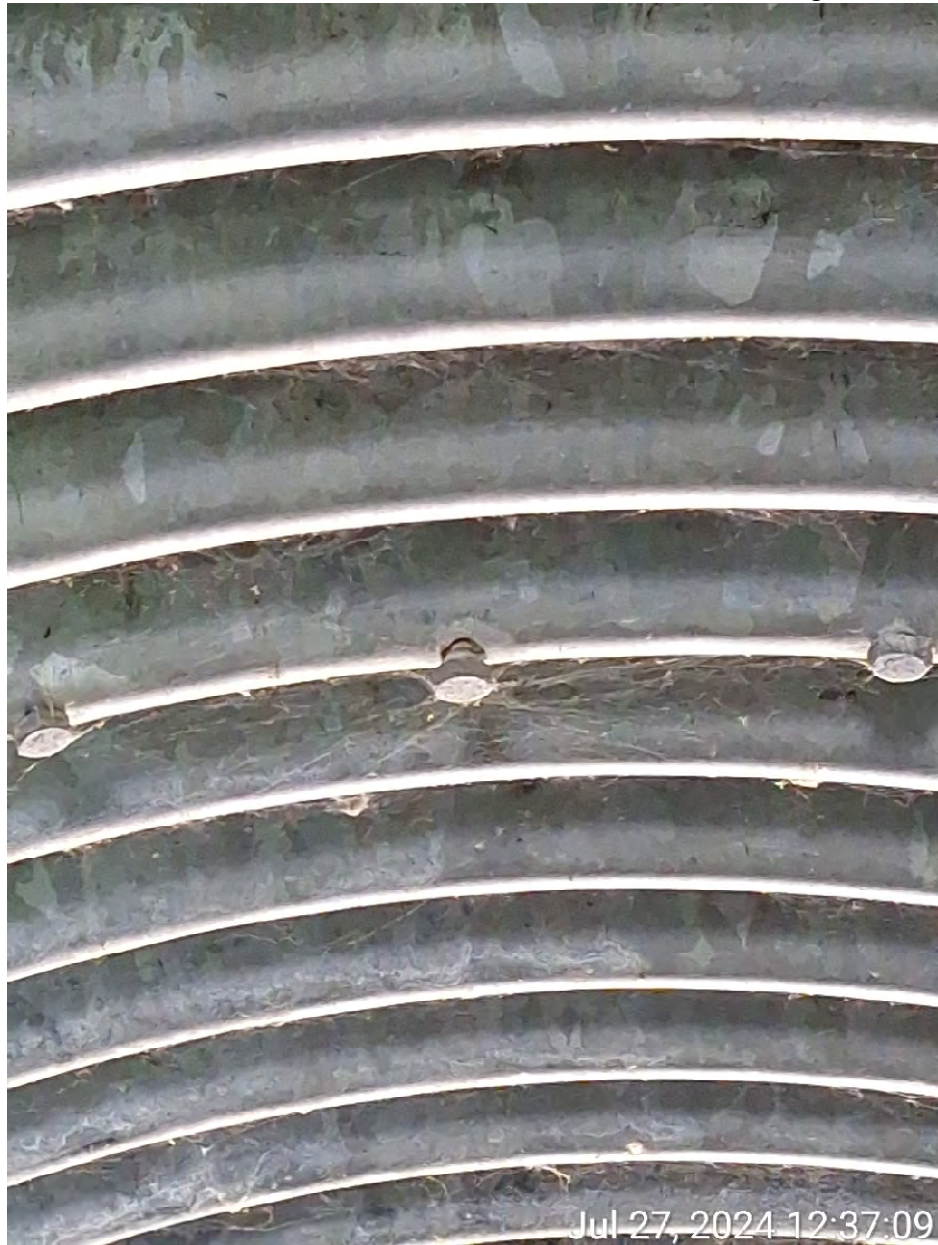
Figure 5: Possible loose bolt connection - could not be reached to be checked.
