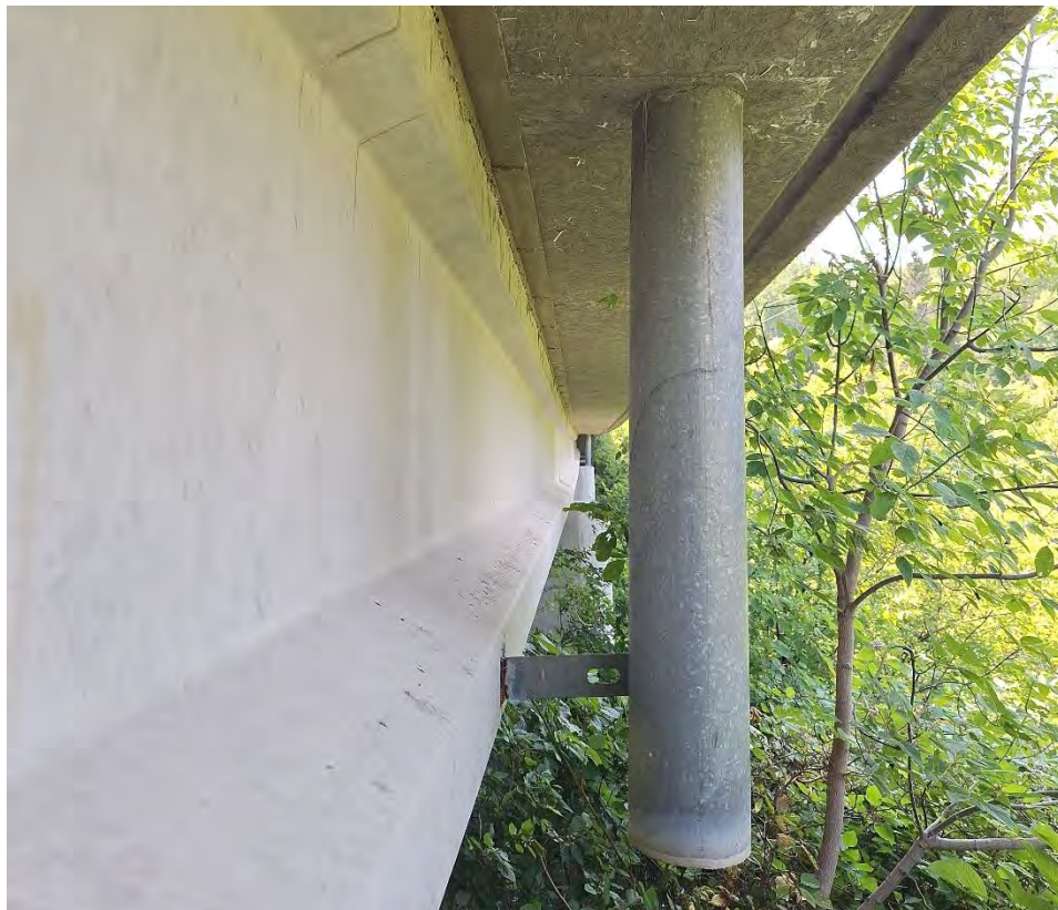
Figure 6 - Drain Pipe
