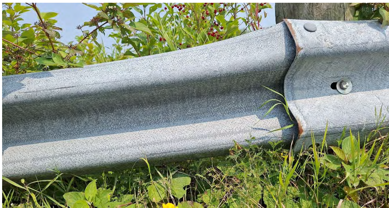
Figure 2 - Barrier Missing Bolts, Poor Connection
