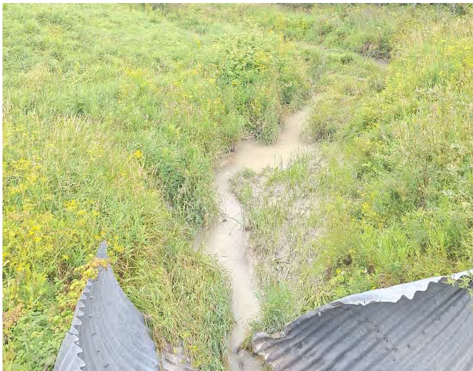
Figure 3 - Inlet Stream, bent culvert barrel.
