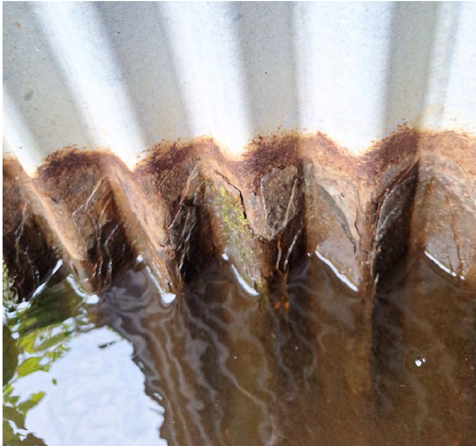
Figure 8: Severe corrosion near water line, flakes evident.
