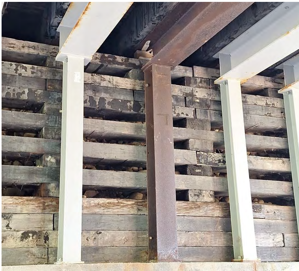
Figure 9 - Severely Corroded Steel Column and Girder (5 th from South) – no stiffener plates present.
