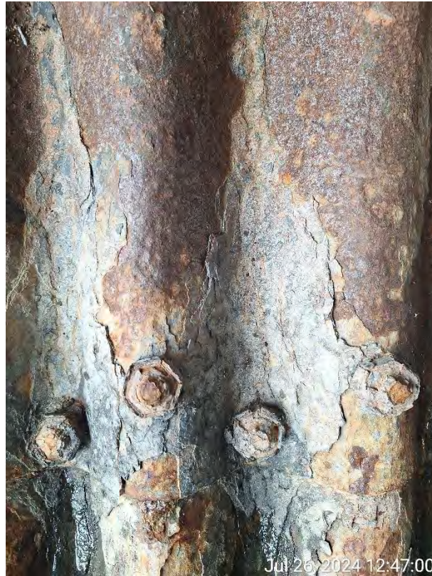
Figure 10: Severe corrosion of culvert barrel, bolts and nuts.
