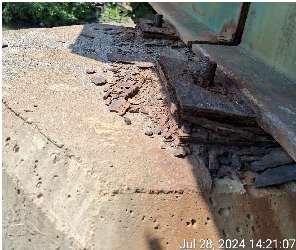
Figure 6 - Severely Corroded Pier Bearings and pines.
