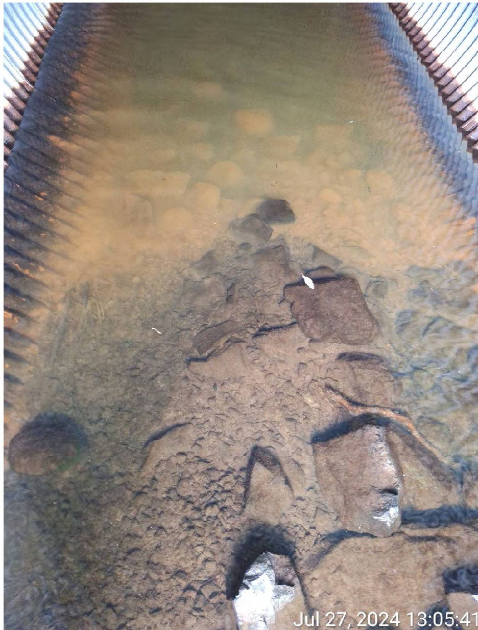
Figure 3 - Debris at Inlet, severe corrosion of barrel along waterline
