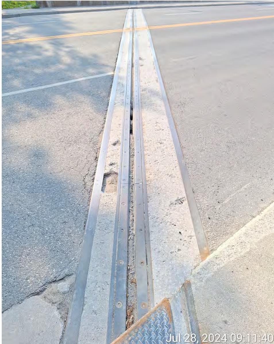
Figure 12 - North Expansion Joint
