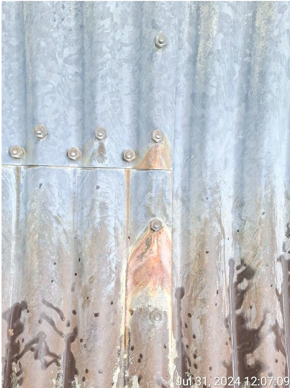
Figure 8: Corrosion near bolts.
