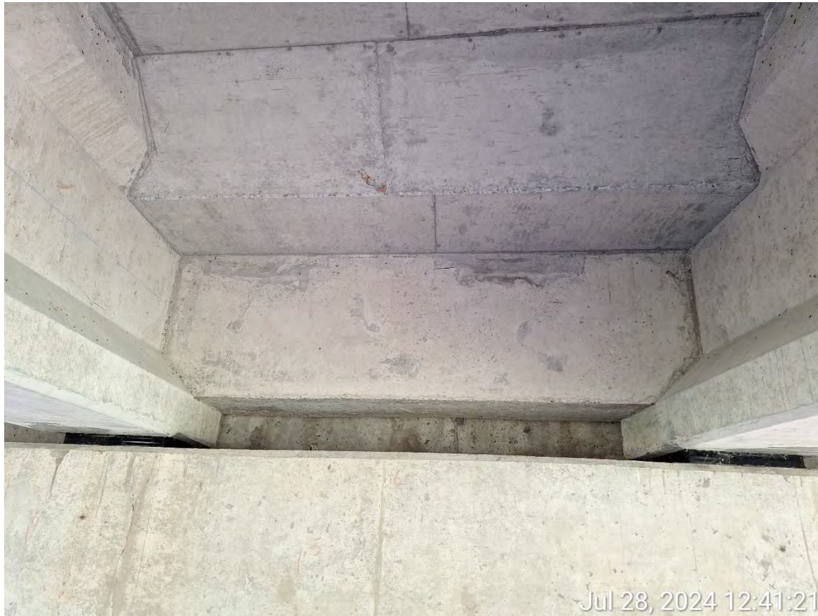
Figure 9: Concrete diaphragm.
