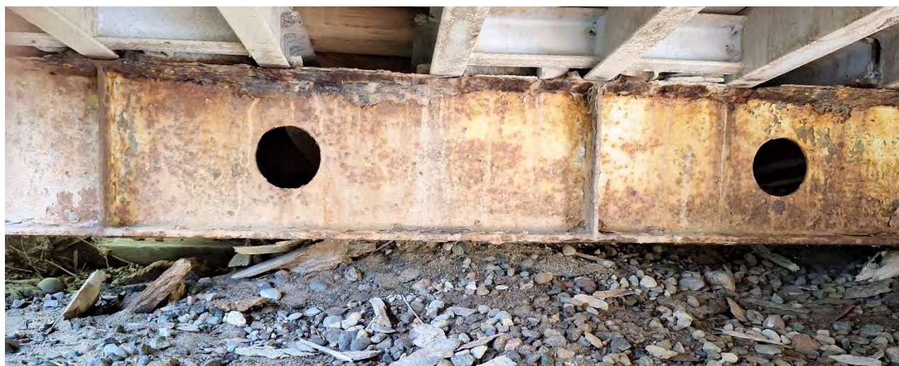
Figure 15 - Corroded Transoms, Top flange
