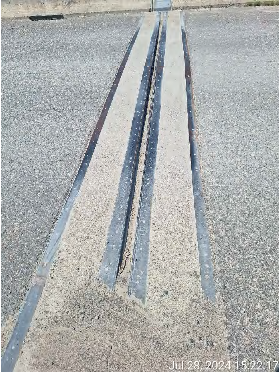
Figure 18 - Expansion Joint
