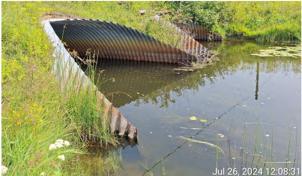
Figure 4 – Culvert Inlet
