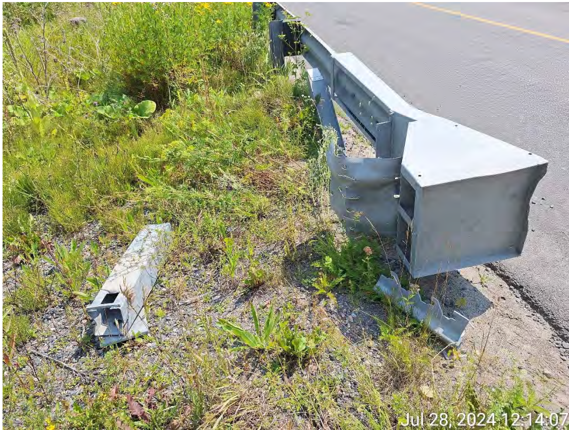
Figure 3: Damaged SBEAT At NW quadrant. In need of immediate repair or replacement. SAFETY CONCERN.
