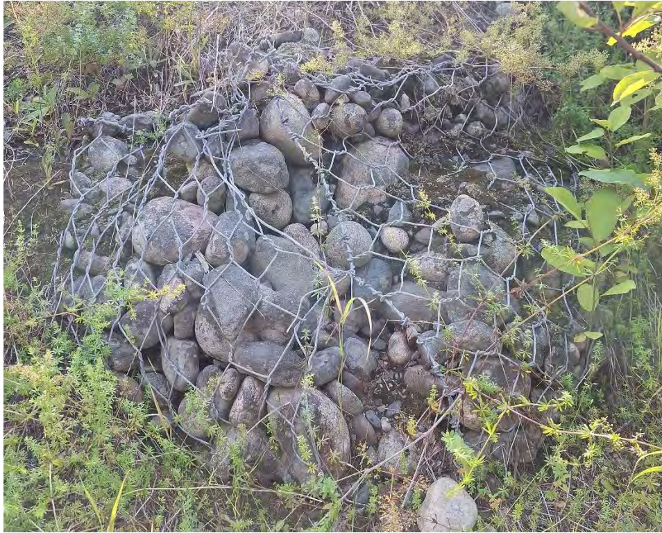
Figure 3 - Hole in Gabion Basket
