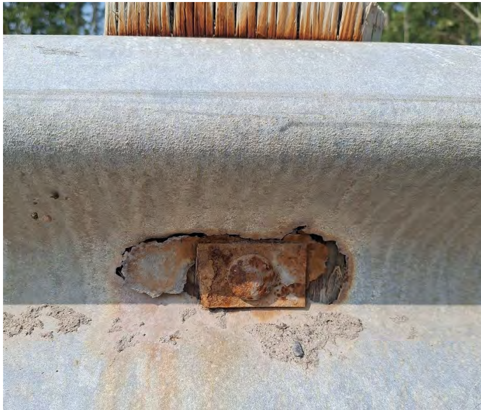
Figure 20 - Rusty rail, bolt and enlarged bolt hole in rail due to deterioration.
