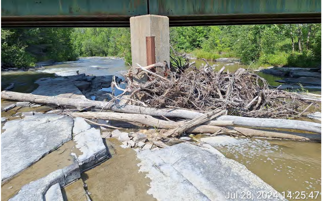
Figure 13 - Debris Buildup on end of Pier
