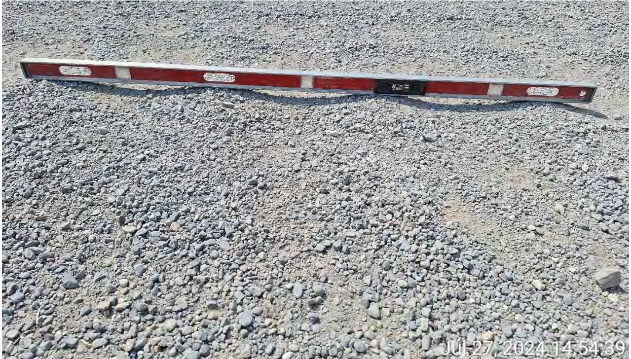
Figure 4 - Wash boarding on gravel Wearing Surface
