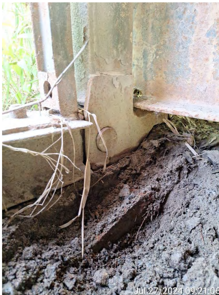
Figure 14: Bearing pad covered in debris
