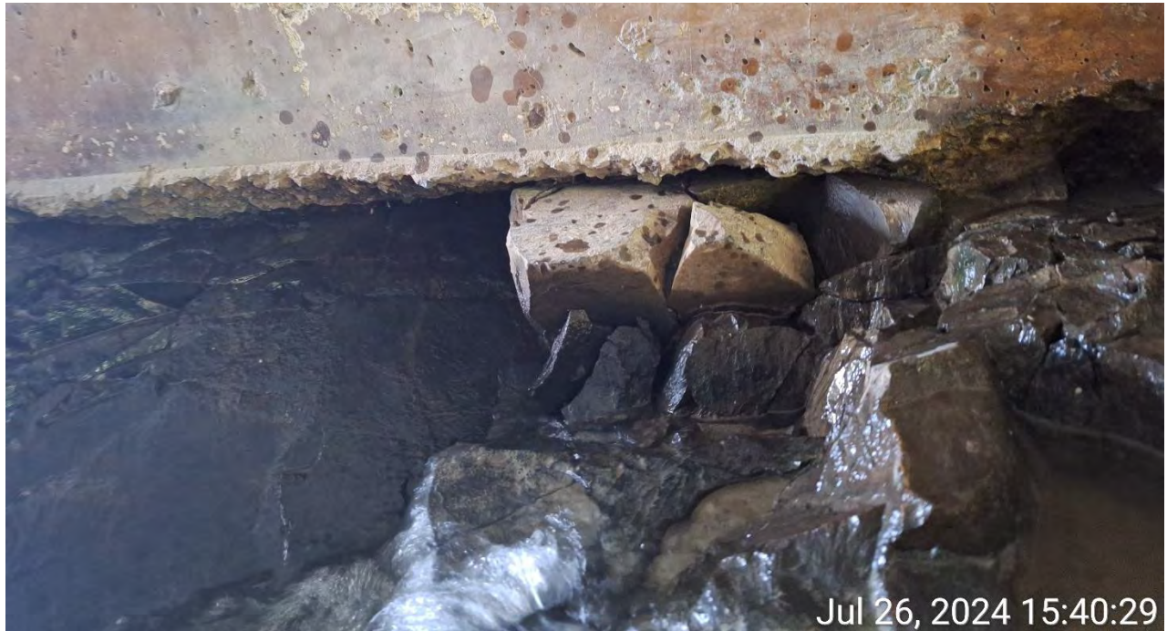
Figure 9 - Undermining at Bottom Footing
