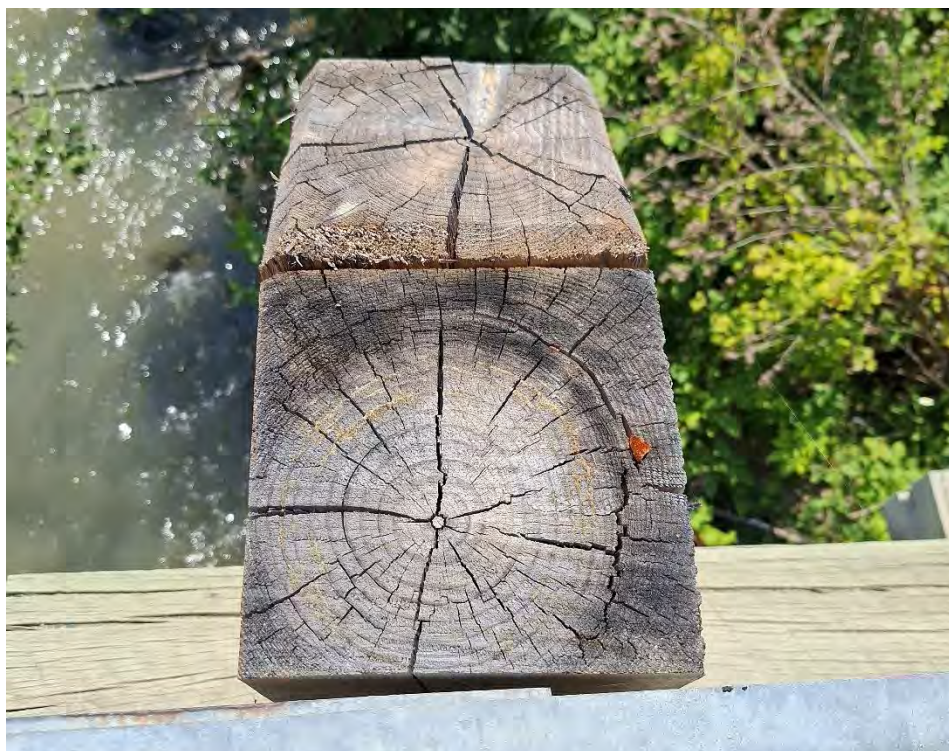
Figure 16 - Light Weathering on Wooden Post
