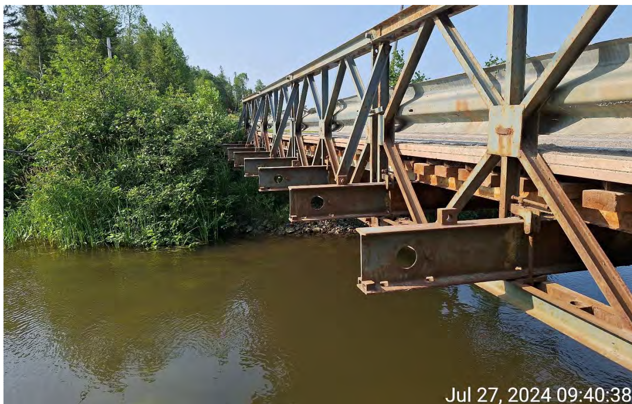
Figure 20 – Outside of Truss, corrosion can be seen throughout.
