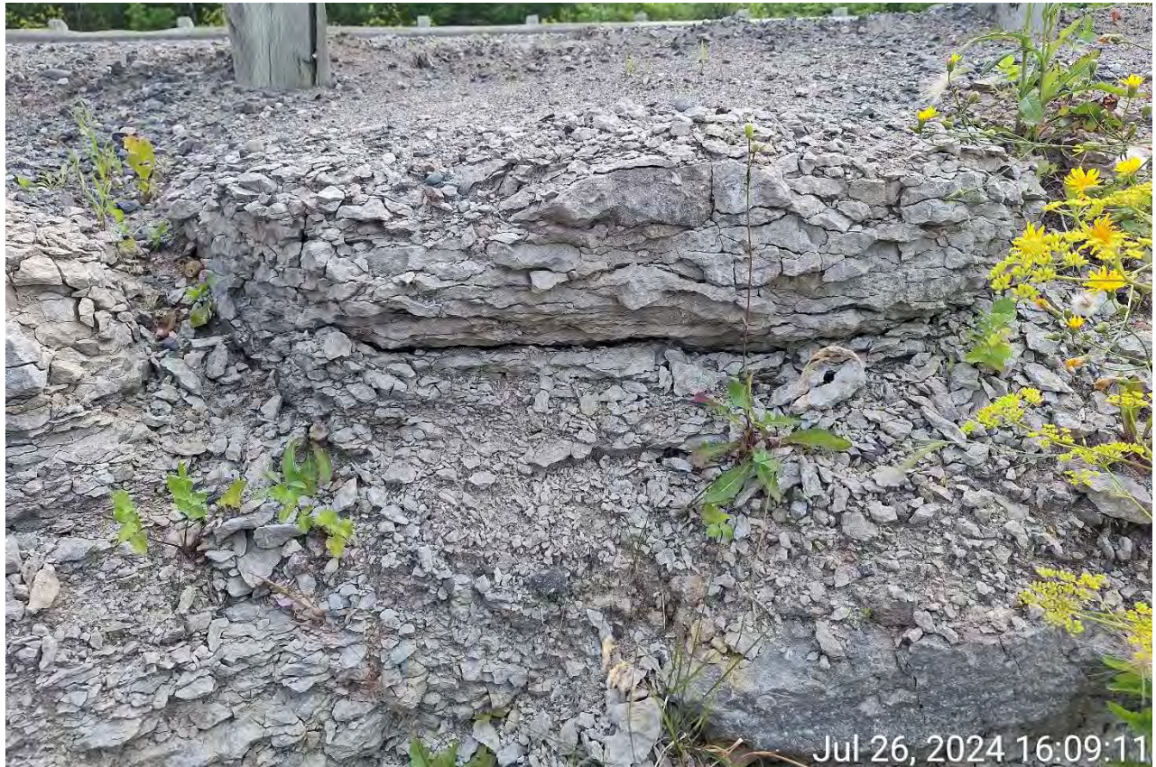
Figure 11 - Disintegration of Retaining Wall
