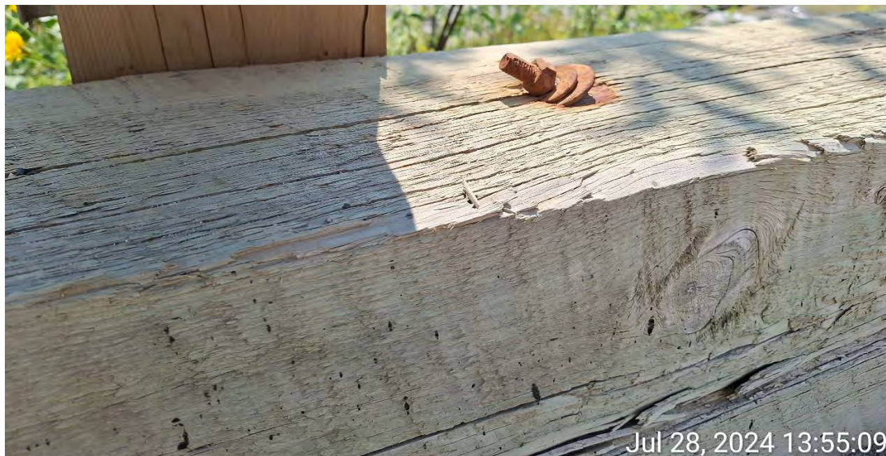
Figure 15 - Damaged Bolt on Curb
