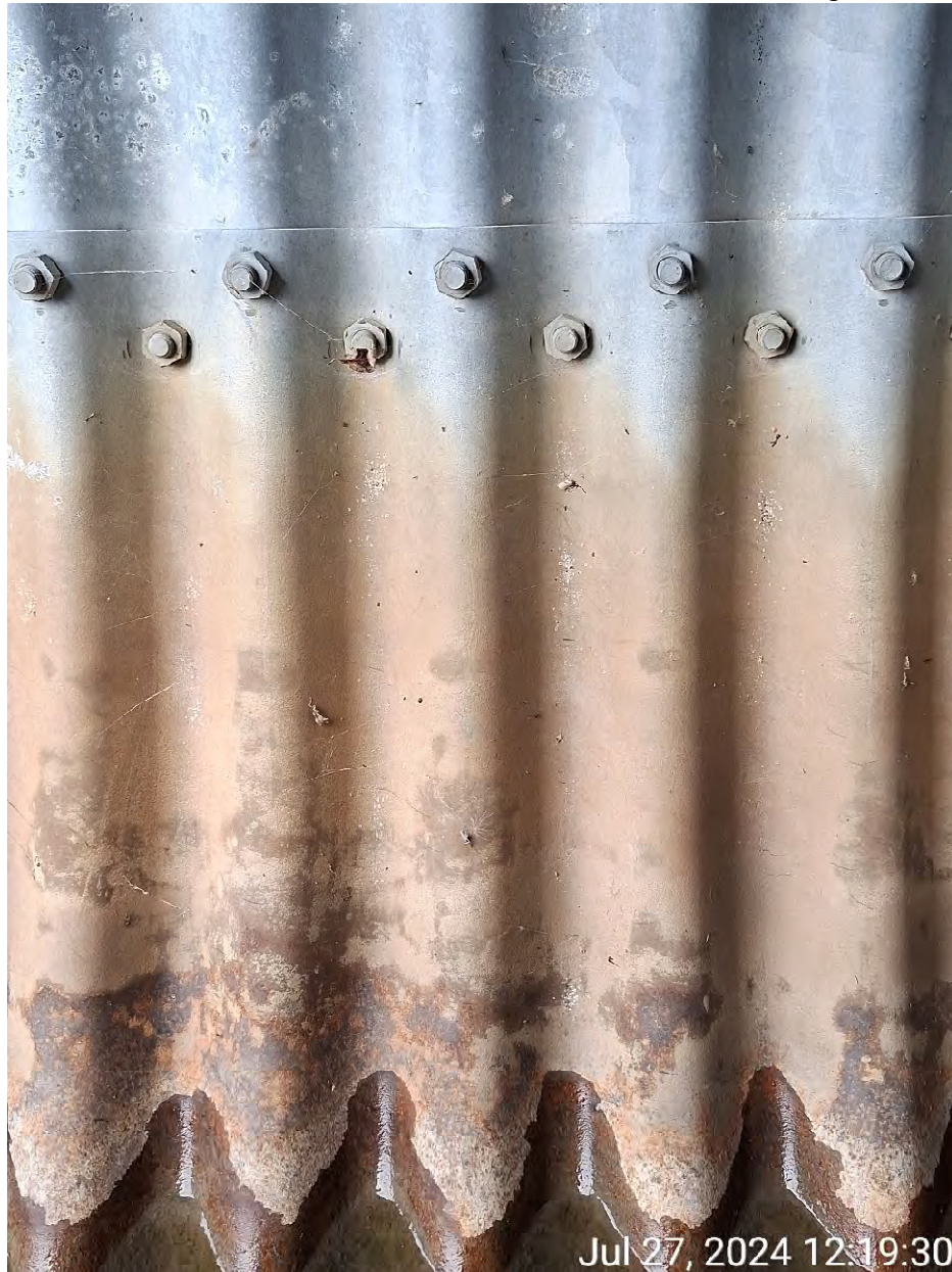
Figure 3: Light and medium corrosion above waterline.
