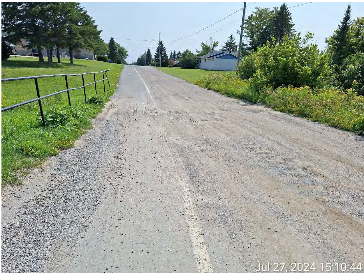
Figure 1: View looking South – asphalt and gravel wearing surface
