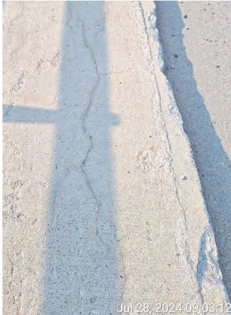
Figure 10 - Cracks and Scaling on Sidewalk
