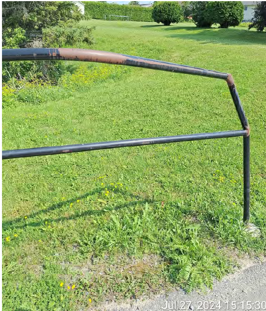
Figure 3: Bent hand rail with corrosion and loss of coating.
