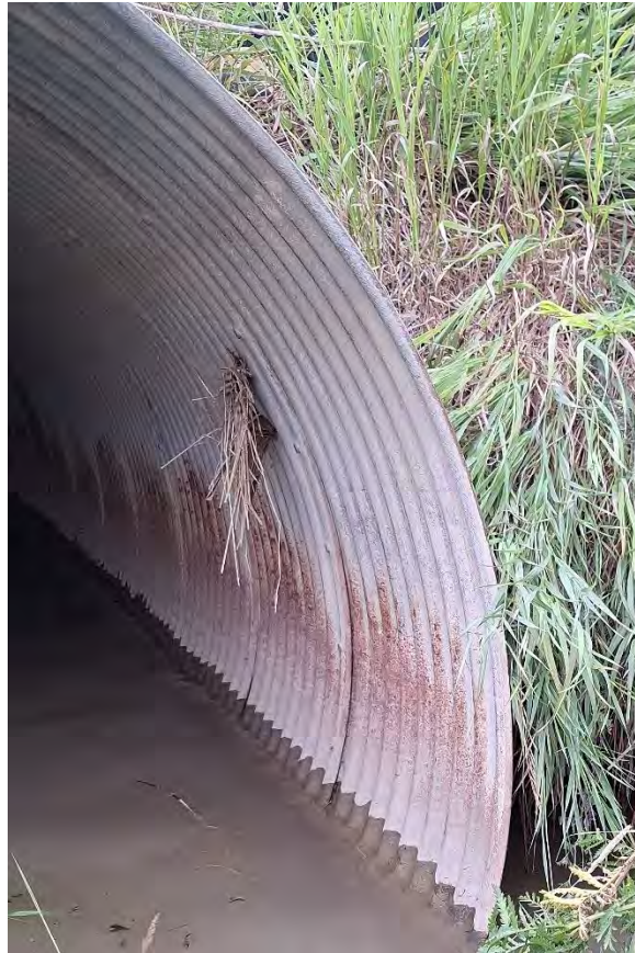
Figure 5: Hole in culvert barrel with grass.
