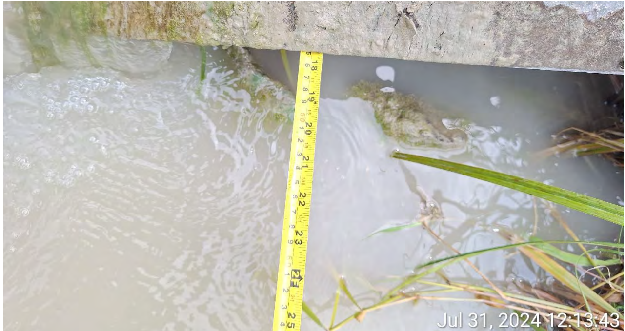
Figure 11 - Undermining at Outlet
