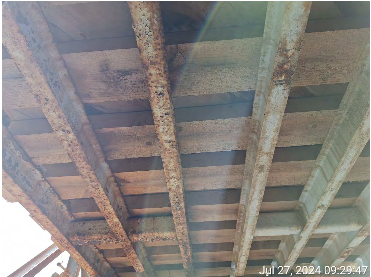
Figure 18 – Stringers with medium (left) and light (right) corrosion.
