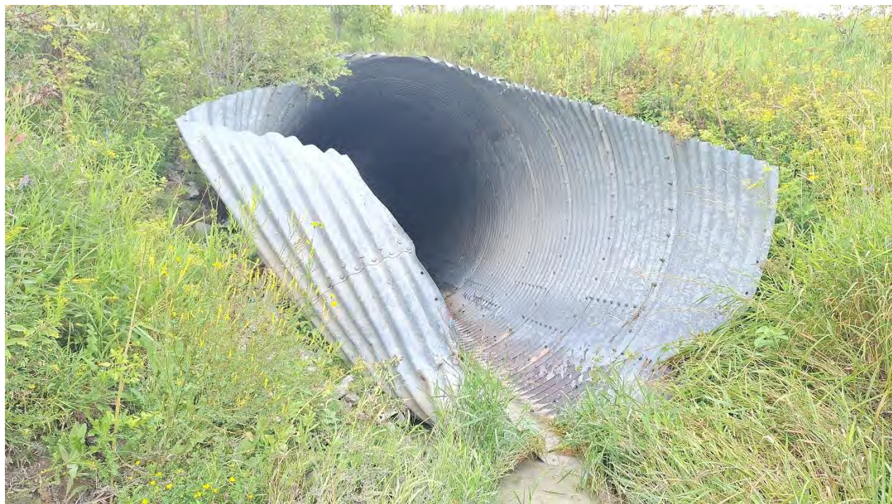
Figure 4 - Damage at Inlet of culvert barrel.
