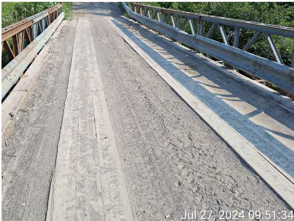
Figure 2 - Wearing Surface running boards and sand on deck top
