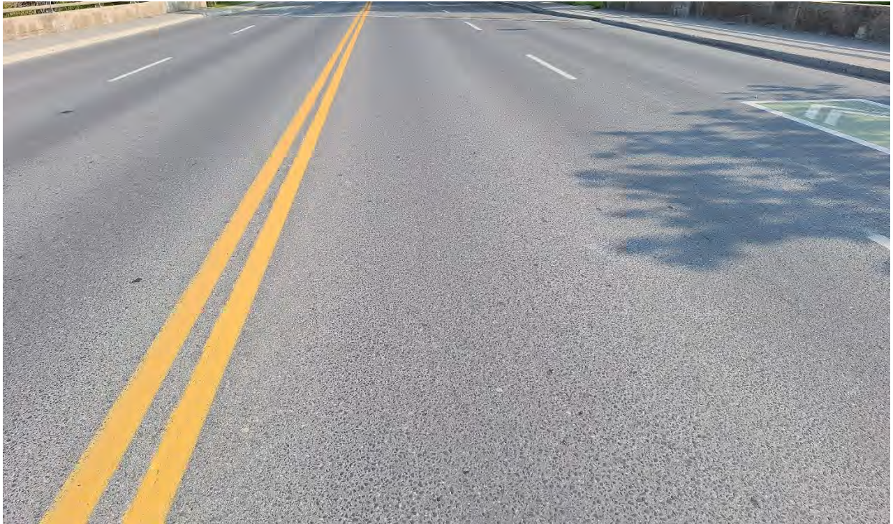
Figure 9 – Asphalt Wearing Surface
