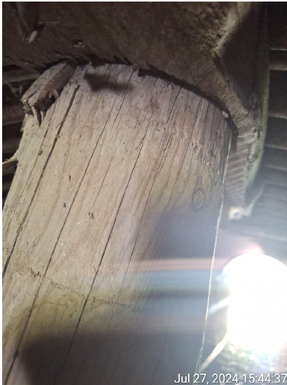
Figure 14: Crushing of block above vertical support.
