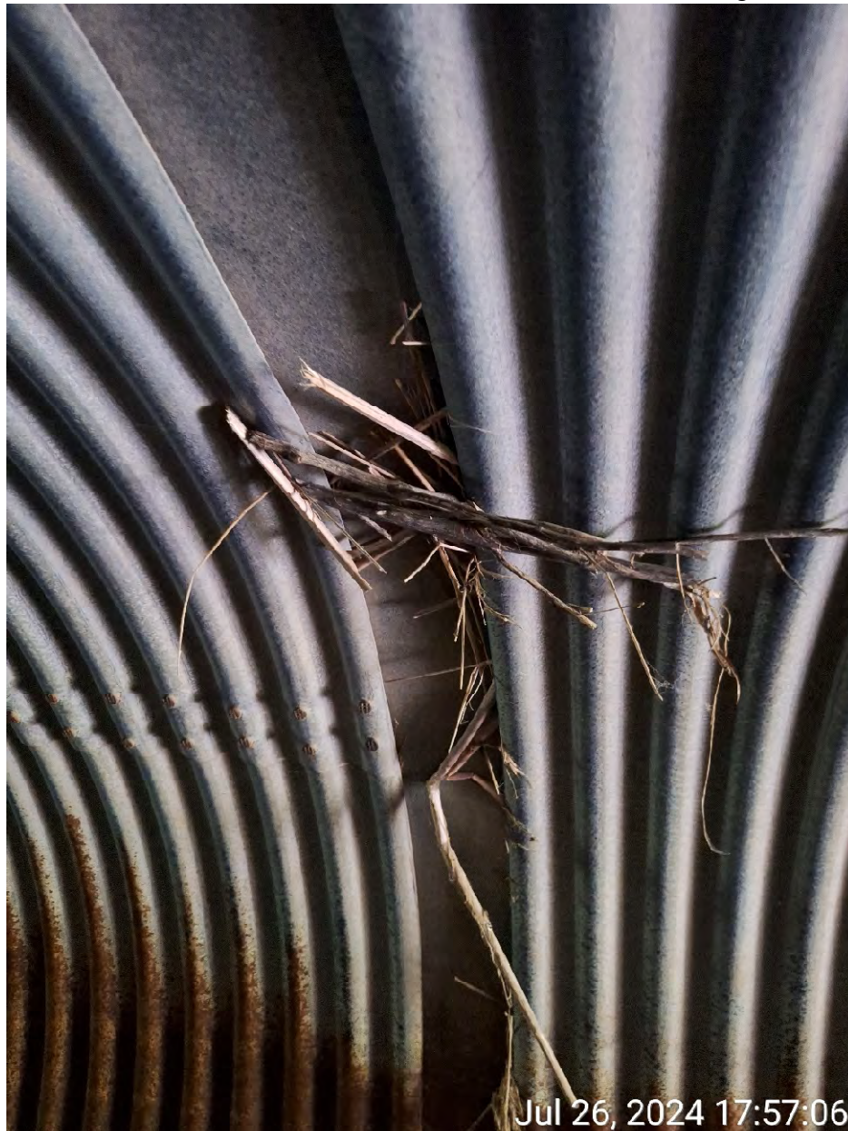
Figure 6: Debris in culvert joint/gap, suspected to be from birds.
