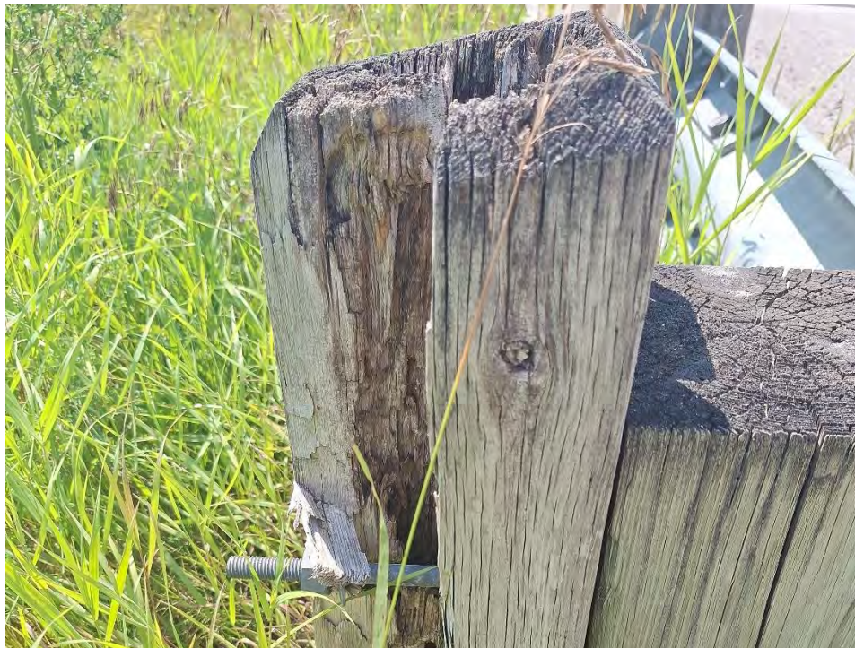
Figure 13 - Severely Damaged Post
