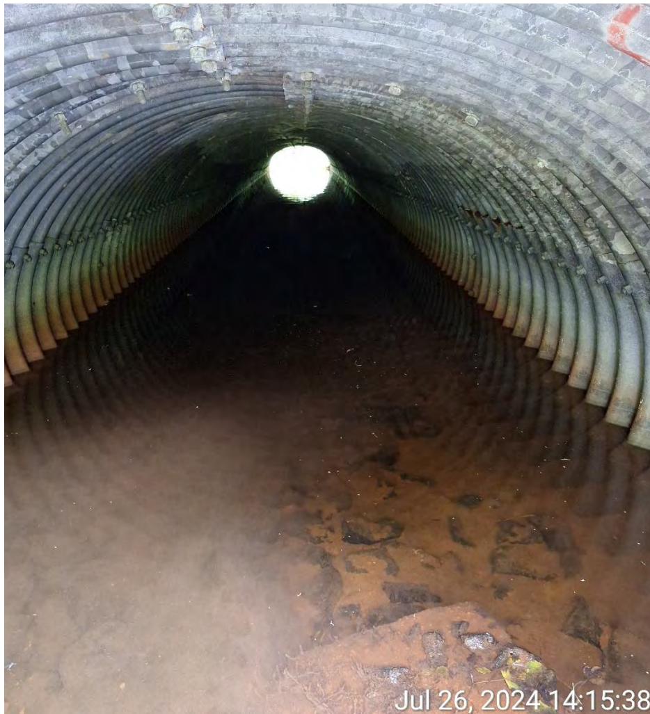
Figure 5 - Debris and Corrosion Throughout Barrel
