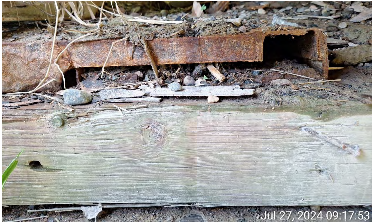
Figure 13 - Bearing Plate with severe corrosion, perforations, and debris.
