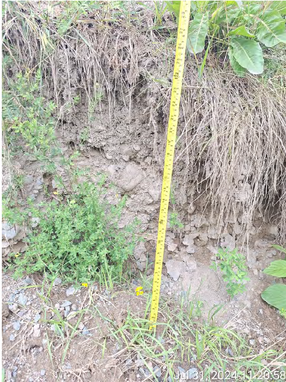
Figure 8 – Erosion Above Outlet immediately adjacent to shoulder
