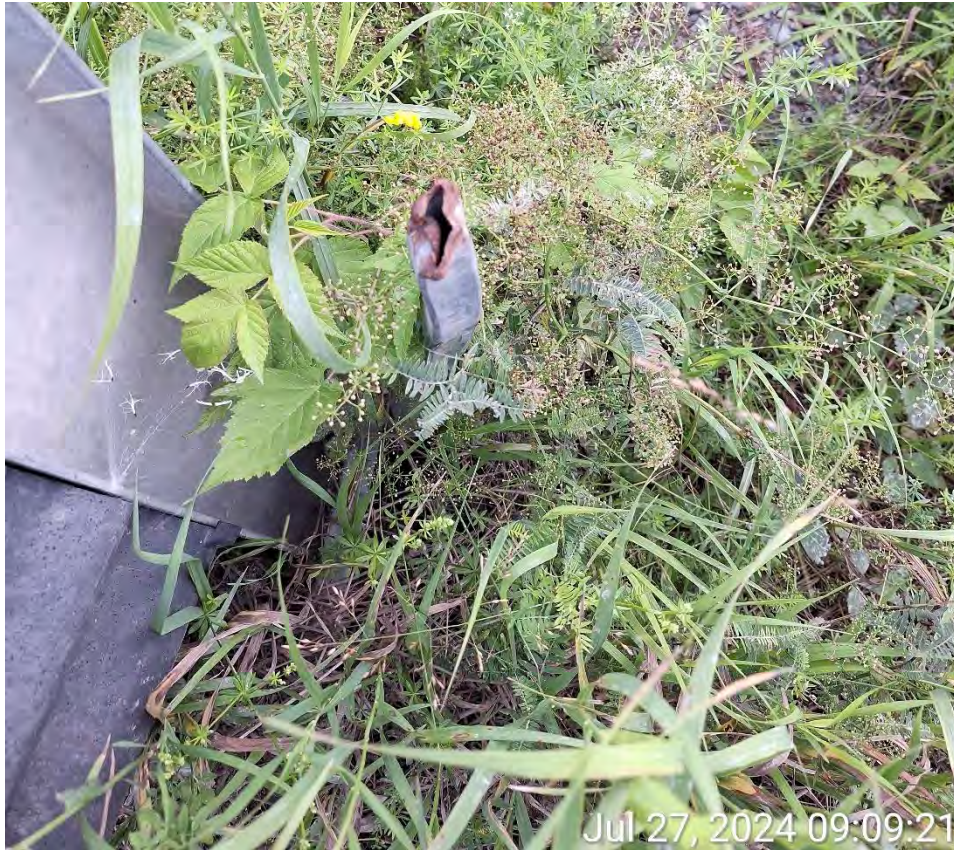
Figure 11: Broken Sign post.
