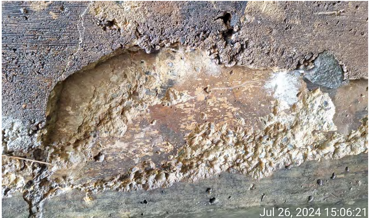
Figure 7 - Delamination and Moisture Staining on culvert barrel, northern portion.
