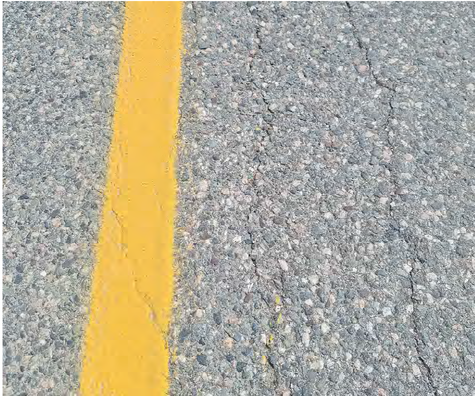
Figure 11 - Longitudinal Cracking Along Center Line
