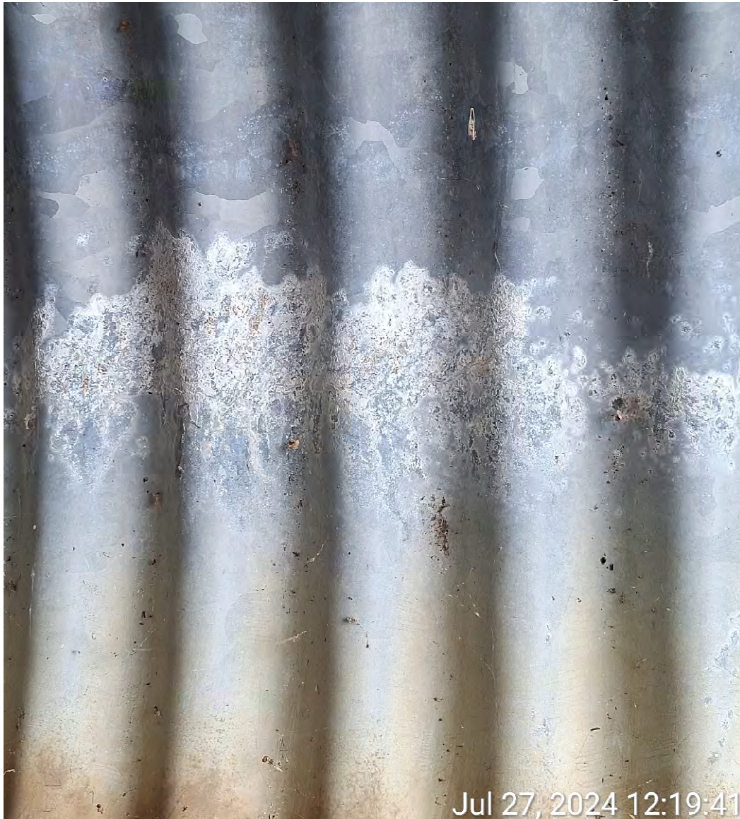
Figure 4: Patches of galvanized coating failure.
