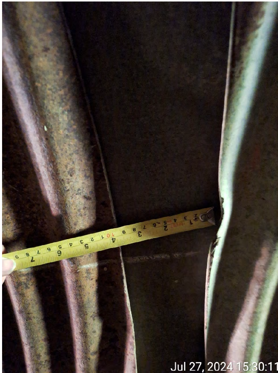
Figure 12: Joint gap
