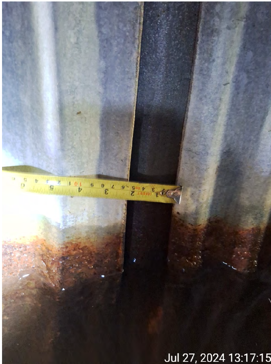
Figure 10: Gap between barrel pieces.
