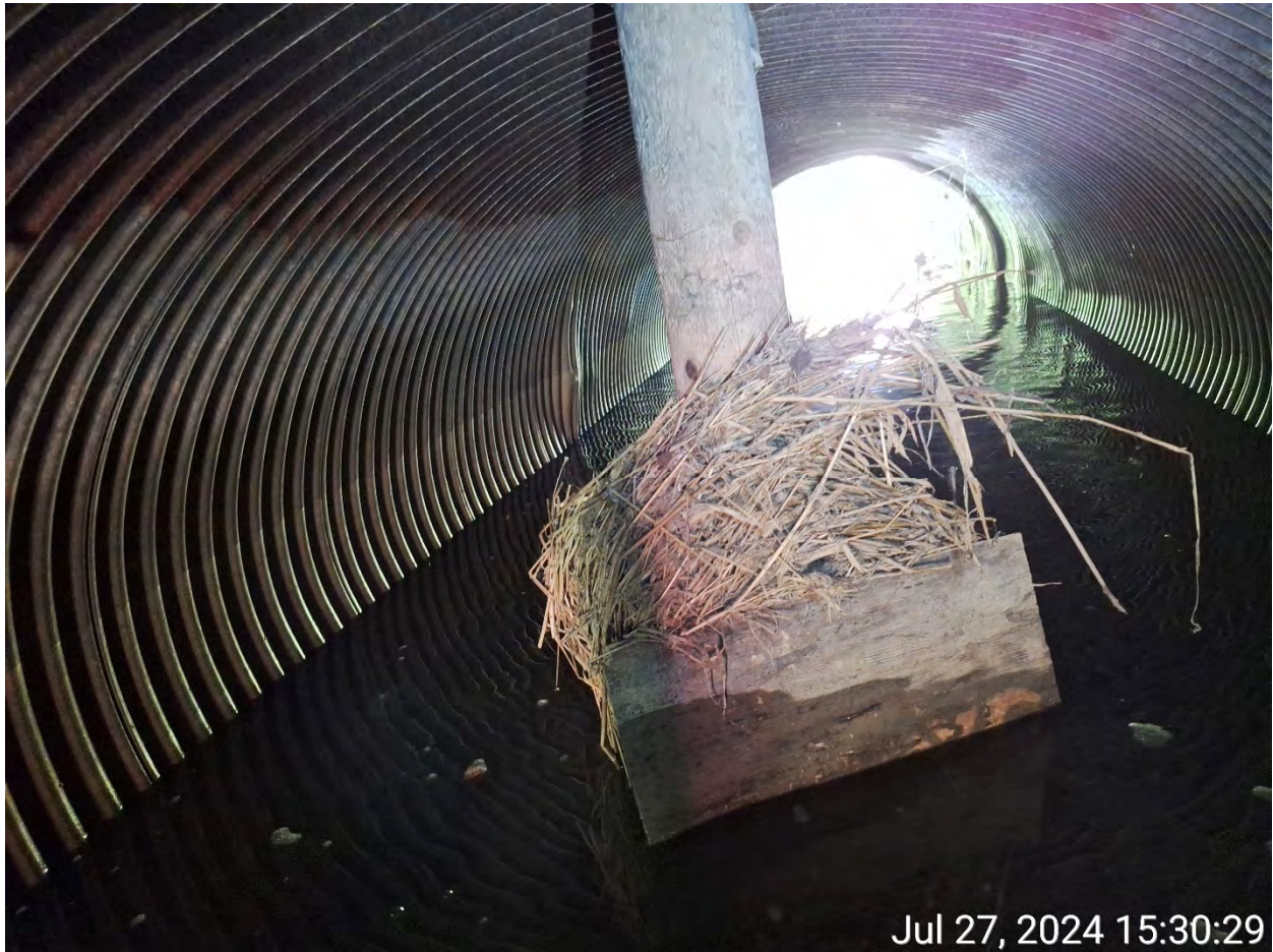
Figure 13: Obstruction in culvert that appears to be acting as a vertical support
