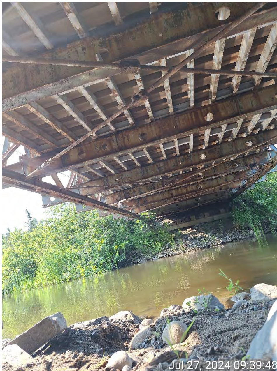
Figure 17: Overall view of underside of bridge showing extensive corrosion
