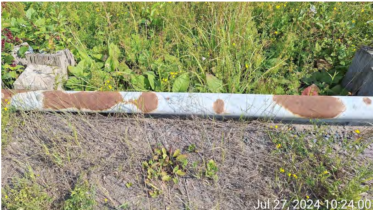
Figure 15 - Guide Rail with Medium Corrosion
