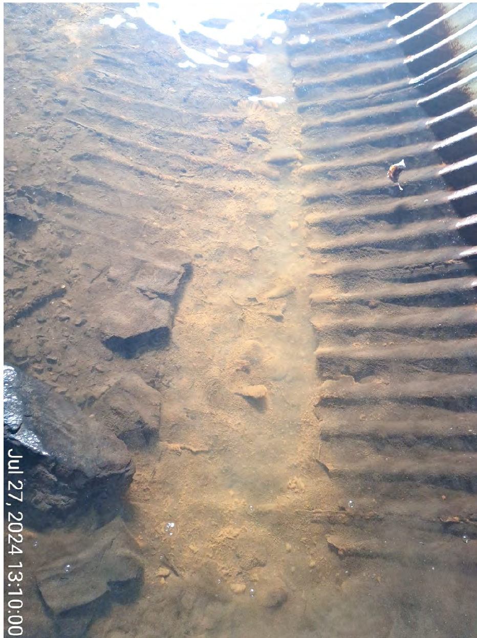
Figure 5: Culvert bottom of barrel is separated
