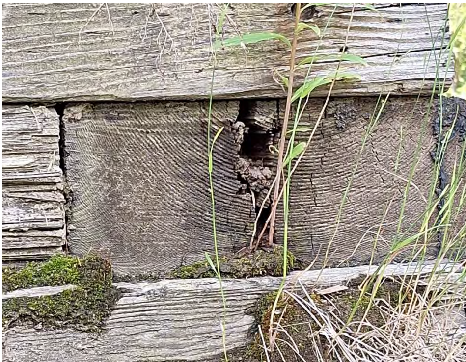
Figure 7 – Timber experiencing weathering and rot.
