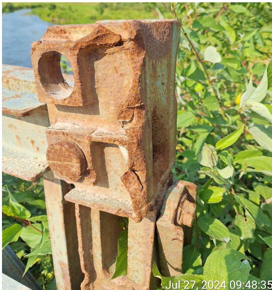
Figure 22: End panel connection point damaged and experiencing extensive corrosion.
