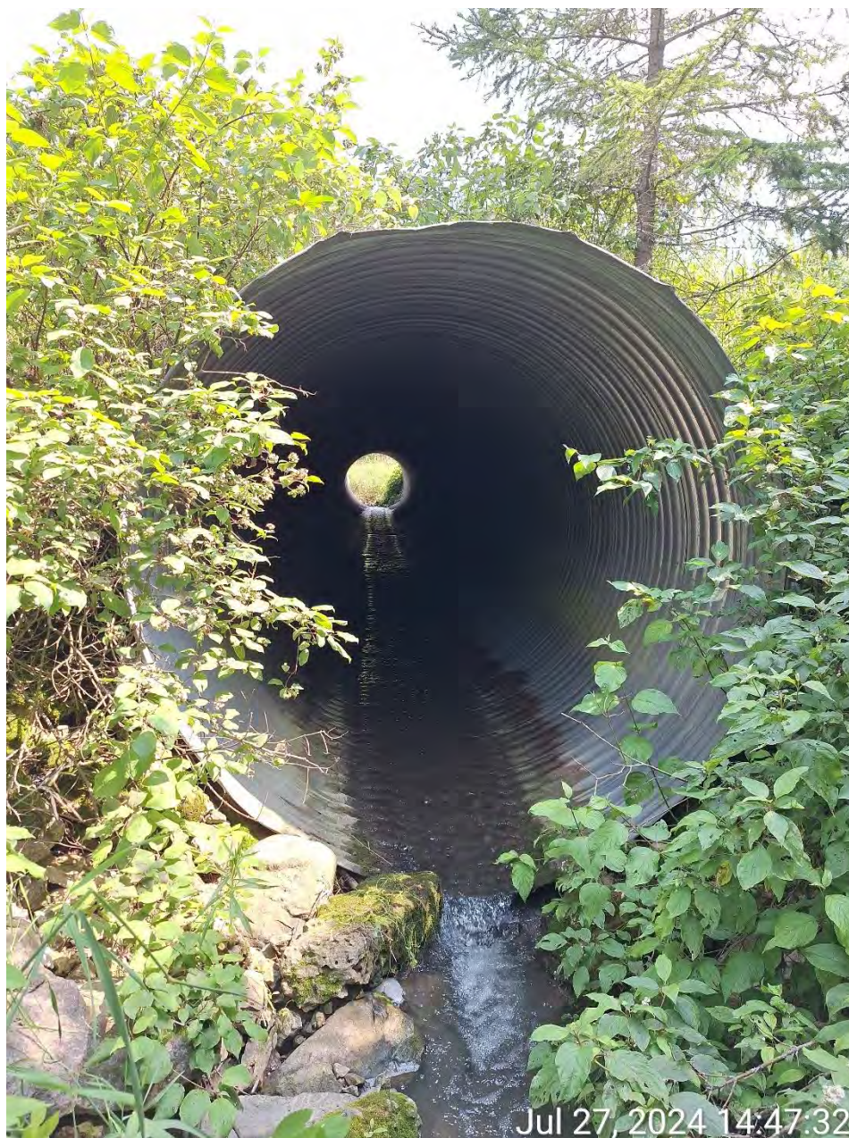
Figure 10: Perched Outlet
