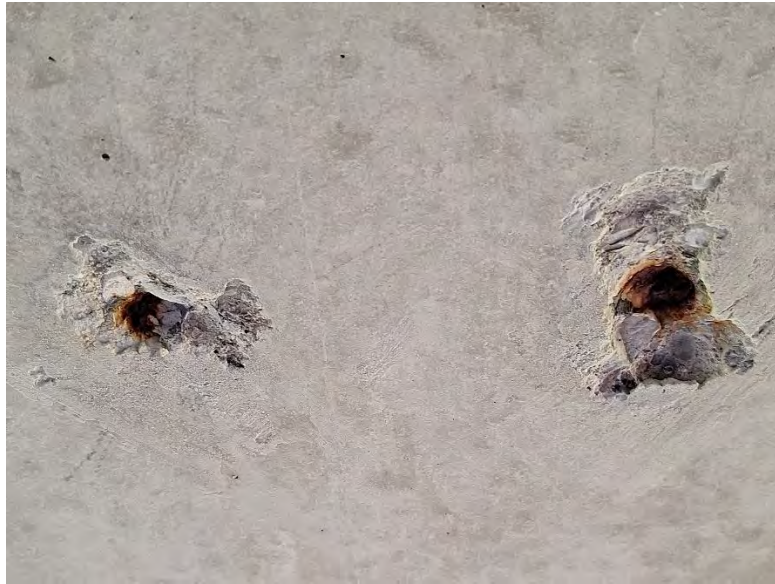
Figure 12: Small spalls exposing rebar on the girder bottom flange, close up of the damage in previous figure.
