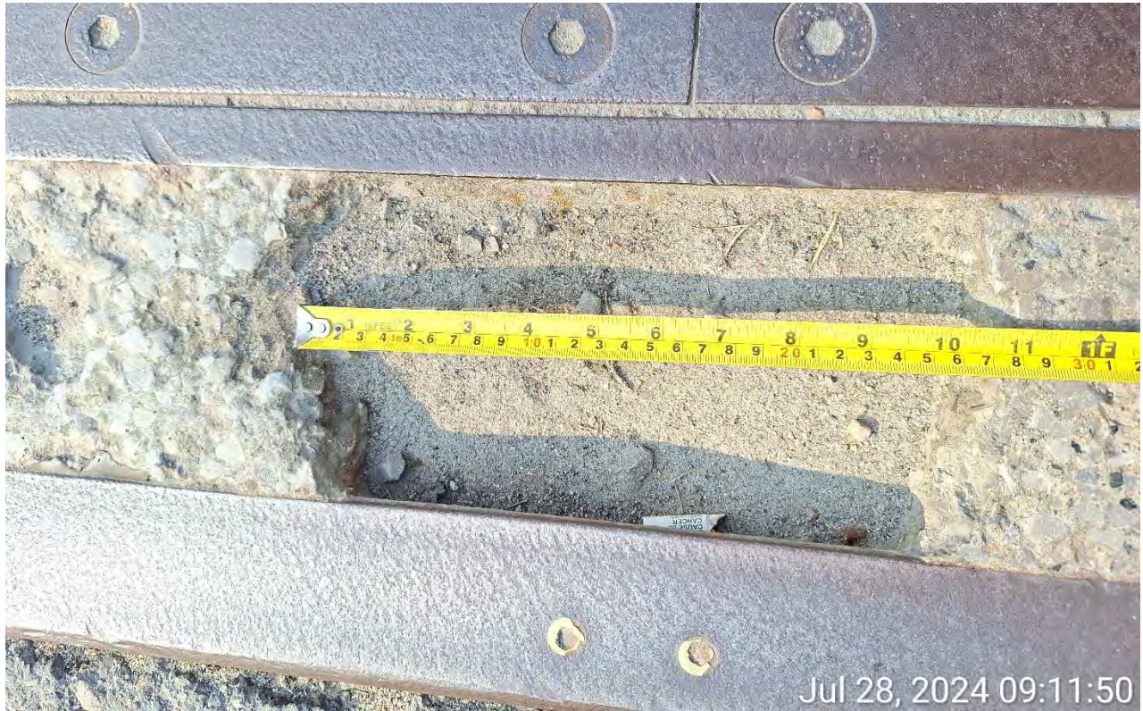
Figure 13 - Damage at North Expansion Joint
