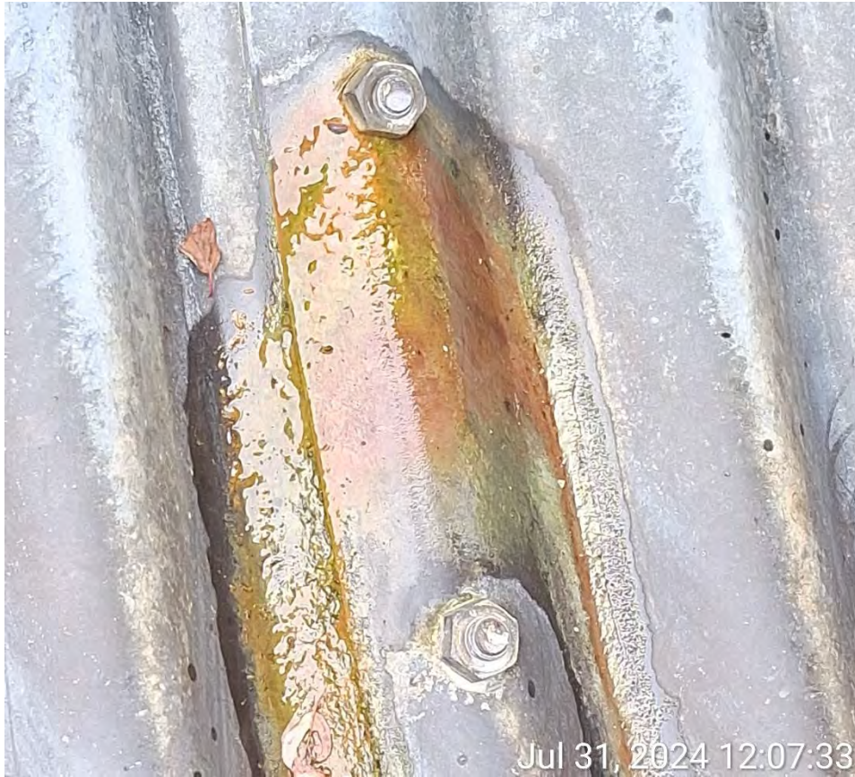
Figure 9 - Corrosion at Connection, water seeping in at bolt connection.
