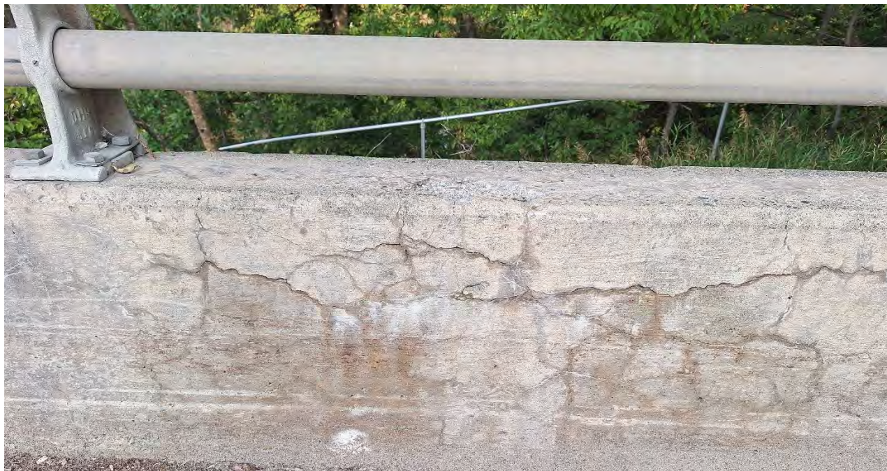
Figure 5 – Cracks and water staining on Interior Barrier Wall
