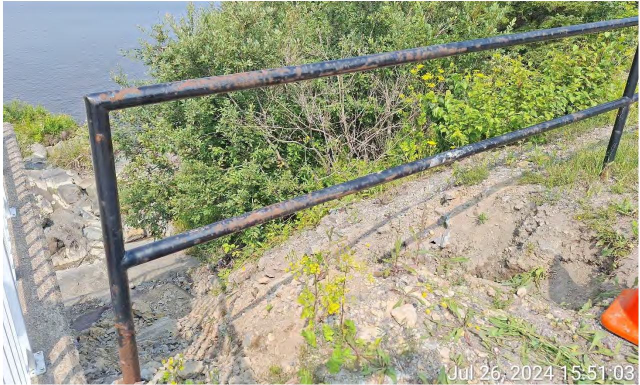
Figure 15 - Corrosion on Railing (North side)
