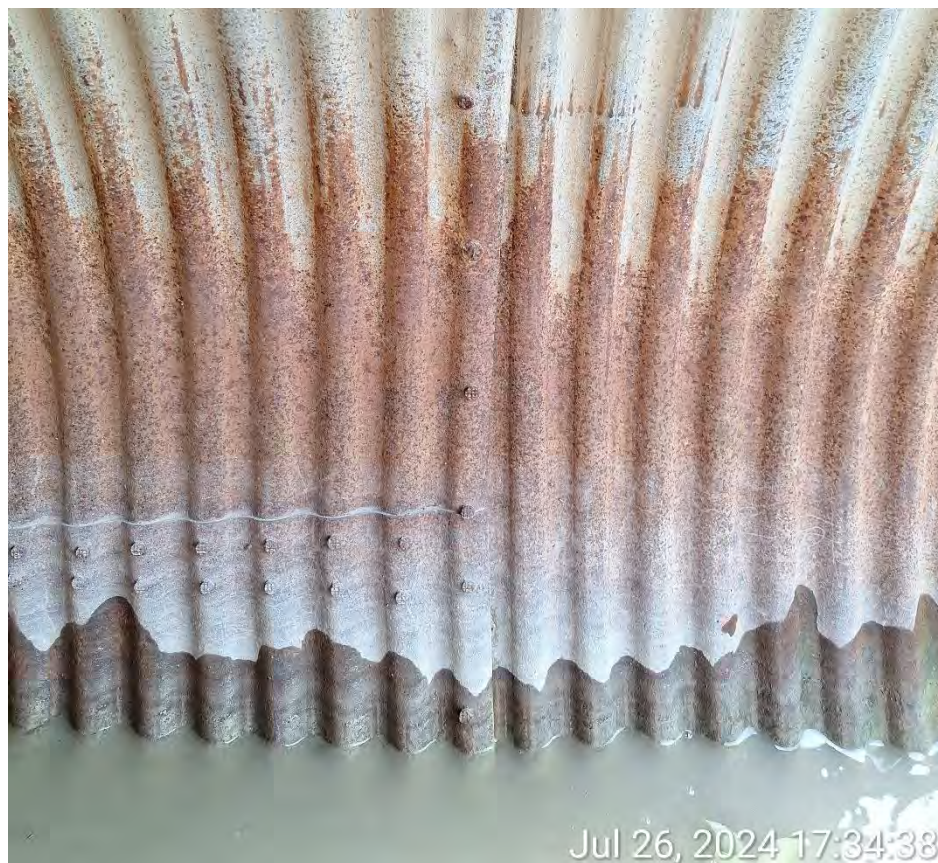
Figure 3 - Corrosion Along Barrel near spring line
