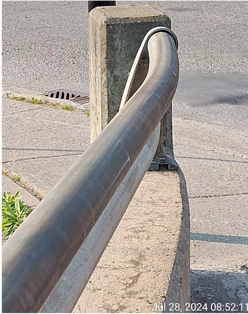
Figure 17: Bent Railing tube.
