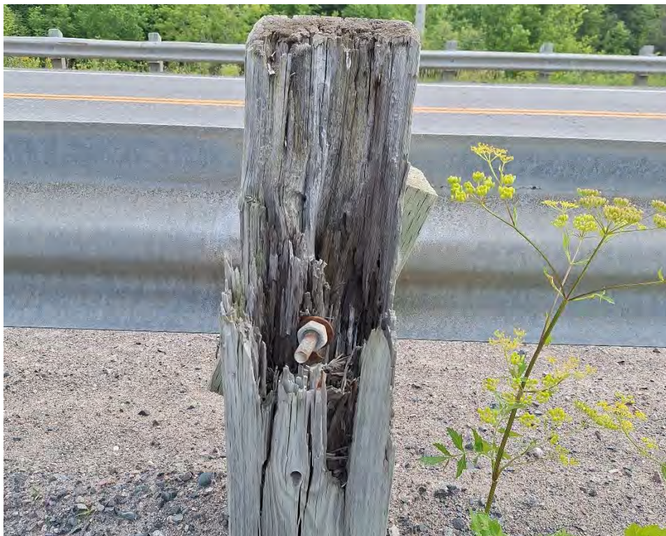
Figure 18 - Severely Damaged/Deteriorated wooden guiderail Post
