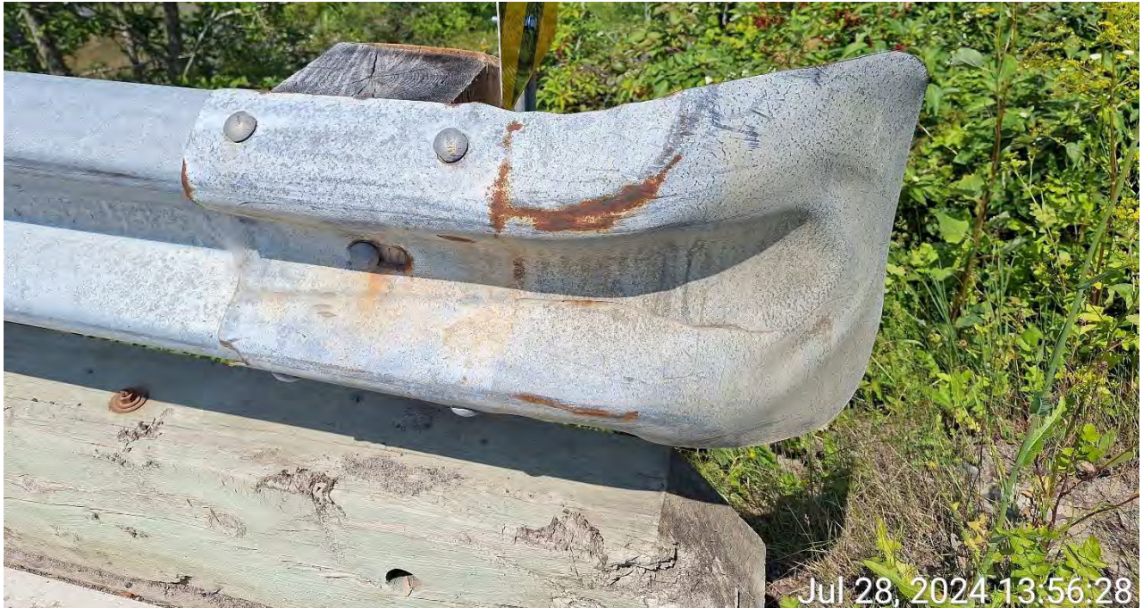
Figure 18 - Damaged End Panel
