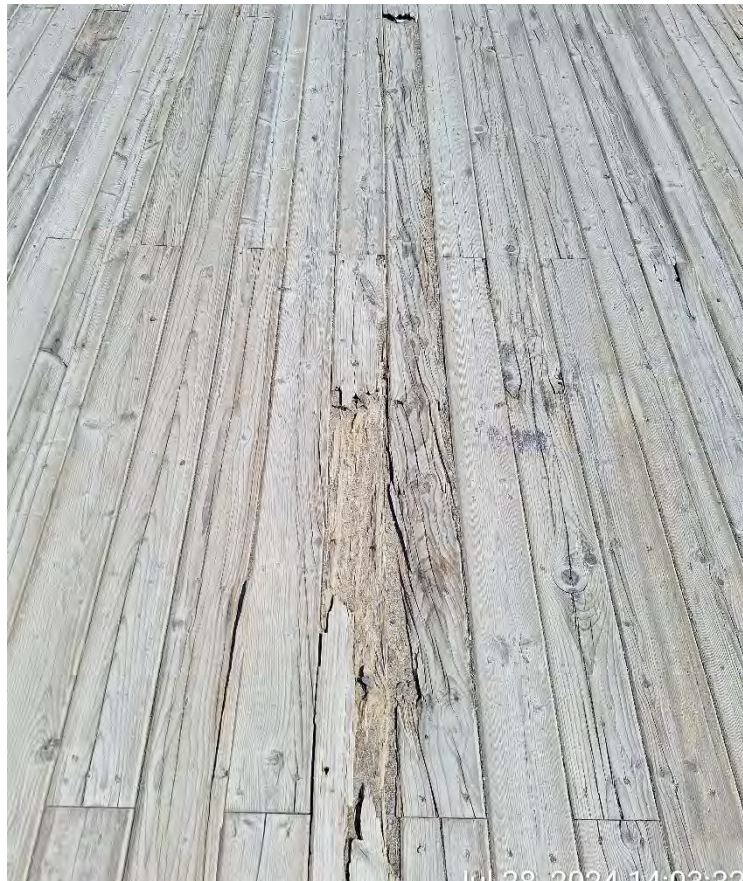
Figure 12 - Damaged Boards in deck wearing surface
