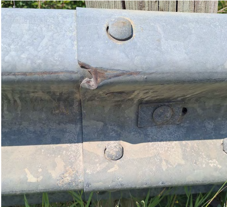
Figure 14 - Damaged Guide Rail
