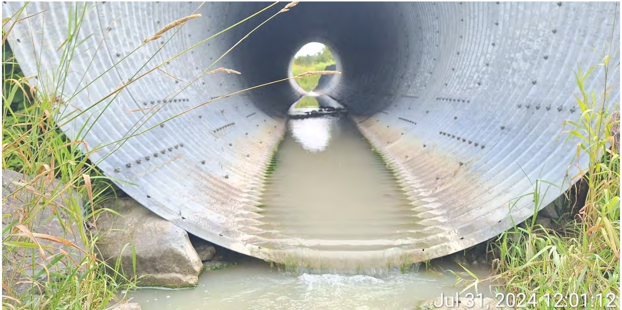
Figure 10 – Light to medium Corrosion at Bottom of Barrel, perched outlet.
