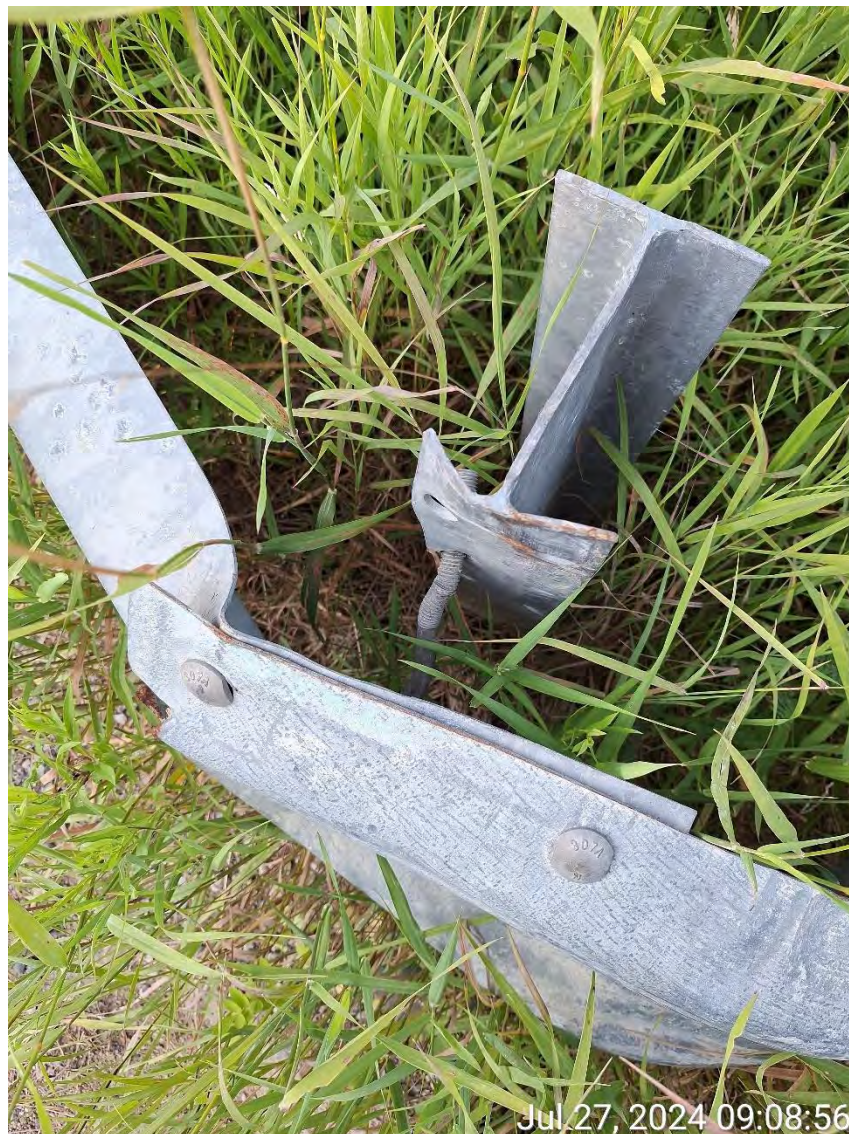
Figure 10: guiderail - improper connection.
