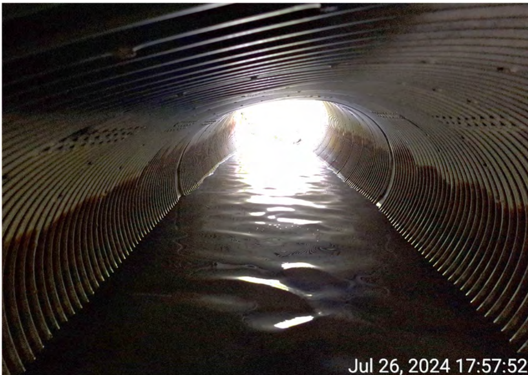
Figure 3 - Deformation in Barrel
