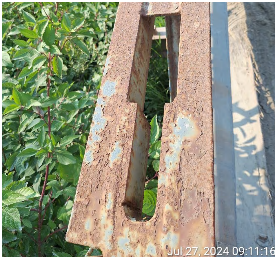
Figure 23 – Failed Coating and Corrosion on Truss
