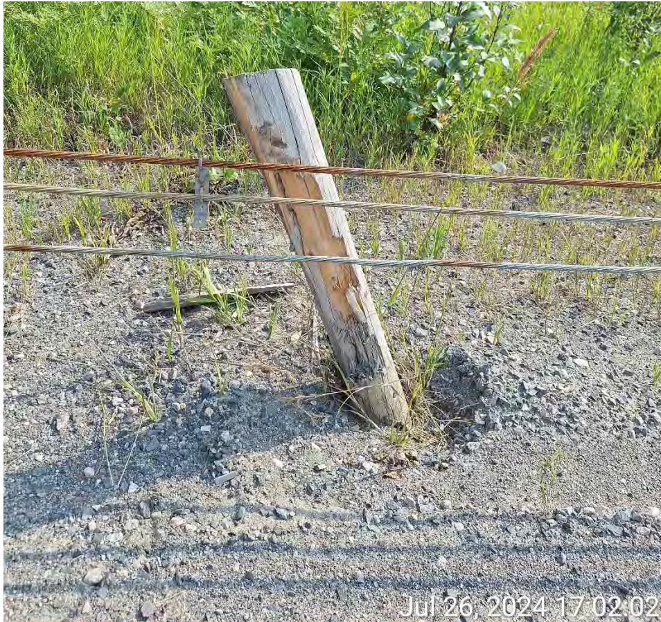
Figure 21 - Damaged wooden 3CGR Post
