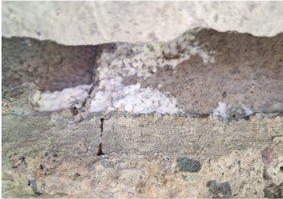
Figure 3 - Efflorescence
