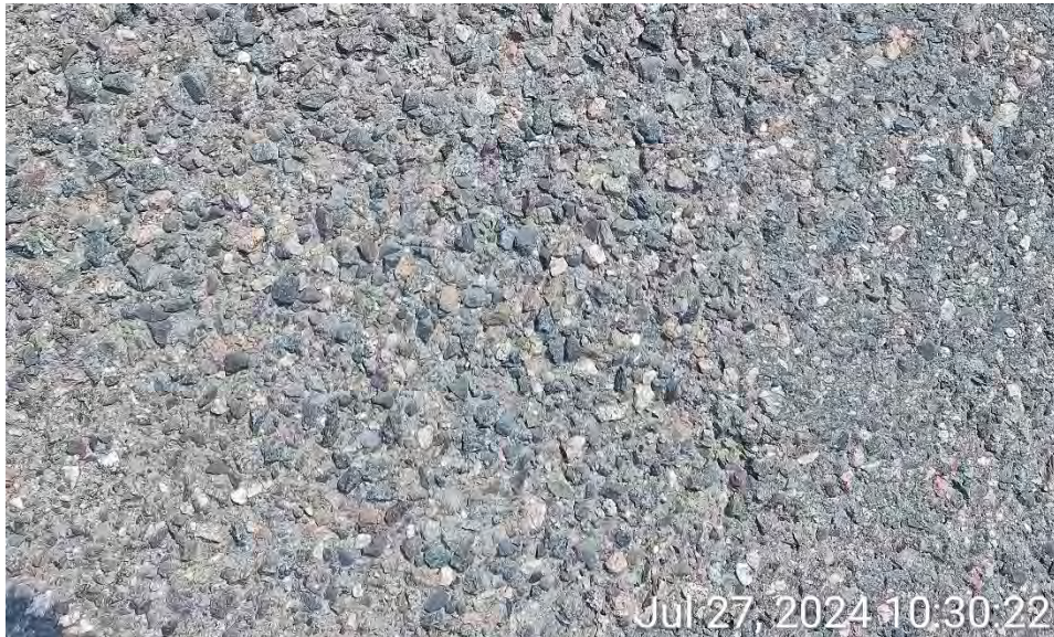
Figure 12 - Raveling on Asphalt Wearing Surface
