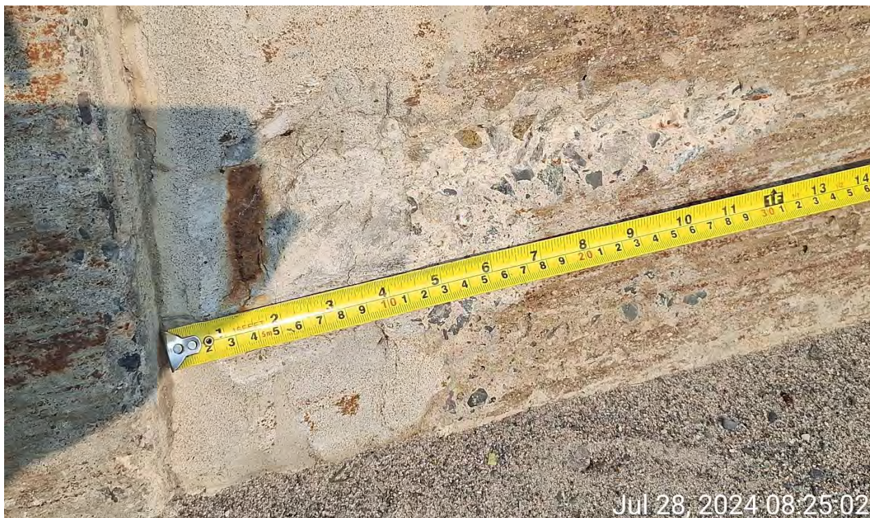
Figure 6 - Exposed Rebar in a Spall on Barrier Wall
