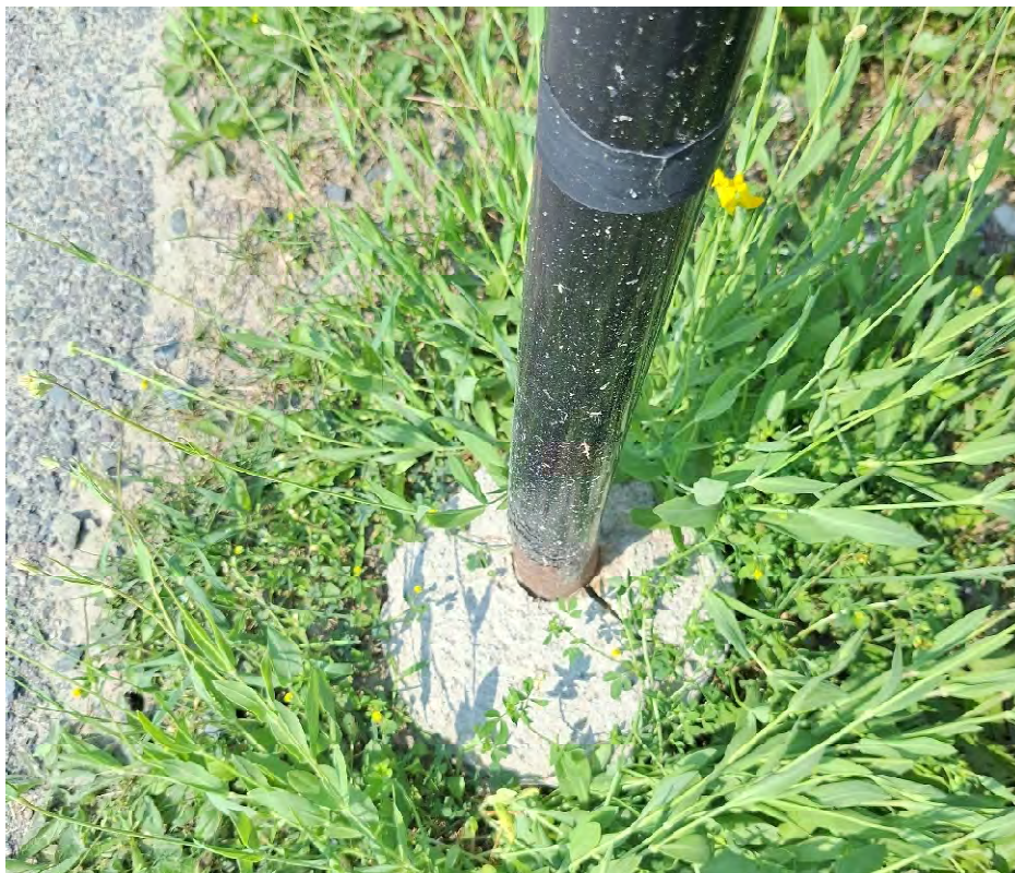
Figure 6: Concrete Footing with crack
