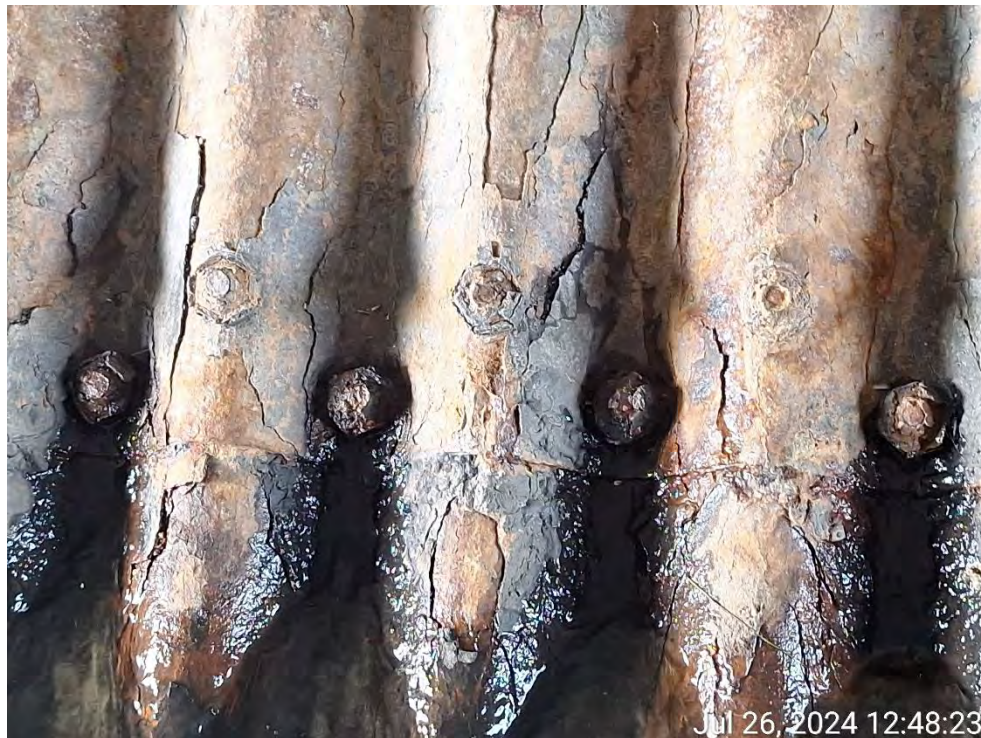
Figure 11: Severe corrosion of culvert barrel, bolts, and nuts near waterline.
