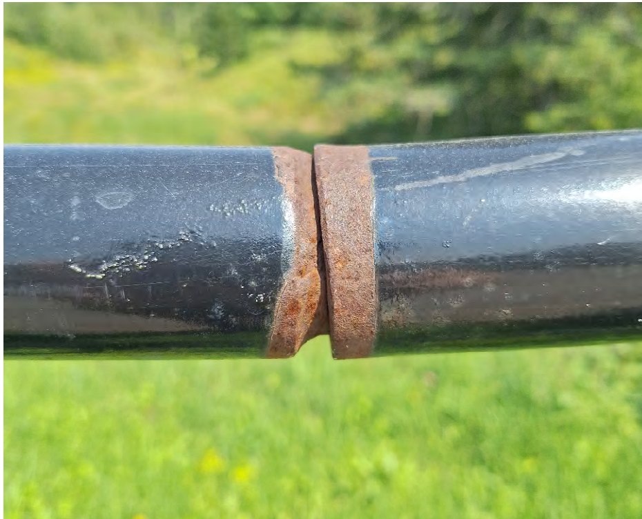
Figure 5: Hand rail joint with corrosion
