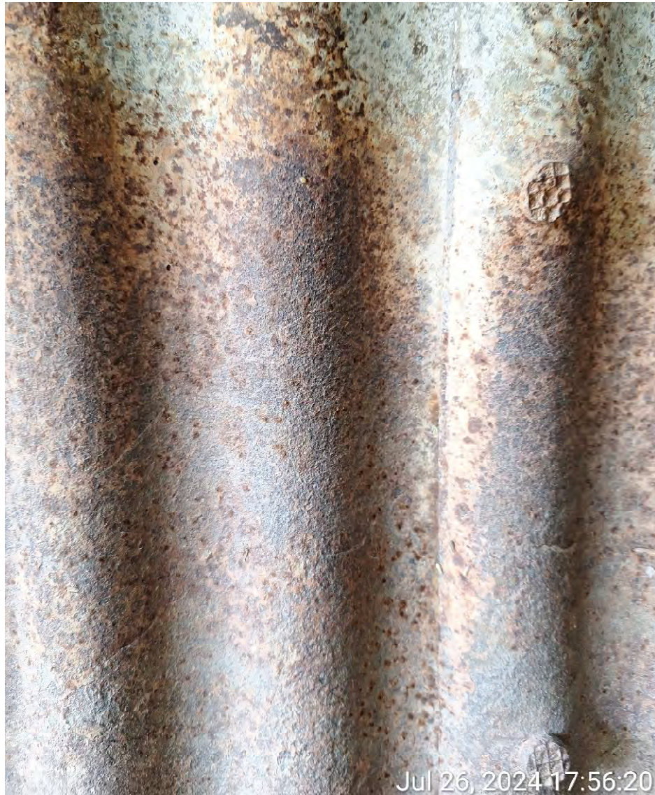
Figure 5: Corrosion of culvert barrel with some pitting.
