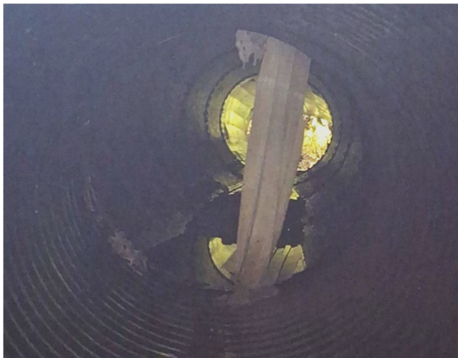
Figure 4 - Hanging Debris and ponding water
