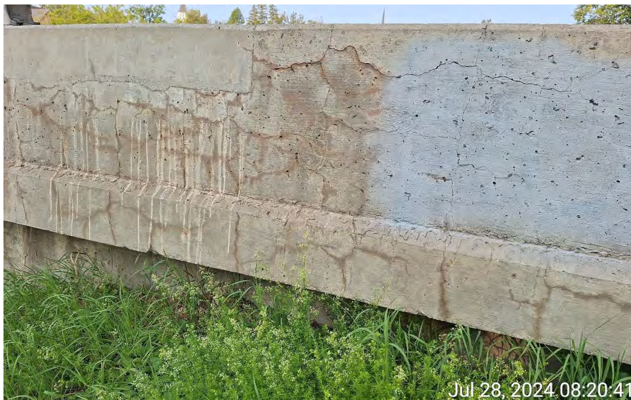
Figure 4 - Outside of Barrier Wall showing cracks, and water staining.
