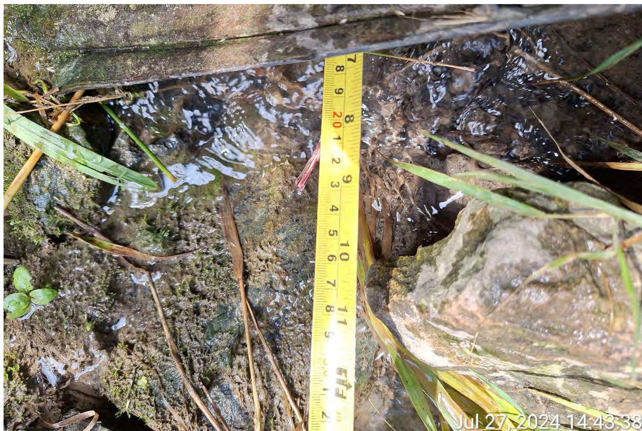
Figure 9 – Undercutting at End of Culvert
