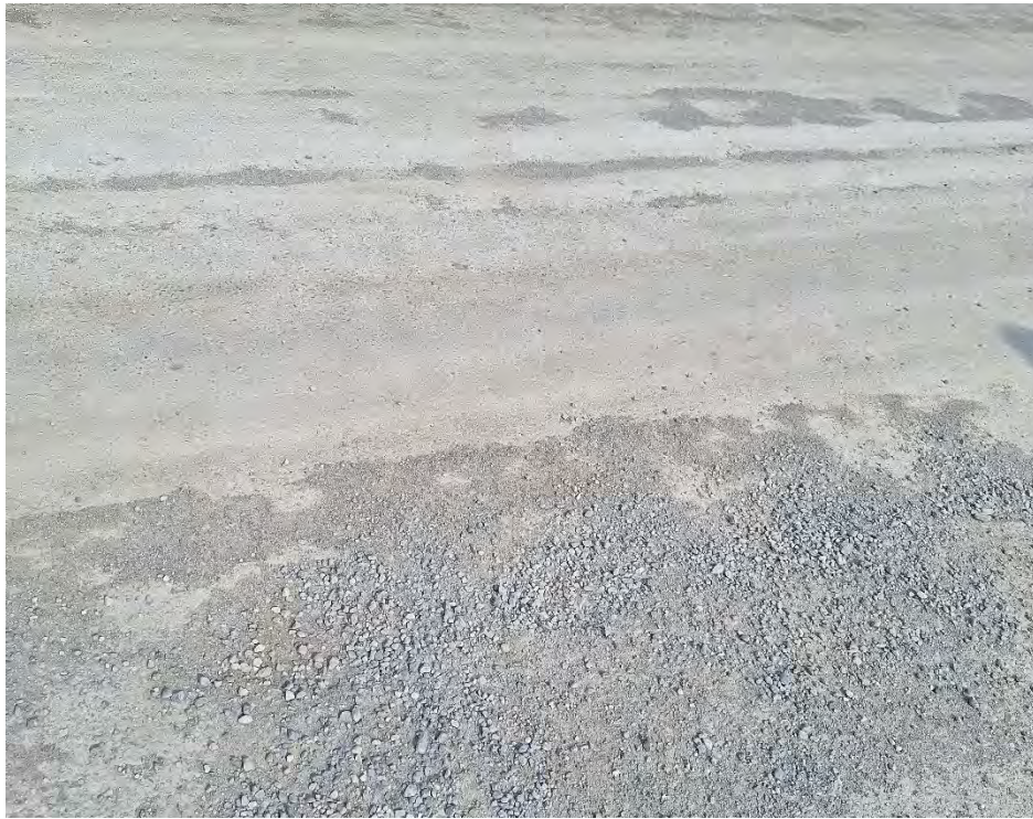
Figure 8 – Granular wearing surface
