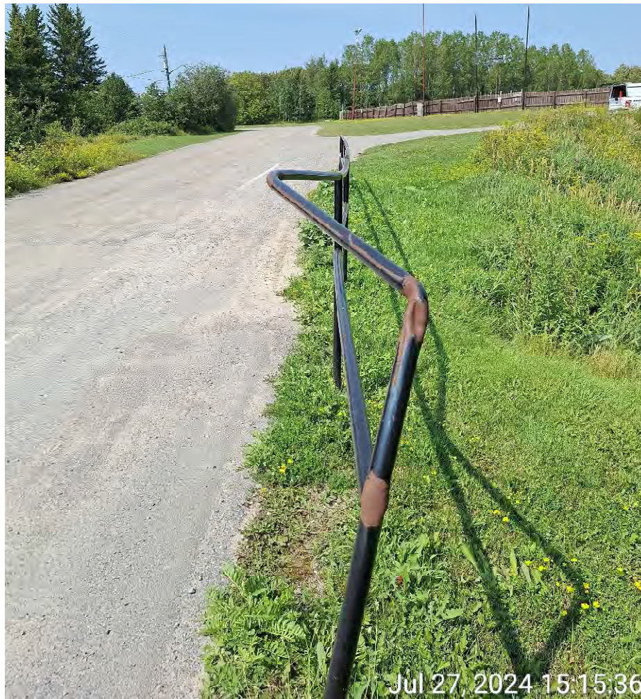
Figure 4: Bent hand rail
