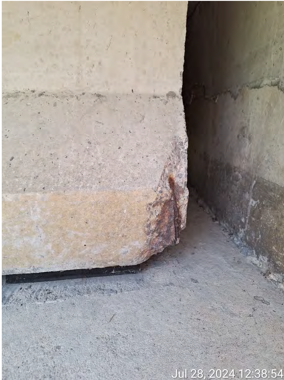
Figure 8: Spall on girder end with exposed and corroded reinforcing steel bar.
