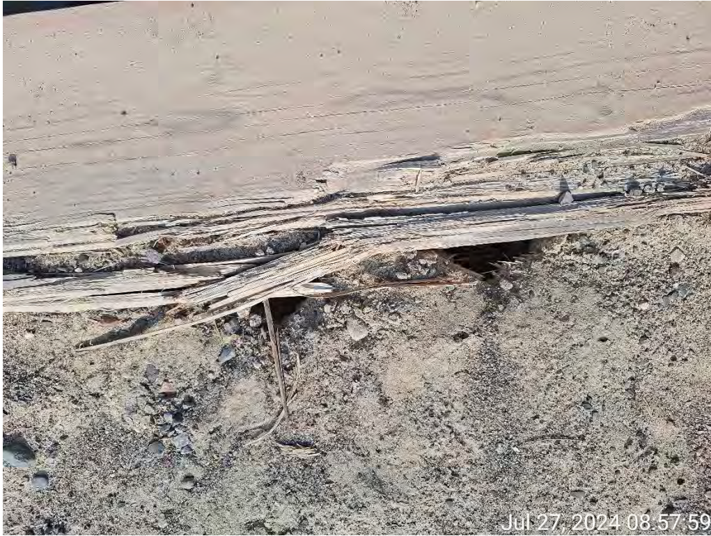
Figure 7: Damaged Timber Curb
