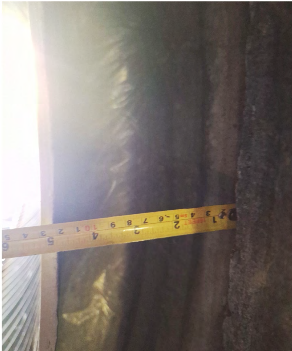
Figure 9 - Joint Gap on the side of the barrel
