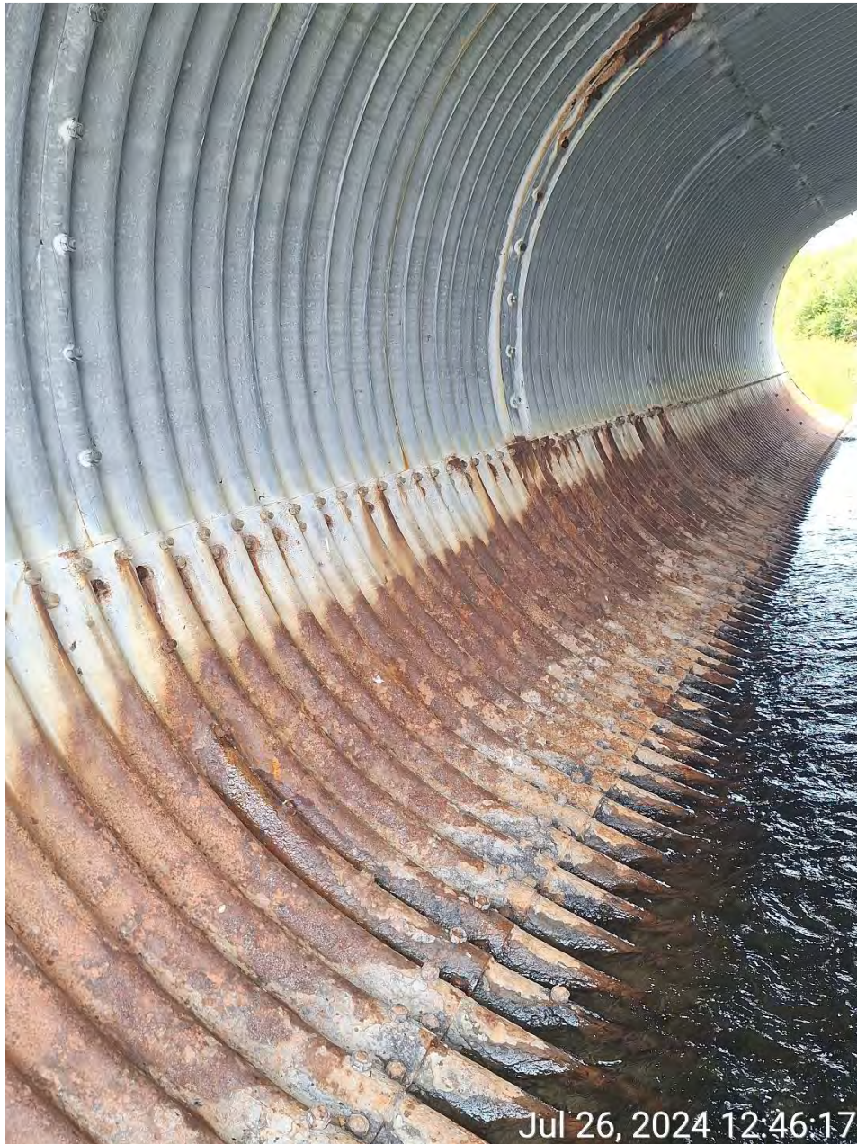
Figure 8: Culvert barrel showing corrosion and water level.
