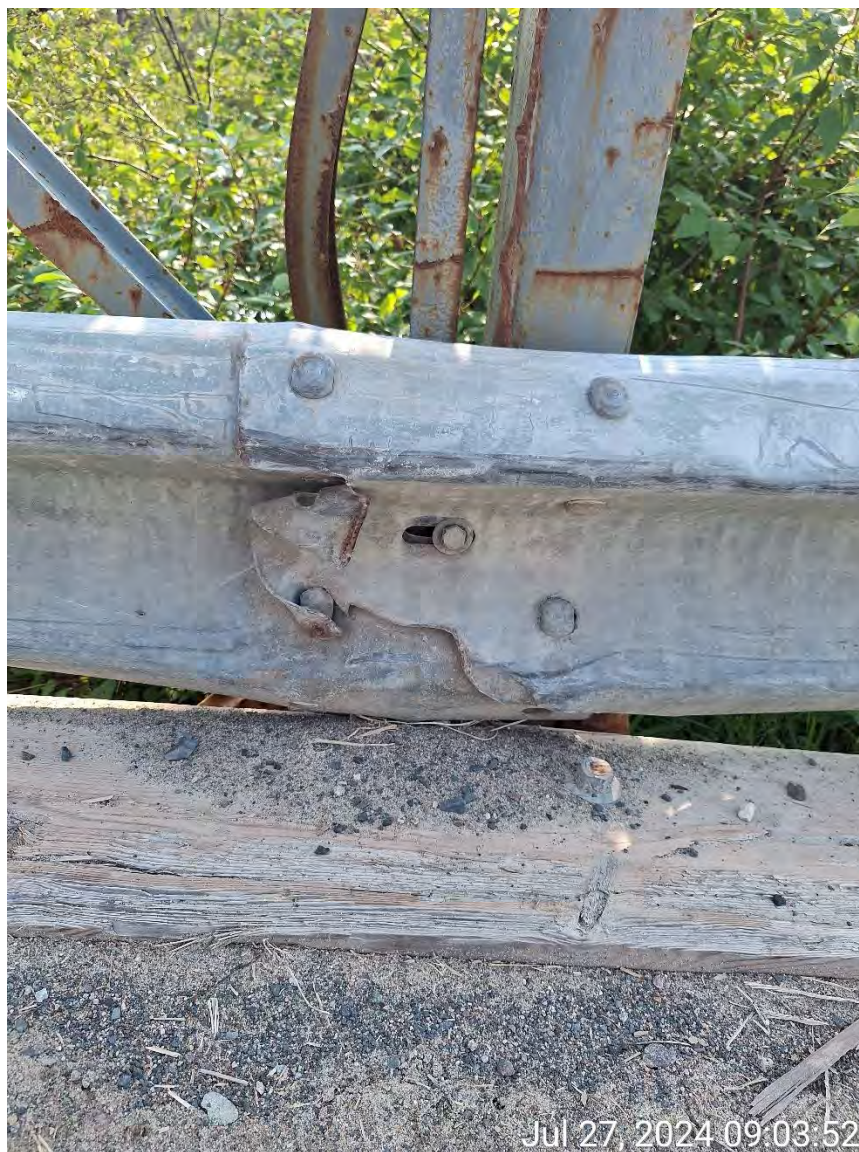
Figure 9: Damaged guide rail at connection point.
