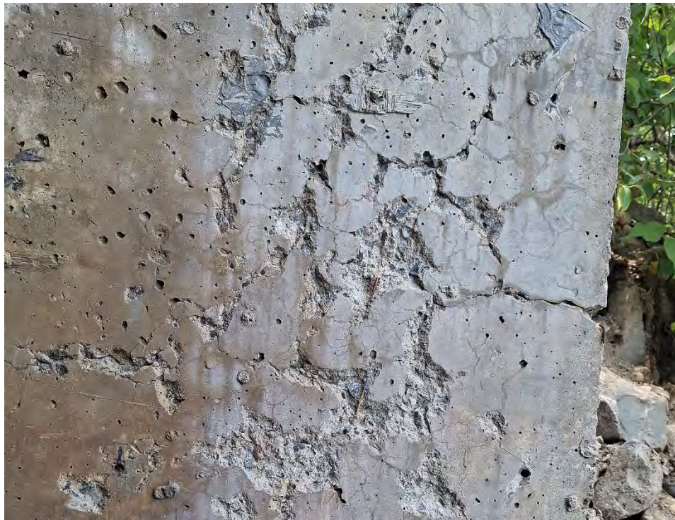
Figure 6 – deterioration and small spalls on culvert Barrel Wall
