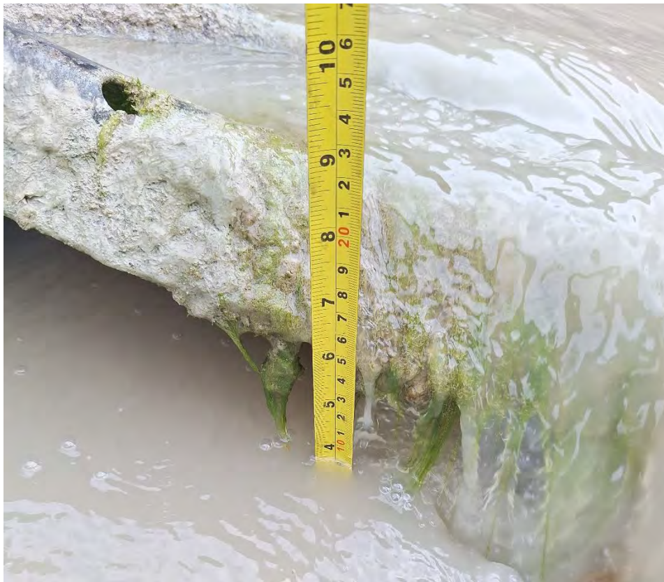
Figure 12 - Undermining At Outlet
