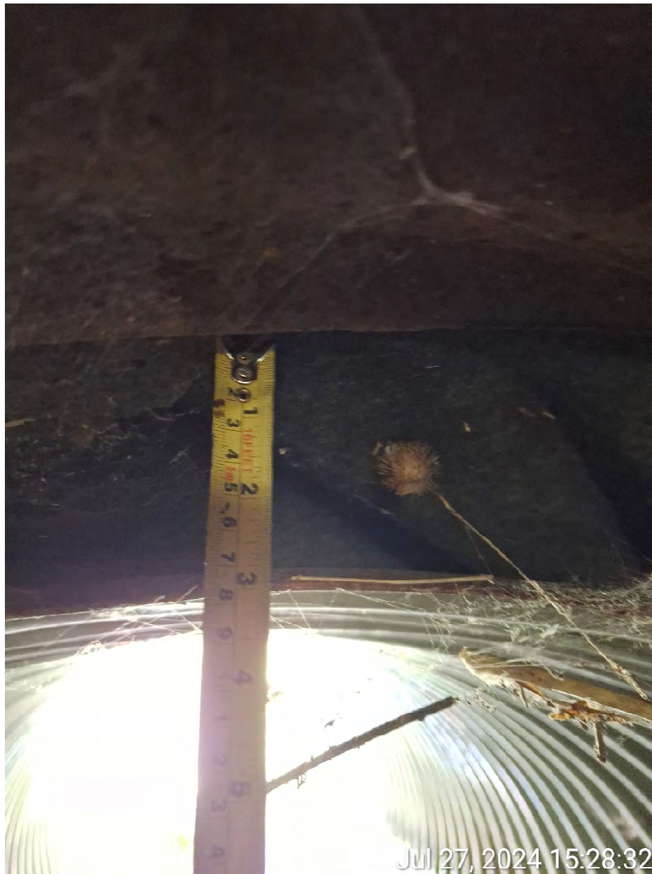
Figure 10: Gap at joint
