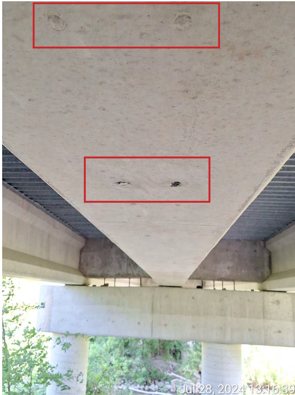
Figure 11: bottom of girder flange, small spalls and some spots that are likely to be future spalls.
