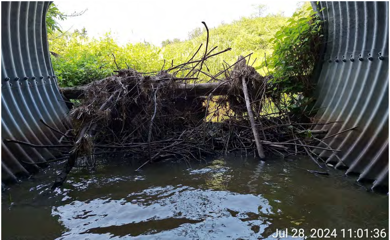
Figure 4 - Debris Buildup at Inlet – suspect beaver dam debris.
