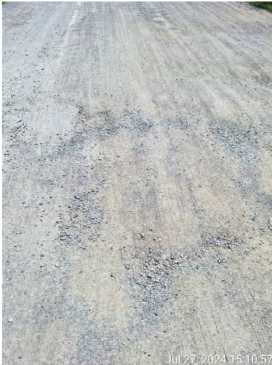
Figure 2: Pot holes in gravel wearing surface
