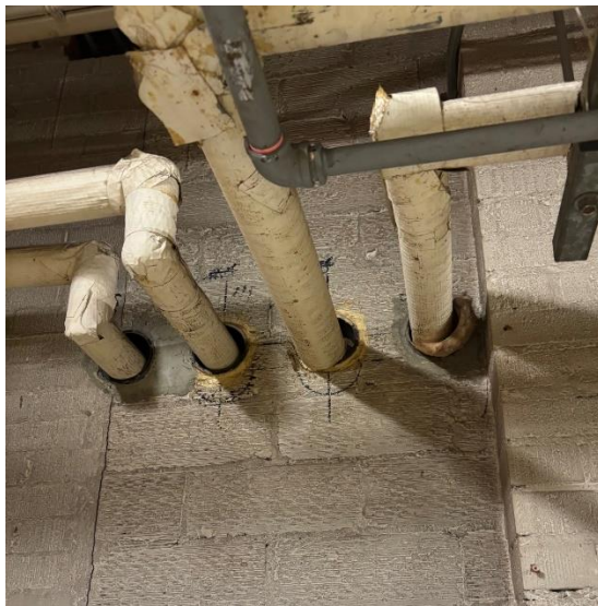
Figure 3 – Wall penetrations which were sealed on request of the TSSA.
