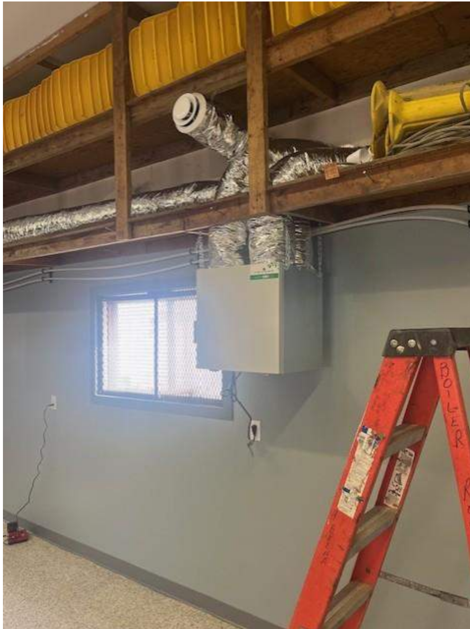
Figure 1 - City staff installed ERV's in the new Animal Pound
