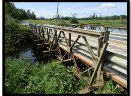
Poor to Failure (Firstbrooke Line Road Bridge)
