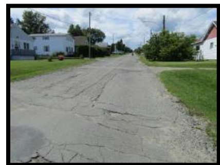
Poor to Failure (Albert Street Asphalt)
