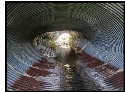
Poor to Failure (River Road Culvert)
