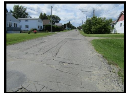
Poor to Failure (Albert Street Asphalt)
