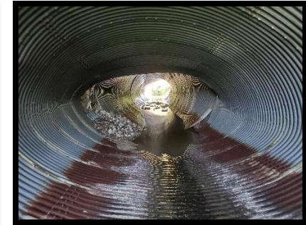
Poor to Failure (River Road Culvert)
