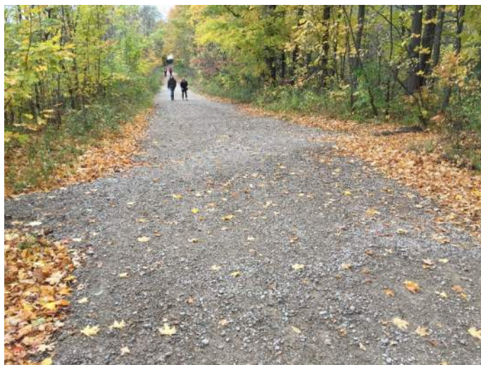
Figure 22 | Photo of rolling grade dip method to mitigate longitudinal slope rutting. Buried log used to create drain break hump (Mount Nemo, Burlington).
