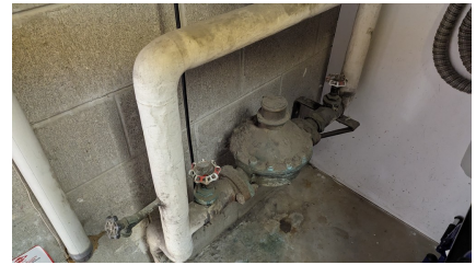
Figure 125: Water meter
