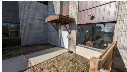
Figure 8: Hollow metal door
