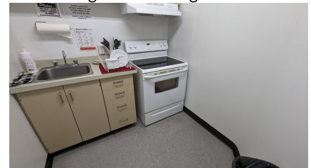
Figure 100: Stove and rangehood in the basement
