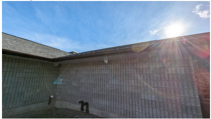
Figure 56: Supply and exhaust for HRV - 2
