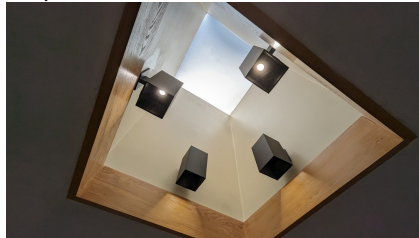
Figure 78: Type F - sconce fixtures with LED lamps
