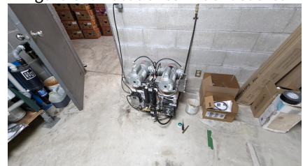
Figure 85: Dental air compressor
