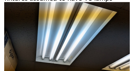
Figure 70: Type A4 - T12 lamps with a magnetic ballast
