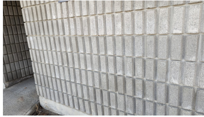
Figure 5: Concrete block exterior walls
