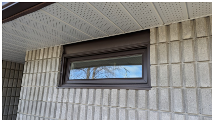
Figure 13: One of the five awning windows added in 2023
