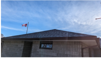
Figure 4: Asphalt shingled roof
