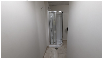
Figure 118: Shower in the basement
