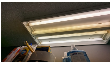
Figure 68: Type A2 - T12 lamps
