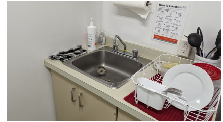
Figure 114: Kitchen faucet in the basement
