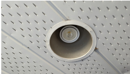
Figure 77: Type C - Soffit LED light
