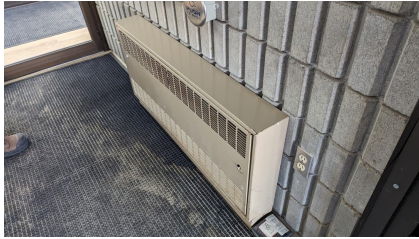
Figure 17: 5 kW electric heater with built-in thermostat
