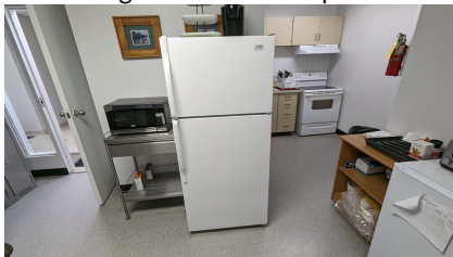
Figure 98: Refrigerator in the basement
