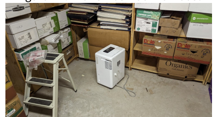
Figure 52: Portable dehumidifier in storage room
