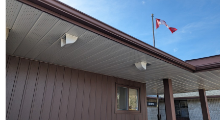
Figure 55: Supply and exhaust for HRV
