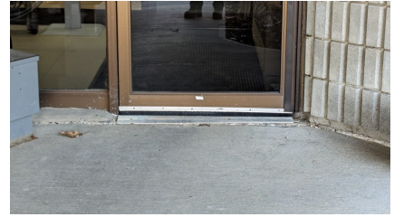
Figure 6: Door sweeps are in good condition
