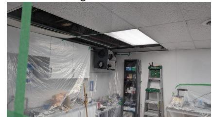
Figure 28: Additional HRV being installed in the old literacy area
