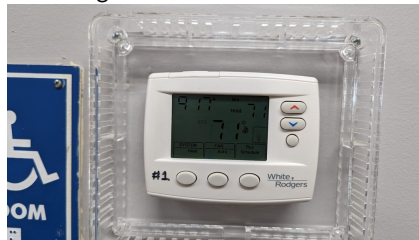
Figure 27: AC4 thermostat control
