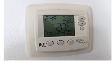
Figure 19: AC1 thermostat
