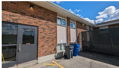
Figure 7: Brick and vinyl siding on the west elevation
