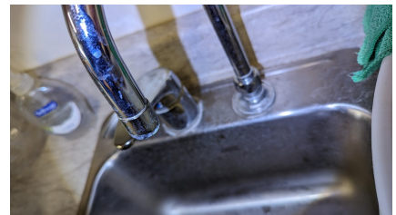
Figure 75: Kitchen sink with 2.2 gpm
