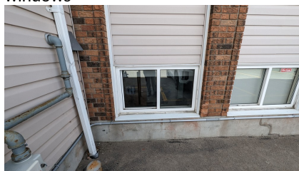
Figure 16: Vinyl window to the lower level
