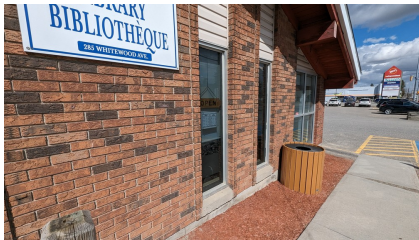
Figure 6: Aluminum-framed windows in lobby area
