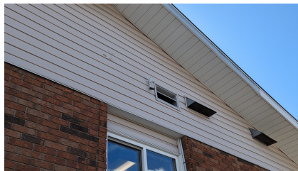
Figure 56: Photocell on the north elevation
