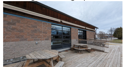
Figure 9: Hall windows and overhead door
