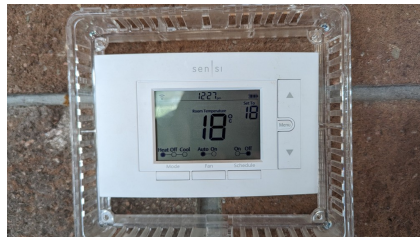
Figure 19: AC1 thermostat
