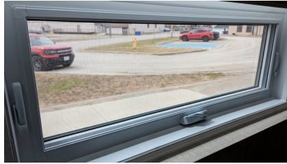
Figure 11: New window in room 27
