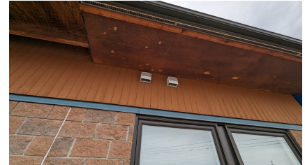
Figure 26: HRV1 Exhaust ports
