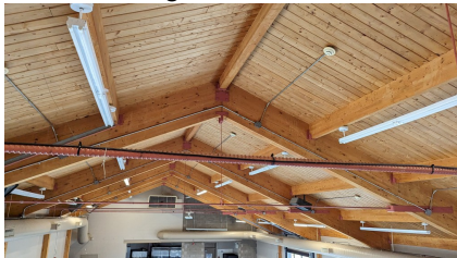
Figure 16: Underside of the roof of the hall
