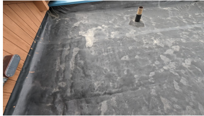
Figure 14: Roof above the kitchen
