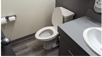
Figure 69: Toilet in radio washroom
