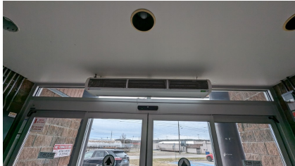
Figure 24: Air curtain
