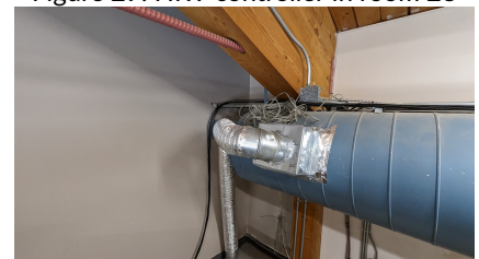
Figure 32: Modified ductwork to supply air to community hall washroom
