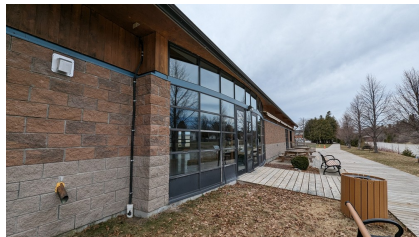
Figure 5: Curtain wall
