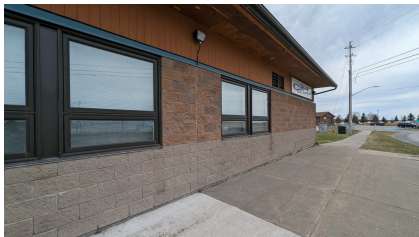
Figure 4: Brick and cedar siding
