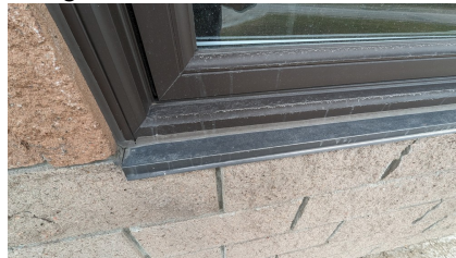
Figure 17: Window sealant in excellent condition
