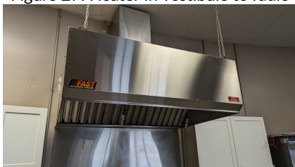
Figure 30: Kitchen exhaust
