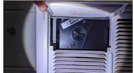
Figure 81: Type H - Electric heater control
