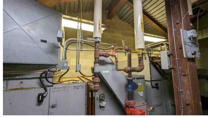
Figure 59: HV1 preheat valves are closed
