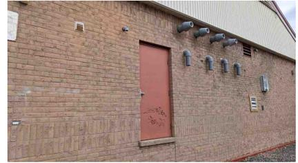
Figure 42: Boiler exhaust ports
