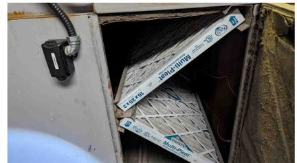
Figure 57: HV1 filters are in good condition
