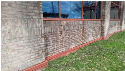
Figure 12: Moisture damage on the south elevation
