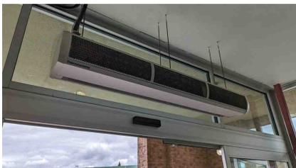
Figure 52: Front entrance electric air curtain
