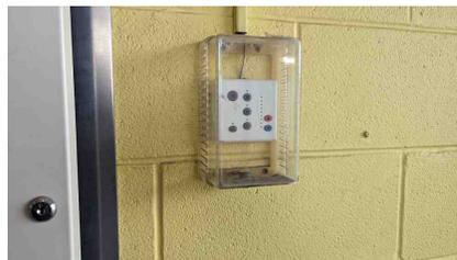
Figure 53: Front entrance electric air curtain controls
