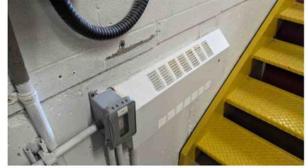
Figure 78: Type F - Electric heater
