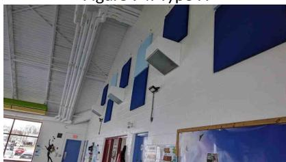
Figure 97: Type K - Natatorium fixtures that appear to be retrofitted with LED corn lamps
