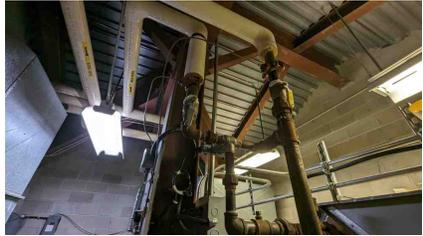
Figure 61: HV1 reheat shut off valves are open
