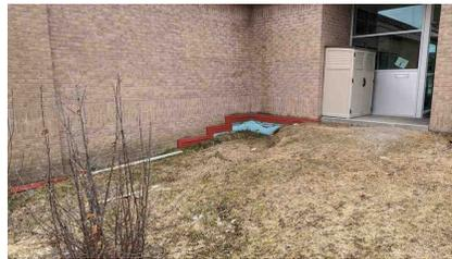
Figure 7: Exposed foundation insulation
