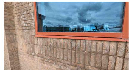
Figure 11: Missing caulking around partial window outside the pool area
