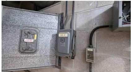
Figure 64: HV2 was removed but disconnect still present
