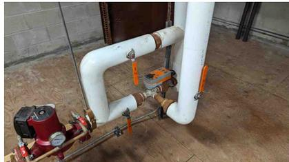
Figure 65: Heating supply valve is closed
