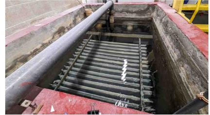
Figure 106: Pool filtration tank
