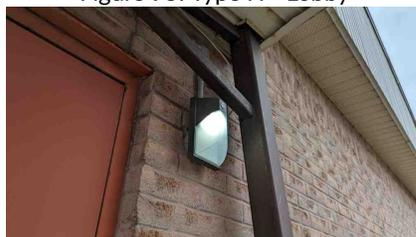
Figure 98: Type O - With integrated photocell
