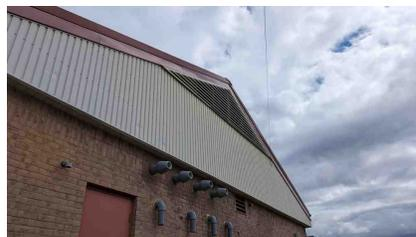
Figure 10: Metal siding on the west elevation with outdoor air louvre
