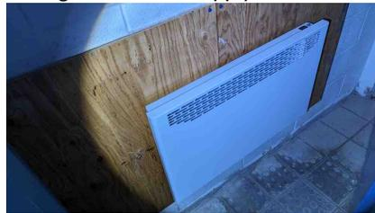
Figure 50: Electric heater in vestibule to natatorium
