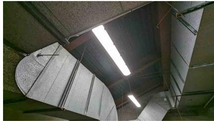
Figure 86: Lighting in pool mezz has been replaced with LED
