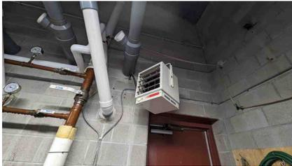
Figure 82: Unit heater in the boiler room
