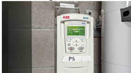
Figure 71: P5 VFD
