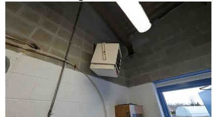
Figure 51: Electric unit heater in the pool mechanical room
