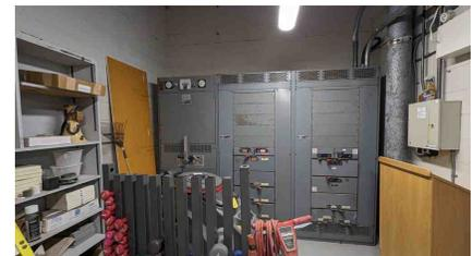
Figure 131: Main switchboard
