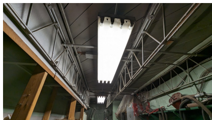
Figure 99: A - Type H - 4 lamp fluorescent
