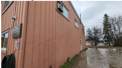
Figure 19: A - Metal siding
