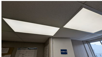
Figure 92: A - Type B - LED 2x4 flat panel
