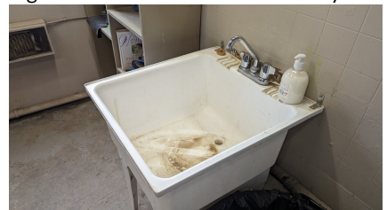
Figure 146: C - Laundry sink
