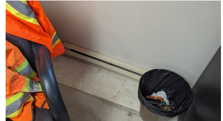
Figure 61: A - Electric baseboard heat in the back office
