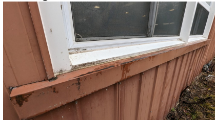
Figure 23: A - Seals on windows are in fair condition
