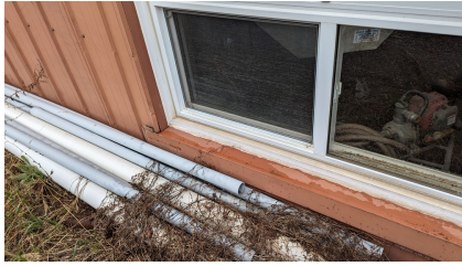
Figure 29: B - Window seals are in fair condition
