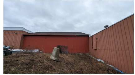
Figure 30: Back of the salt storage
