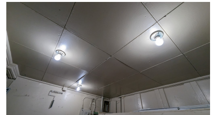
Figure 112: C - Type P - LED lamps
