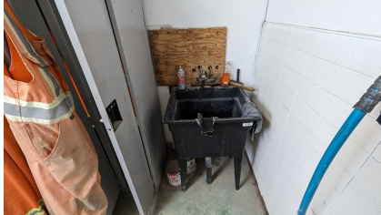
Figure 142: B - Laundry sink
