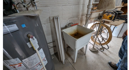
Figure 143: B - Second-floor laundry sink
