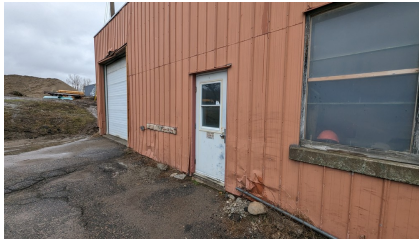
Figure 35: C - Loader bay and entrance doors
