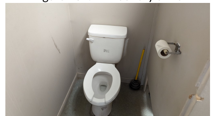
Figure 137: A - Lunchroom washroom toilet
