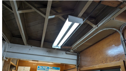
Figure 105: B - Type K - T12 fixture
