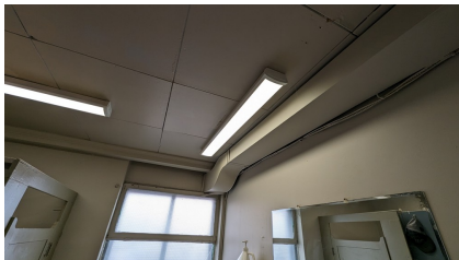
Figure 110: C - Type N - LED strip light
