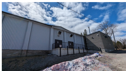
Figure 54: Exhaust fans for the arena
