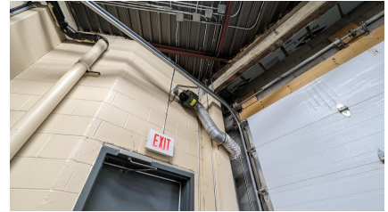
Figure 43: EF06 - ice resurfacers room
