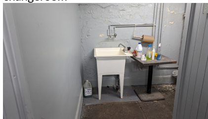
Figure 164: Washroom sink for 54s changeroom
