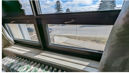
Figure 10: Awning window in the palette and brush room
