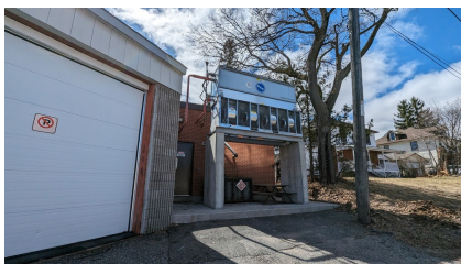
Figure 124: Evaporative condenser
