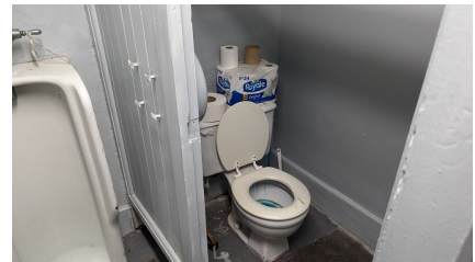
Figure 159: Toilet - 54s changeroom
