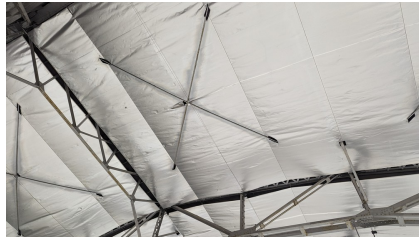
Figure 134: Low emissivity room over ice rink
