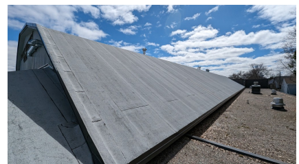
Figure 23: Roof over the arena
