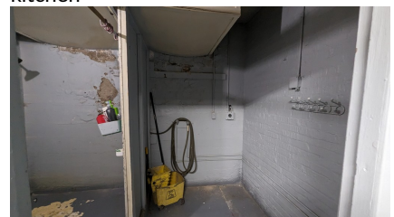
Figure 126: former area of washer and dryer in 54s
