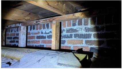
Figure 9: Attic above the Open Studio Libre
