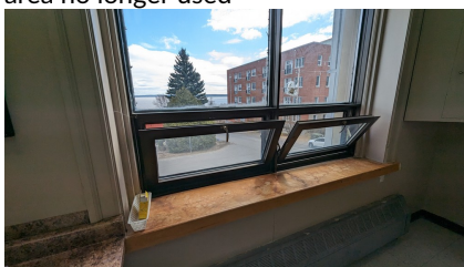
Figure 86: Windows open in the 2nd floor women's washroom
