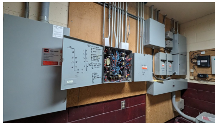
Figure 92: Lighting controls
