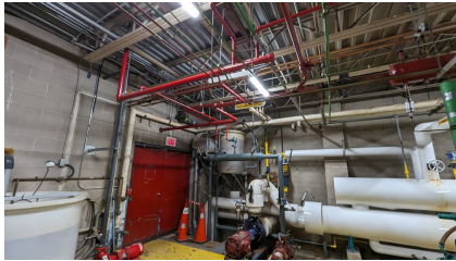
Figure 130: HX2 - for underfloor heating
