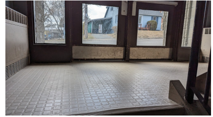
Figure 11: Doorsweep replacement of the southwest entrance required
