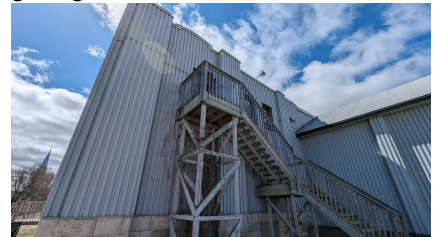
Figure 17: Fire exit for the Studio Libre
