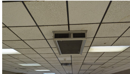
Figure 66: RTU1 - return
