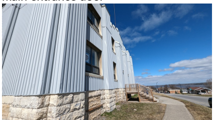
Figure 21: Metal siding
