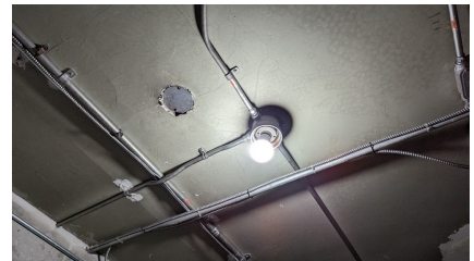
Figure 96: Type A - standard socket with LED lamp
