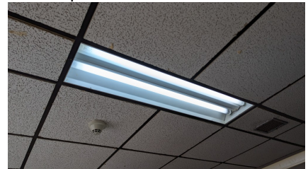
Figure 99: Type C1 - T12 lamp
