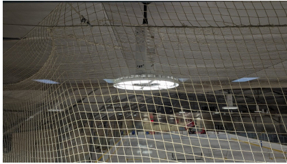
Figure 103: Type F - high bay LED
