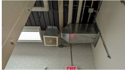
Figure 41: EF04 - changeroom hallway
