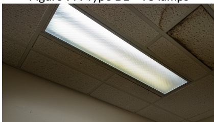
Figure 100: Type C - T8 lamps
