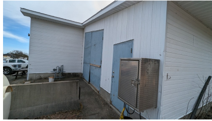
Figure 5: Doors to the cold storage area
