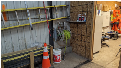
Figure 54: Former sink retrofitted with a garden hose
