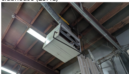
Figure 28: UH2 - mothballed
