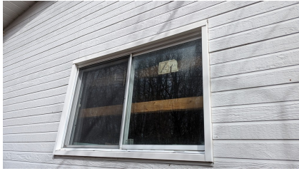
Figure 4: Aluminum framed window
