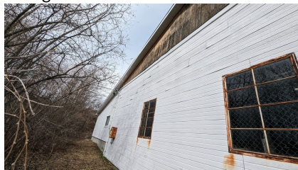
Figure 17: Windows on the south elevation appear original to the building
