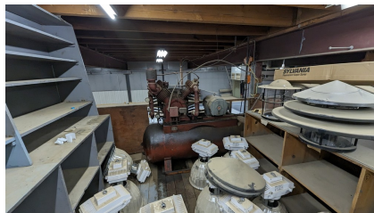
Figure 43: Air compressor
