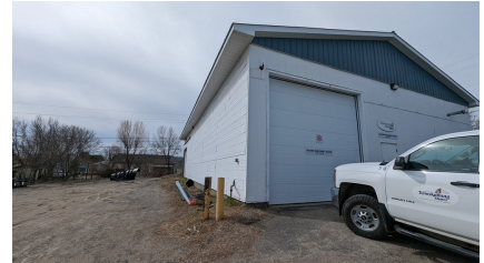
Figure 12: Overhead door on the north elevation
