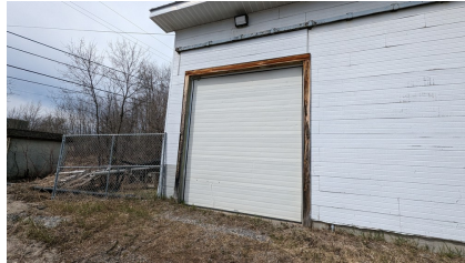
Figure 11: Overhead door on the east elevation
