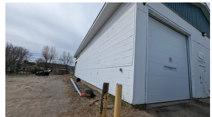
Figure 18: Wood siding
