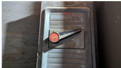
Figure 65: Main disconnect
