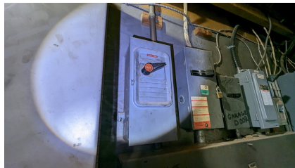
Figure 62: Compressor disconnect
