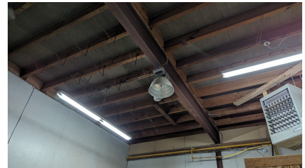
Figure 15: Underside of roof
