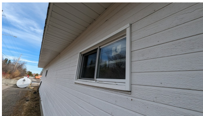
Figure 16: Windows on the cold storage side
