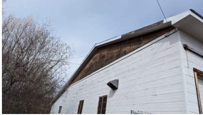
Figure 7: Gable end has exposed siding on the south elevation
