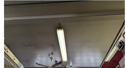
Figure 58: Type G - Bays 4 and 5
