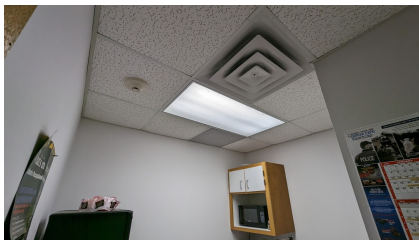
Figure 50: Type D - 2x4 fixture
