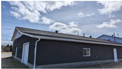
Figure 4: Asphalt shingle roof
