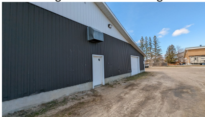
Figure 16: Overhead door to storage and entry door
