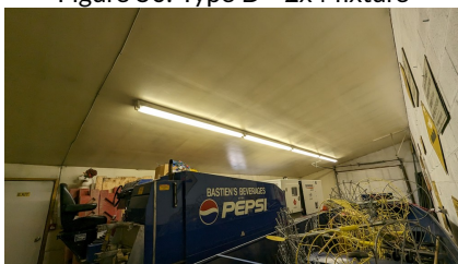
Figure 53: Type E1 - T12 lamps
