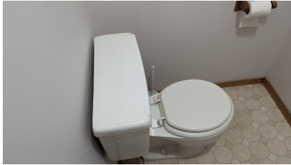
Figure 92: Toilet - Fire station office washroom
