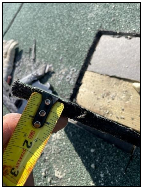
Coverboard and Cap Sheet
