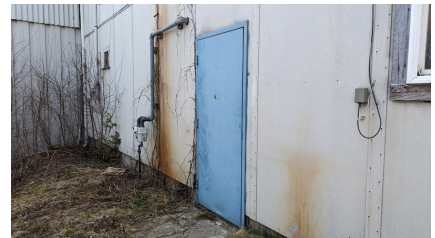
Figure 12: Hollow metal door on north elevation
