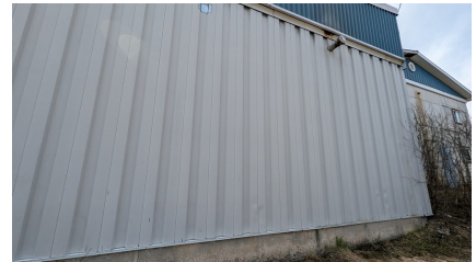
Figure 15: Metal siding on the east elevation
