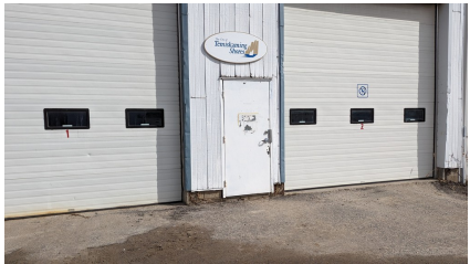
Figure 13: Hollow metal door
