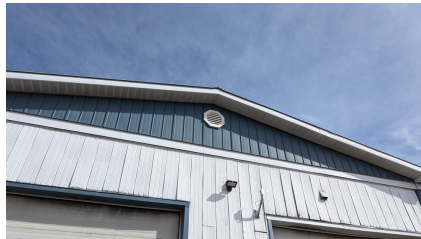
Figure 14: Metal siding on gable end
