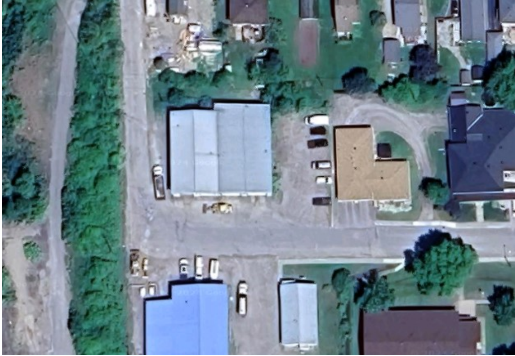
Figure 3: Haileybury Public Works Garage aerial view
