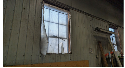
Figure 21: Windows from mechanic shop
