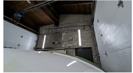
Figure 86: Type H - LED wall-mounted
