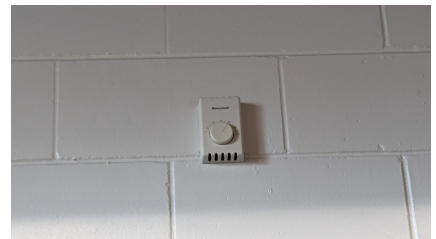
Figure 31: EF03 - thermostat
