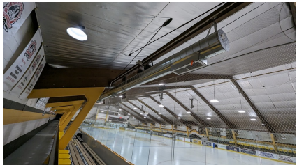
Figure 23: Bleachers ductwork
