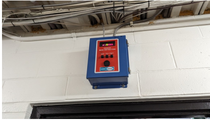
Figure 100: Ammonia gas detector
