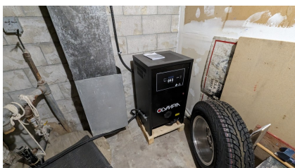
Figure 115: Ice resurfer charger
