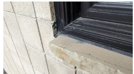
Figure 15: Office window seals in good condition
