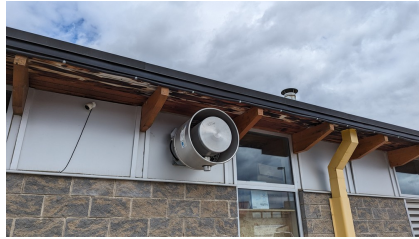
Figure 36: EF05 - Storage room
