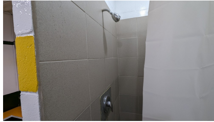
Figure 138: Shower in changeroom 5
