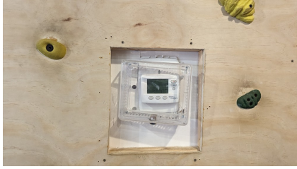
Figure 71: UH05 - thermostat not on
