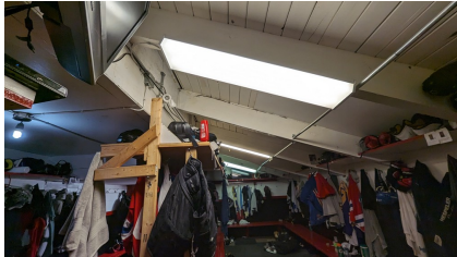
Figure 87: Type I - 2x4 fixture
