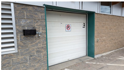
Figure 16: Overhead door
