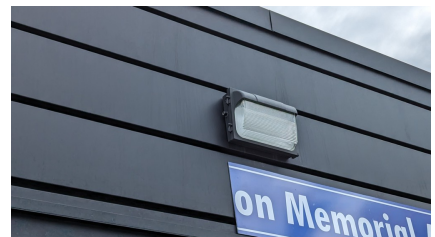
Figure 98: Type T - LED wall pack
