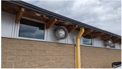
Figure 35: EF04 - from the exterior
