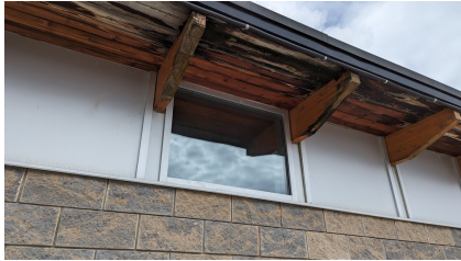
Figure 7: Aluminum-framed windows for south changerooms
