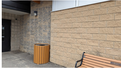
Figure 8: Concrete block from original and addition
