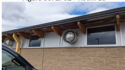
Figure 33: EF03 - from the exterior
