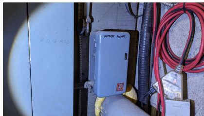
Figure 76: Exterior lighting control
