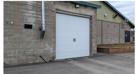
Figure 12: Ice resurfacers overhead door
