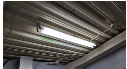
Figure 80: Type B - T8 fluorescent
