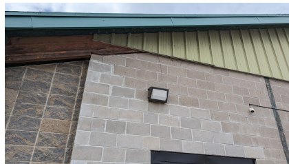
Figure 94: Type P - wall pack light
