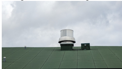
Figure 39: EF08 - ice rink exhaust
