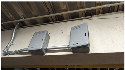
Figure 41: EF11 and EF12 timers
