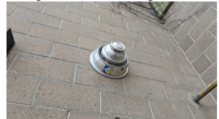
Figure 40: EF09 - ice surfacer room exhaust
