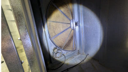
Figure 43: Heat wheel motor on ERV1
