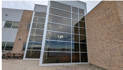
Figure 7: The curtain wall on the east elevation
