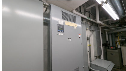
Figure 134: Transfer switch
