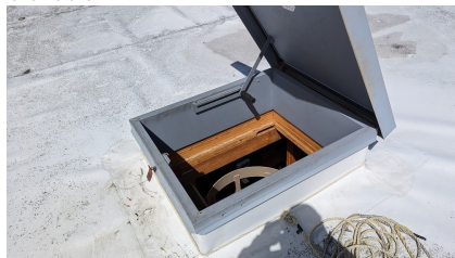
Figure 16: Roof hatch for access to Northern roof
