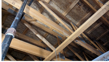
Figure 19: Underside of the roof
