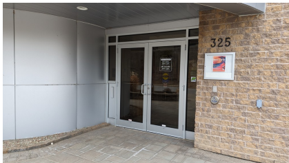
Figure 9: Front entrance doors with glazing
