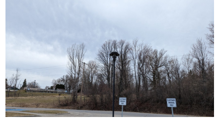
Figure 107: Type J fixture in the parking lot
