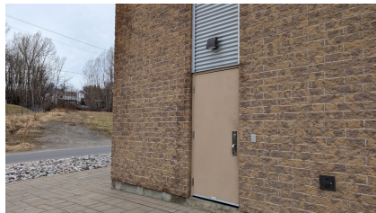
Figure 10: The hollow metal door on the south elevation
