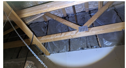
Figure 11: Insulation above the ceiling in the Receiver room
