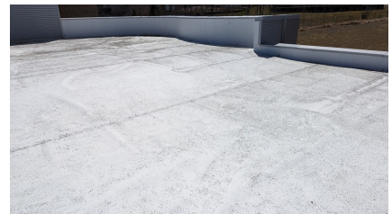
Figure 17: The roof membrane on the north section
