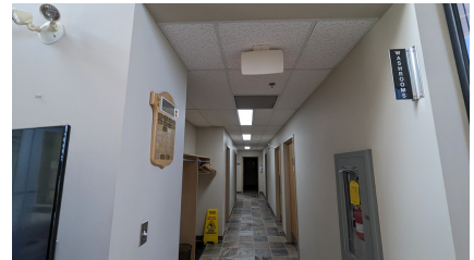
Figure 98: Type C fixture in the north corridor
