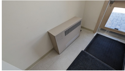
Figure 49: Hydronic cabinet heater
