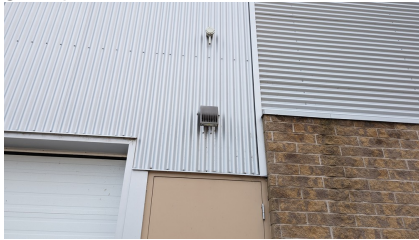
Figure 108: Type L fixture on the north elevation
