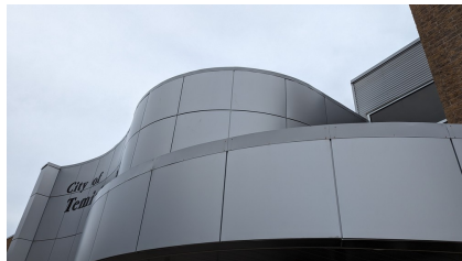
Figure 13: Metal panelling on the west elevation
