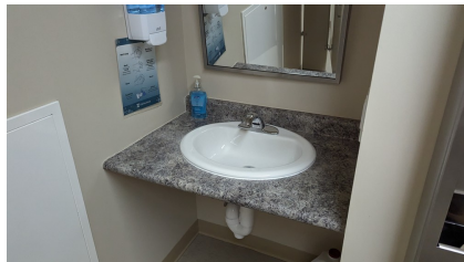
Figure 119: Motion-activated handwashing faucet
