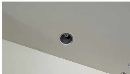
Figure 103: Type G fixture on the second floor
