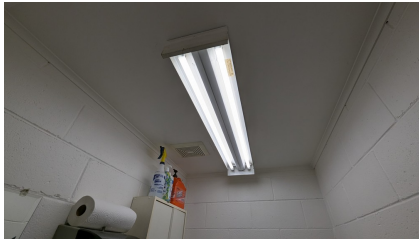
Figure 47: Type B - surface-mounted T8 fluorescent fixture
