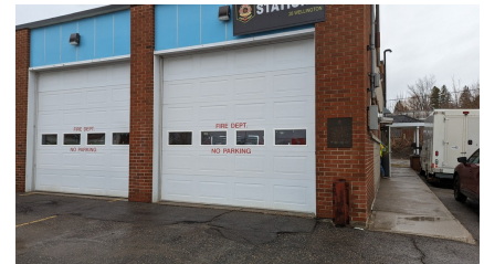
Figure 13: Overhead bay doors
