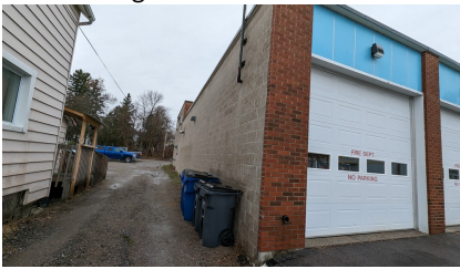
Figure 8: Concrete block wall along the south elevation
