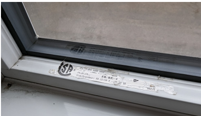
Figure 11: Nameplate information for typical window
