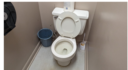
Figure 73: Toilet in the upstairs washroom
