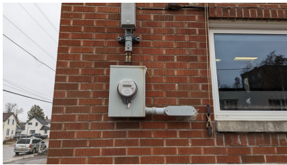
Figure 76: Electric meter
