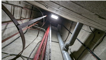
Figure 48: Type C - hose tower fixture
