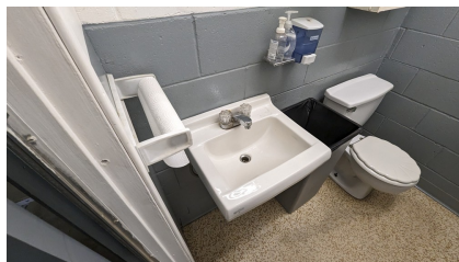
Figure 72: Sink in washroom adjacent to the firehall
