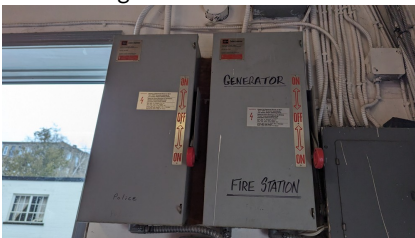
Figure 82: Transfer switch
