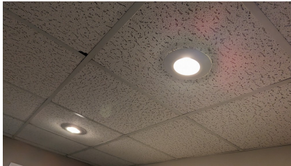
Figure 50: Type D - pot lights with CFL lamps
