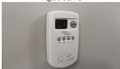
Figure 34: Thermostat assumed to control F2
