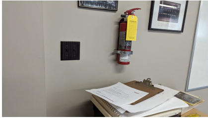
Figure 41: Manual switches for lights on the second floor
