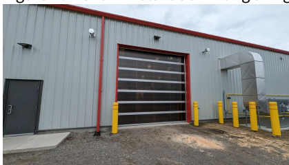
Figure 10: Overhead door at the rear
