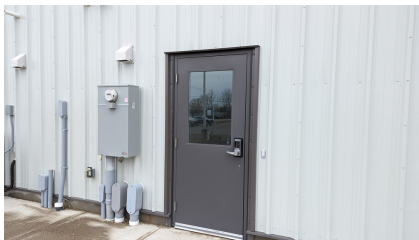
Figure 7: Hollow metal door with glazing
