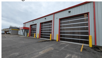
Figure 11: Overhead doors at the front
